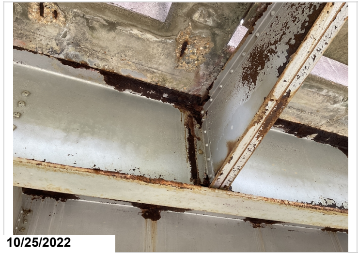
Span 6, Girder 1, 3rd Sidewalk Support: 1 missing bolt and top bolt sheared.
