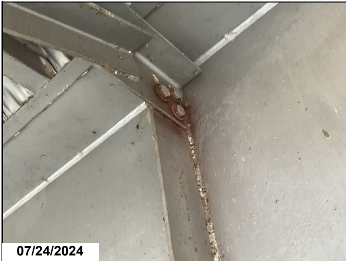
Span 5, girder 2, dia 4: loose bolts.
