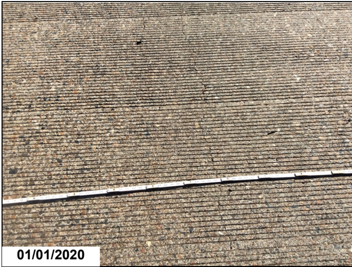
Span 8, longitudinal & transverse cracks up to .020".
