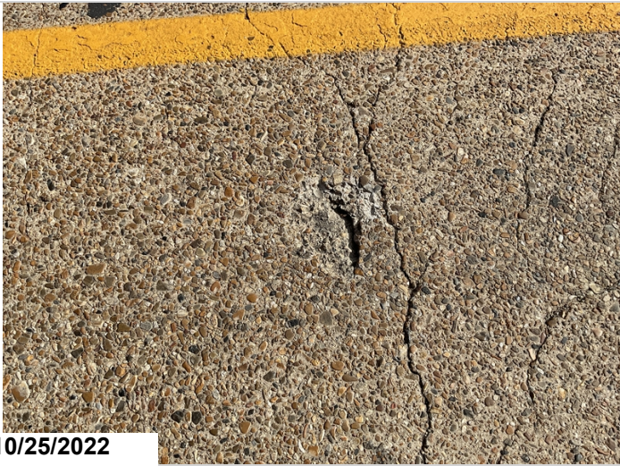
Span 1: Spalling.
