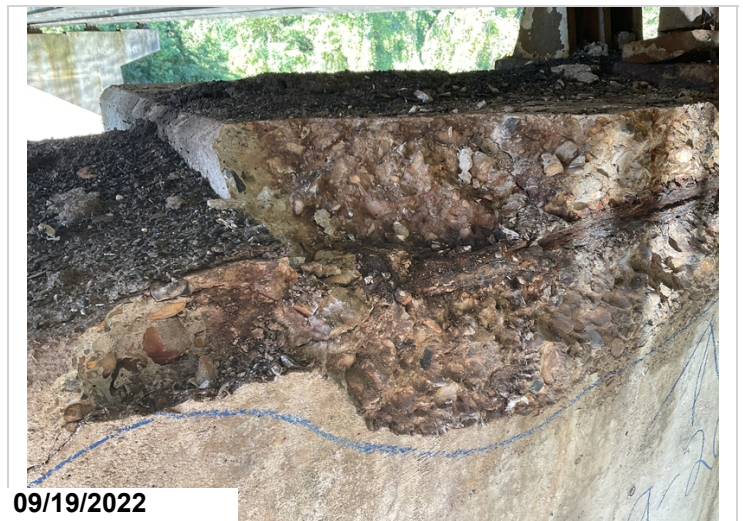
Main span, Pier 2, Rebar exposed near bearing area, CS3
