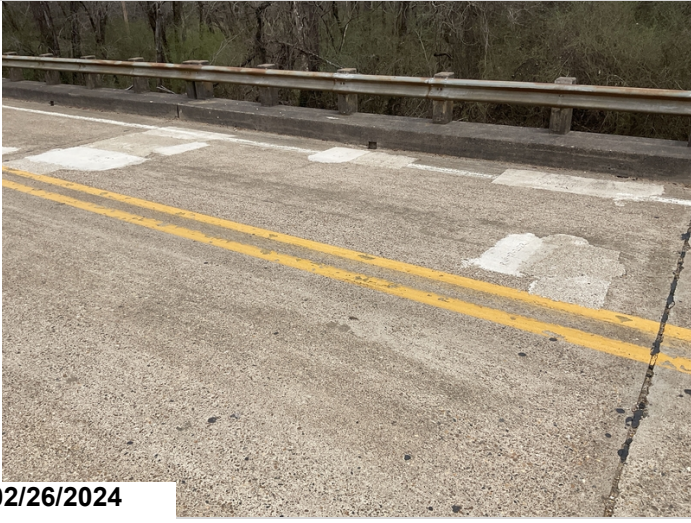
Approach span 15, Northbound lane, Patched areas, CS2
