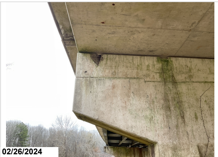
Main span, Pier 1, Looking ahead, Rebar exposed to left side of cap, 1 LF, CS3
