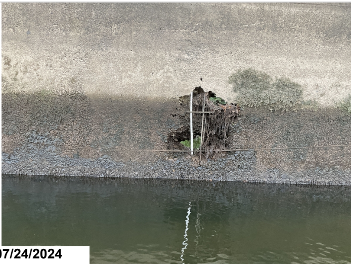
Pier 5: at the centerline of the pier a large spall with exposed rebar that is believed to be a previous location for utility pipe.
