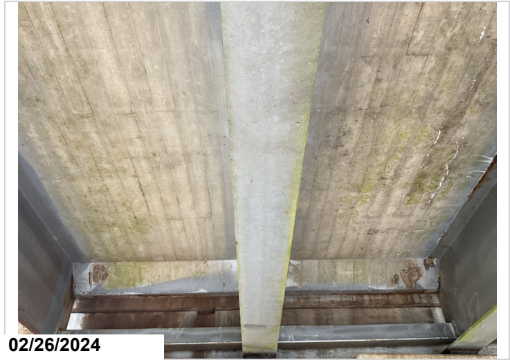
Main span 1, Beam 4, Corrosion to bottom flange, 2 Sq Ft, CS2
