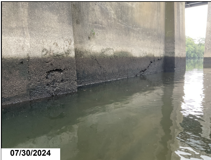
Backside Pier 2: 8' severe abrasion has created spalls CS3-5'
