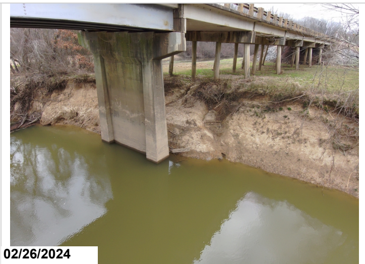
Erosion around pier 4
