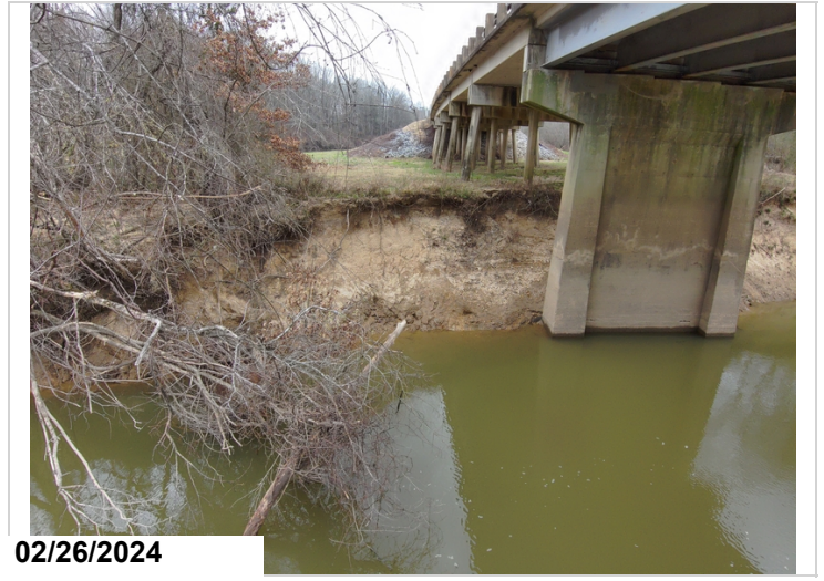
Erosion around pier 4
