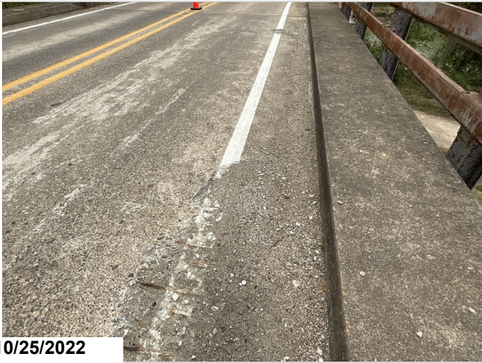
Span 17: Spalling with exposed reinforcing steel with section loss.
