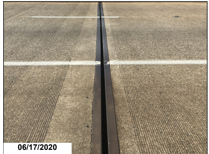
Pier 4, missing joint seal.
