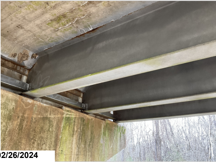
Main span 1, Beam 3, Corrosion to bottom flange, 2 Sq Ft, CS2
