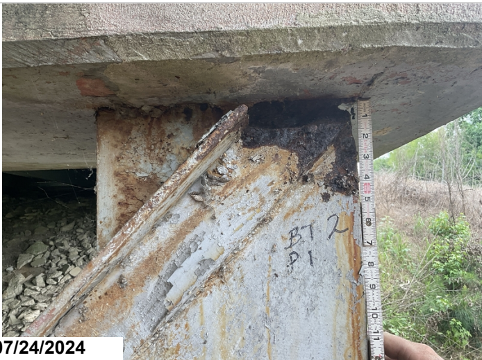
Bent 2, pier 1: the flange has a 1/2' hole on the edge and approximately 4" of section loss up to 3/16" adjacent to the cap. CS3-1
