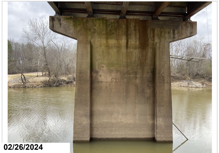
Main span, Pier 2, Looking ahead, Rebar exposed, CS2
