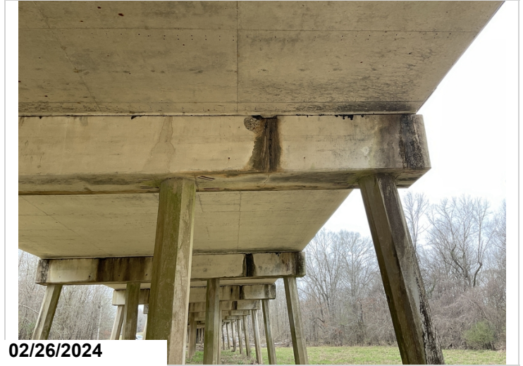
Approach span, Bent 13, Pier Cap, Looking back, Spalling between piles 1 & 2, 1 LF, CS2
