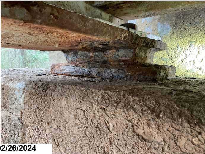
Main span 1, Pier 1, Bearing 5, Active corrosion, CS3
