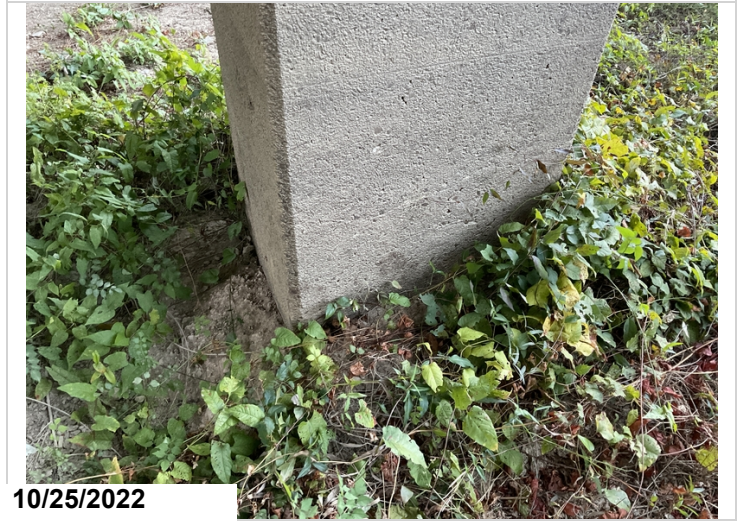
Bent 2, Column 2: Cracking.
