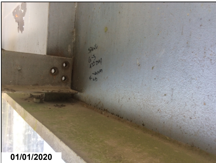
Span 6 girder 3 4th diaphragm has missing bolts
