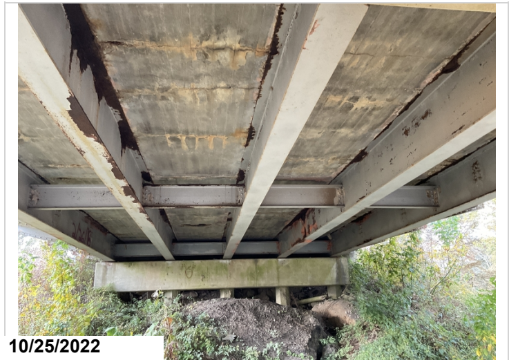
Span 1: Typical active corrosion with section loss on top flanges.
