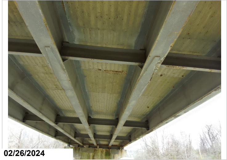
Welded cover plates on steel beams
