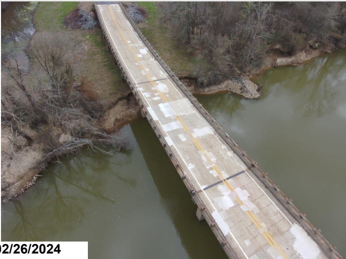
Main span, Deck Patching, CS2 & CS3
