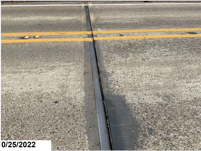
Bent 16, Joint: Loss of adhesion.
