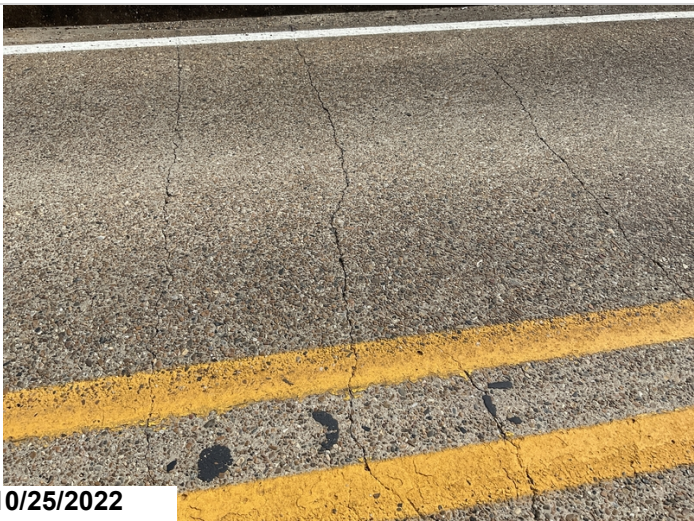
Typical cracking.
