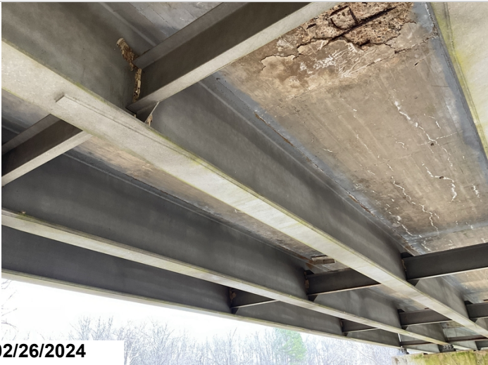
Welded cover plates
