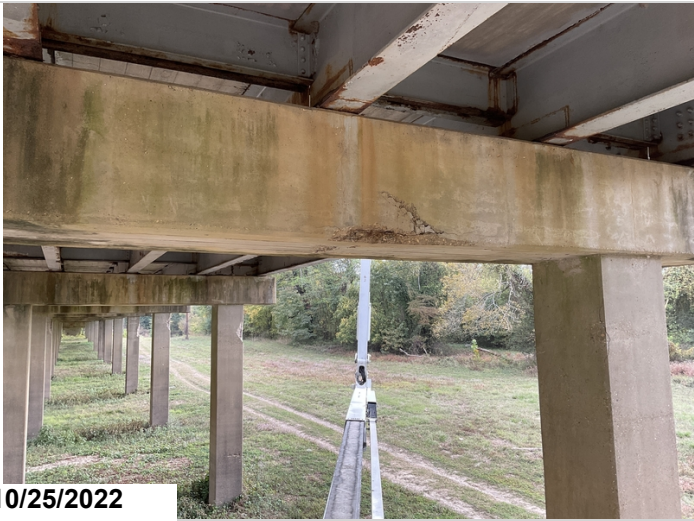
Bent 4, Back, Girder 3: Spalling with exposed reinforcing steel with section loss.
