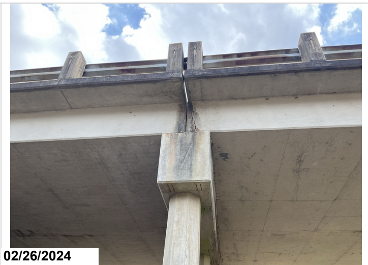
Approach span, Bent 28, Delam on left side, CS3
