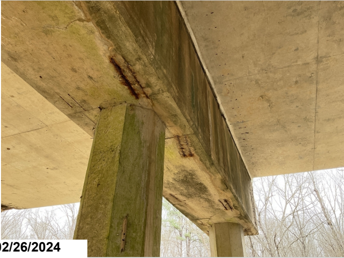
Approach span, Bent 2, Pier Cap, Exposed rebar on underside of cap, CS2
