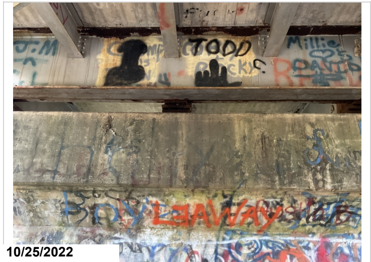
Pier 4, Back: Spalling with exposed reinforcing steel with section loss.
