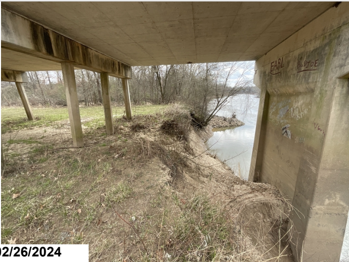
Scour around Pier 4, Scour is approximately 8' from reaching Bent 25 pile
