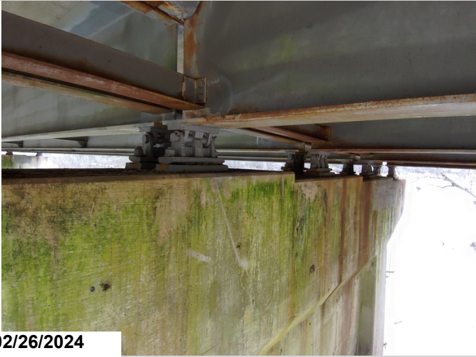
Bearings at pier 2
