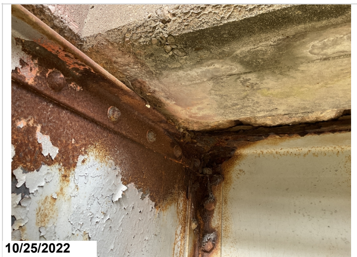
Span 6, Top Flange @ Sidewalk Supports: Active corrosion with knife edge section loss.
