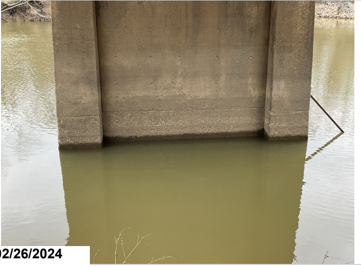
Main span, Pier 2, Looking ahead, Abrasion to both columns 1 & 2, CS2
