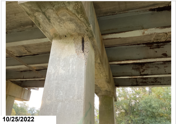
Bent 14, Column 1: Spalling with exposed reinforcing steel with section loss.
