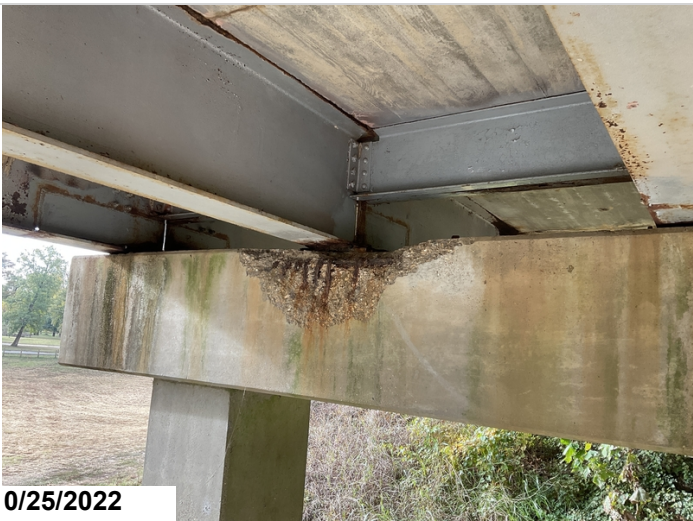
Bent 2, Ahead, Girder 4: Spalling with exposed reinforcing steel with section loss.
