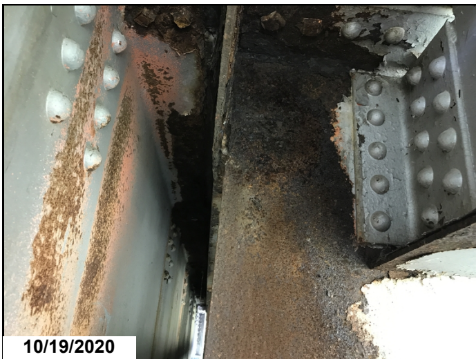
Pier 4 (AHD) has approximately 1/4" section loss
