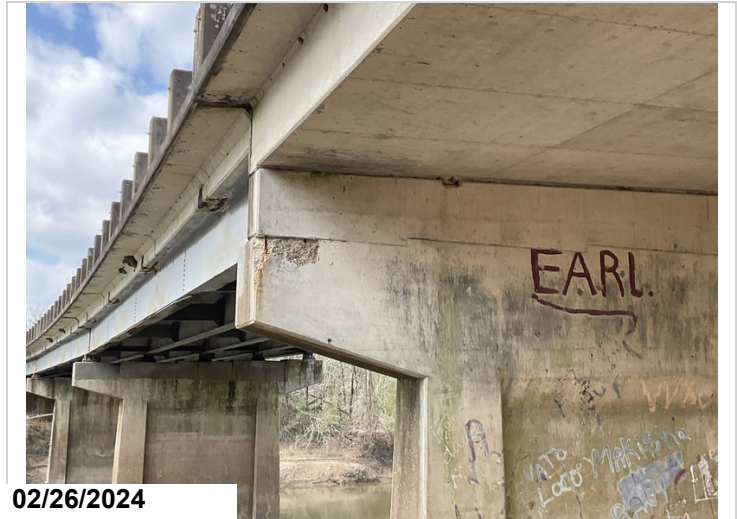
Main span, Pier 4, Looking back, Cracking on right side, 1 LF, CS2
