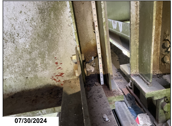
Girder 4: 3"x 3" hole in the web between the stiffeners above the bearing at pier 2. CS4-1'
