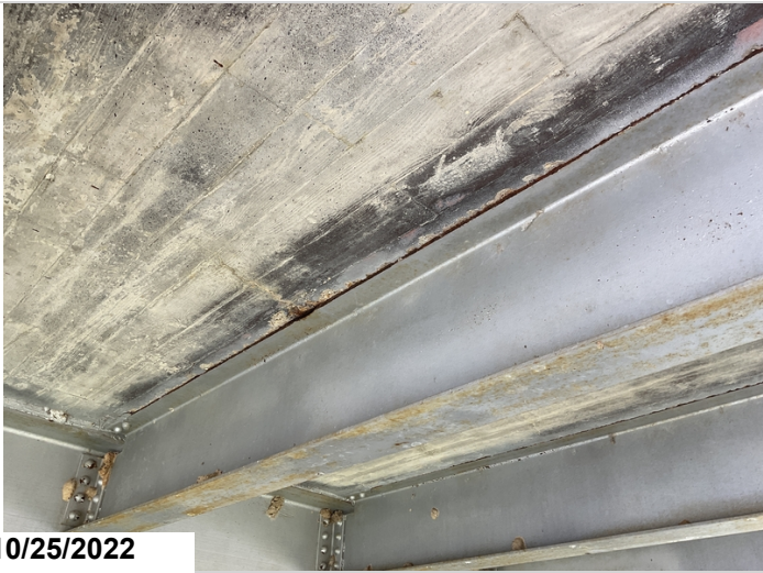
Typical minor active corrosion on top flanges.
