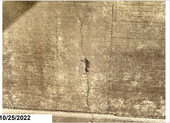
Pier 2, Back: Spalling with exposed reinforcing steel with section loss.
