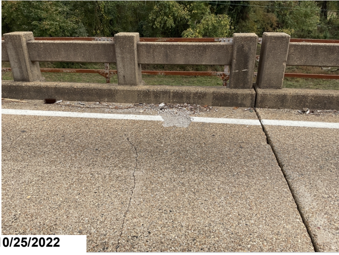
Span 9, Right: Spalling.
