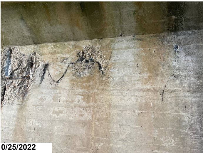
Pier 1, Ahead: Spalling.
