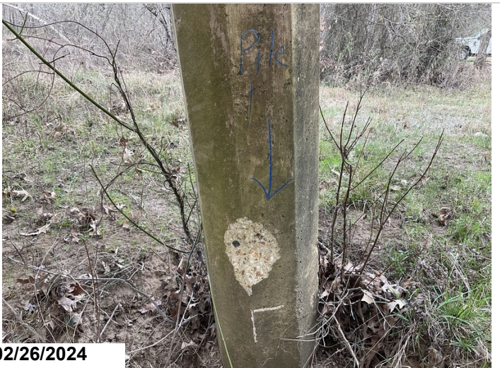
Approach span, Bent 24, Spall on pile 1, CS2
