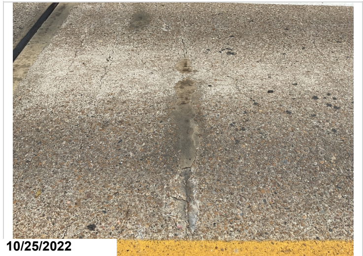
Truss Span 3: Spalling with exposed reinforcing steel with section loss.
