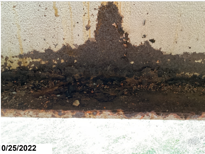
Span 1, Girder 4 & 5: Active corrosion with section loss in bottom flange. Approximately 6' back of Bent 2.
