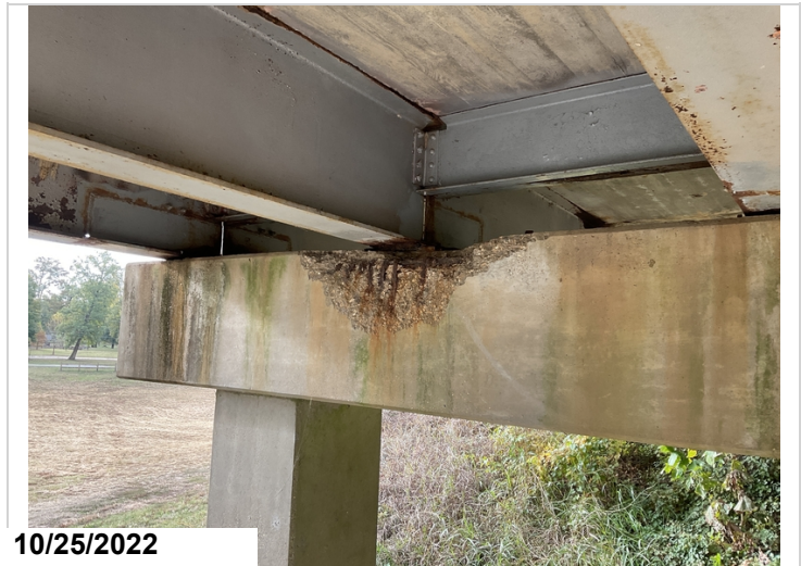
Spalling on each side of exposed reinforcing steel.
