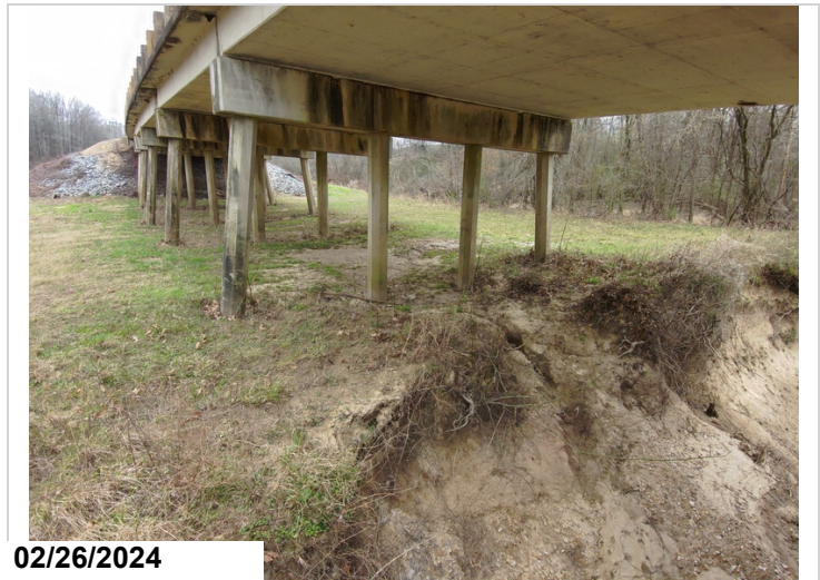
Erosion between pier 4 and bent 24
