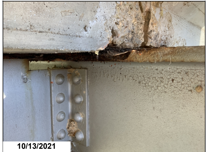
Span 16 Floor beam 5 Knife edge section loos.
