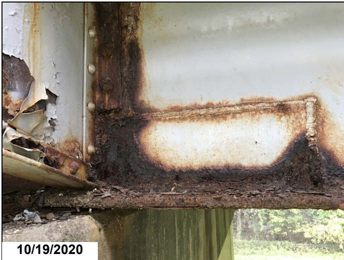
Typical corrosion along the beam ends
