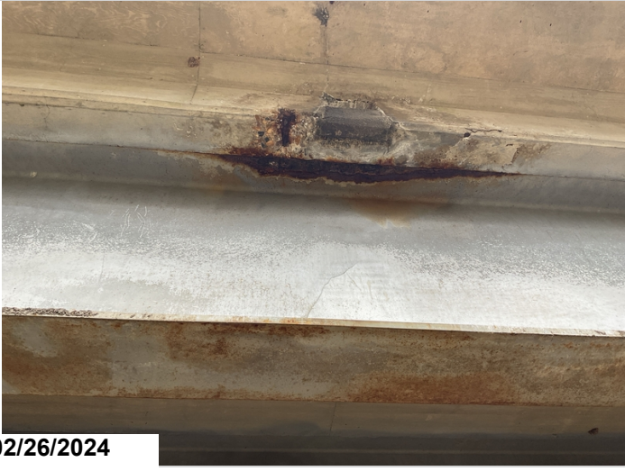
Main span 1, Outside of beam 5, Loss of effectiveness, 1 Sq Ft, CS4
