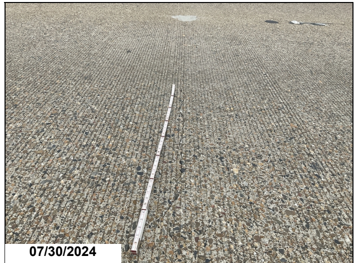
Span 5: unsealed transverse crack (0.020")
