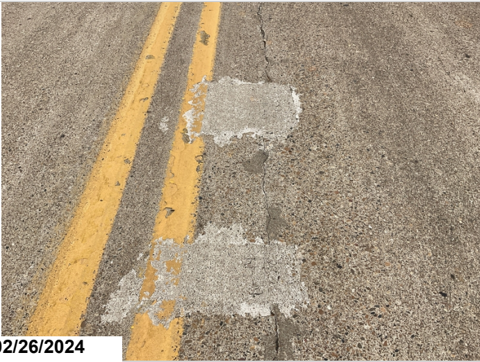
Approach span 4, Centerline, Patched areas, 2 Sq Ft, CS2
