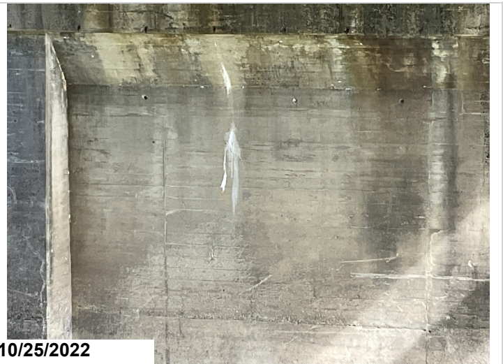
Pier 3, Back: Cracking with efflorescence.
