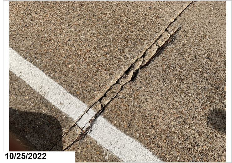
Bent 2: Spalling.
