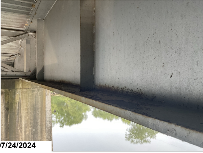
Span 6, girder 2: scattered freckled rust to the top of bottom flange and lower web. Common to all beams.
