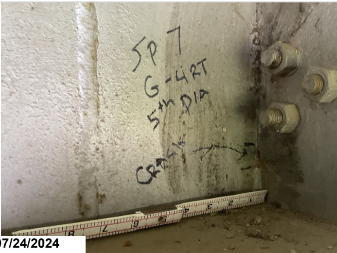
Span 7, girder 4, diaphragm 5: 1" crack in weld. CS4-1'
