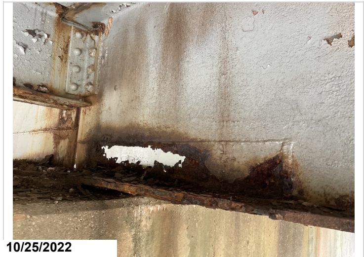
Bent 13, Span 13, Girder 3: Hole rusted through web, 16" long X 3" tall.
