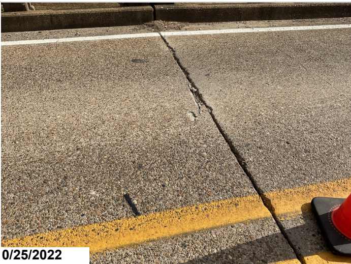
Bent 2: Spalling.
