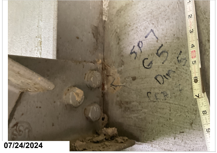
Span 7, girder 5, diaphragm 5: Cracked weld. CS4-1
