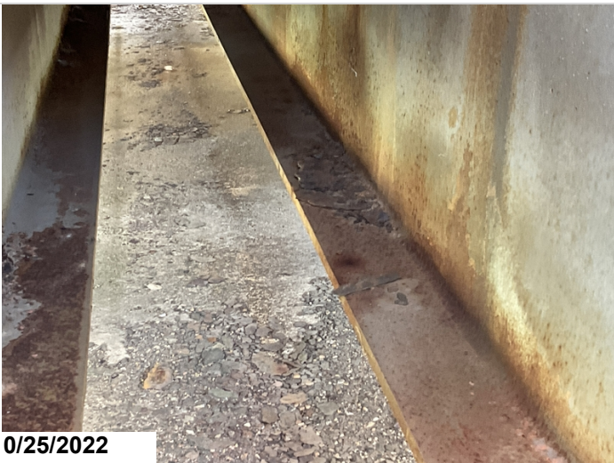
Typical active corrosion with flaking rust at joints.
