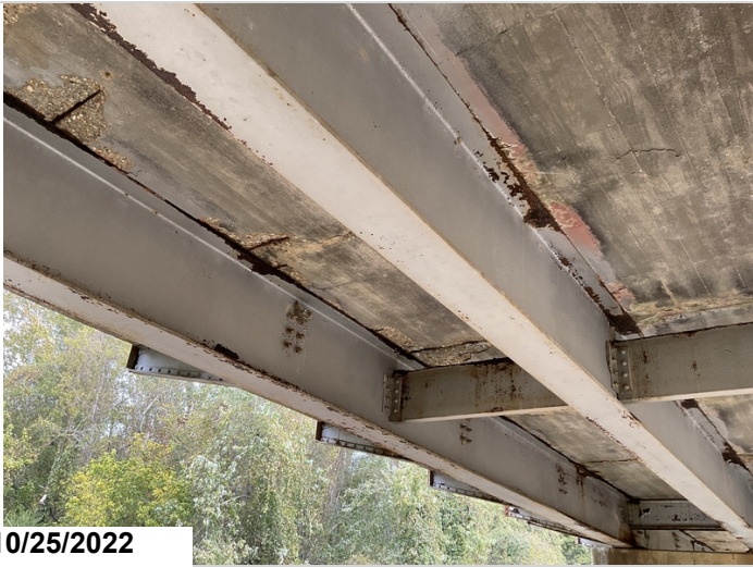
Span 2: Typical active corrosion with section loss on top flanges.
