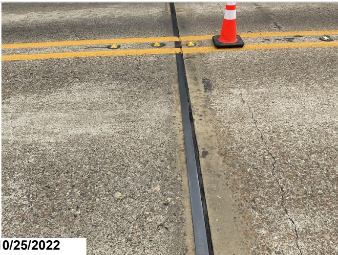
Pier 4, Joint: Loss of adhesion.
