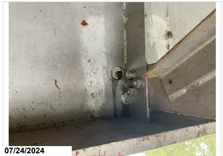
Span 6, girder 3, diaphragm 3; HBM repaired previous crack into the web. Common to all spans that have had previous cracks that propagated into the web.
