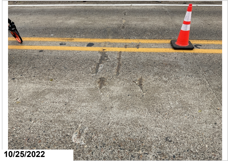
Truss Span 1: Spalling with exposed reinforcing steel with section loss.
