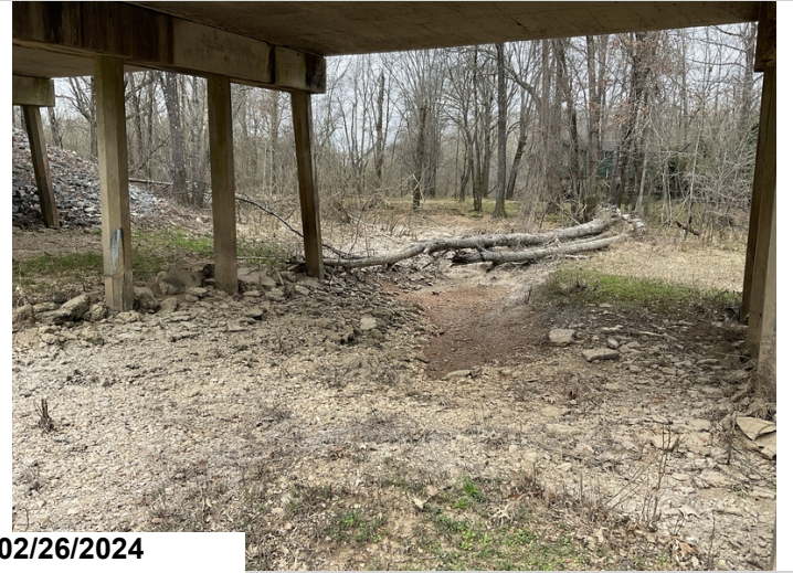
Minor scour between bents 3 & 4 in approach span
