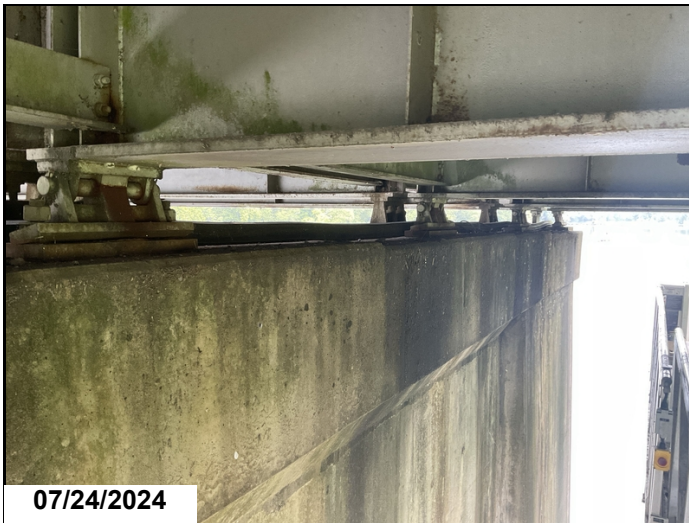
Pier 5: Joint seal has fallen out and I'd sitting atop the pier
