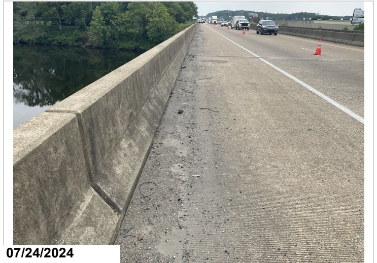
Dirt and debris in the gutter line of the deck.
