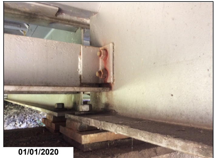
Bent 2 girder 3 ahead side loose bolts in diaphragm connection.
