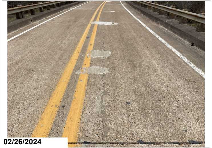
Approach span 4, Northbound lane, 30' longitudinal deck cracking, CS3
