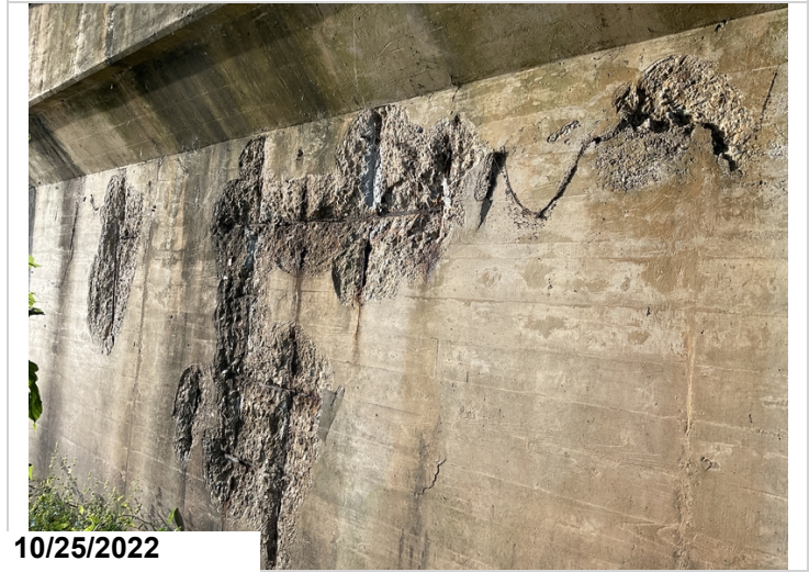
Pier 1, Ahead: Spalling with exposed reinforcing steel with section loss.
