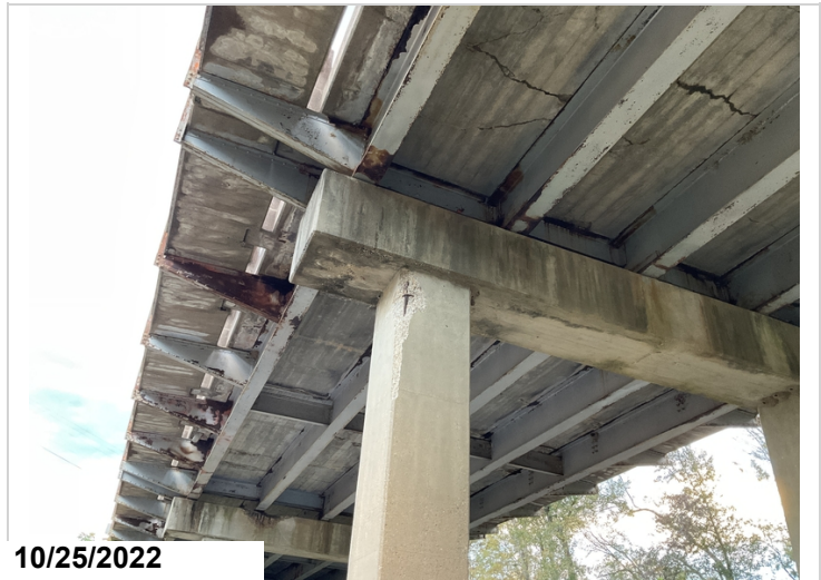
Bent 3, Column 2: Spalling with exposed reinforcing steel with section loss.
