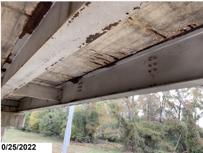
Span 4: Typical active corrosion with section loss on top flanges.
