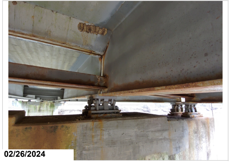
Various locations of beam end corrosion, CS2.
