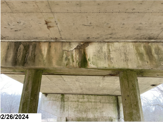
Approach span, Bent 23, Pier Cap, Looking ahead, Spalling between piles 2 & 3, 2 LF, CS2
