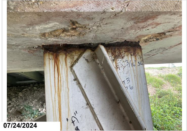
Bent 3, pile 6 backside: the entire flange adjacent to the cap has up to 3/16" section loss. CS3-1
