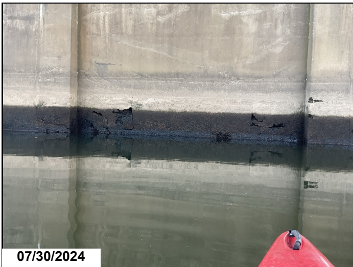
Backside Pier 3: multiple spalls due to abrasion and previous utility location. CS3-15'
