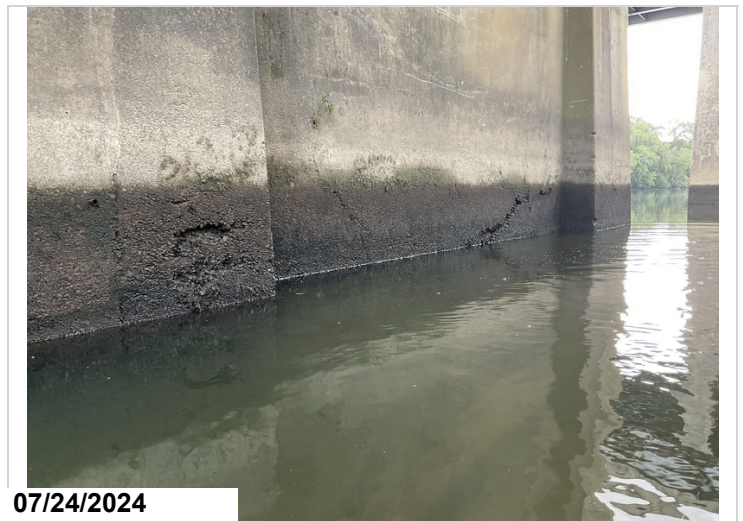
Backside Pier 2: 8' severe abrasion has created spalls CS3-5'
