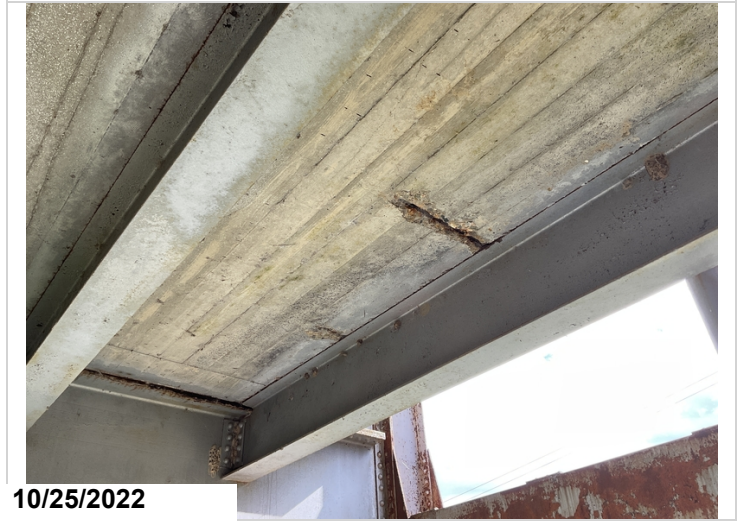
Typical exposed reinforcing steel with section loss in truss spans.
