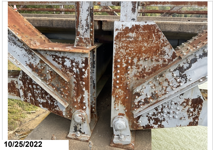
Minor active corrosion on gusset plates.
