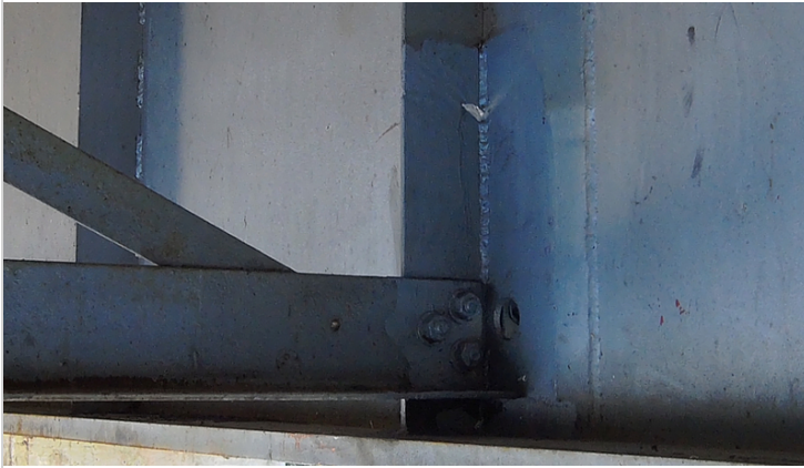
Span 7, girder 3, diaphragm 4: crack has been arrested. CS2-1'
