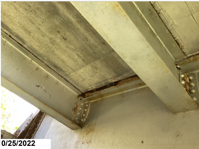
Truss Span 1, PP 1: Active corrosion with flaking rust.
