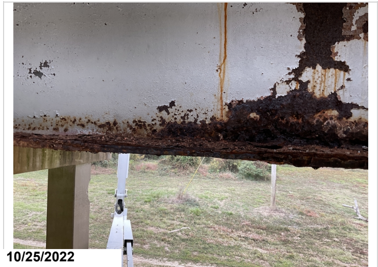
Span 4, Girder 1, 10' Back from Bent 11: 1/4" section loss to bottom flange.
