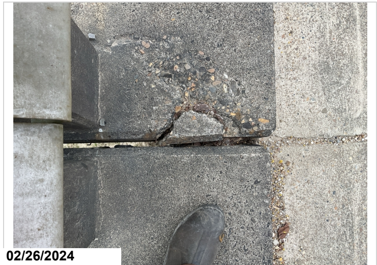
Approach span at right side of bent 17, spalling, CS3
