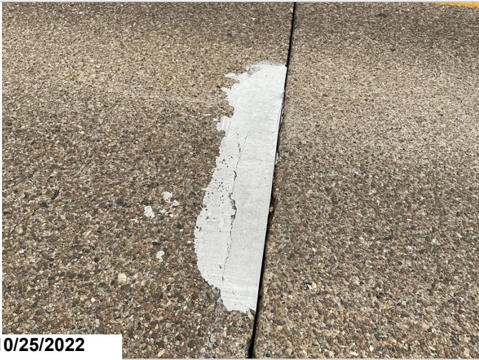
Bent 11, Span 11: Failing repair.
