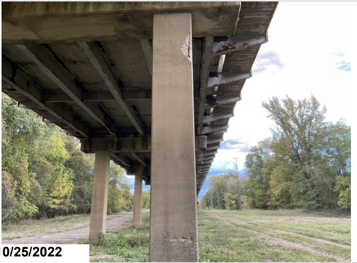
Bent 4, Column 2: Spalling with exposed reinforcing steel with section loss.
