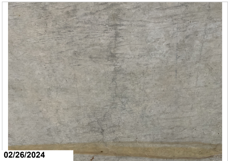
Approach span 1, Underside of deck, Deck cracking, CS2
