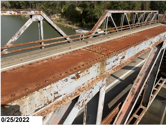
Minor active corrosion in top chord.
