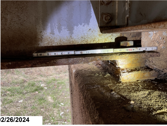
Main span 1, Beam 5 at Pier 1, 1/4" section loss to beam end & 1/8" section loss at haunch area, CS3
