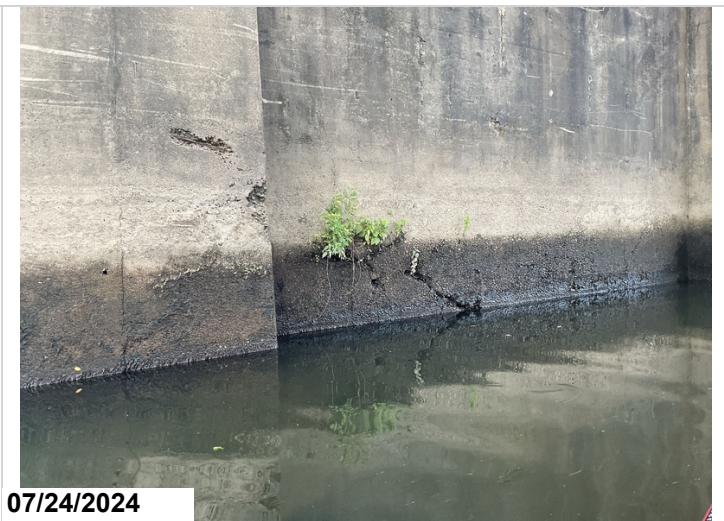
Ahead side pier 2: severe abrasion at the water line. CS3-11'
