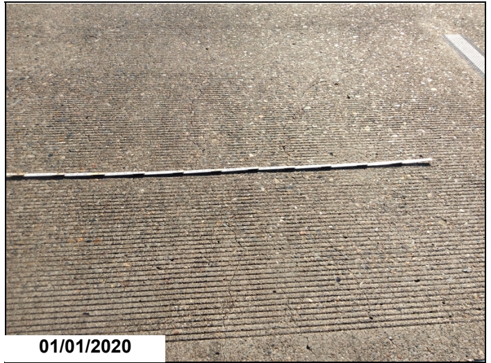
Span 3, longitudinal cracks up to .025".
