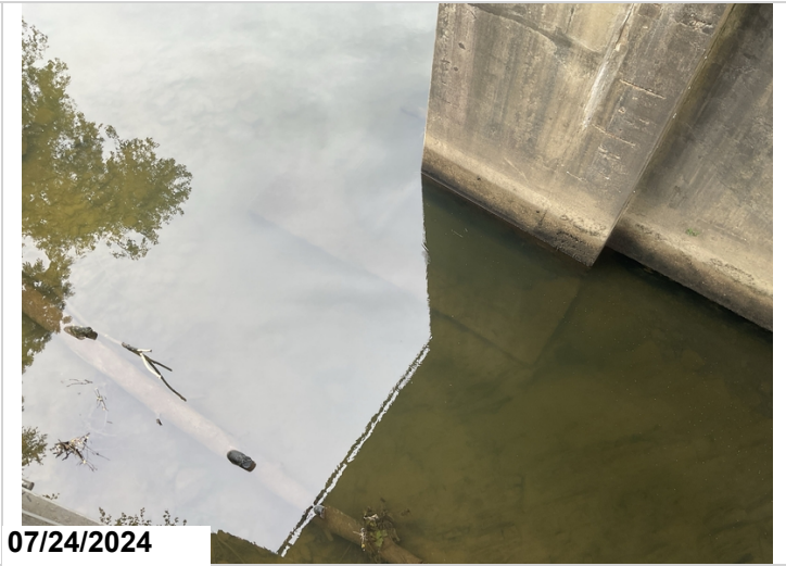
Pier 5: footing is exposed.
