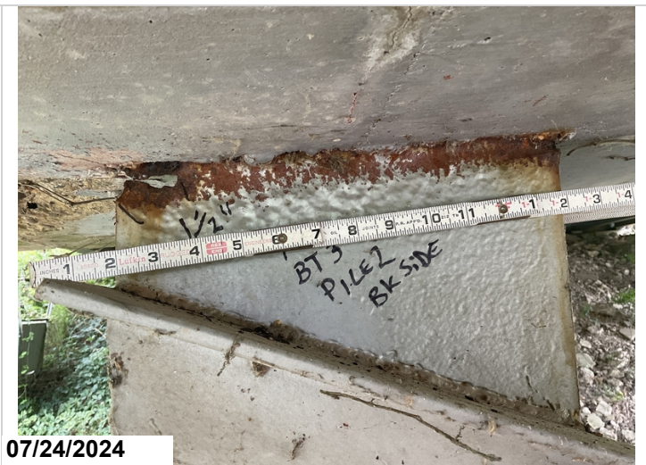
Bent 3, pile 2 backside: The flange has a 1 1/2" hole. CS4-1
