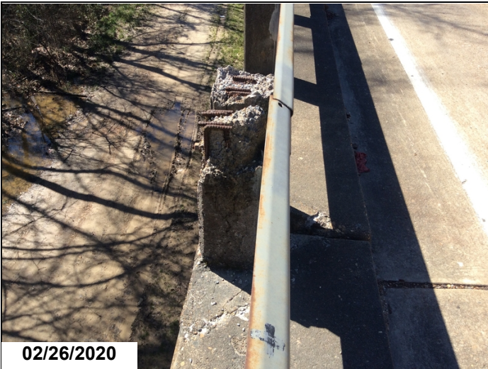
Span 17,18 Lt side post spalled and curb spalled
