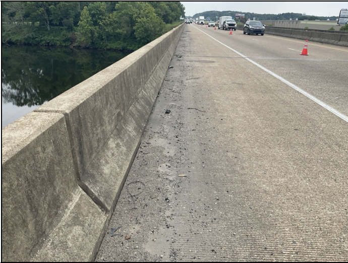
Dirt and debris in the gutter line of the deck.
