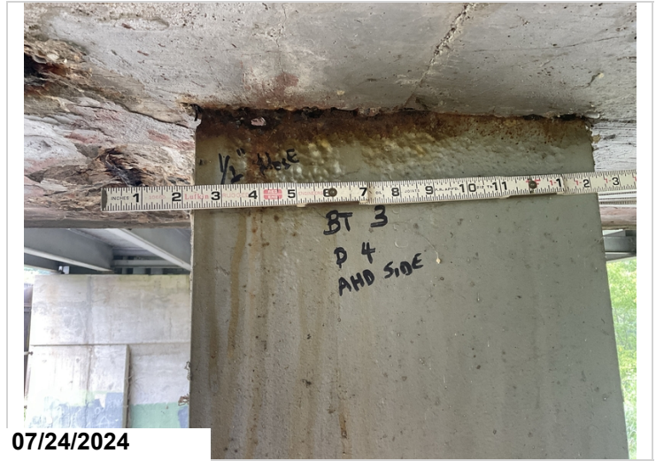
Bent 3, pile 4 ahead: The flange has a 1/2" hole and the remainder has approximately 3/16" section loss adjacent from the cap. CS4-1
