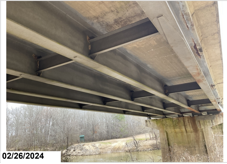
Typical photo, Painted steel beams in main spans
