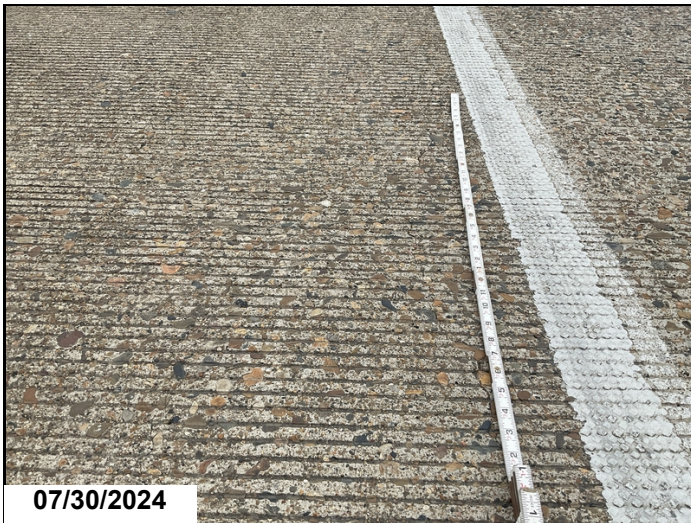
Span 4: unsealed longitudinal crack. (0.020")
