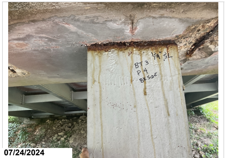
Bent 3, pile 4 backside: the entire flange adjacent to the cap has up to 1/4" section loss. CS3-1
