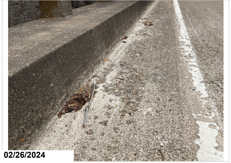
Approach span 2, Southbound lane, Abrasion along gutterline, CS2
