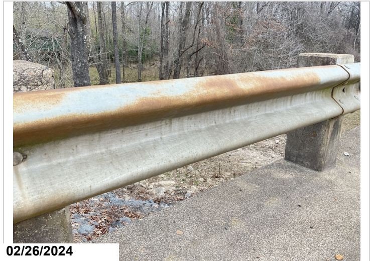
Both right and left sides of approach spans, corrosion, CS2
