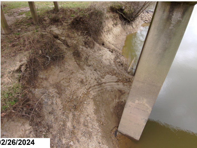
Erosion around pier 4
