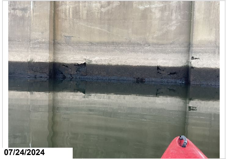
Backside Pier 3: multiple spalls due to abrasion and previous utility location. CS3-15'
