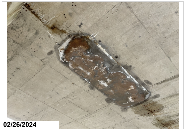
Approach span 4, Underside of deck, Patched area, 16 Sq Ft, CS2
