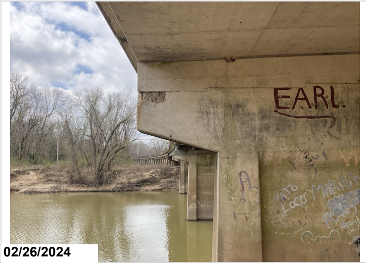
Main span, Pier 4, Looking back, Rebar exposed on right side, 1 LF, CS3
