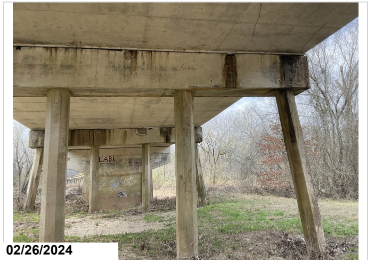
Approach span, Bent 24, Pier cap, Looking back, Spall between piles 2 & 3, 1 LF, CS2
