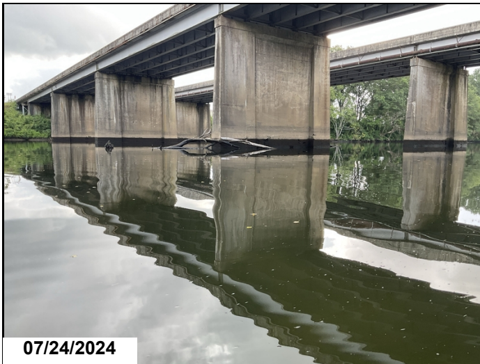
Pier 3: drift has accumulated on the upstream end of pier.
