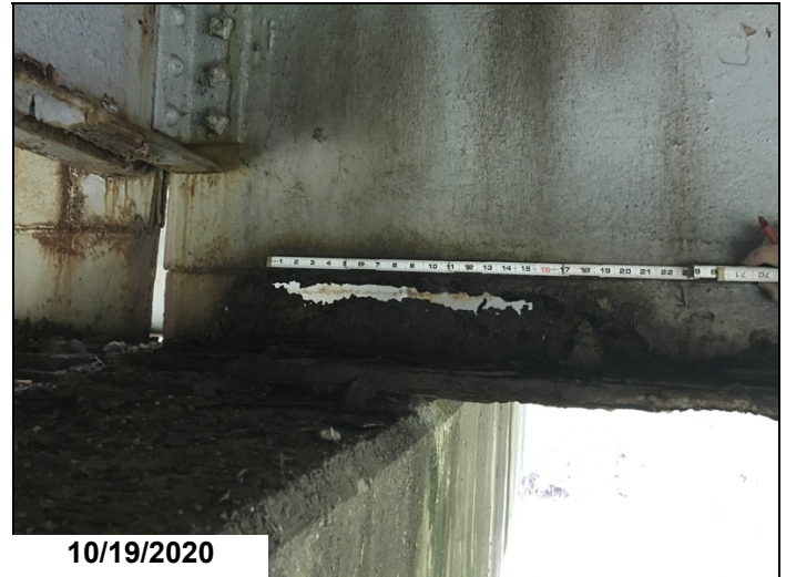
Span 13 bent 13 Girder 3 has a hole rusted through the t-splice repair.
