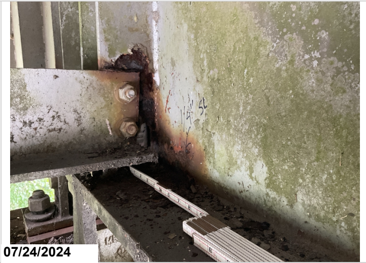
Girder 2, Pier 2, span 4: up to 1/4" section loss to the lower web. (4"x2" area) Large hole in the adjacent stiffener. CS3-1'
