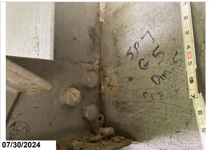
Span 7, girder 5, diaphragm 5: Cracked weld. CS4-1
