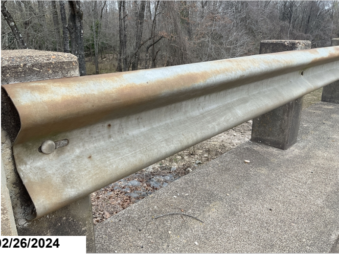
Both right and left sides of approach spans, corrosion, CS2
