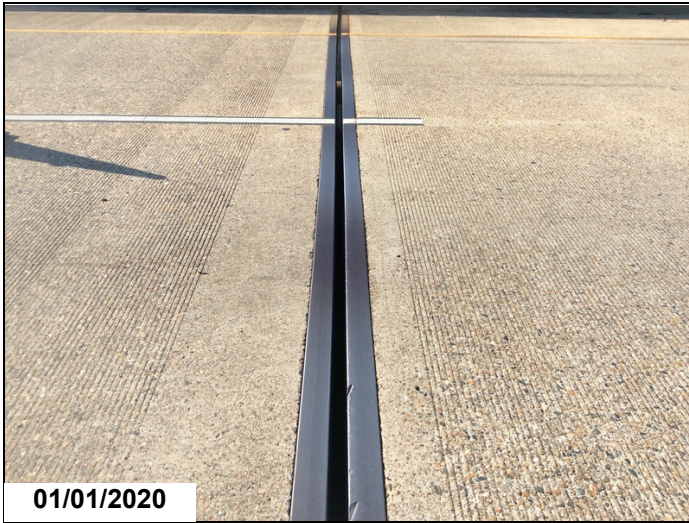
Pier 4, joint seal has fallen out.
