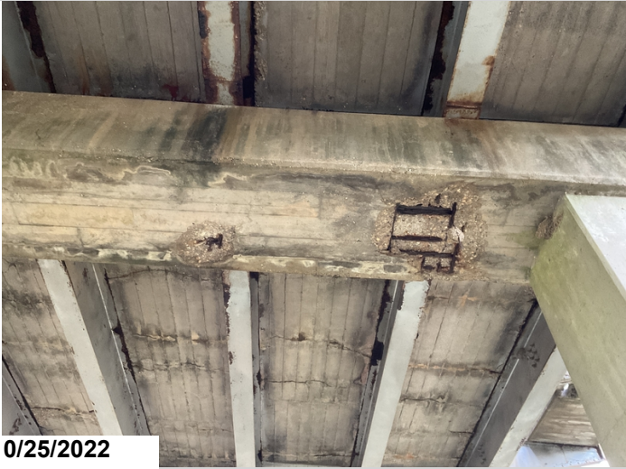
Bent 11: Spalling with exposed reinforcing steel with section loss.
