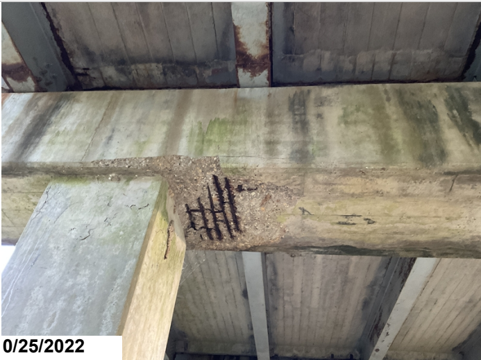
Bent 15, Spalling with exposed reinforcing steel with section loss.
