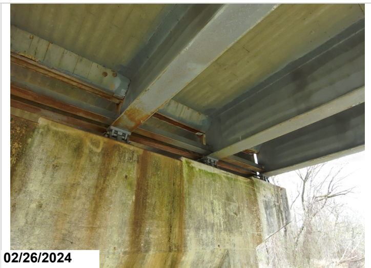
Various locations of beam end corrosion, CS2.
