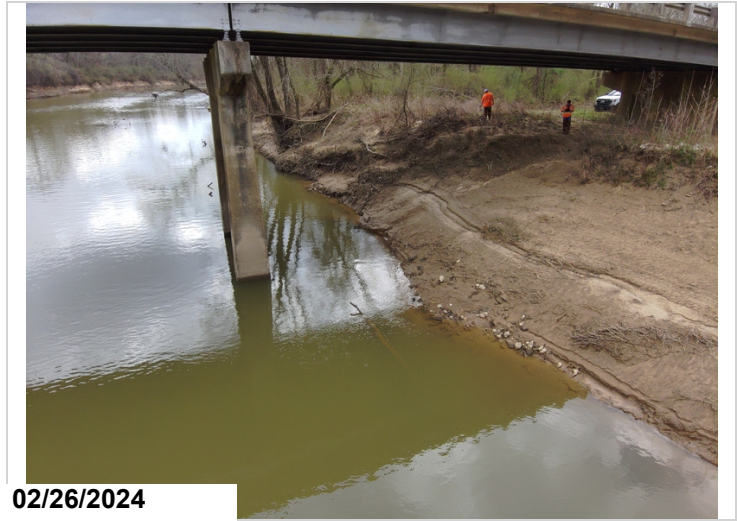
Erosion around pier 2 channel bank
