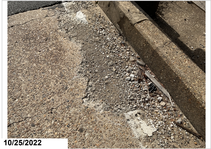
Span 1, Left: Spalling.
