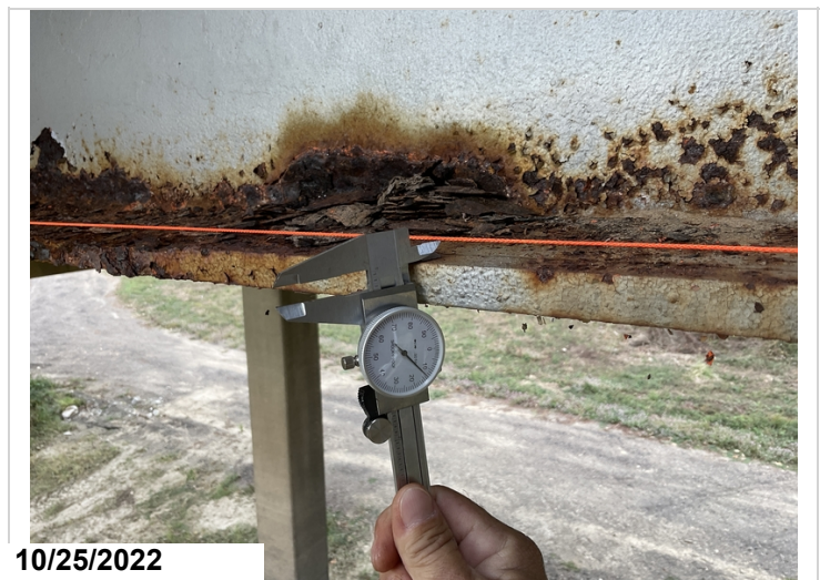
All spans have approximately 0.31" of sag in girders.
