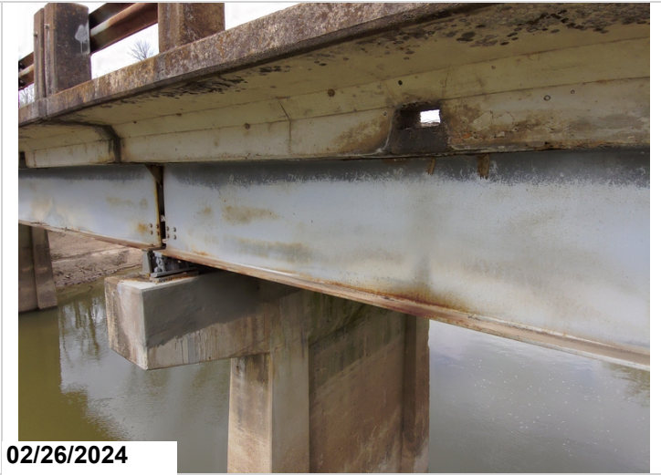
Beam 5 near pier 2, corrosion on steel beams, CS2.
