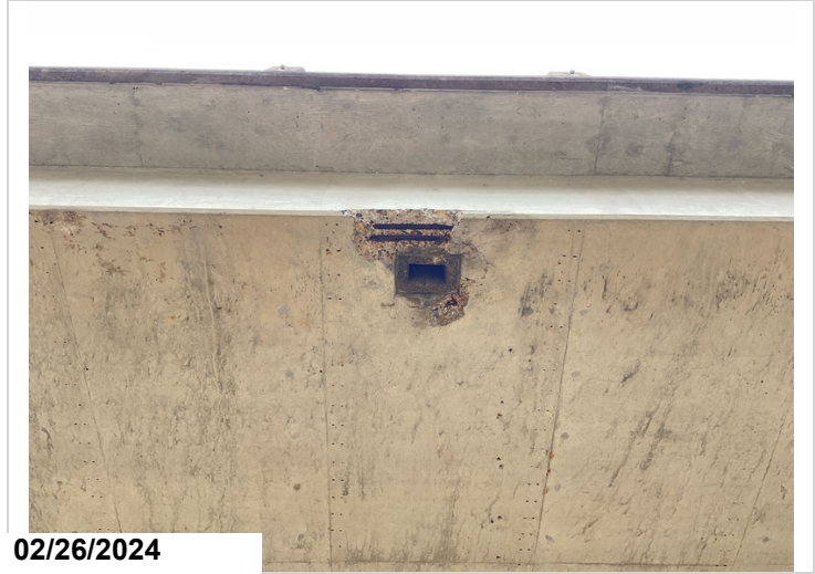
Approach span 3, Underside of deck, Right side, Exposed rebar at drain, 1 Sq Ft, CS3
