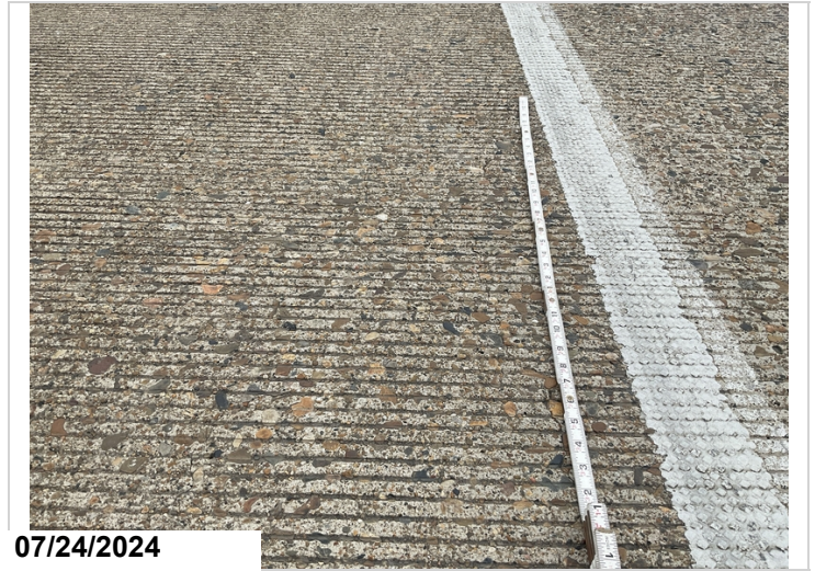
Span 4: unsealed longitudinal crack. (0.020")
