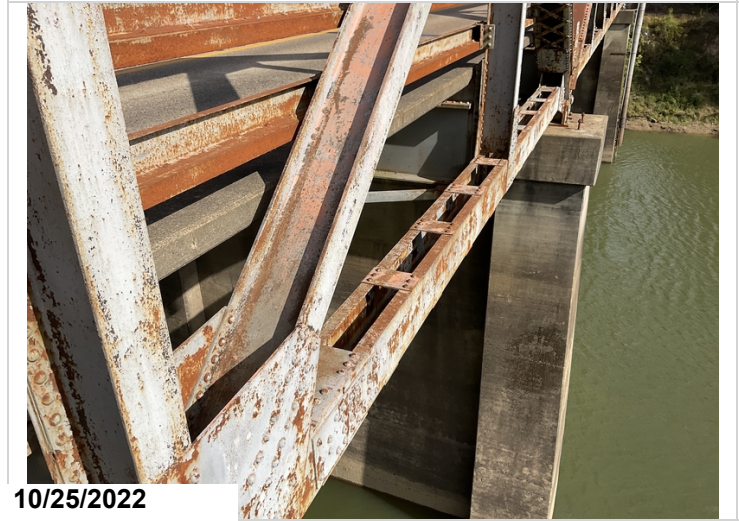
Minor active corrosion in bottom chord.
