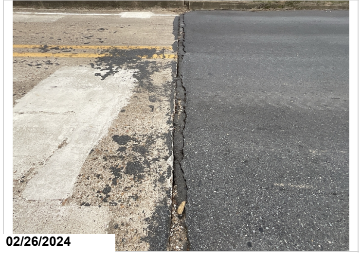
Approach span bent 29, asphalt overlay impacting joint, CS3
