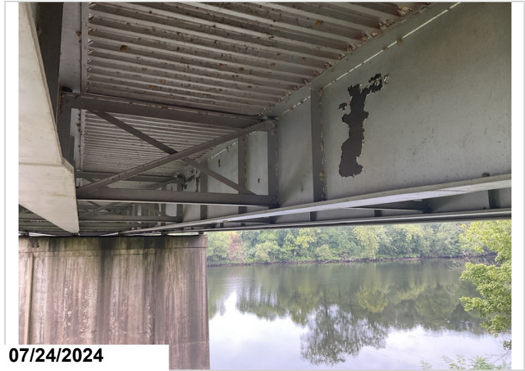
Span 7, girder 3: paint flaking
