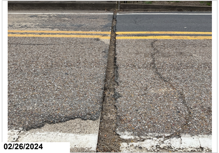
Approach span bent 1, missing joint material, CS4
