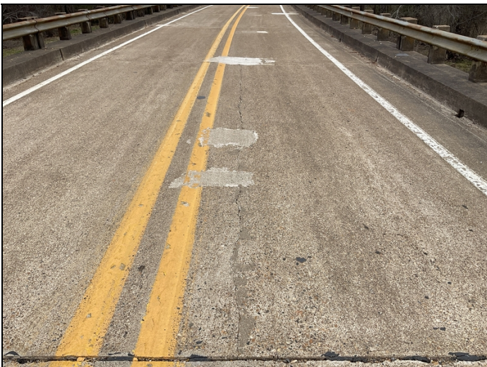
Approach span 4, Northbound lane, 30' longitudinal deck cracking, CS3
