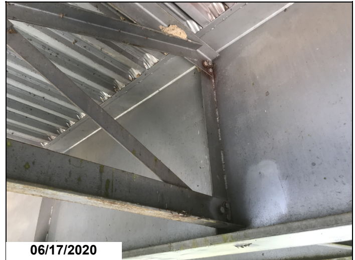
Span 5, loose bolts in top of diaphragm
