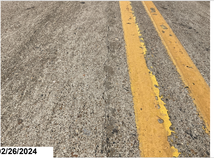
Approach span 1, Southbound lane, Longitudinal deck cracking in all spans, CS3
