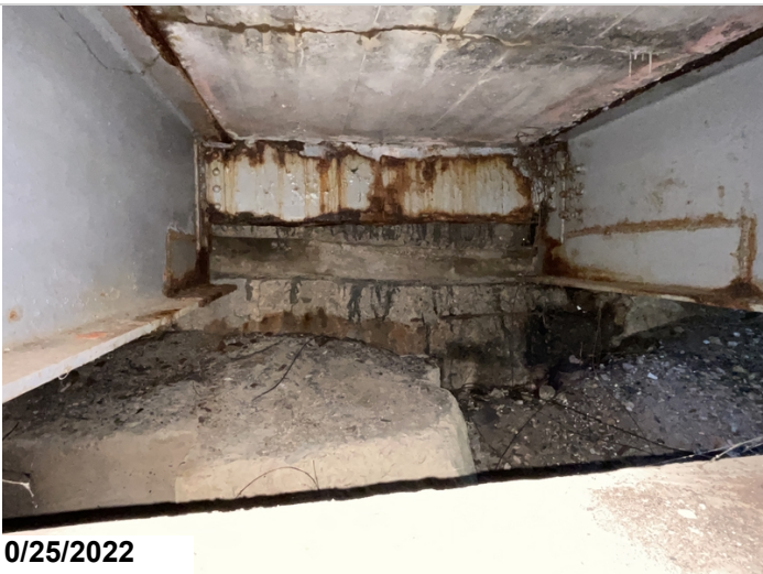
Bent 1, Back: Girders are suspended.
