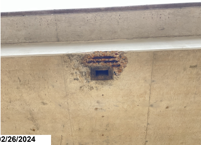
Approach span 2, Underside of deck, Right side, Exposed rebar at drain, 1 Sq Ft, CS3
