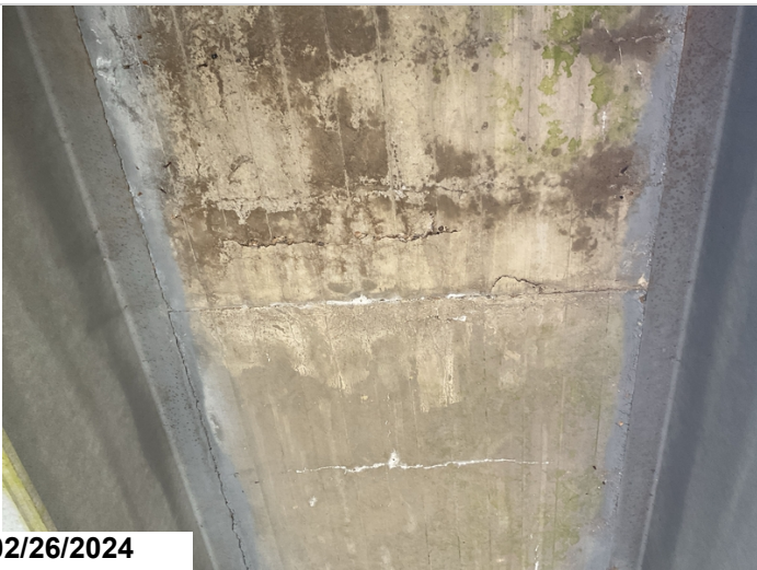
Main span 1, Underside of deck, Delam in bay 4, 3 Sq Ft, CS2
