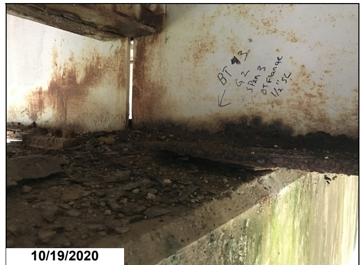
Bent 3 girder 2 1/2" section loss bottom flange
