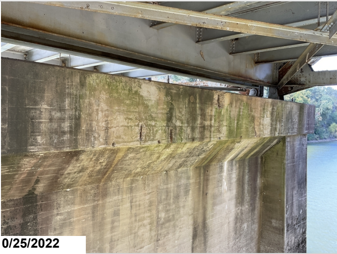
Pier 3, Ahead: Spalling with exposed reinforcing steel with section loss.
