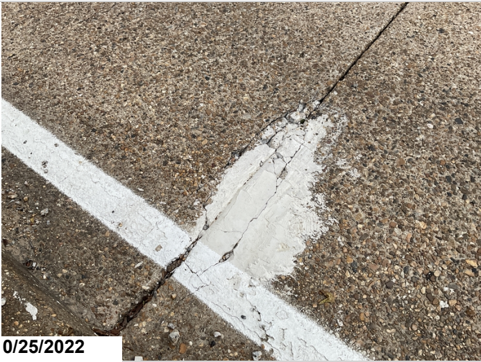
Bent 12, Span 11: Repair failing.
