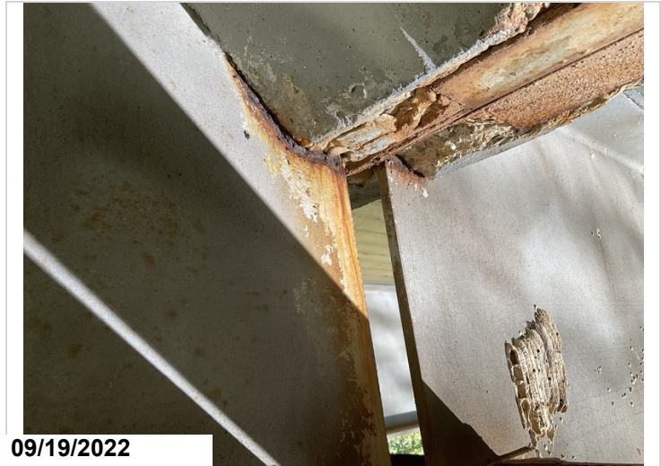
Main span 2 at pier 2, Beam 3, Corrosion on beam end, CS3
