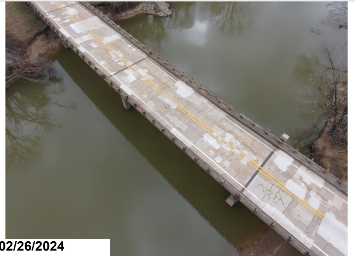
Main Span, Deck Patching, CS2 & CS3
