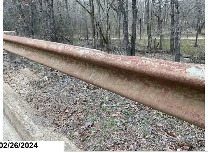
Corrosion and minor damage to bridge railing transition, typical in various locations
