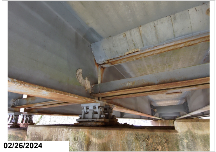
Various locations of beam end corrosion, CS2.
