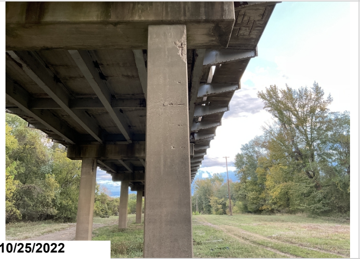
Bent 5, Columns 1 & 2: Spalling with exposed reinforcing steel with section loss.
