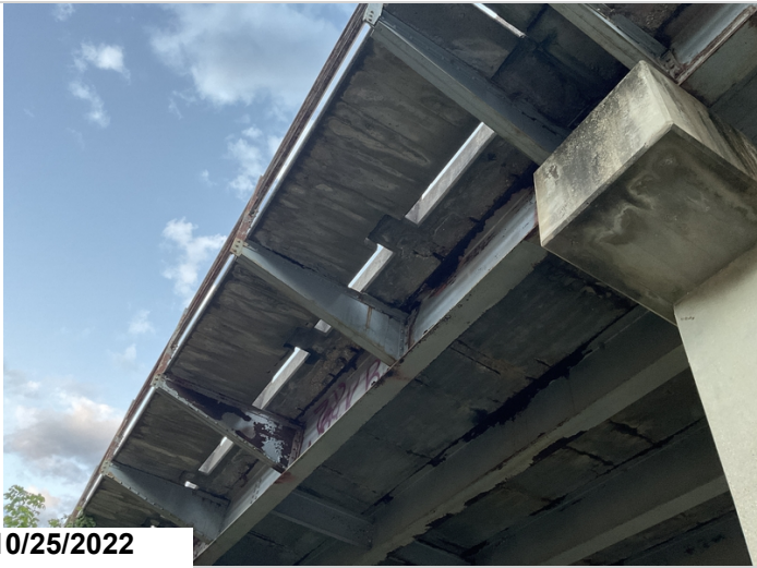
Typical spalling with exposed reinforcing steel with section loss
