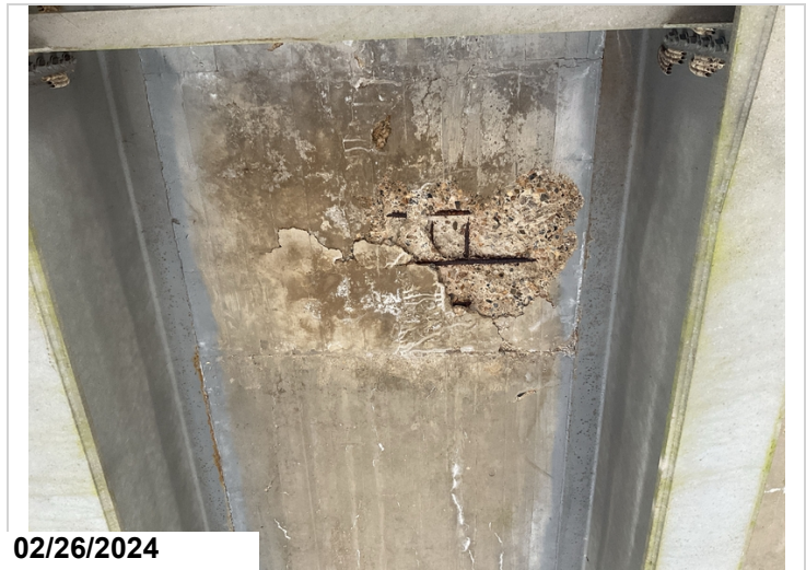
Main span 1, Underside of deck, Rebar exposed in bay 3, 2 Sq Ft, CS3
