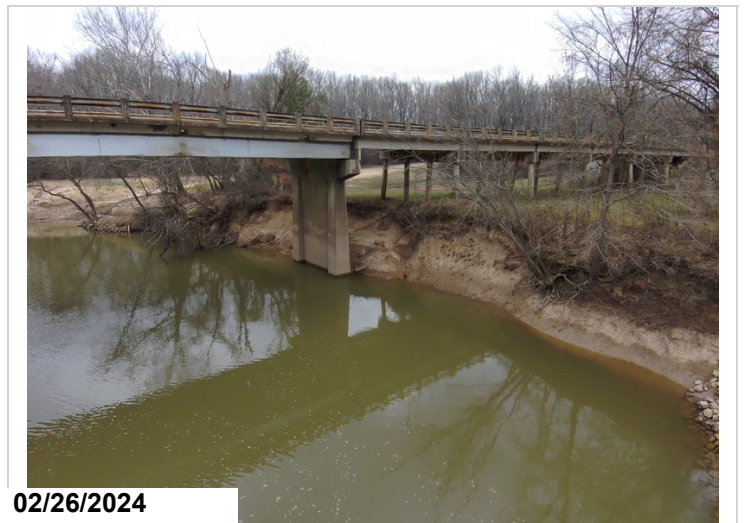
Erosion around pier 4
