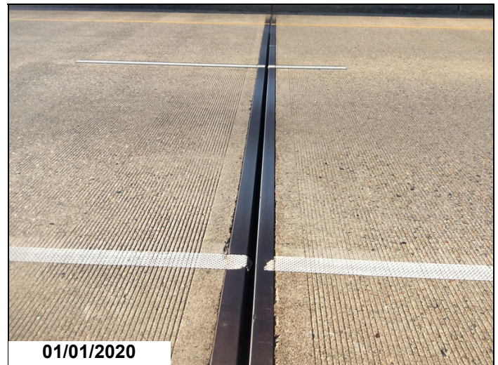
Pier 1, joint seal has fallen through.
