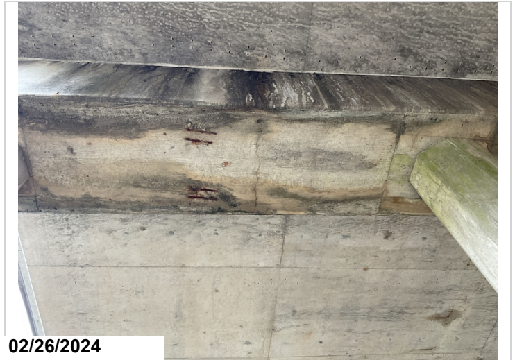
Approach span, Bent 3, Pier Cap, Cracking on underside, 1 LF, CS2
