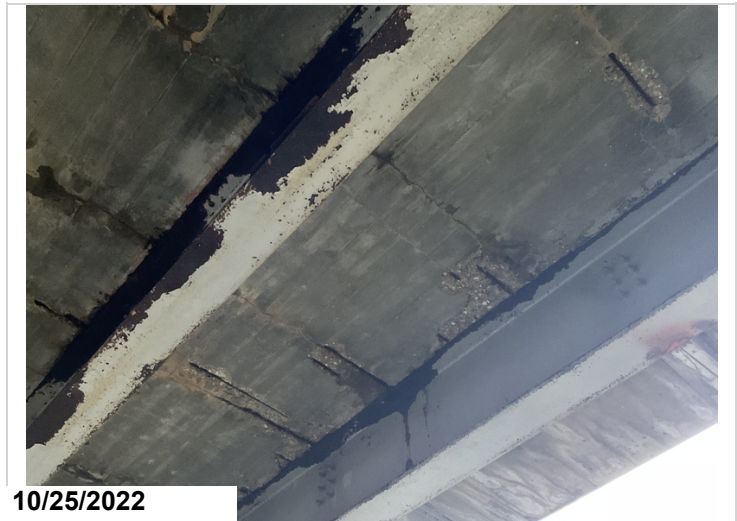
Typical exposed reinforcing steel with section loss in multi-girder spans.
