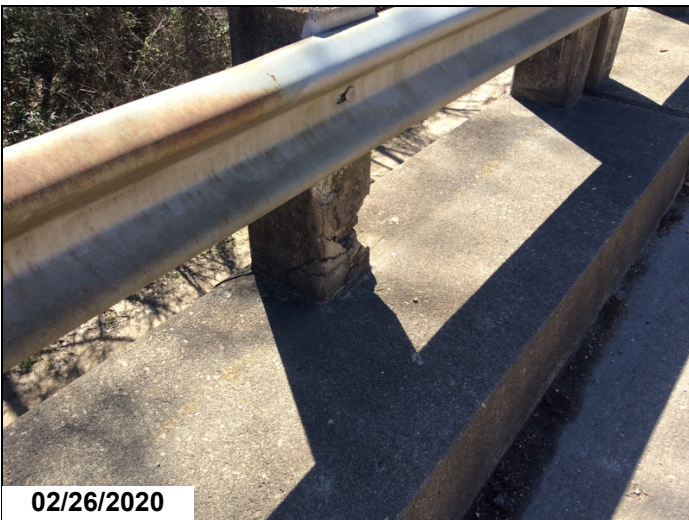
Span 19 Lt side post spalled
