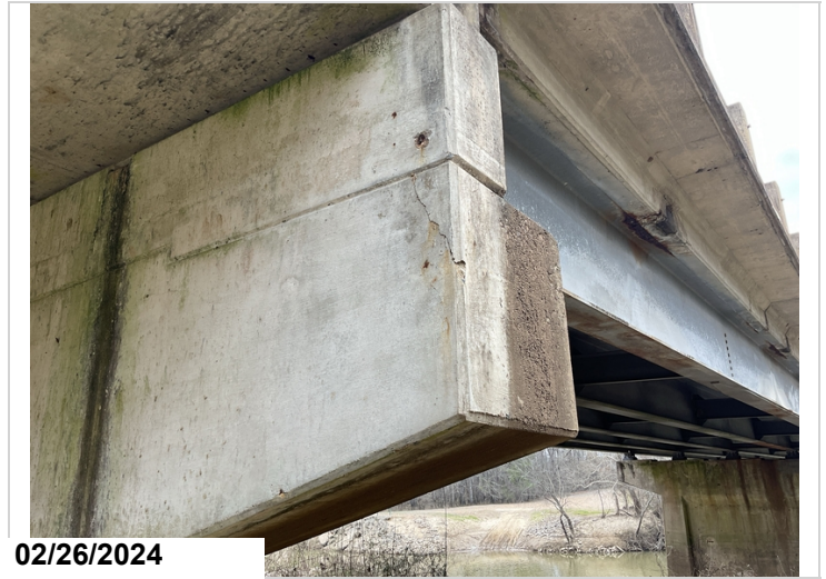
Main span, Pier 1, Looking ahead, Delam to right side of cap, 1 LF, CS2
