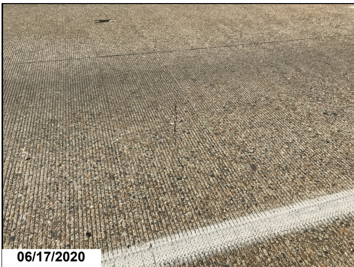
Span 7, large transverse cracks.
