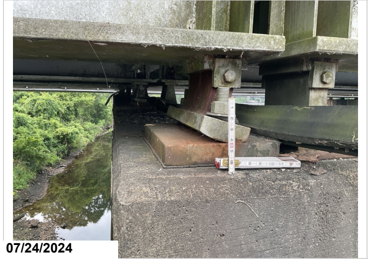
Pier 5, girder 1: bearing rocked back. Common to all bearings at this span.
