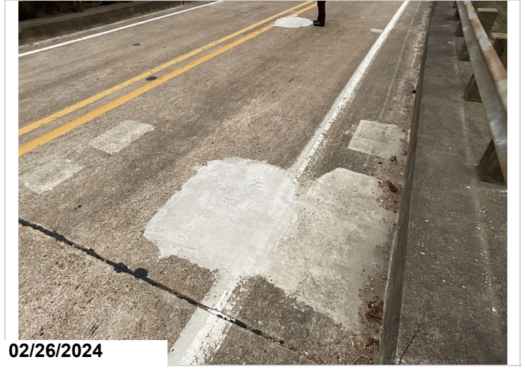
Approach span 6, Northbound Lane, Patched areas, 8 Sq Ft, CS2
