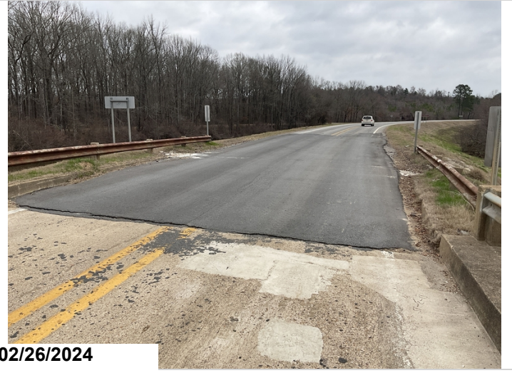
Asphalt overlay butted up to the end of bridge.
