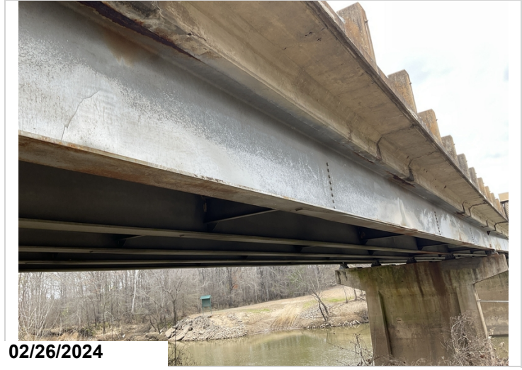
Main span 1, Outside of beam 5, Chalking, CS2
