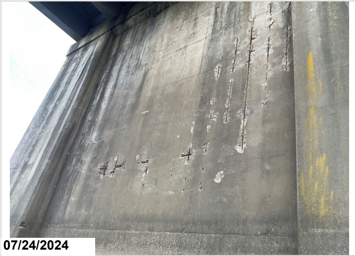
Backside of pier 4: numerous spalls with exposed rebar to the pier wall. CS3-10'
