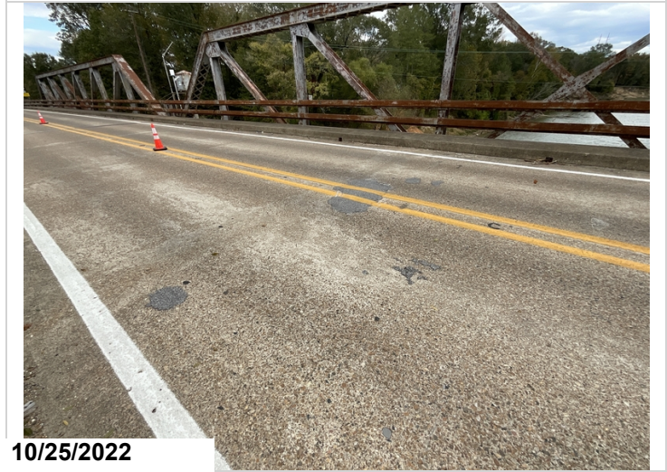
Truss Span 2: Spalling with asphalt repairs.
