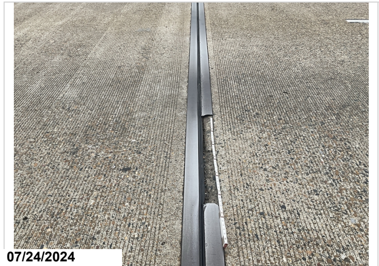
Pier 7: 3' of joint armor missing in the right west bound lane
