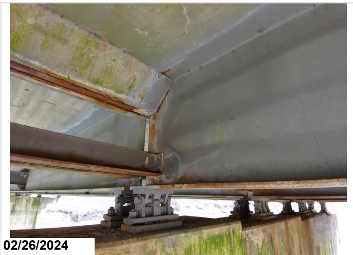
Pier 2 beam end corrosion, CS2.
