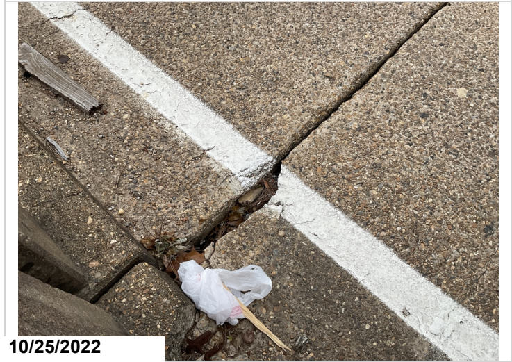
Bent 11, Span 11: Spalling.
