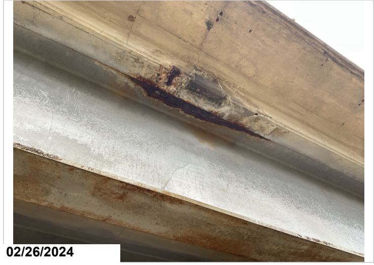
Main span 1, Beam 5, Corrosion to top flange, 1 Sq Ft, CS3
