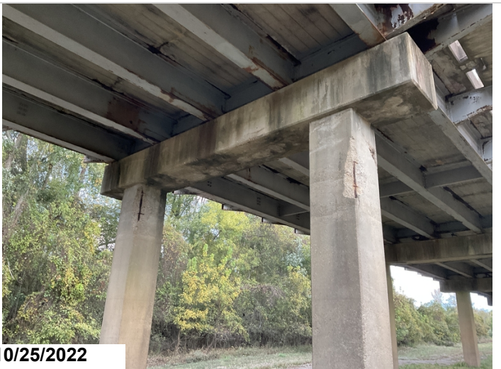
Bent 7, Columns 1 & 2: Spalling with exposed reinforcing steel with section loss.
