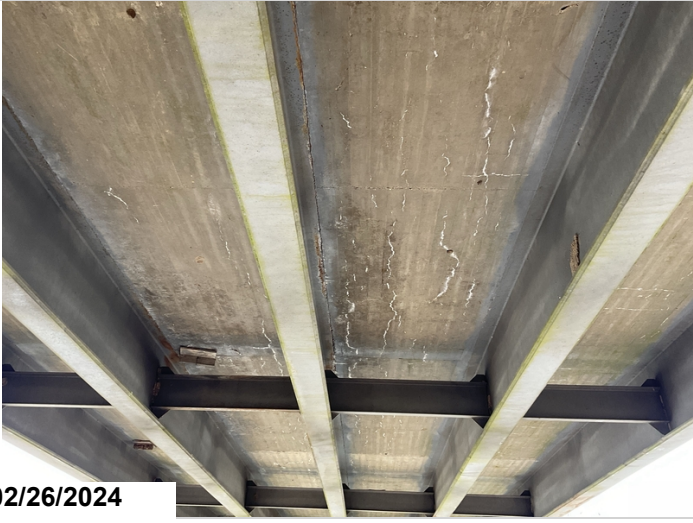
Main span 1, Underside of deck, Efflorescence in all bays, CS2
