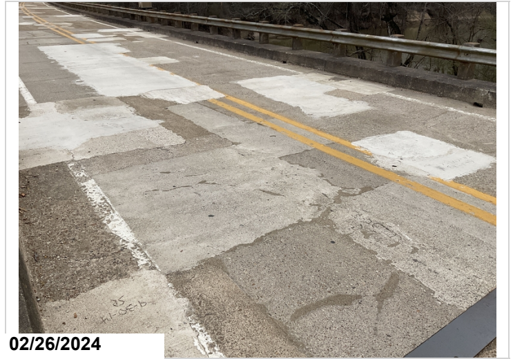
Main span 1, Both North and Southbound lanes, Patched areas, CS2 & CS3
