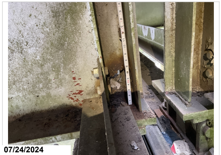
Girder 4: 3"x 3" hole in the web between the stiffeners above the bearing at pier 2. CS4-1'
