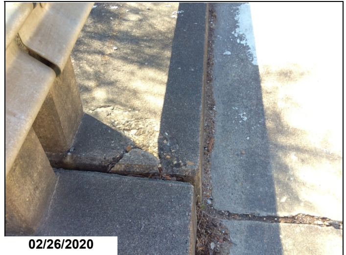
Span 17 Lt side curb spalled
