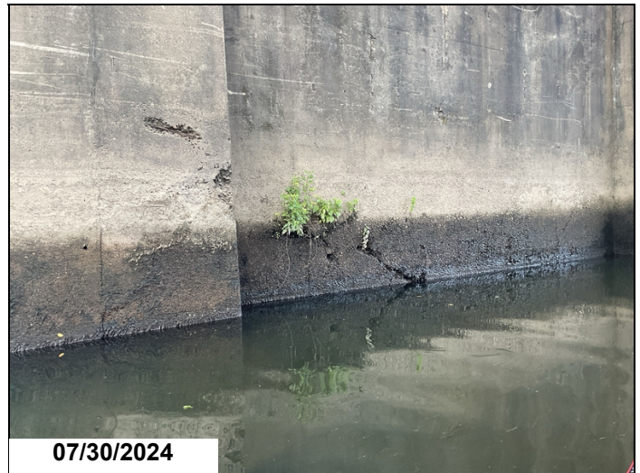
Ahead side pier 2: severe abrasion at the water line. CS3-11'
