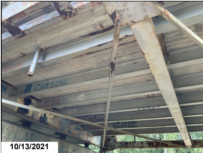
Collision damage
