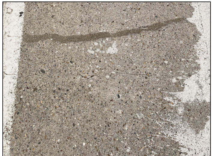
Main span 1, Southbound lane, Deck cracking, CS2
