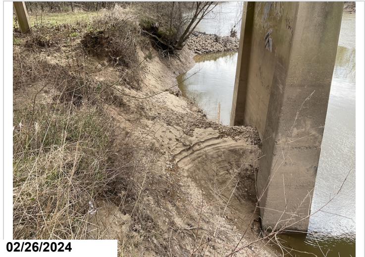
Scour around Pier 4, Scour is approximately 8' from reaching Bent 25 pile
