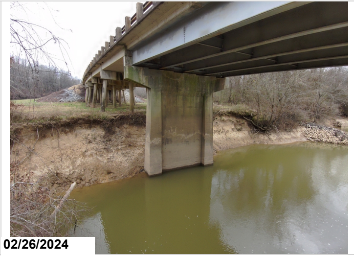
Erosion around pier 4
