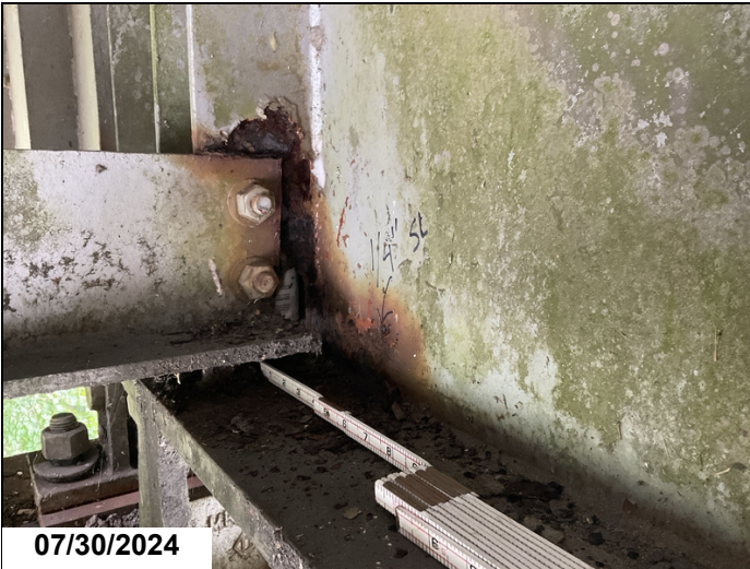
Girder 2, Pier 2, span 4: up to 1/4" section loss to the lower web. (4"x2" area) Large hole in the adjacent stiffener. CS3-1'
