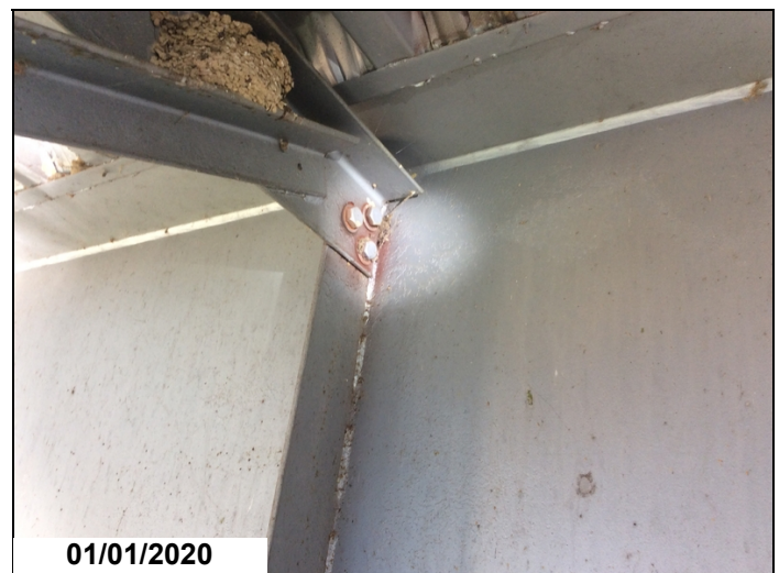
Span 5 girder 2 right, diaphragm 4, bolts are loose at top.
