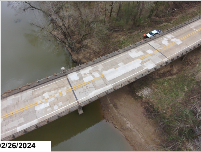
Main Span, Deck Patching, CS2 & CS3
