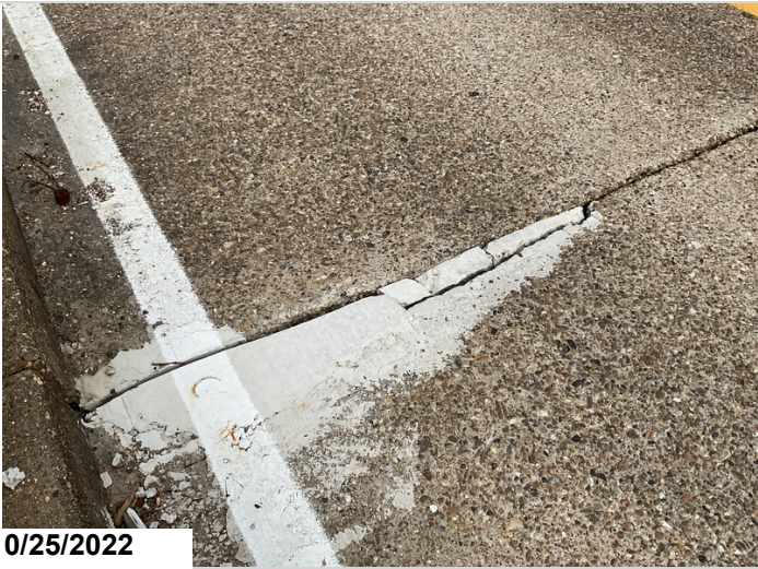
Bent 5, Span 4: Failed repair.
