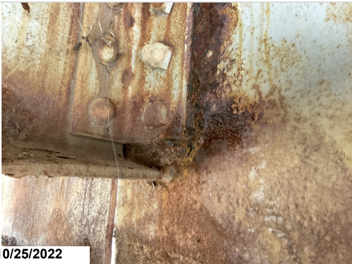
Bent 8, Girder 3, Right: 7/16" section loss, 3" long X 1" tall.
