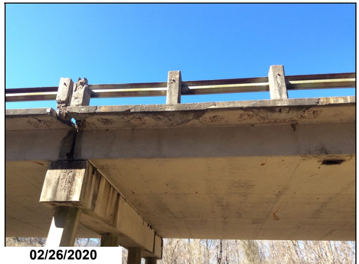
BT 18 over hand spalls cracks and rebar exposed
