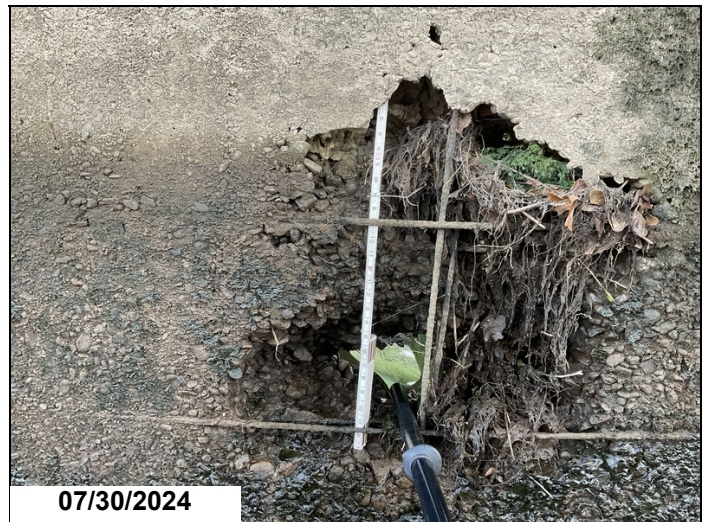
Pier 5: at the centerline of the pier a large spall with exposed rebar that is believed to be a previous location for utility pipe. (1 1/2' x 1') CS4-1'
