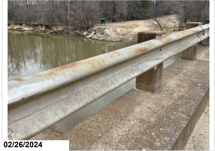
Both right and left sides of main spans, corrosion, CS2
