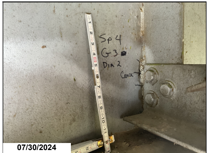
Span 4, girder 3, diaphragm 2: a 2" crack in the weld. CS4-1'
