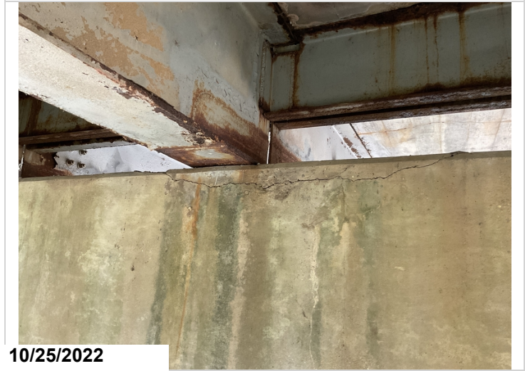
Bent 2, Back, Girder 2: Cracking.
