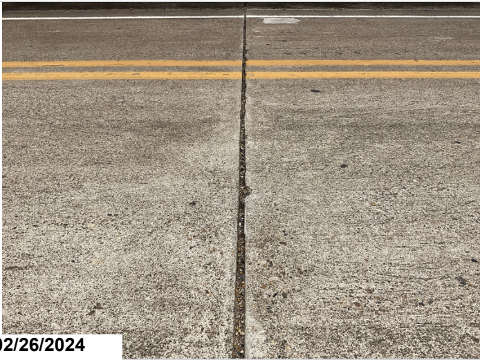
Approach span bent 3, missing joint material, CS4
