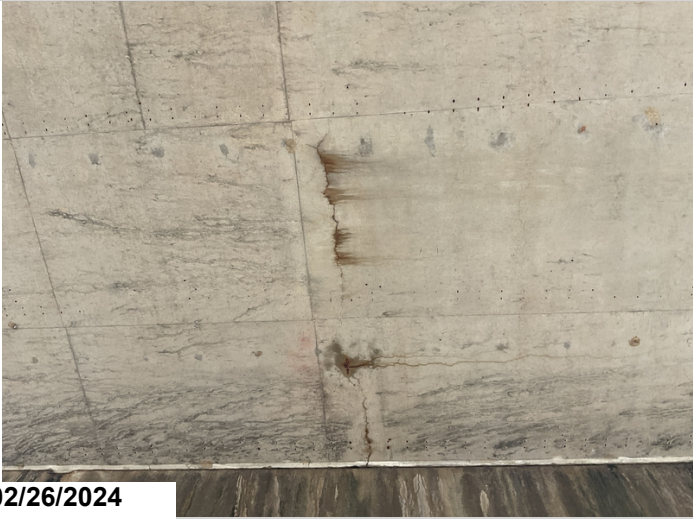
Approach span 3, Underside of deck, Efflorescence with rust staining, CS3
