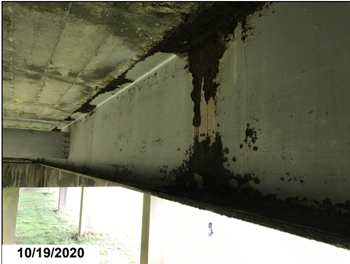
Typical corrosion along the webs in various locations
