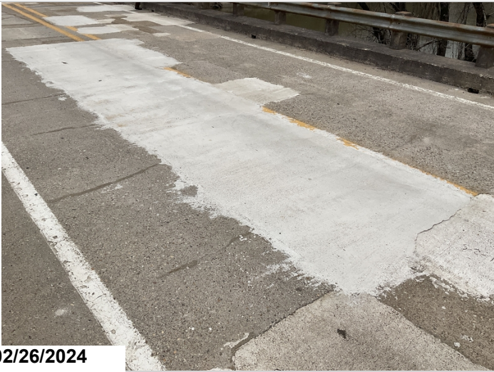
Main span 1, Southbound Lane, Large patched area, 63 Sq Ft, CS2
