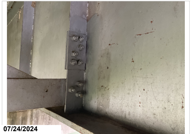
Span 7, girder 3, 6th diaphragm: previous cracked weld has been repaired. CS2-1'
