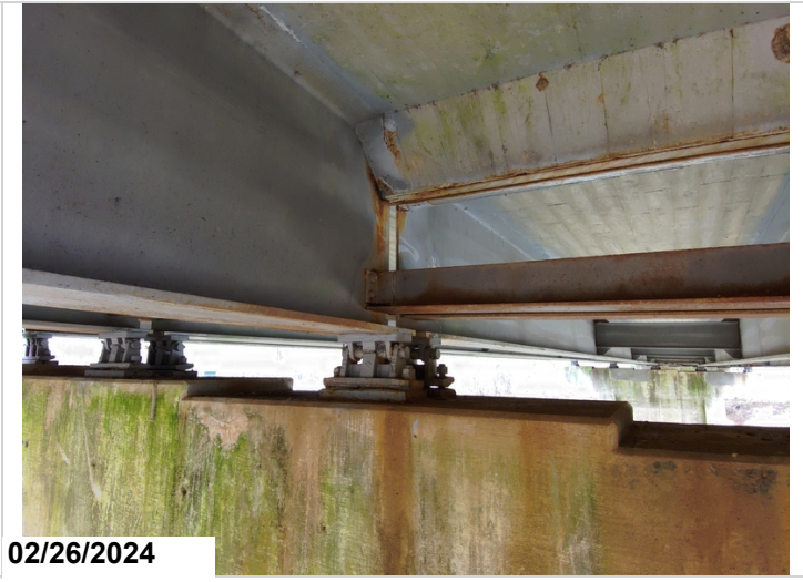
Various locations of beam end corrosion, CS2.
