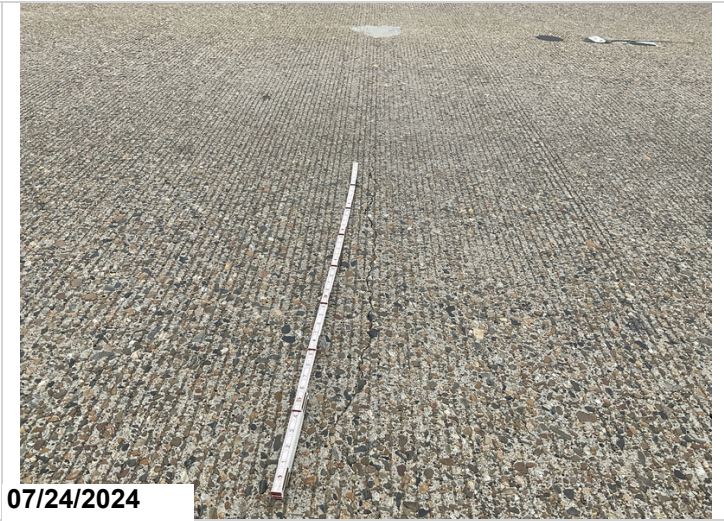
Span 5: unsealed transverse crack (0.020")
