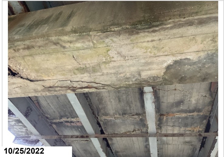
Bent 14: Delam.
