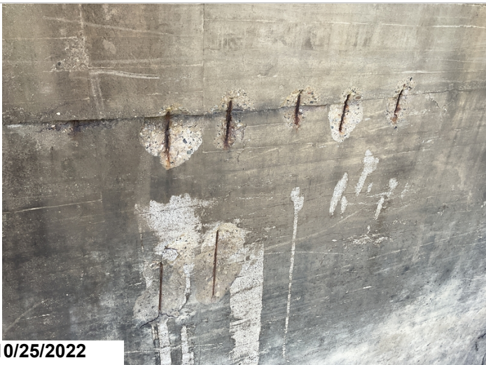
Pier 2, Ahead: Spalling with exposed reinforcing steel with section loss.
