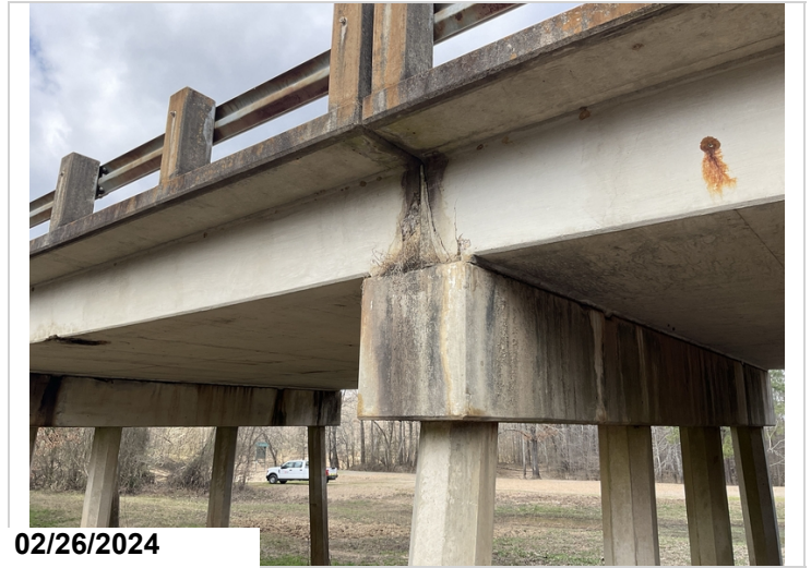
Approach span, Bent 28, Looking back, Delam on right side, 1 Sq Ft, CS3
