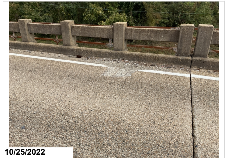
Span 8, Right: Spalling with exposed reinforcing steel with section loss.
