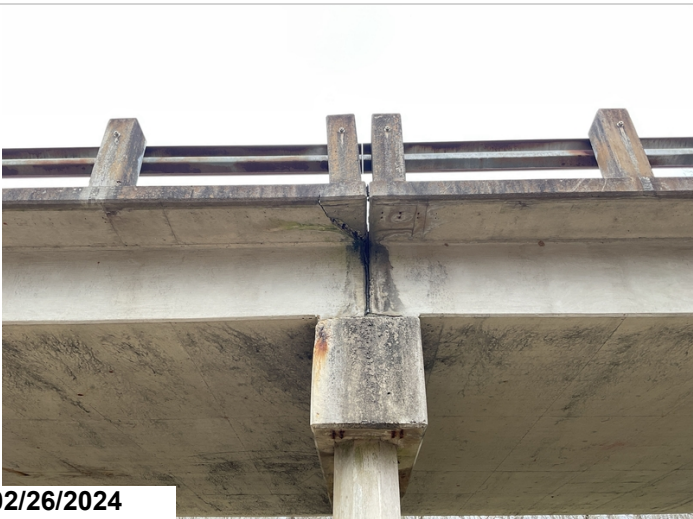
Approach span at right side of bent 17, spalling, 1 Sq Ft, CS3
