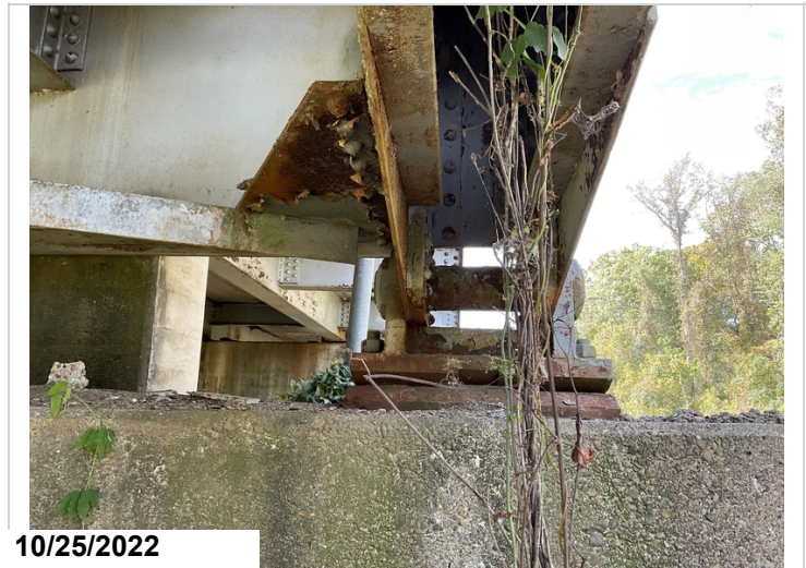
Pier 1, Bearings: Minor active corrosion.
