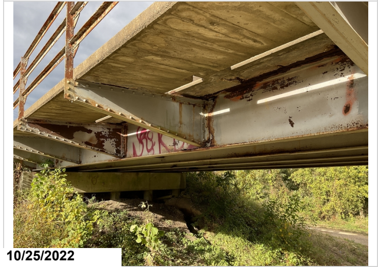
Typical active corrosion with flaking rust in cantilever brackets.
