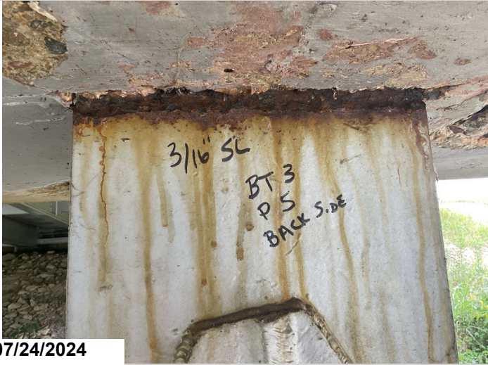
Bent 3, pile 5 backside: the entire flange adjacent to the cap has up to 3/16" section loss. CS3-1
