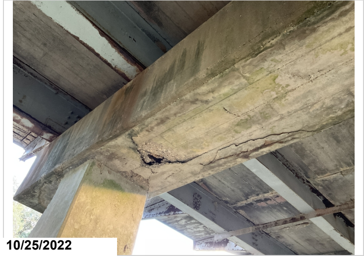
Bent 14: Spalling with exposed reinforcing steel with section loss.
