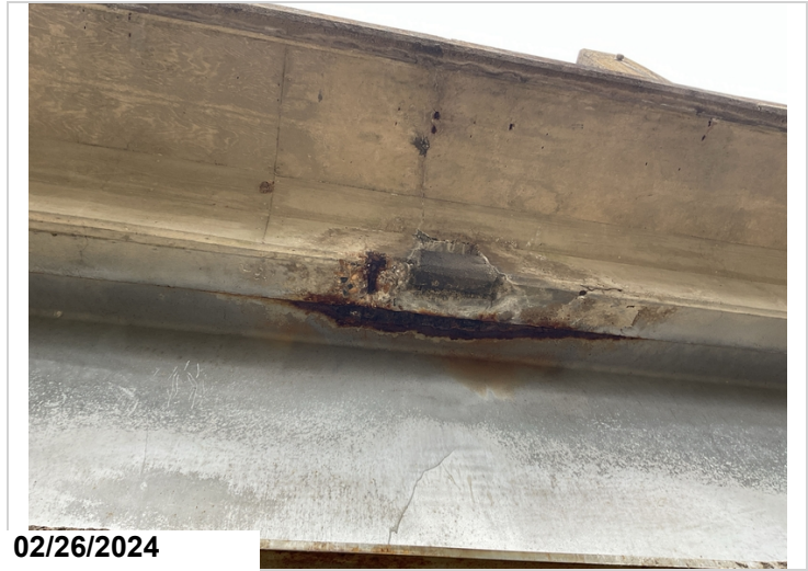
Main span 1, Underside of deck at right side, Rebar exposed at drain, 1 Sq Ft, CS3
