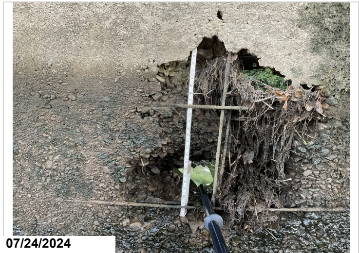
Pier 5: at the centerline of the pier a large spall with exposed rebar that is believed to be a previous location for utility pipe. (1 1/2' x 1') CS4-1'
