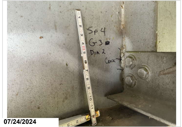
Span 4, girder 3, diaphragm 2: a 2" crack in the weld. CS4-1'
