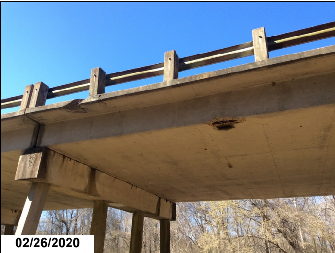
Span 19 spall at drain and over hang spalled and cracked Lt side
