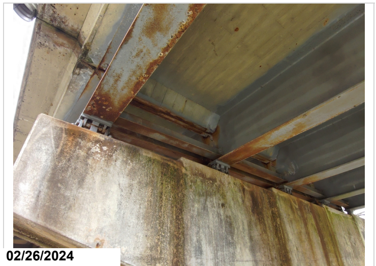
Various locations of beam end corrosion, CS2.
