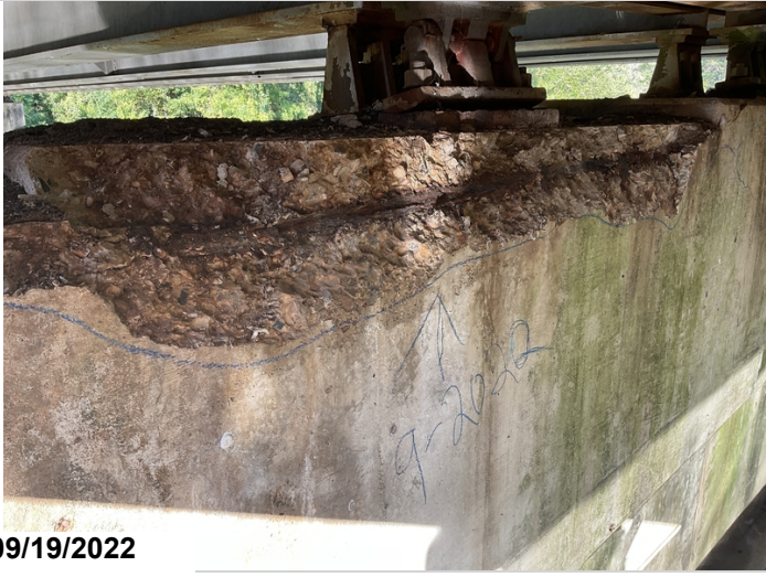
Main span, Pier 2, Rebar exposed near bearing area, CS3
