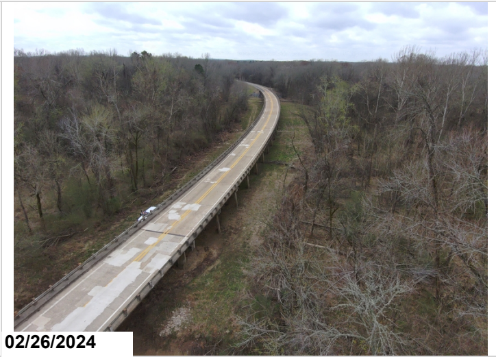
Approach span, Deck patching, CS2
