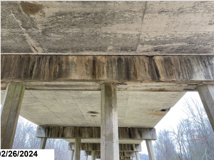
Approach span, Bent 6, Pier Cap, Looking ahead, Delam above pile 3, 1 LF, CS2
