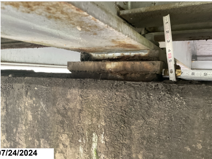
Bent 2, span 2, girder 4: bearing with some pack rust. Worst case.
