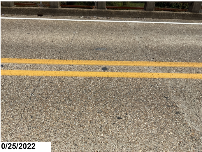
Typical cracking.
