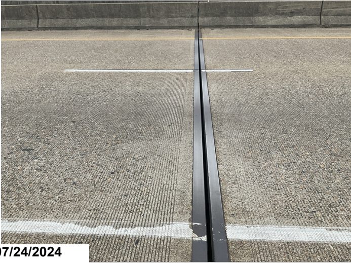
Bent 3: entire compress seal has fallen out.
