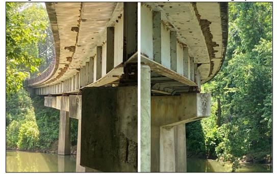
Figure 6-3: Cliff Swallow Nests on the I-49 Ramp off of I-40 over Frog Bayou
