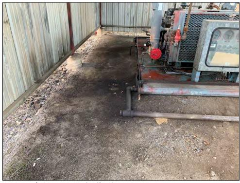
**Photo 29:** View of oil staining around wellhead compressor at Merit Energy Company, LLC USA 1-34.
