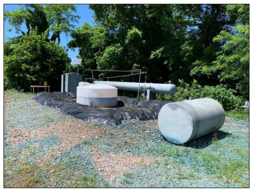
**Photo 13:** View northwest of produced water tank and gas-water separator (**Exhibit 2 Map ID #19**) near Cazort #5 and #8 wells. Green herbicide staining also visible.
