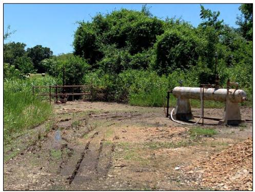
Photo 3: View west/southwest of Brown 1-1 wellhead (Exhibit 2, Map ID #3) with gas/water separator.
