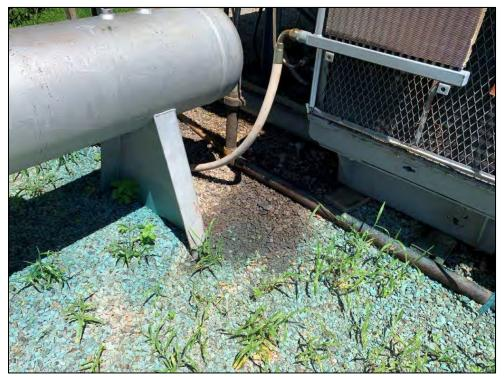
**Photo 14:** Oil staining below compressor at location above. Green herbicide staining also visible.
