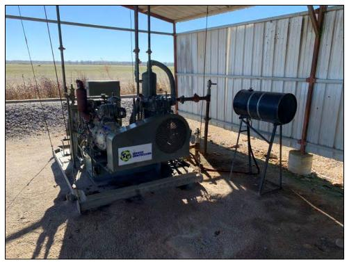
Photo 20: Well head compressor near Tibbitts #5-11 well head (Exhibit 2, Map ID #8). Some stained gravel evident.
