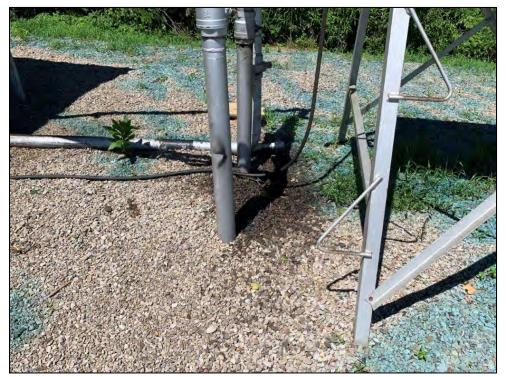
Photo 16: Oil staining below AST at location above. Green herbicide staining also visible.
