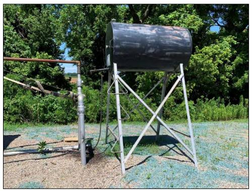
Photo 15: Diesel AST at compressor station near Cazort #8 well (Exhibit 2 Map ID #19). Green herbicide staining also visible.
