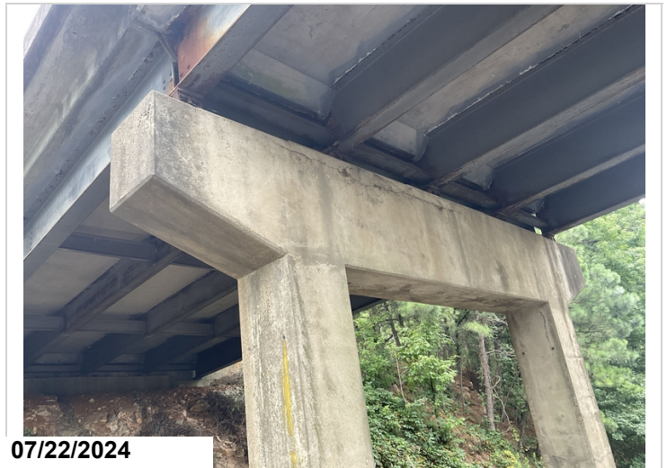
Bent 4 crack on backside. CS3
