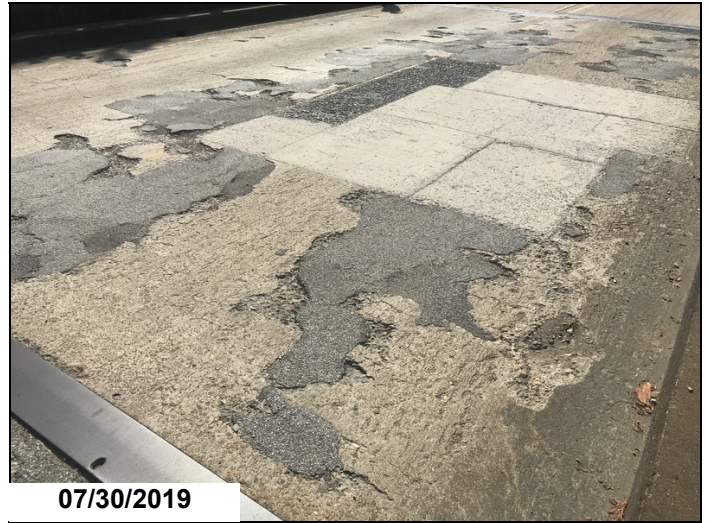
Span 4 has large spalls, spalls with asphalt and large patched areas
