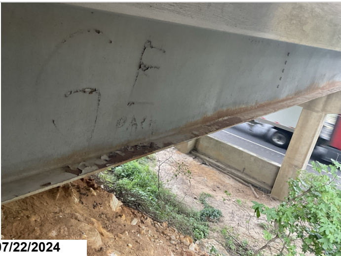
Span 4 girder 1 paint condition
