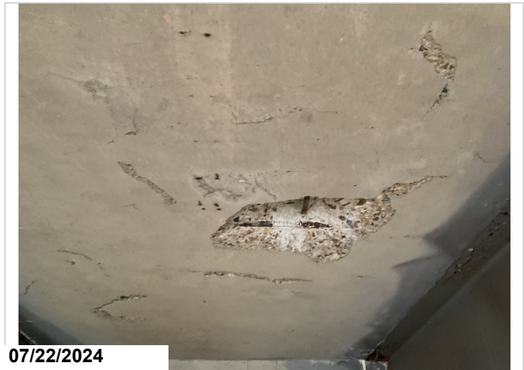
Span 4 bay 4 at bent 5, spall with exposed rebar in under surface.CS3
