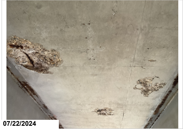
Span 1 bay 1 spalls with exposed rebar on under surface. CS3
