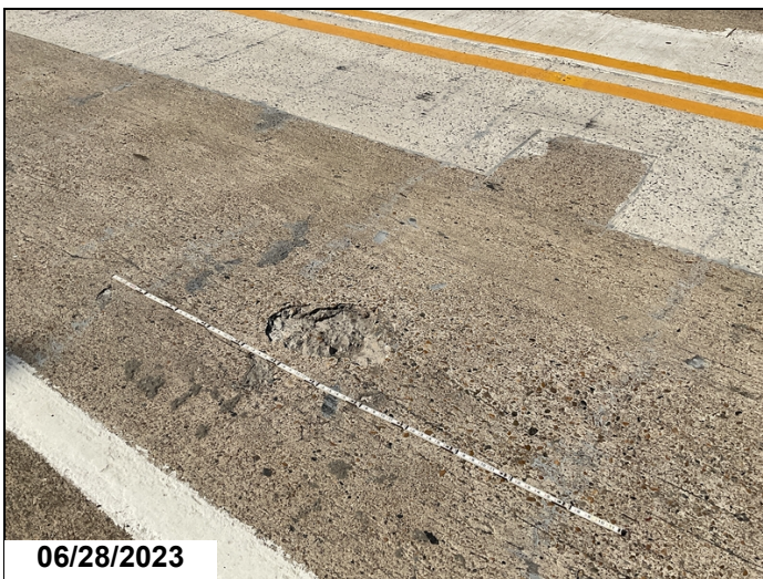
Span 1: open spall 2023
