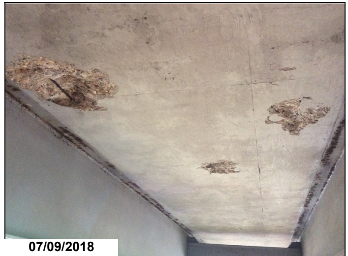
Span 4 spall with exposed reinforcing steel at center line.
