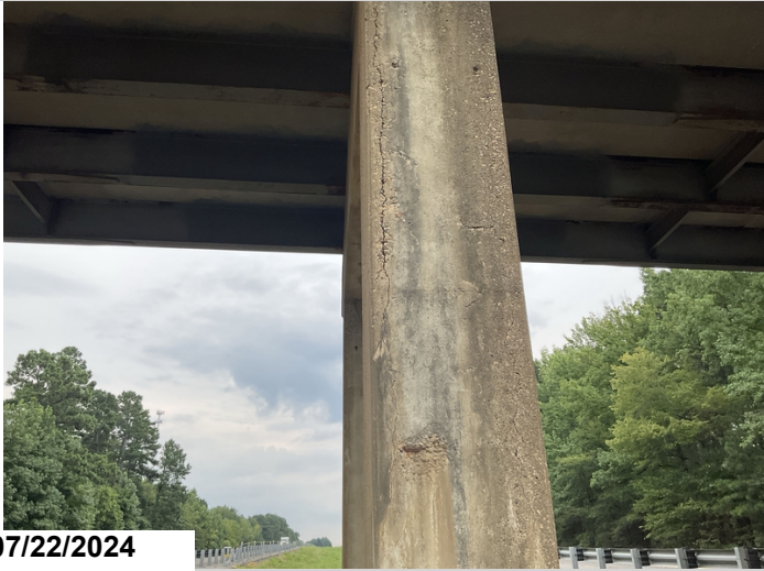
Bent 3 column 2, large crack on corner up to 1/4" and spall with exposed rebar. CS3
