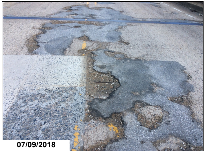
Span 4 spall with exposed reinforcing steel at center line.
