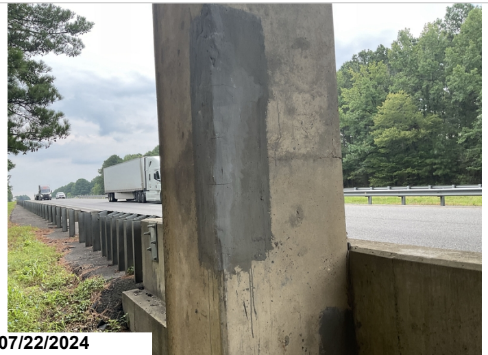
Bent 2 column 1, spalls have been patched. Common column 2. CS2
