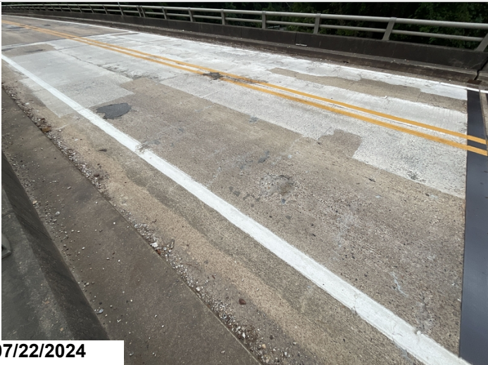
Span 1, spall with exposed rebar, spalls filled with asphalt and patched area. CS2 CS3
