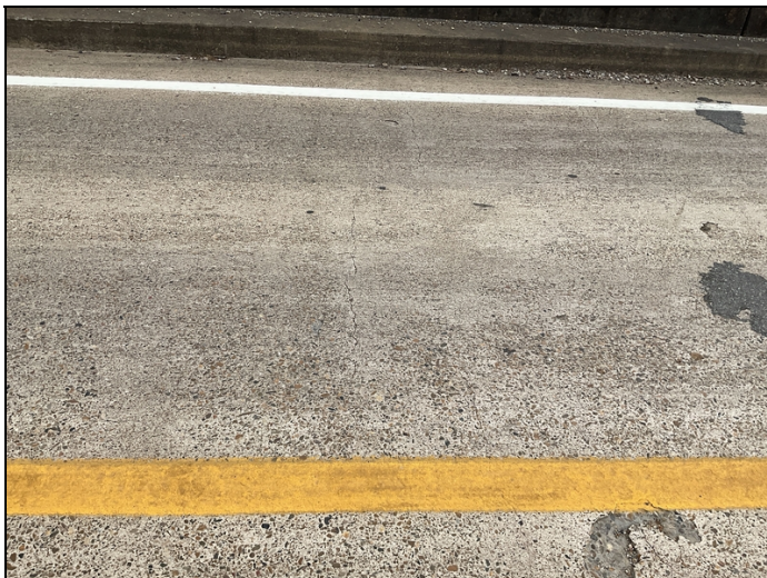
Span 2 unsealed transverse cracks up to 0.080". CS3
