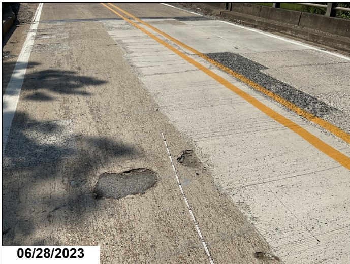
Span 4: couple of open spalls and spalls filled with asphalt. 2023
