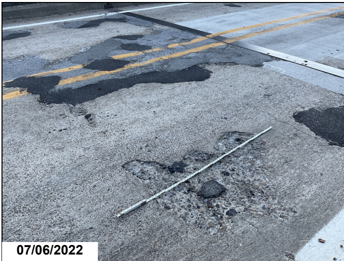
Span 3: couple of large open spall in the travel lane. 2022
