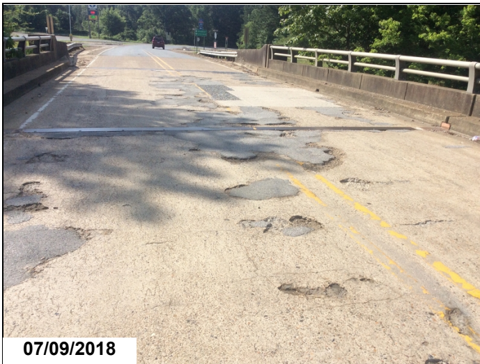
Span 3 failed asphalt patches.
