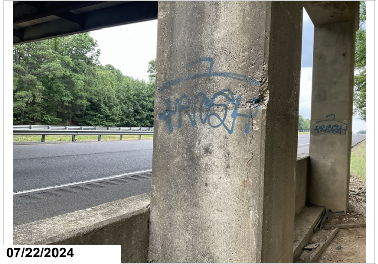
Bent 4 column 2, spall and crack up to 0.060" CS3
