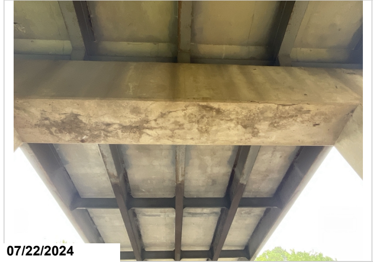
Bent 4 crack in between columns. CS3
