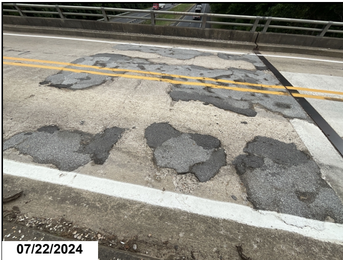
Span 3 at bent 4, numerous spalls filled with asphalt. CS3
