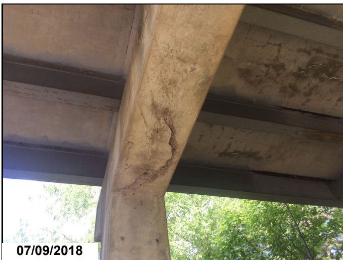
Large spall and delaminated area at bent 2 underside of cap.
