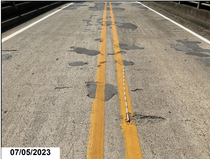
Span 3: numerous open spalls and large unsealed transverse cracks. 2023
