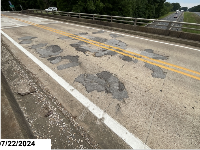
Span 2, spalls, spalls filled with asphalt and patched area. CS3
