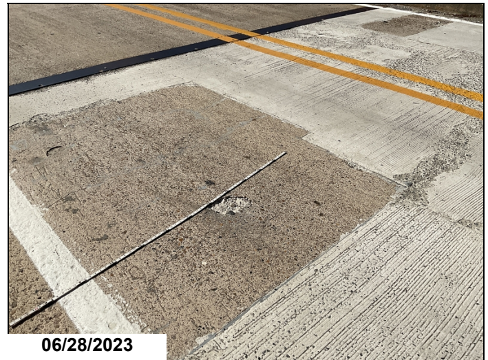
Span 1: small open spall in the right lane. 2023
