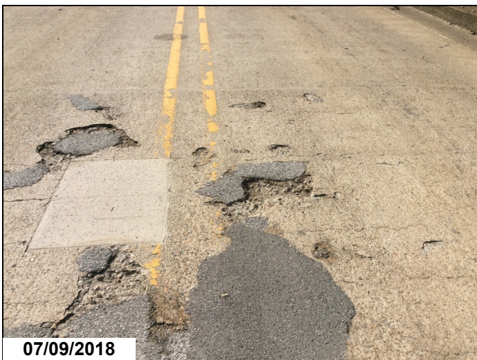
Span 3 right lane spall with exposed reinforcing steel.
