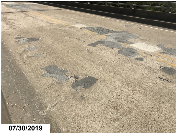
Span 2 has large spalls filled with asphalt and large patched areas
