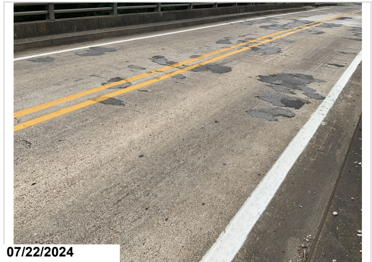
Span 3, spalls, spalls filled with asphalt and patched area. CS3
