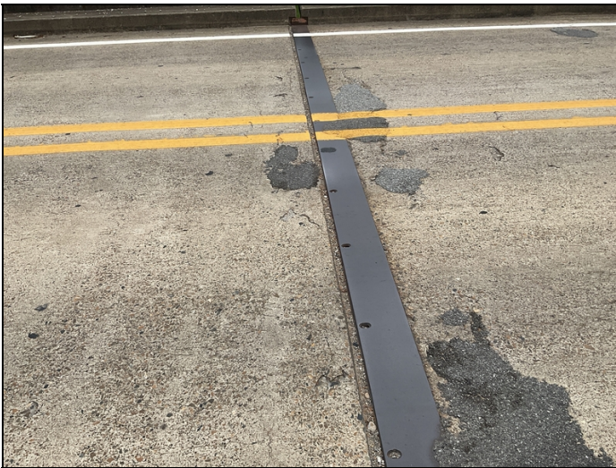
Bent 3, joint is half full of debris
