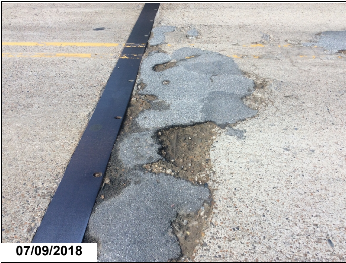
Span 1 left lane spall with exposed reinforcing steel.
