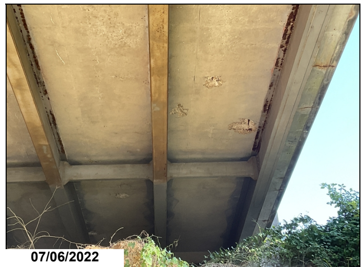
Span 1: few spalls in the soffit
