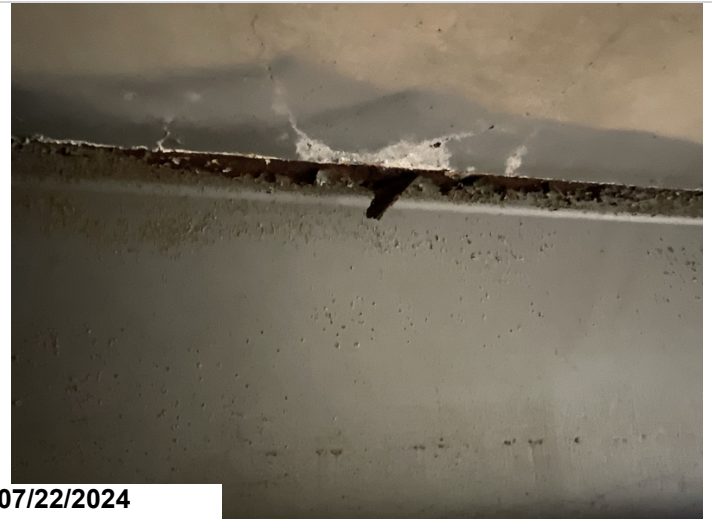
Span 4 girder 3 corrosion with minor section loss to top flange. CS3
