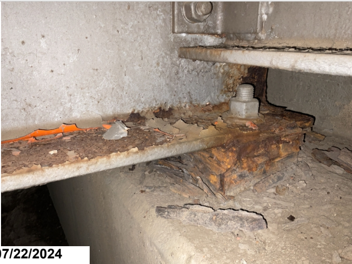
Span 4 girder 2 at bent 5, laminating rust with section loss on girder end. CS3
