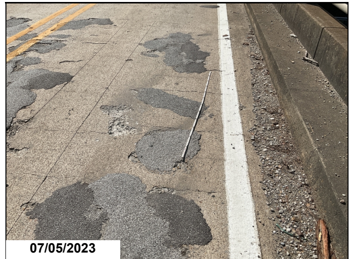
Span 2, right lane: numerous spalls and large unsealed transverse cracks at average 3' spacing. 2023
