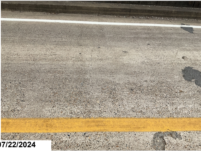
Span 2 unsealed transverse cracks up to 0.080". CS3
