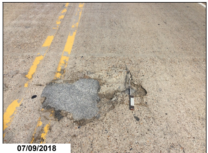
Span 3 has 6' of spall with exposed reinforcing steel at center line.
