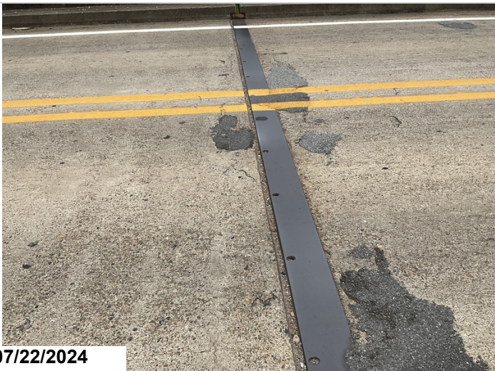
Bent 3, joint is half full of debris
