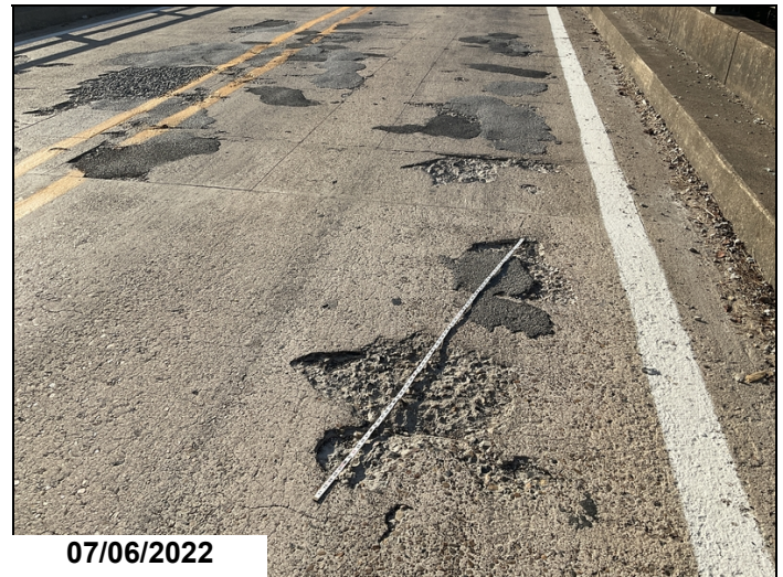
Span 2: Multiple large open spalls. 2022
