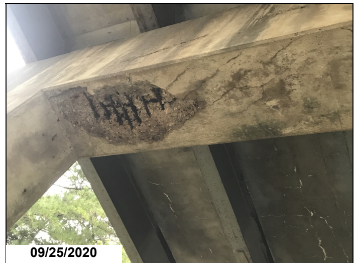
Bent 2 cap bottom has spall with exposed rebar.
