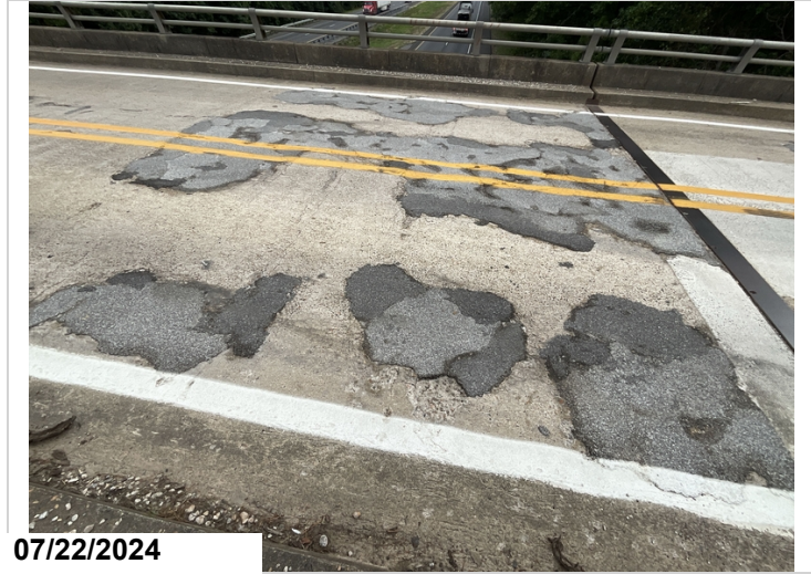
Span 3 at bent 4, numerous spalls filled with asphalt. CS3
