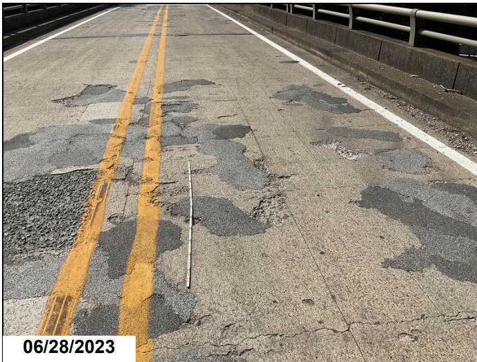
Span 2: numerous spalls filled with asphalt and open spalls. 2023
