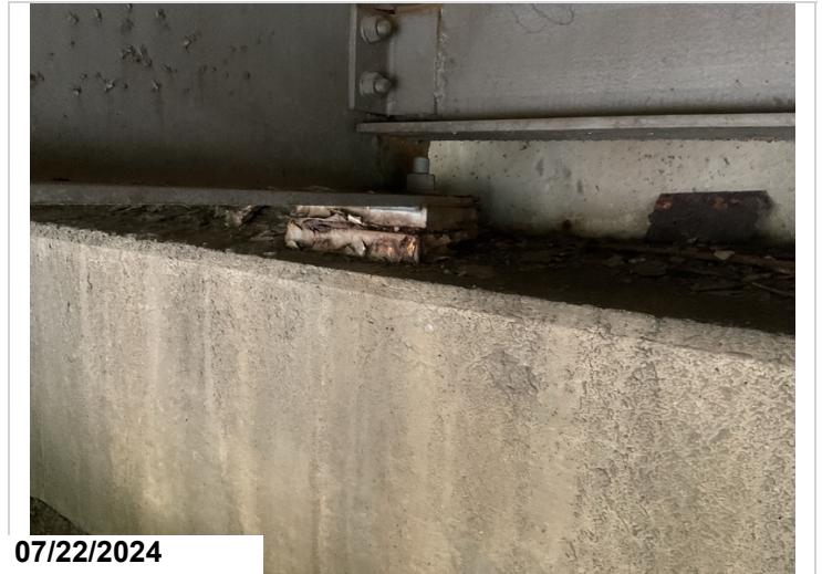
Bent 5 bearing 3, laminating rust. CS3
