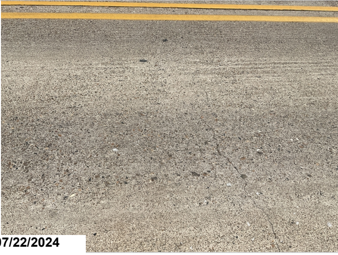
South Approach slab, transverse crack up to 0.070". CS3
