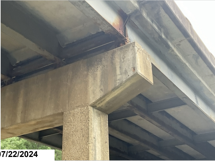
Bent 3 back right corner of cap has a delam. CS2
