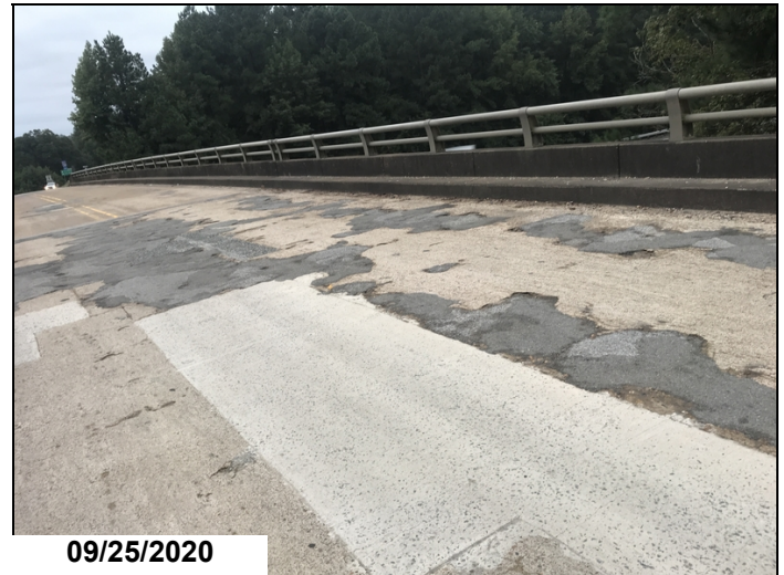
Spalls and spalls filled with asphalt in deck span 1.
