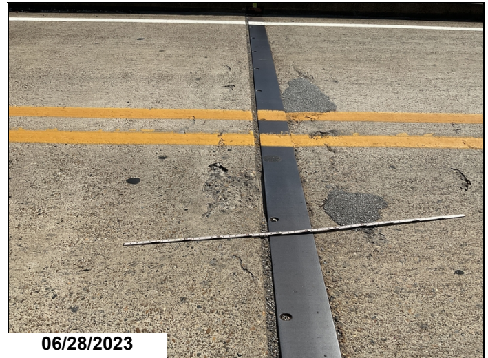
Span 2 at bent 3: spalls adjacent to the joint. 2023
