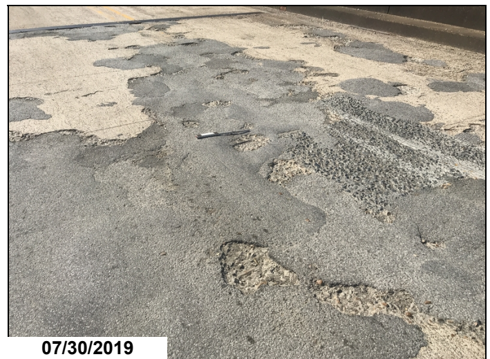
Span 1 has large spalls, spalls with asphalt and spalls with rebar
