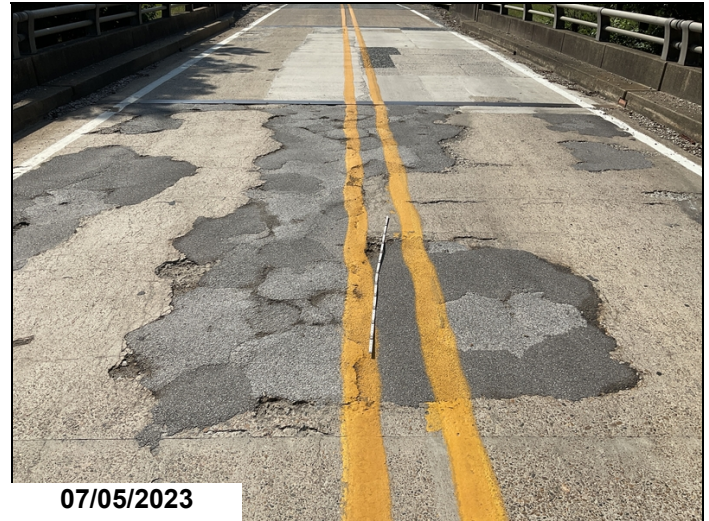
Span 3: Approximately 260sf of spalls filled with asphalt. 2023
