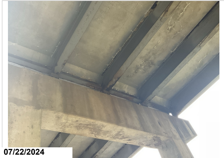
Bent 2, span 1, all girders have measurable section loss to the upper web at the haunch, lower web and bottom flange. CS3
