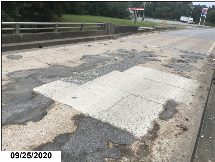
Span 4 deck has spalls and spalls filled with asphalt.
