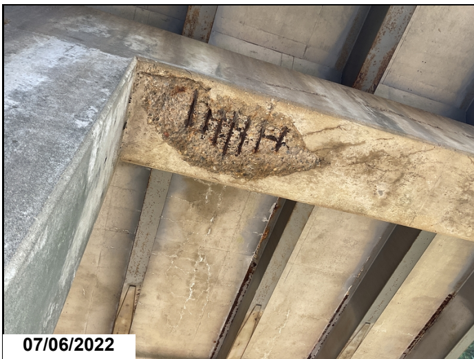
Bent 2: large spall with exposed rebar at the bottom of cap.
