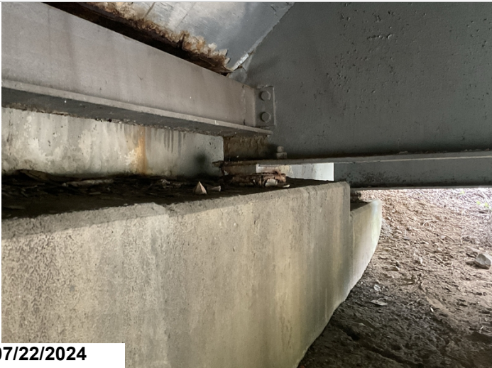
Bent 5 girder 4 has a broken anchor bolt.
