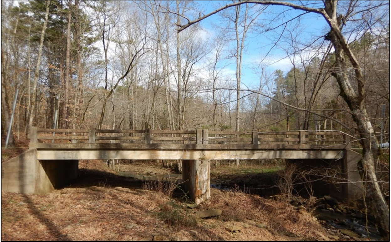
ARDOT Highway 215 Bridge over Wolf Pen Creek (facing upstream)
