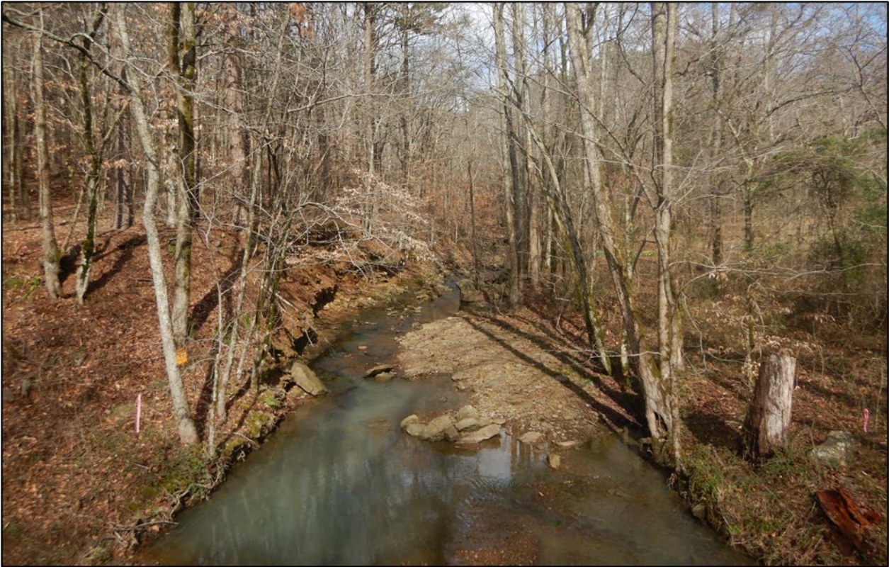
View from Bridge (facing north) upstream
