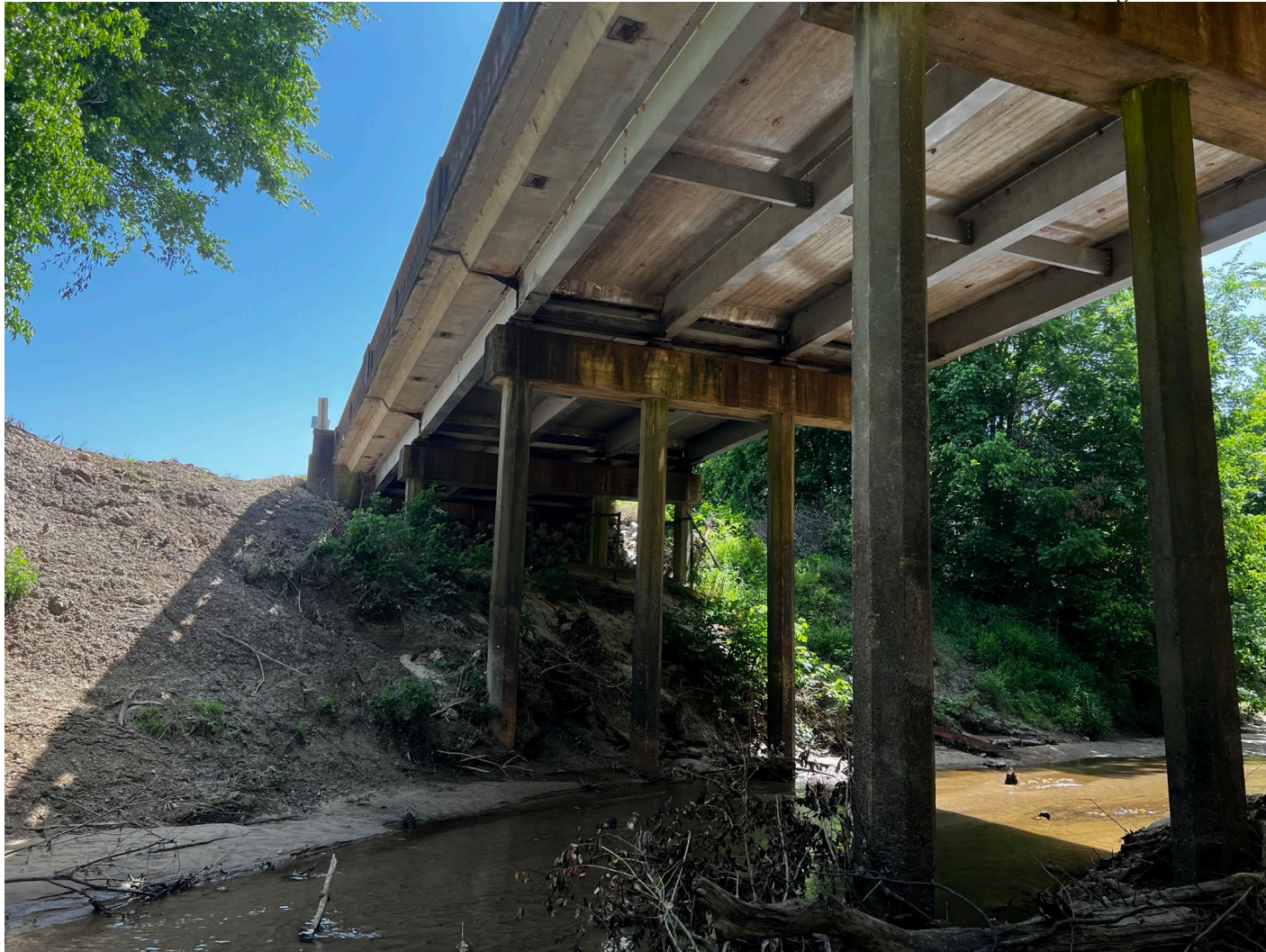
Site 2-Locust Creek slope at the north abutment
