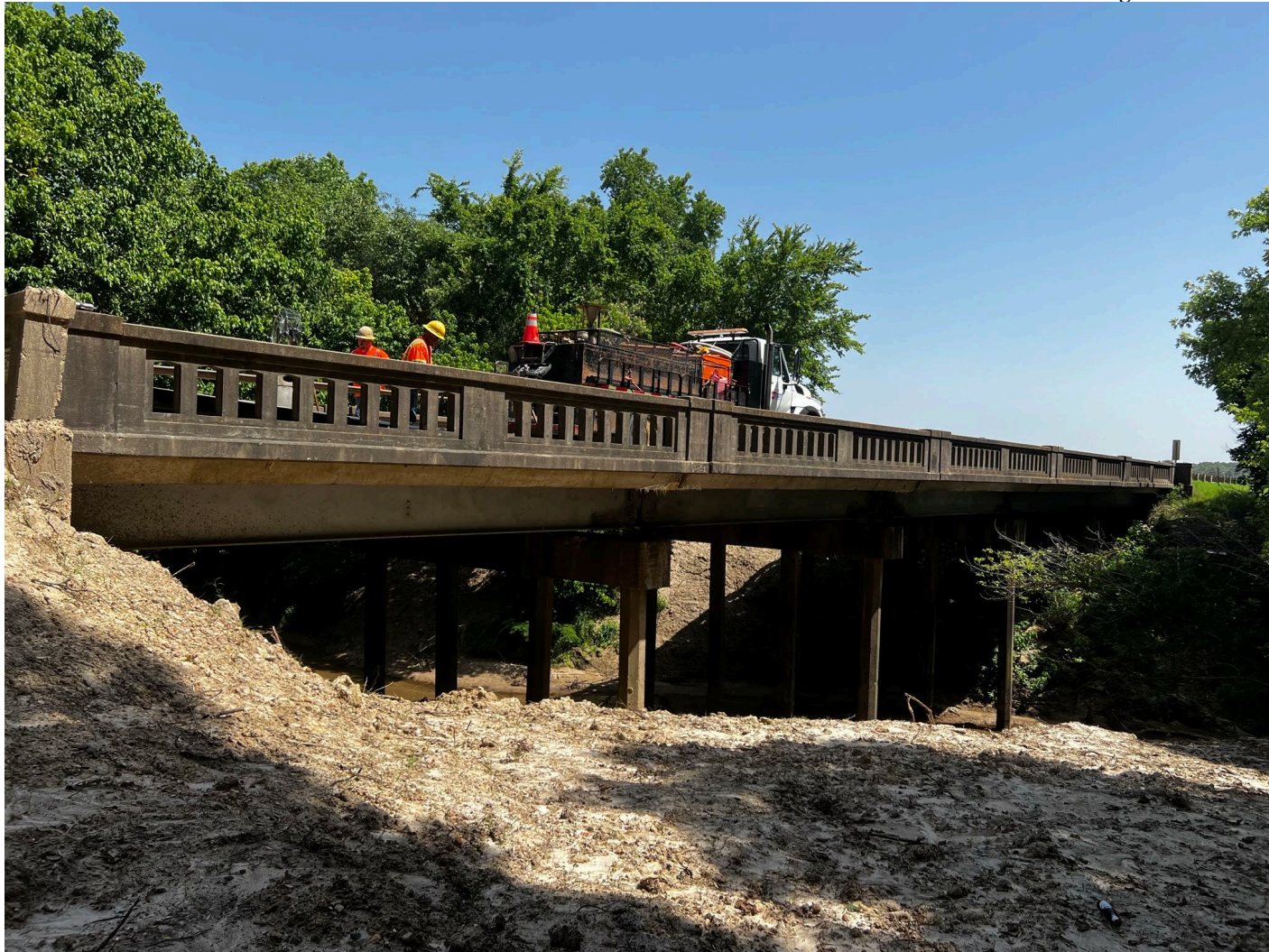
Site 2-Locust Creek east side of the bridge (June 2022)
