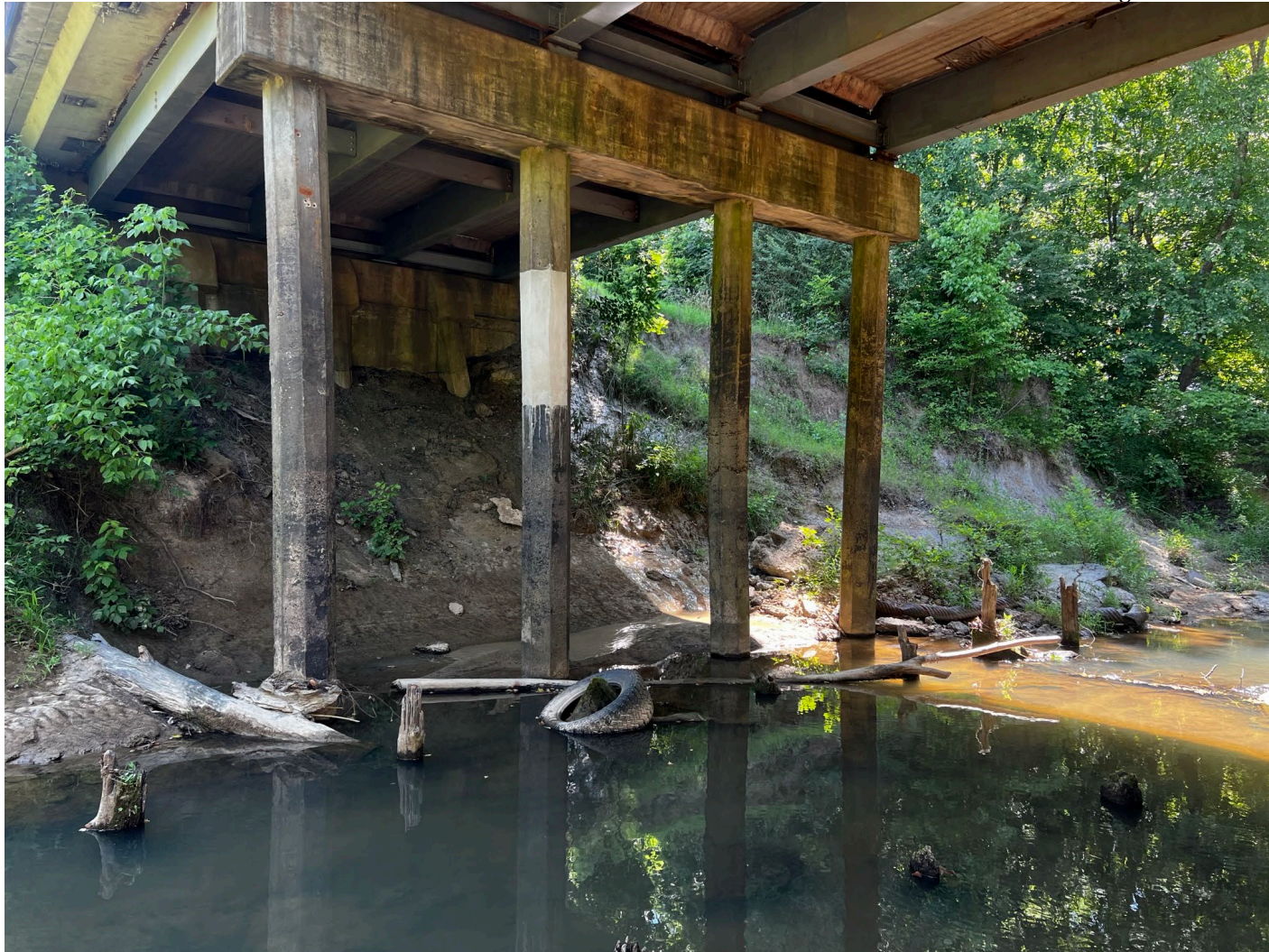
Site 1-Jacks Creek north end bridge abutment (June 2022)
