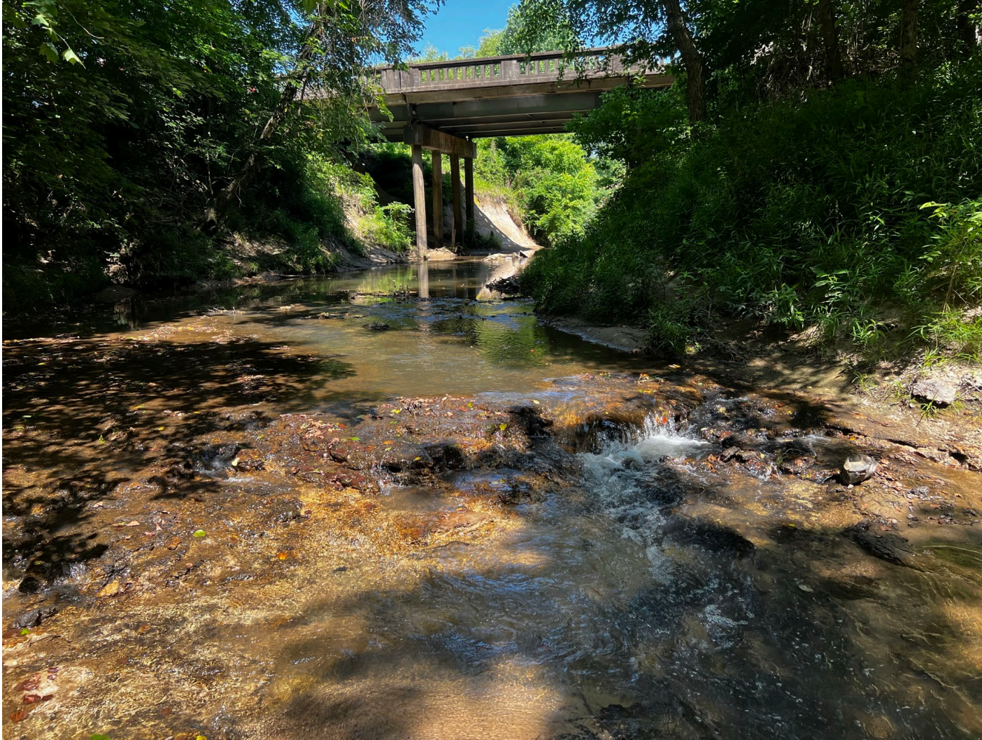
Site 1-Jacks Creek looking west (upstream) at the east side of the bridge (June 2022) Silty Clay exposed in channel
