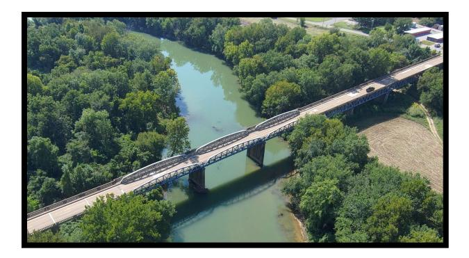
ARDOT Bridge Number 01984 currently carries State Highway 62 over the Spring River and BNSF Railroad north of Imboden. C.F. Lytle, of Sioux City, Iowa, constructed the bridge in 1937. It has six main spans: three Parker pony truss spans and three Pratt deck truss spans. Each truss span is approximately 112 feet long (for a total length of 672 feet) and 24 feet wide.
