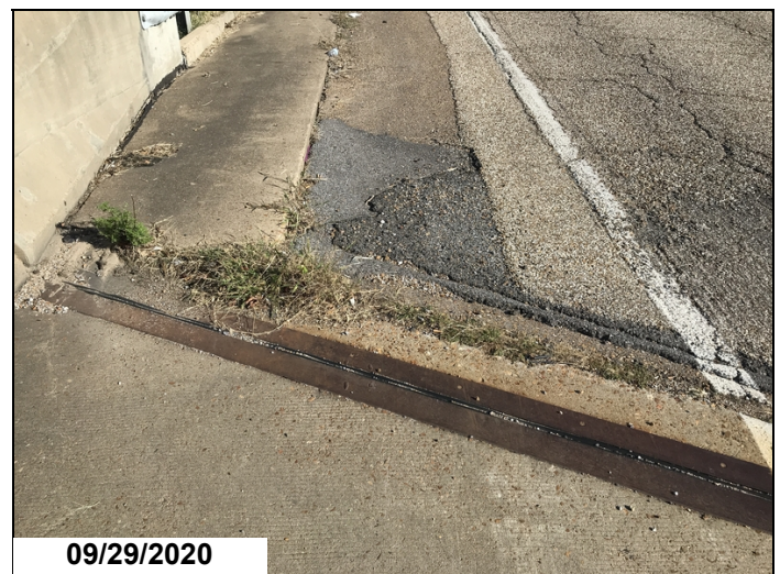
Abutment 2 left approach shoulder has settled 2 " at bridge end.
