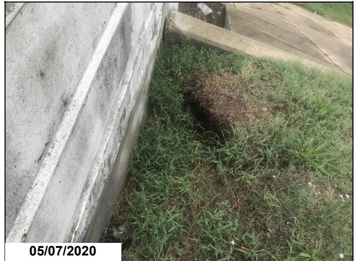
Hole at abutment #2 left side
