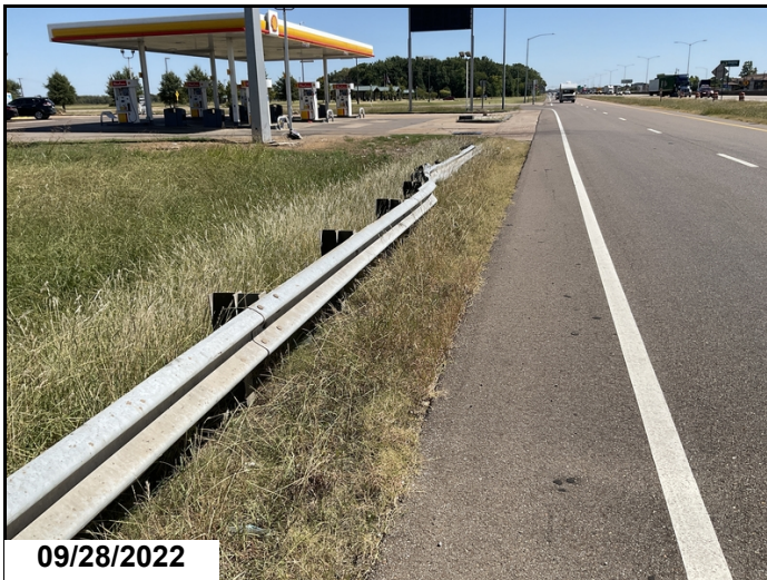
West bound service road right approach rail has collision damage
