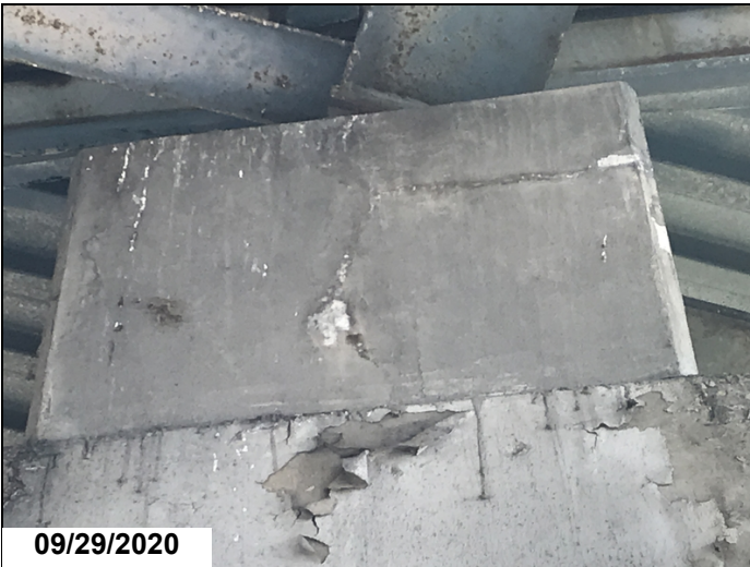
Typical vertical crack on bearing risers.
