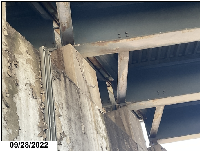
Bent #6 girder 8 riser on back face has two foot delamination.
