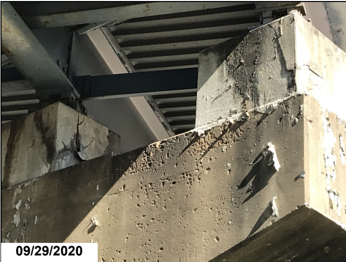
Bent #3 cap back face bearing risers girders #9,10 right sides are cracked and delaminated.
