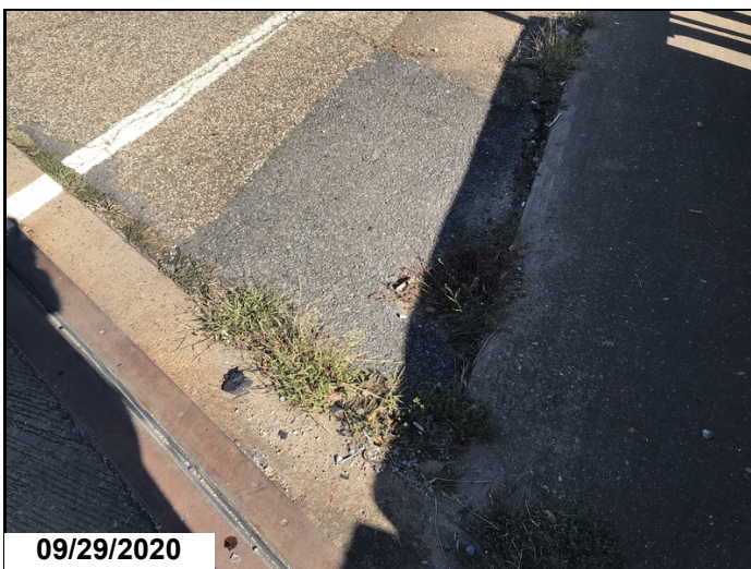
Abutment 2 right approach shoulder has settled 2 " at bridge end.
