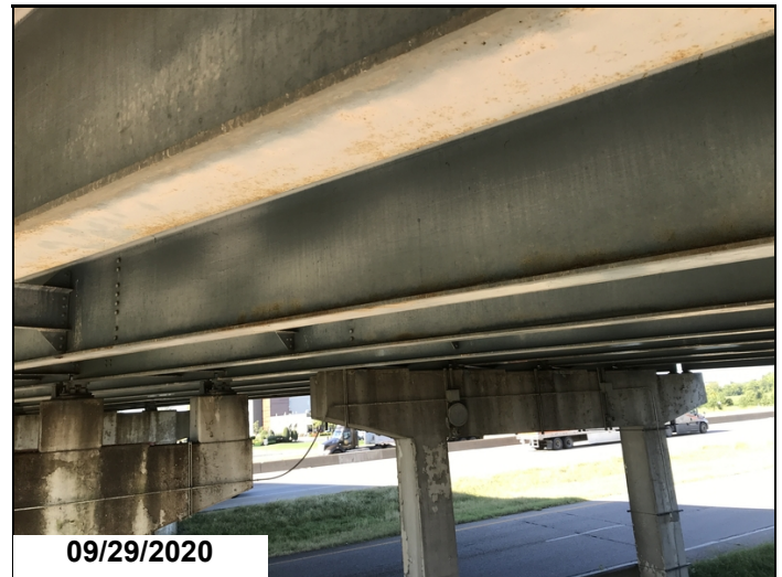
Typical interior girder paint condition
