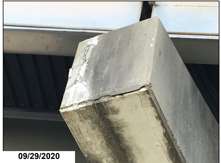
Bent #3 cap lt. end and back face of cap are cracked.
