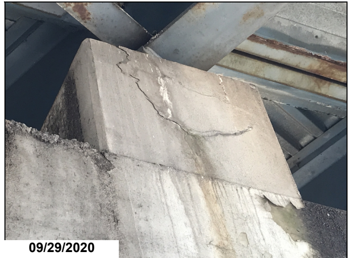
Bent #6 girder 8 riser on back face has 2' delamination.
