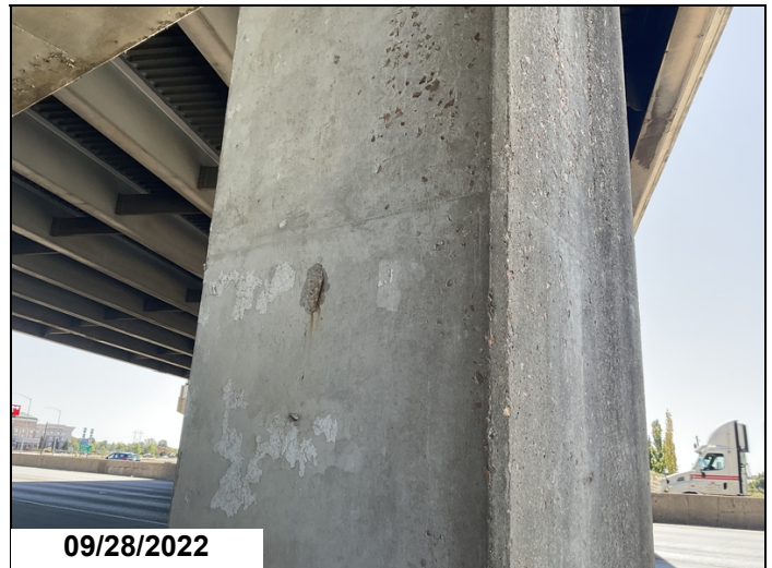
Bent #5 column #1 has six inch spall with exposed rebar on ahead face six feet up from ground no section loss.
