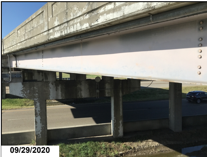
Typical outside girder paint condition.
