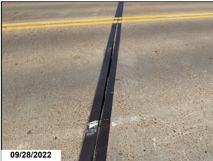
Bent #3 joint seal sagging
