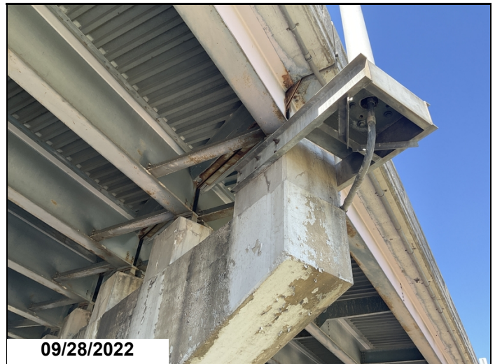
Bent #6 risers under girders #6, #9 and #10 are cracked on back face verticals.
