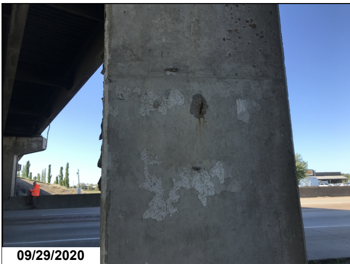
Bent #5 column 1 has 6" spall exposed rebar on front face 6' up from ground no section loss.
