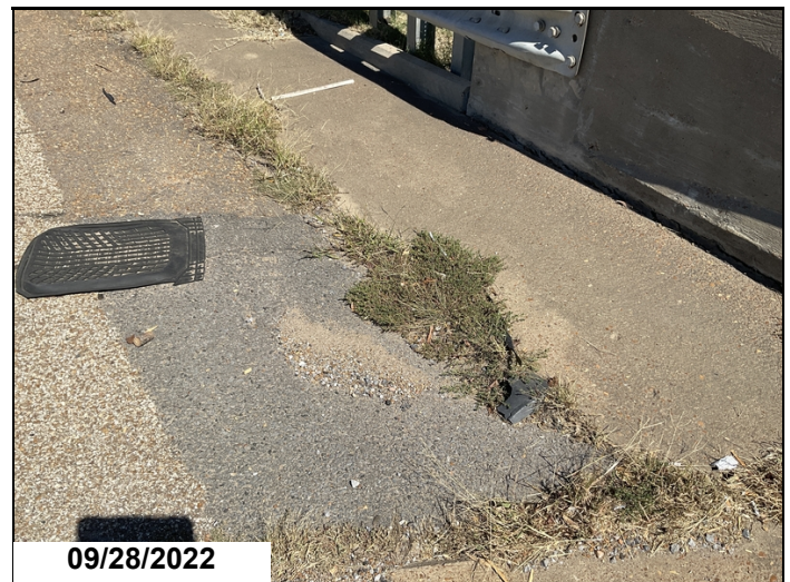
Abutment #2 right approach shoulder settlement
