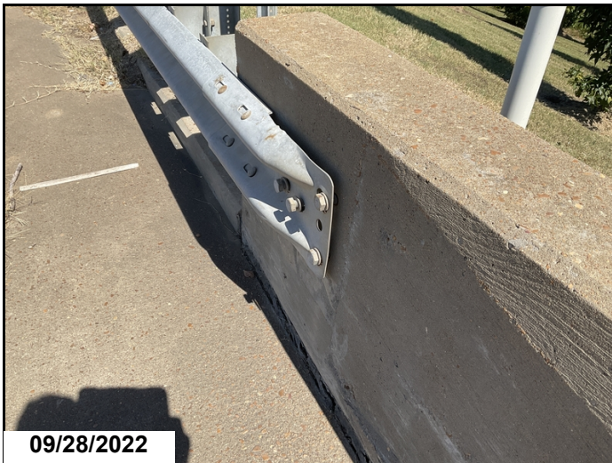
Loose bolts at abutment #2 right approach rail connection
