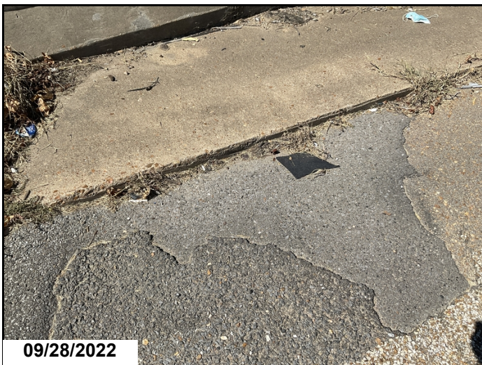
Abutment #2 left approach shoulder settlement
