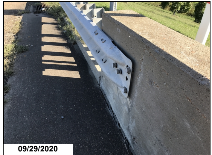
Abutment #2 rt. approach rail attachment to bridge has several loose bolts.
