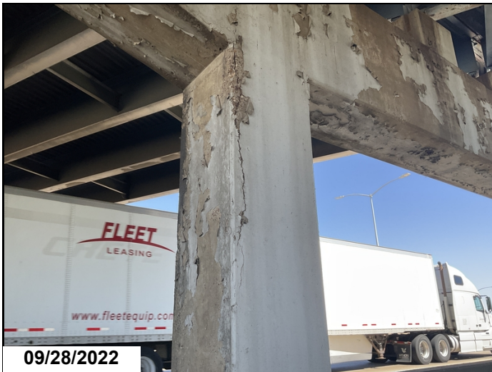
Bent #3 column #3 left back corner cracked and delaminated for five feet. Cs3
