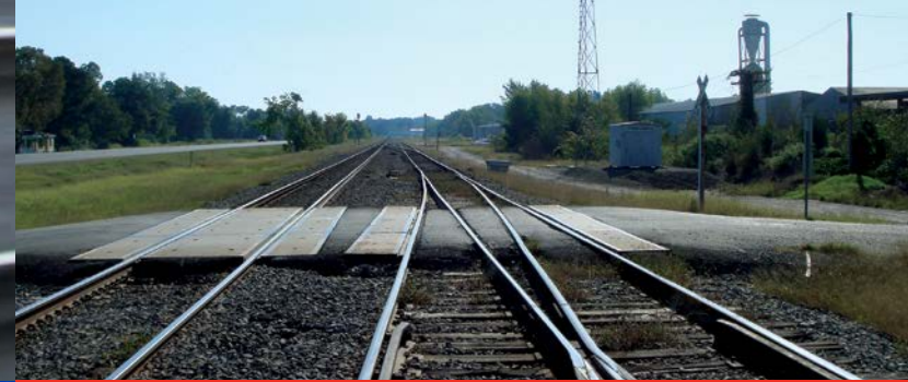
Multi-track surface on King Street in Lewisville, Arkansas.
