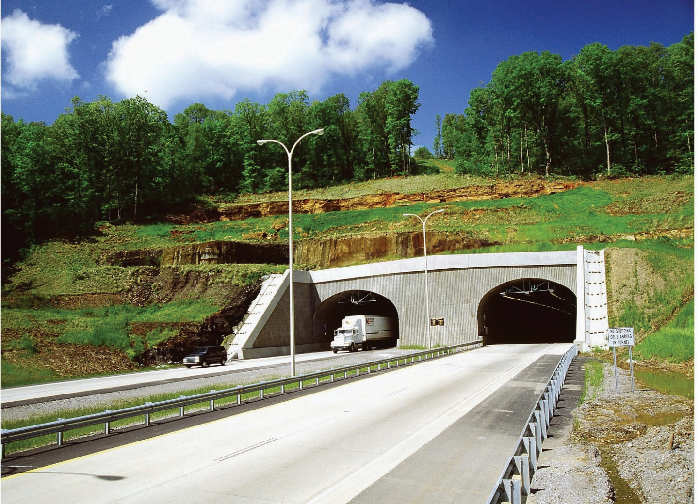
The Bobby Hopper Tunnel on Interstate 540 in Washington County
