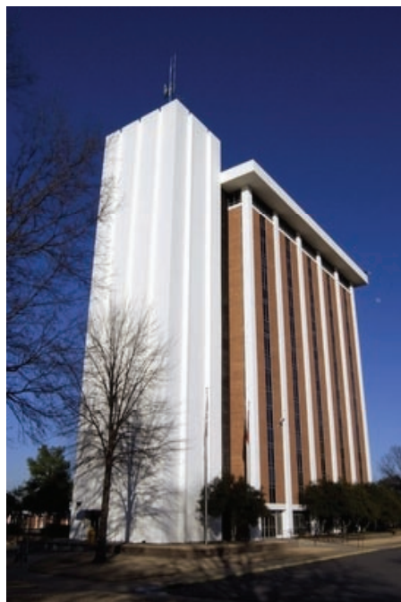
AHTD Central Office Building
