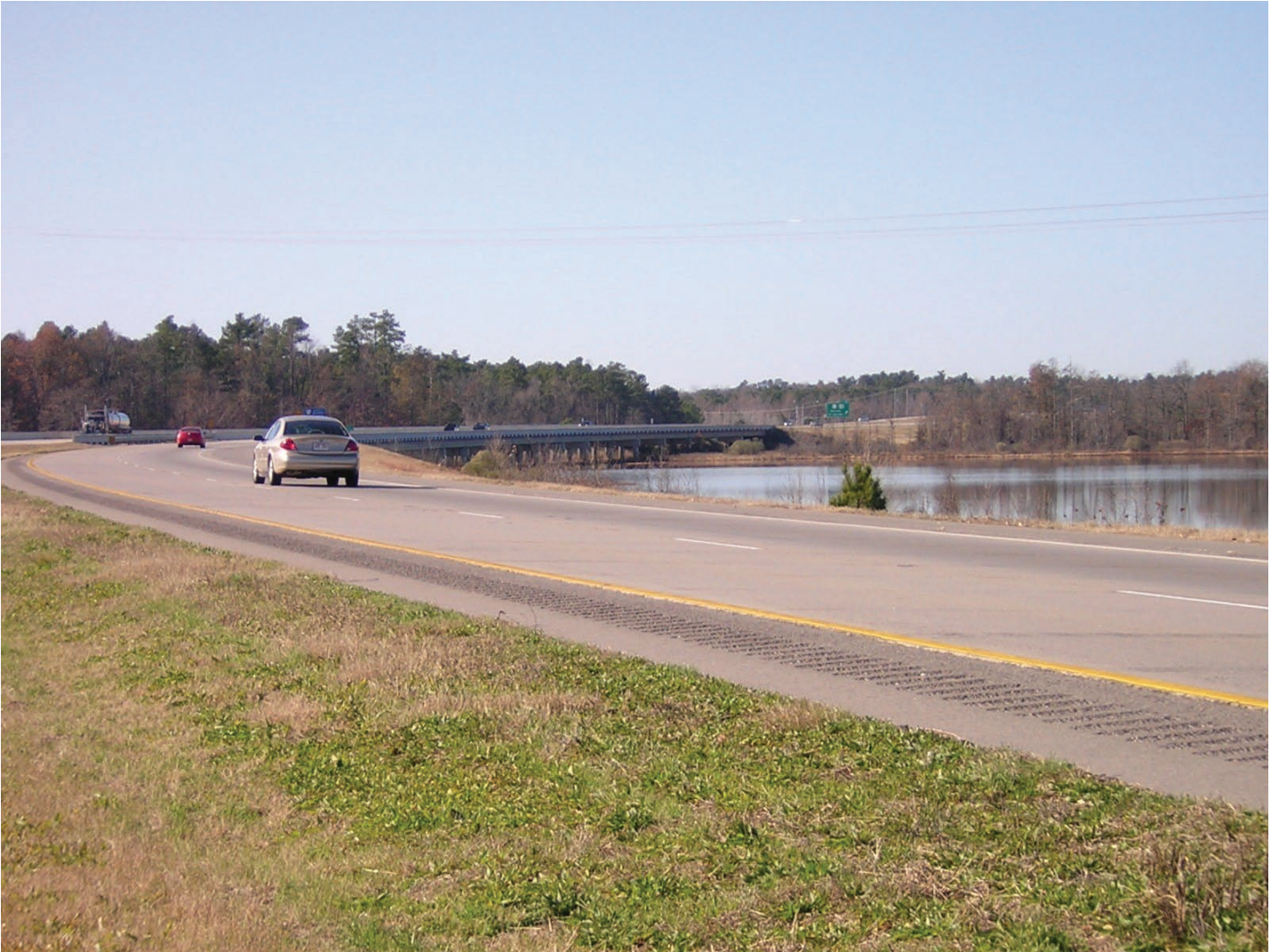
Interstate 530 in Pine Bluff, Jefferson County
