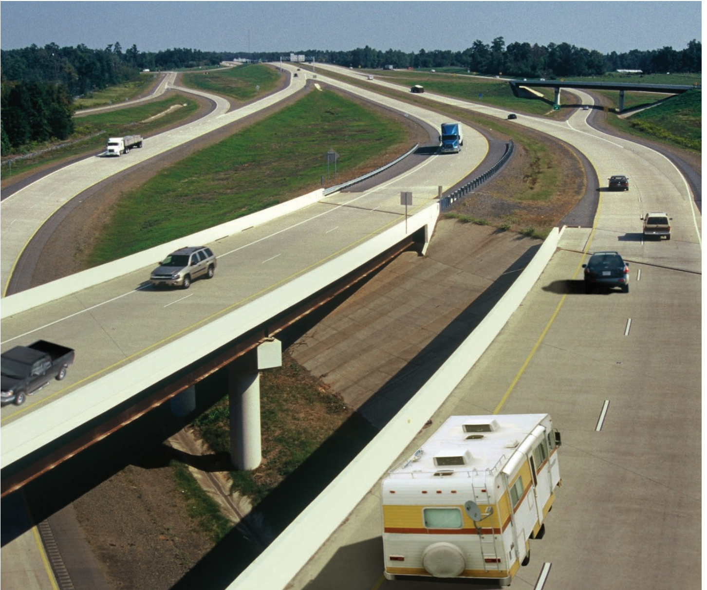
Highway 549 just south of Texarkana is part of future Interstate 49.
