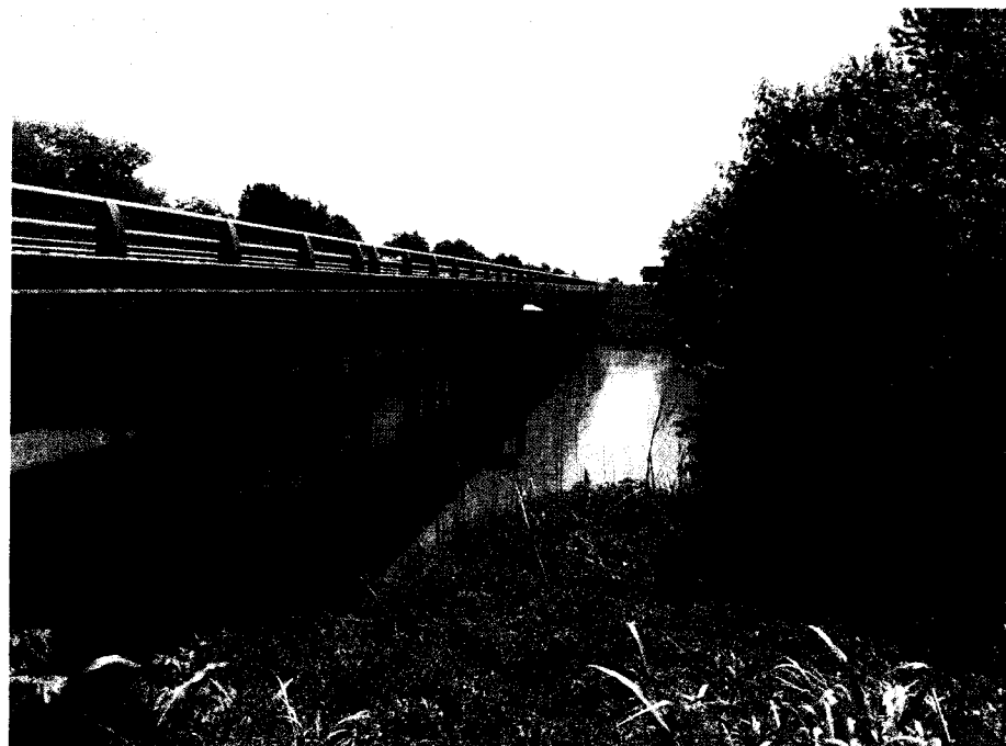
SITE NO. 1 - BRIDGE NO. A5189
