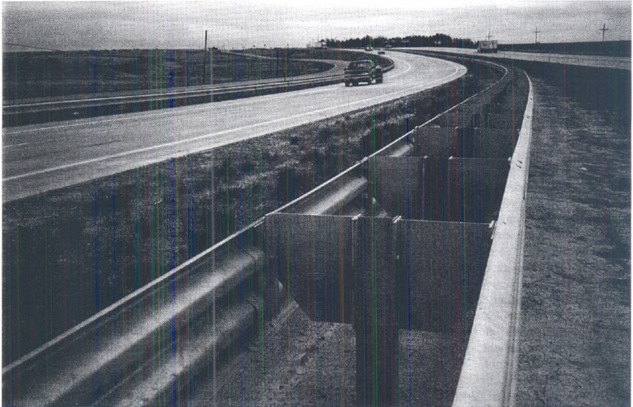
FIGURE 6.6 Modified thrie-beam median barrier
