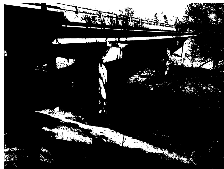
SITE NO. 6 - BRIDGE NO. A5311
