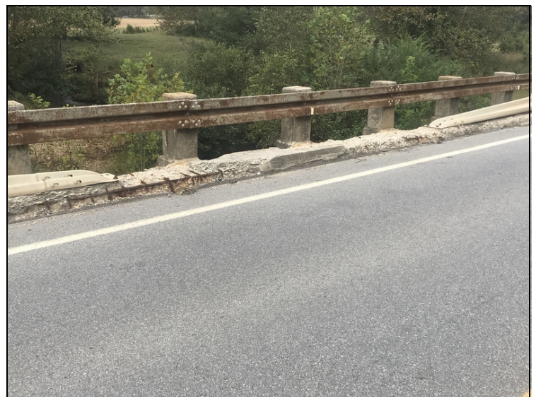
Heavy spalls & deterioration to Left & Right Curbs with rebar exposed.
