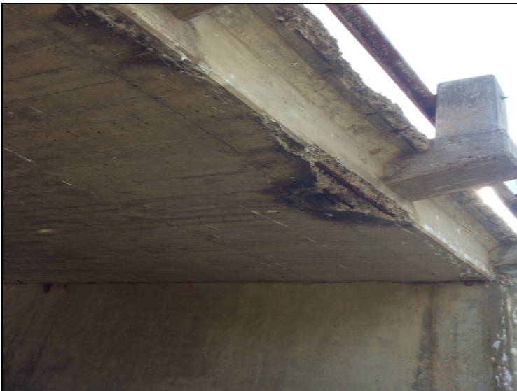
Span 1 - Large spalls & efflorescence cracking to Left Edge & Outside Edge of Deck below with rebar exposed.
