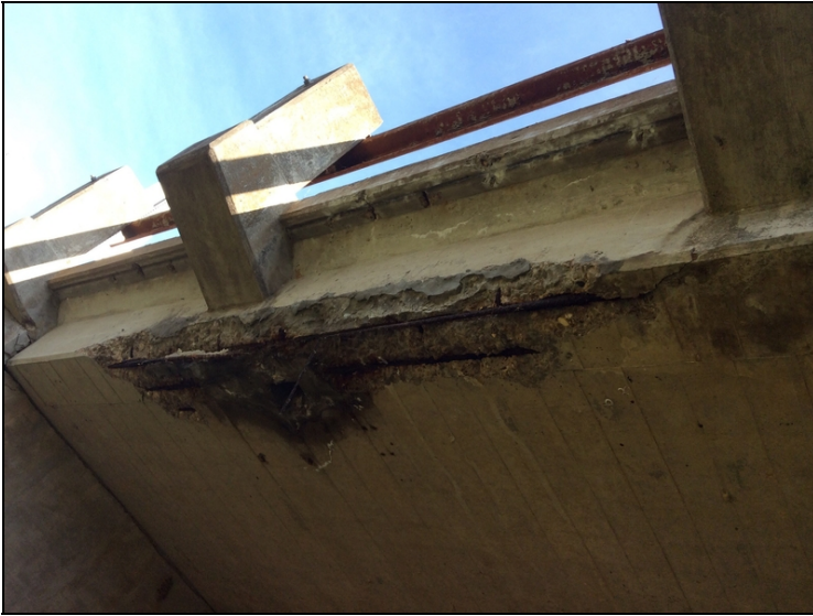
Span 3 - Large spalls & efflorescence cracking to Left Edge & Outside Edge of Deck below with 25' total rebar exposed with heavy section loss to Rebar @ Span 1.
