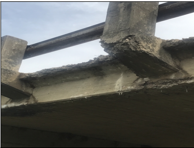
Efflorescence cracking & spalling to bottom of Concrete Guardrail Post & Outside Edge of Deck, some with rebar exposed. (Mostly on Left side)
