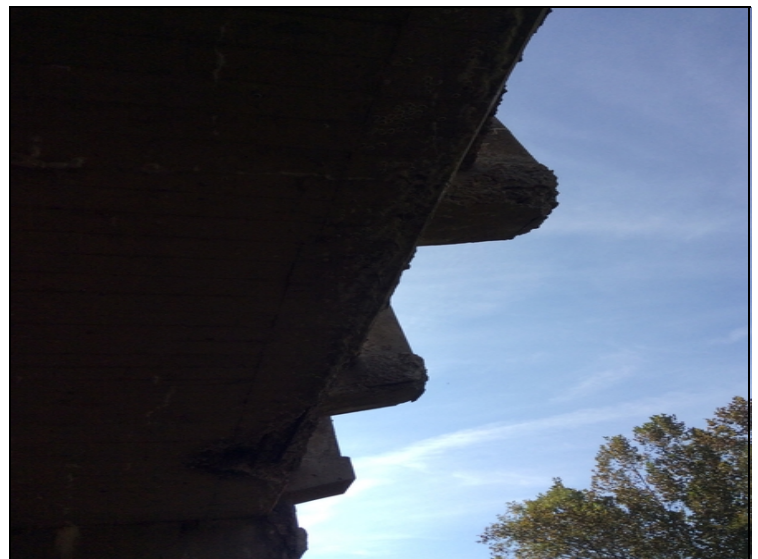
Span 2 - Large spalls & efflorescence cracking to Left Edge & Outside Edge of Deck below with rebar exposed.
