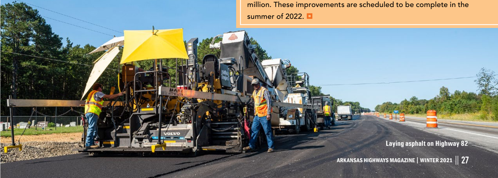
Leveling the surface on Highway 82
