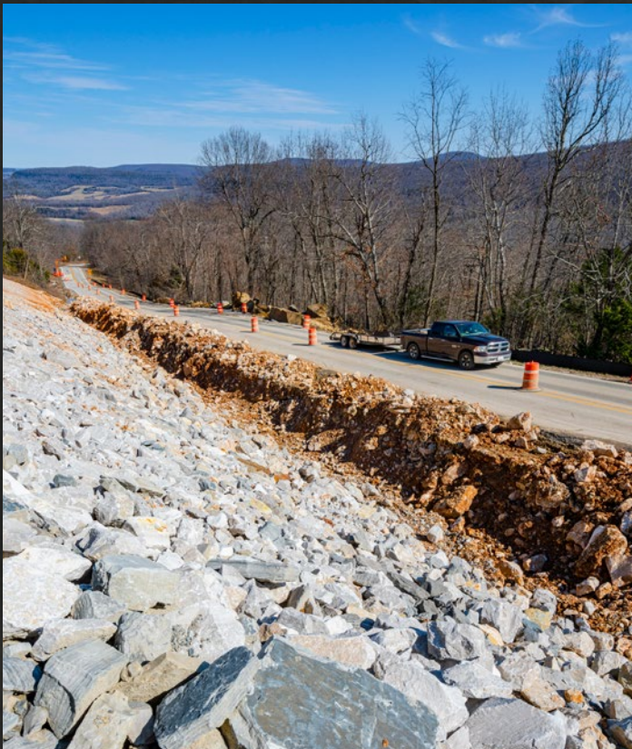
Rock buttresses are used to address slide issues.
