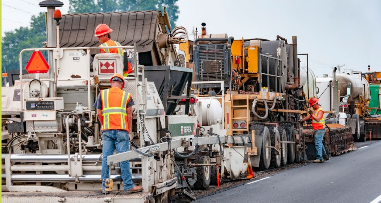
The equipment "train" only utilizes one travel lane.
