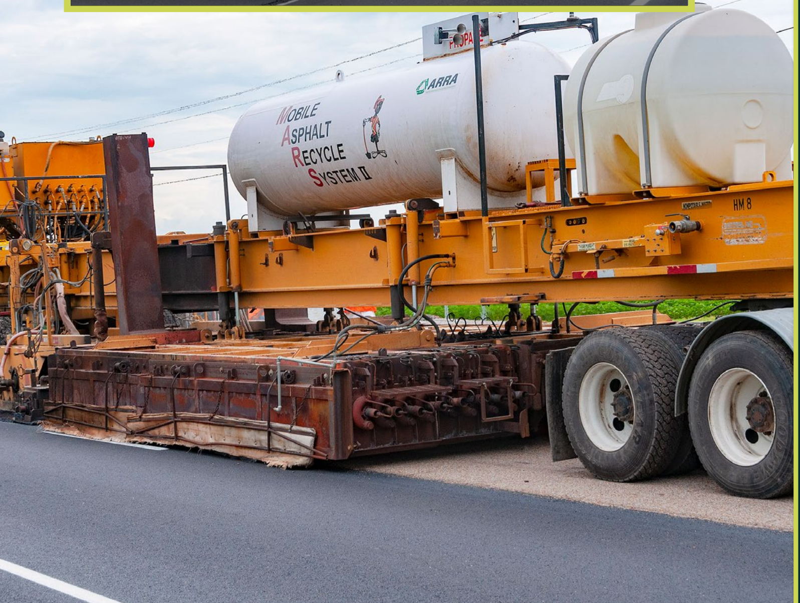
A propane-fueled preheater preps the road surface.
