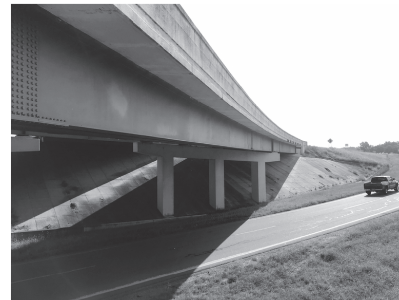
SITE NO. 5 - BRIDGE NO. B6273
