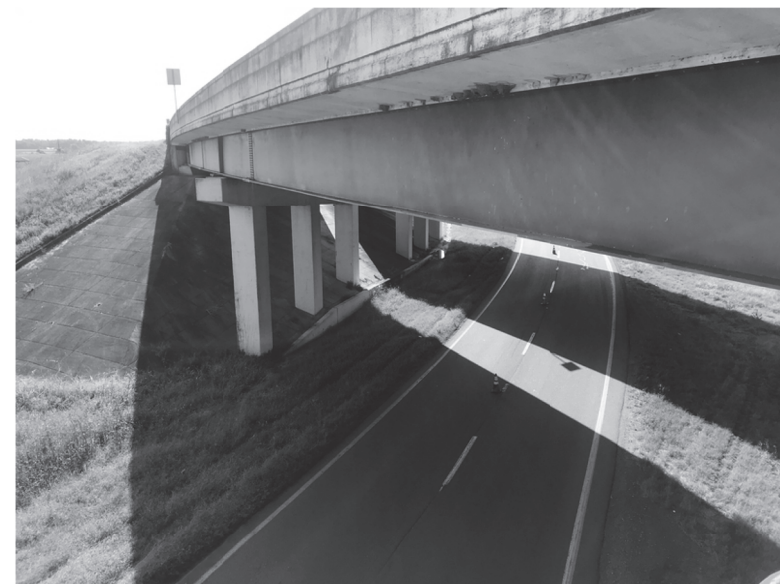
SITE NO. 4 - BRIDGE NO. A6273
