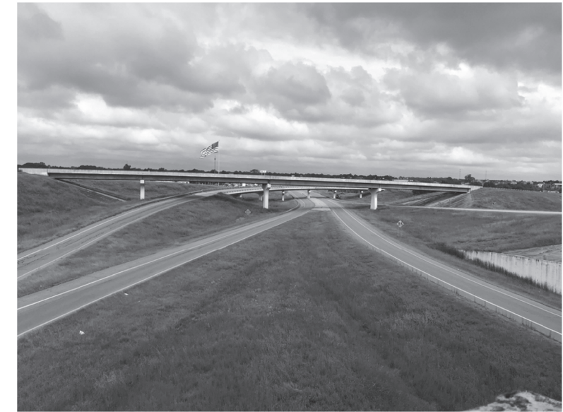
SITE NO. 3 - BRIDGE NO. 06275
