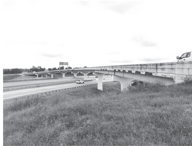
SITE NO. 2 - BRIDGE NO. 06274
