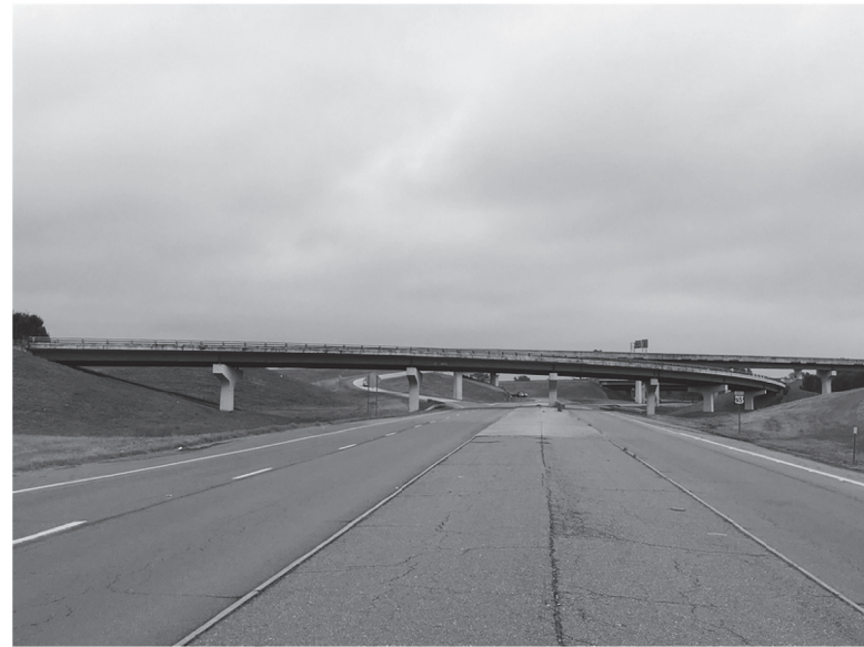
SITE NO. 1 - BRIDGE NO. 05422
