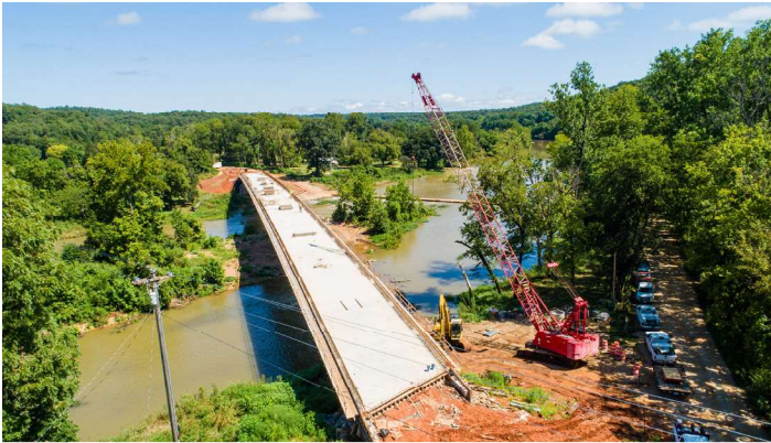
SPRING RIVER BRIDGE REPLACEMENT
