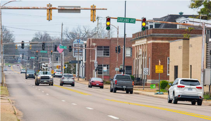
HIGHWAY 1B RESURFACING
