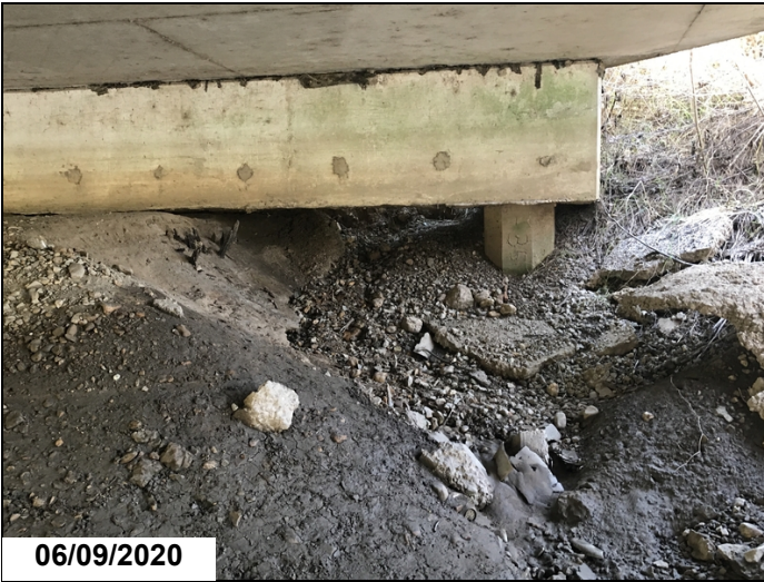
Bent 4 erosion RT SIDE 2019
