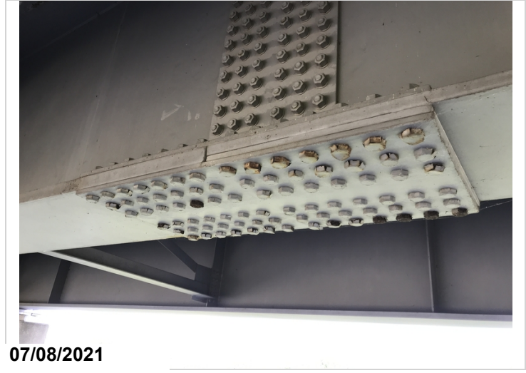
Typical paint flaking and corrosion at splice
