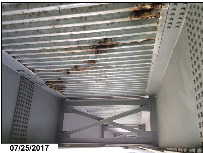
typical soffit under saw cut joints
