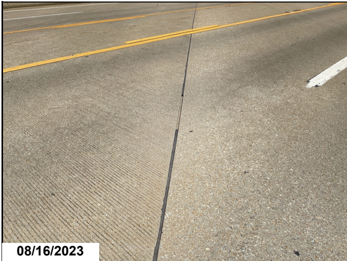
Saw cut joint
