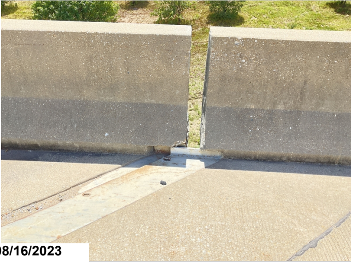
5" gap at Rt rail over bent 5
