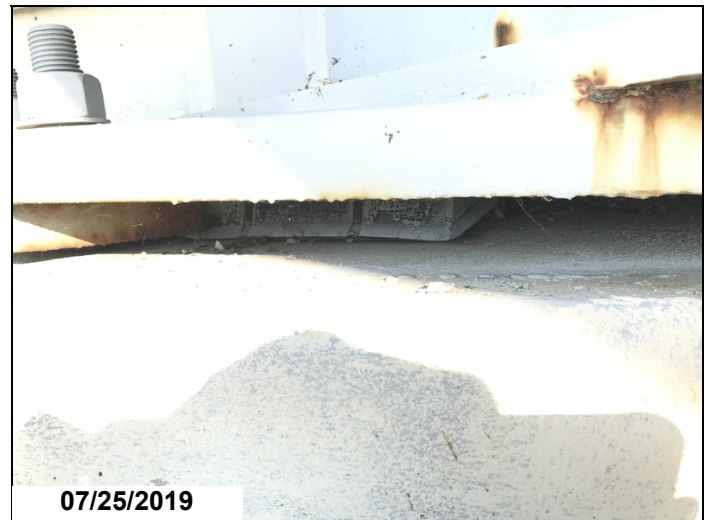
Span 1 Bent 1 bearing 8 twisted 2019
