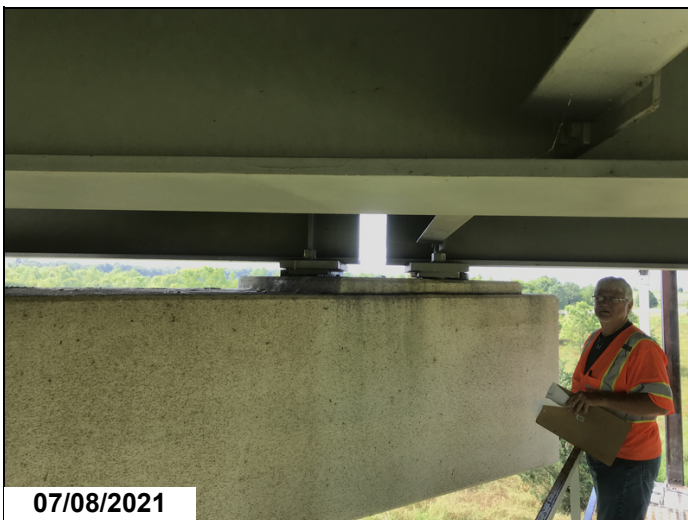
Span 4 bent 5 bearing 8 both moving 2021
