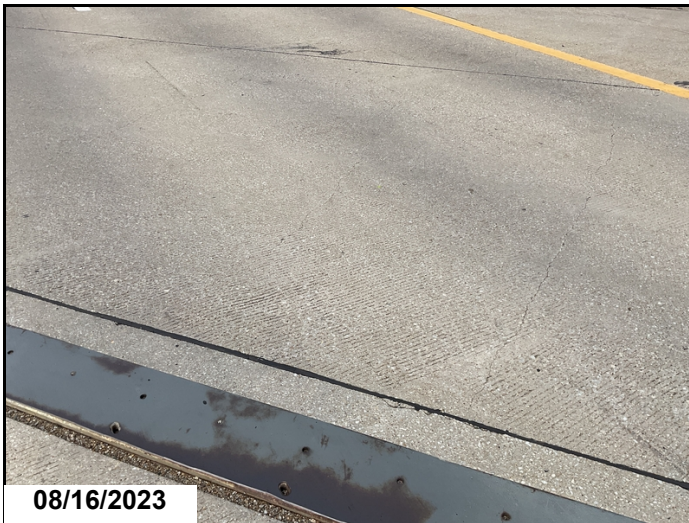
Approach slab cracks
