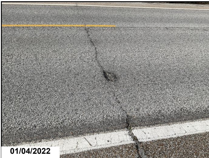
Span #3 right lane overlay at joint has a one foot long by five inch wide shallow spall
