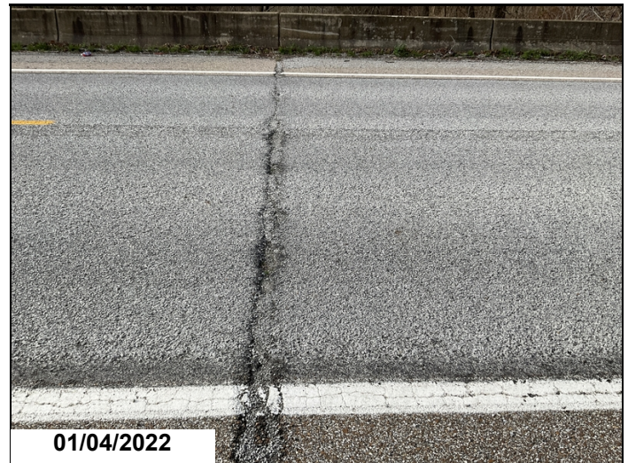
Bent #2 overlay at joint has several shallow spalls
