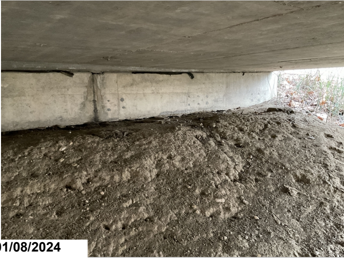
Abutment #1 cap undermining
