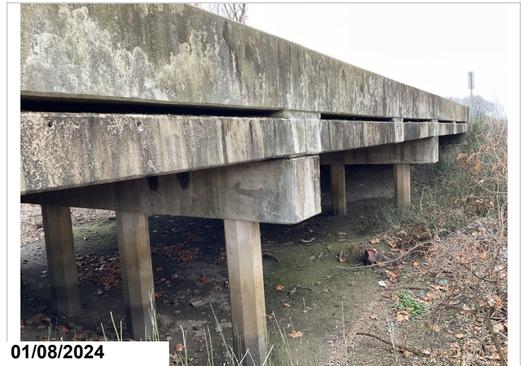
Typical side of slab crack at bents.
