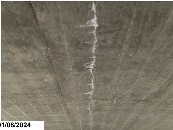
Typical soffit-under surface crack in center with efflorescence
