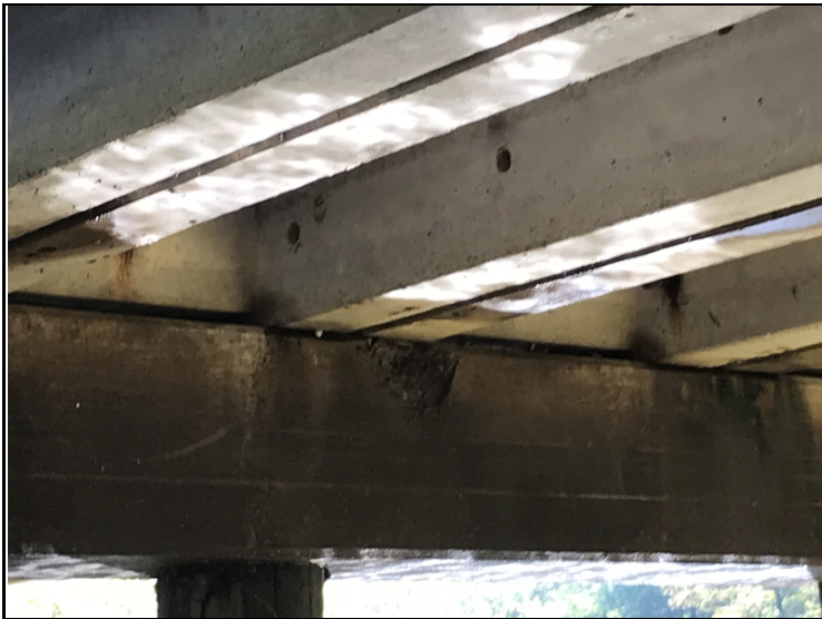
Typical bolt missing between units.
