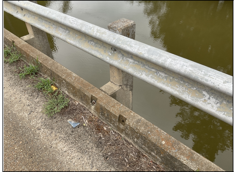
Span #2 second post right side is cracked.
