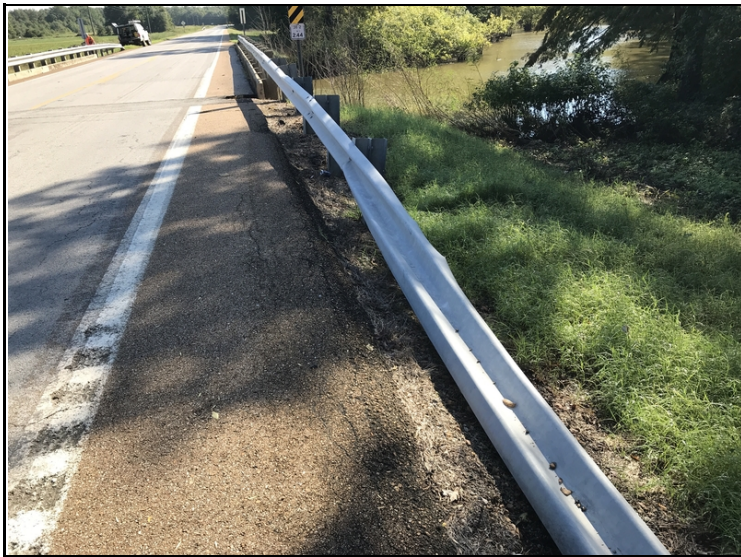
Abutment #1 right approach rail turn down has collision damage.
