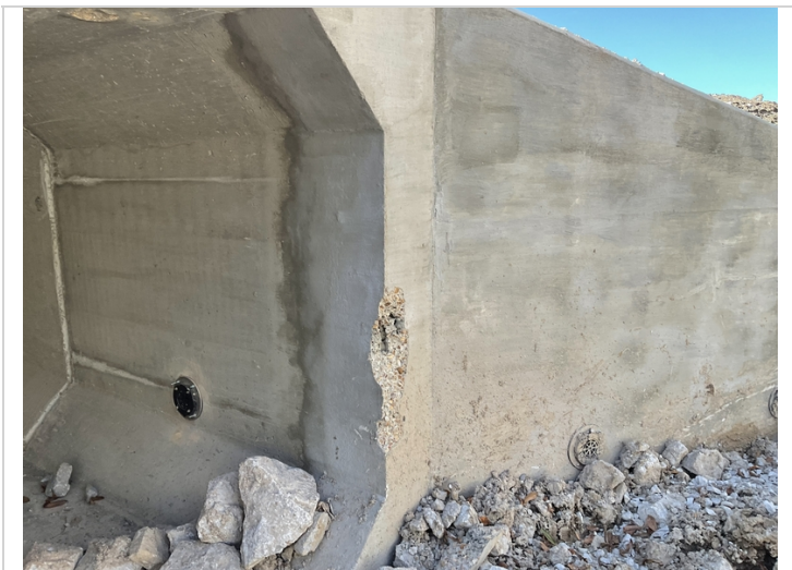
Barrel #1 left end back wall has a 1' spall no rebar exposed.
