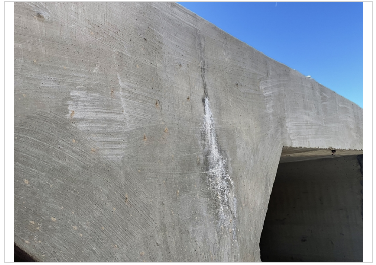
Ends of culvert between barrels have hairline cracks with light efflorescence.
