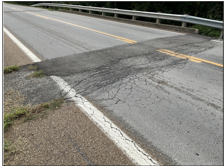
Abutment #1 approach roadway has been repaired
