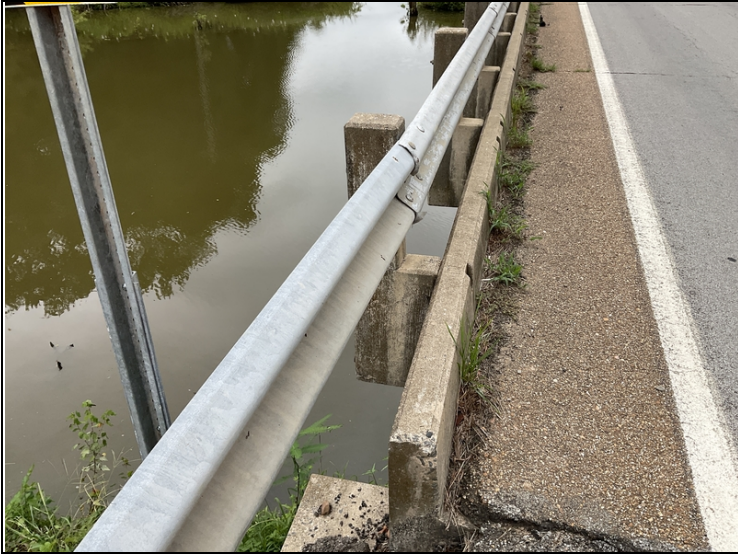
Span #1 first post left side is cracked.
