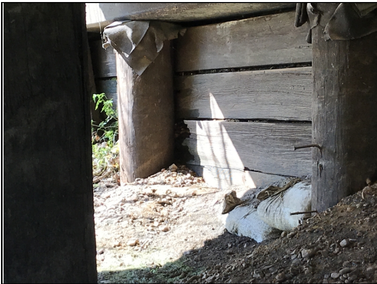
Abutment #1 back wall decay.
