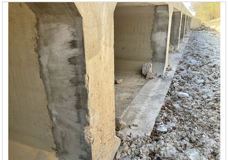
Barrel #6 left end back wall has two 6" spalls no rebar exposed. Barrel #8 left end back wall has a 6" spall no rebar exposed.
