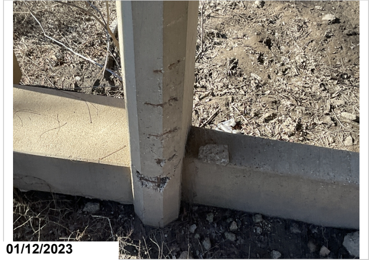
Bent #8 column #3 is spalled on ahead face four foot above ground with five feet of exposed rebar 5% section loss.
