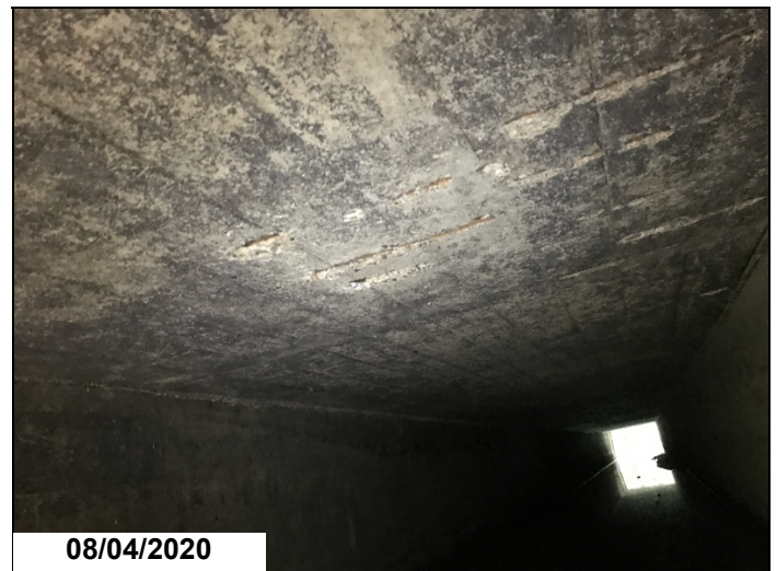
Span # 2 soffit has areas of delamination with small spalls on lt. end 15' - 20' inside and exposed rebar 8' total.
