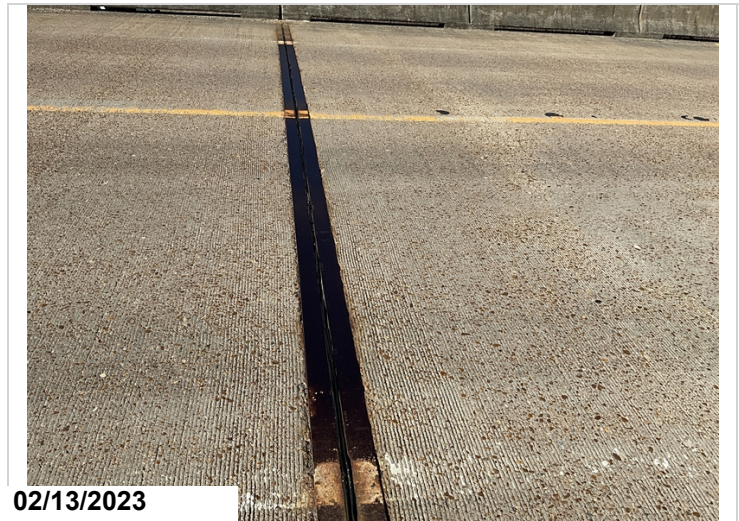
Bent 11, torn seal, cs 3.
