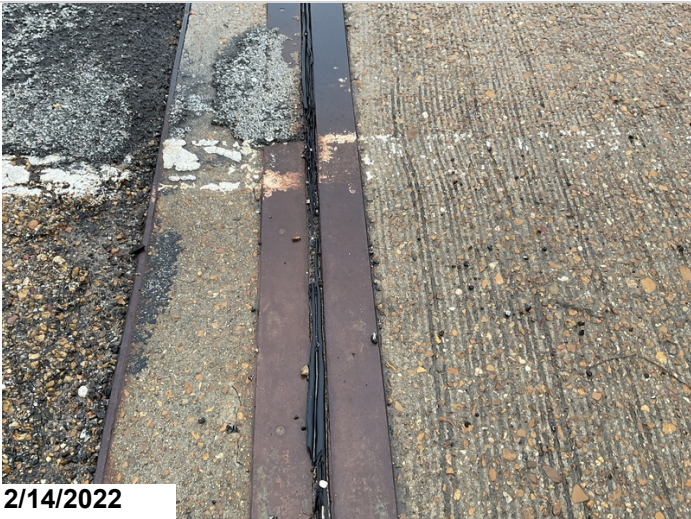
Abutment #1 joint seal weathered and torn
