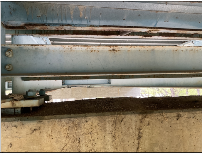
Typical debris on cap bent #5
