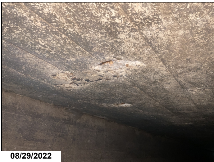
Exposed rebar barrel #1 soffit left side
