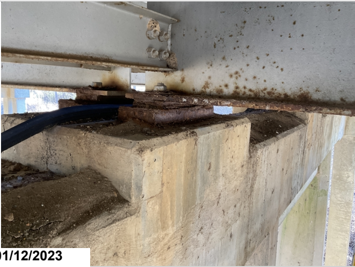
Bent #7 corrosion on girder ends and bearing.
