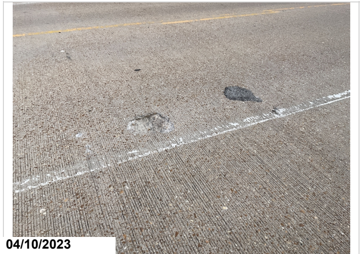
Span #13 right lane has a one foot achm patch. Span #13 right lane has a 1' spall with exposed rebar.
