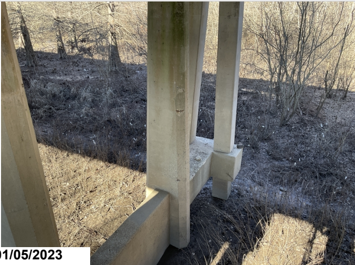
Bent #9 column #3 ahead face has one six inch spall, and one six inch delaminated area.
