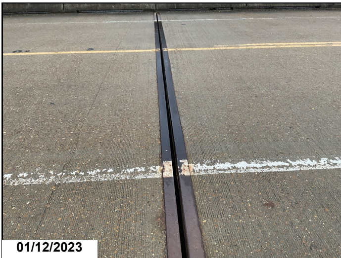
Bent #7 joint has fallen out
