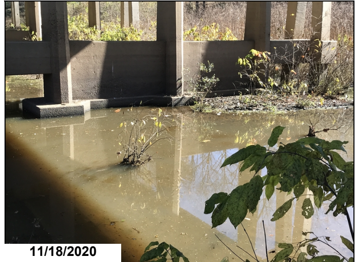
Bent #5 footing exposed left end 3' and 1' at the right end.
