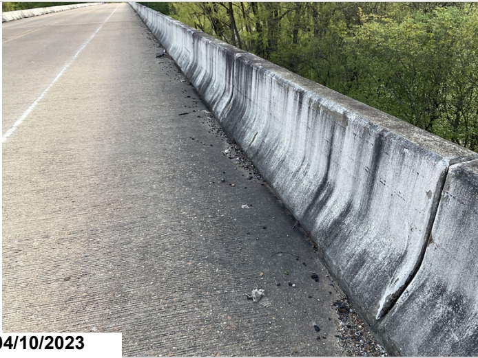
Typical debris in gutters
