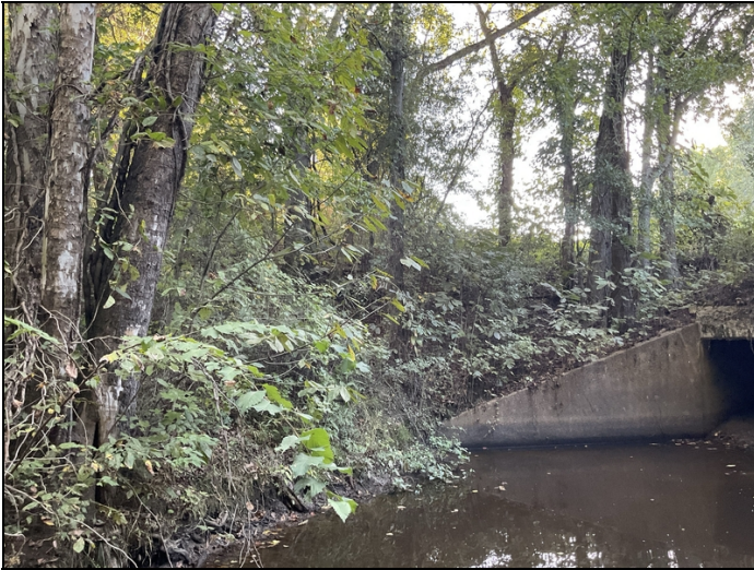
Culvert: heavy vegetation growth on both sides.
