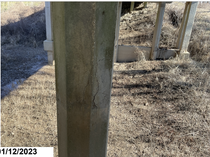
Bent #9 column #2 back face has two foot delaminated area.
