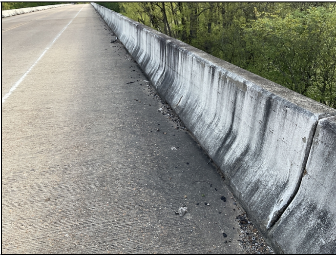
Typical debris in gutters
