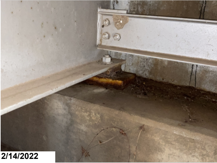
Typical abutment bearing
