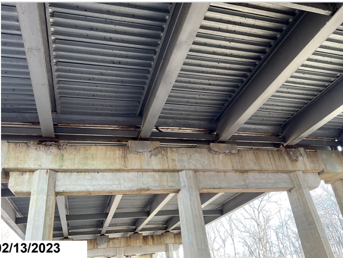
Bent 10 ahead, bearings 2 and 5, loss of bearing area.
