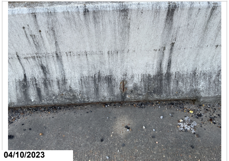
Typical exposed rebar on bridge rail
