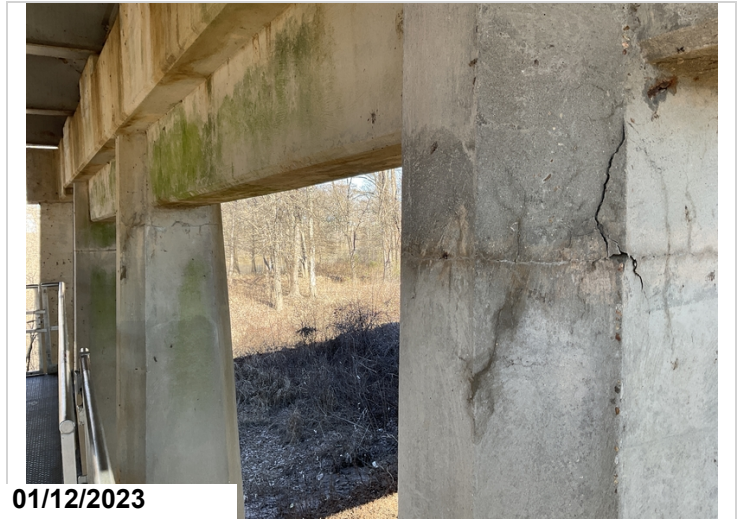
Bent #10 columns #1, 2, 3 have horizontal cracking with light efflorescence six inches to one foot below cap.
