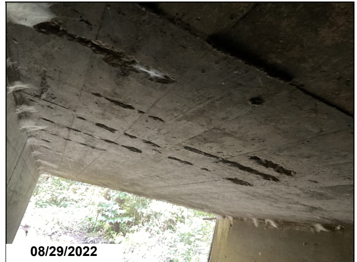
Exposed rebar barrel #2 left end.
