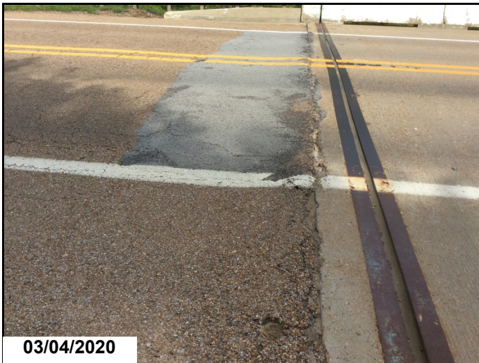
Abutment #1 approach roadway has settled 1"-2" increasing impact loading on bridge.
