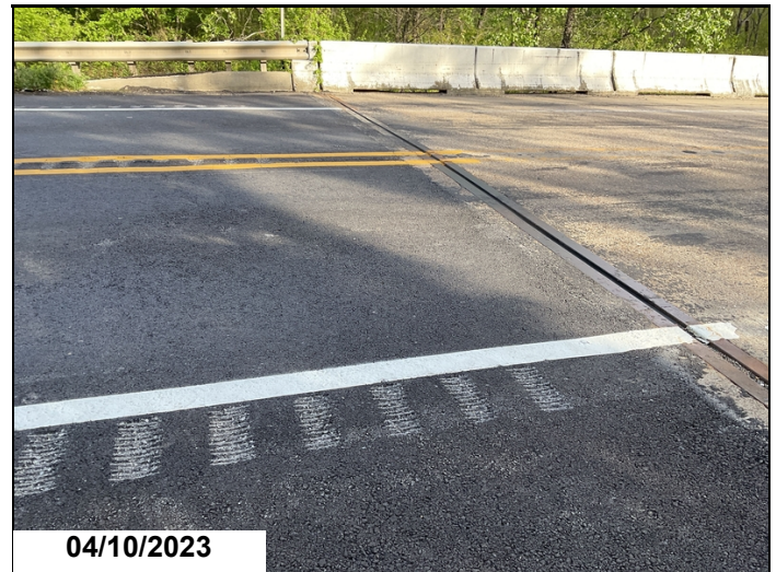
Abutment #1 approach roadway has been leveled since last inspection
