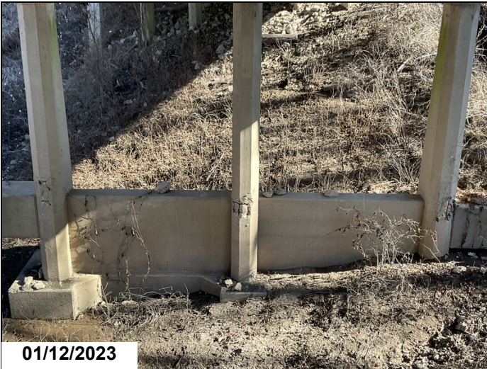
Bent #10 column #1, 2, 3 each have one foot spalls four foot above ground on the back face with rebar exposed 10% section loss.
