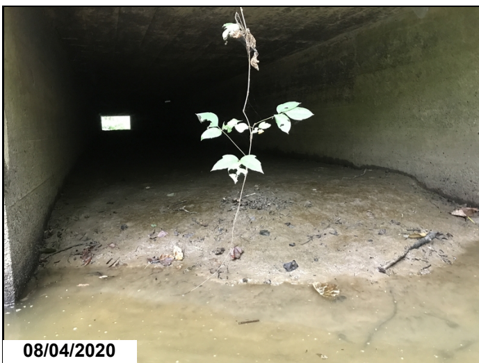
Barrel #1 has 4' of silt full length
