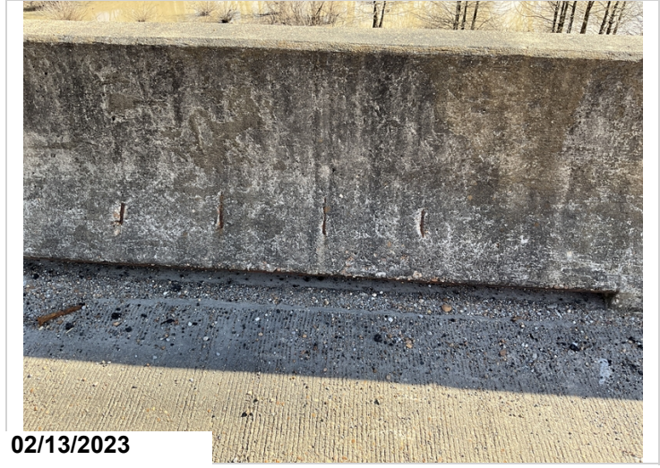
Span 8, left, exposed reinforcing steel, cs 2. Typical 7 , 6 , 4 , 3 , 2, 1.
