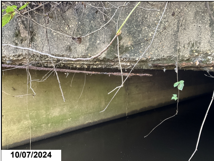
Barrel 1, Left Headwall: Spalling with exposed reinforcing steel with 100% section loss and loss of bond. CS4. 1'.
