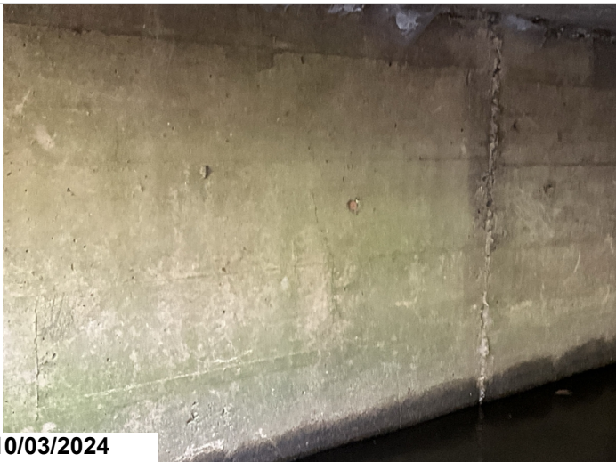
Intermediate Wall: Minor vertical cracking. CS2.
