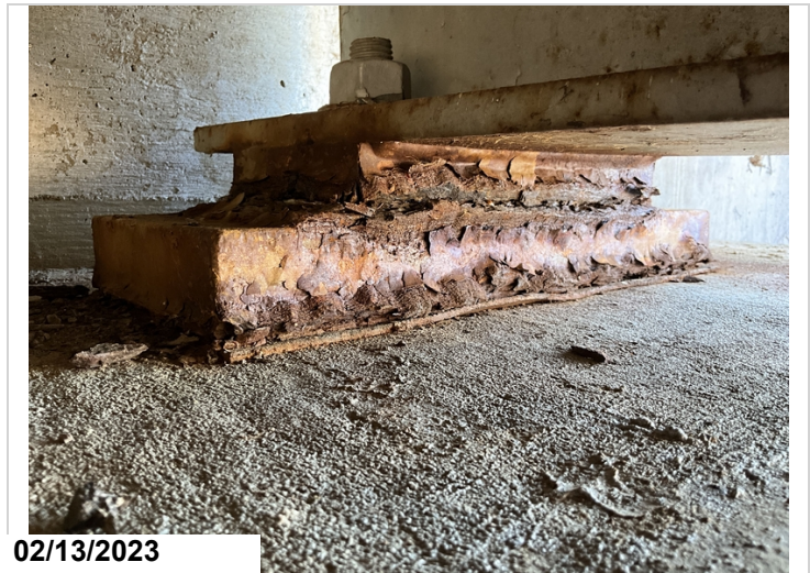
Bent 12, bearing 6, corrosion cs 3.
