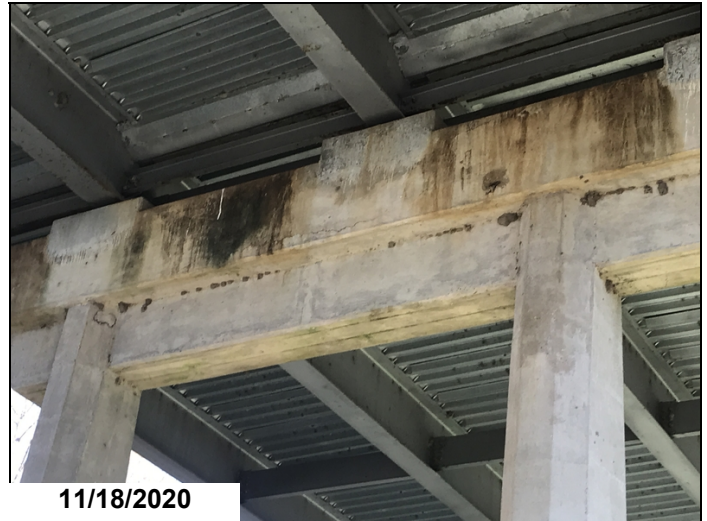
Bent #6 cap back face has 4' long crack under girder #3.
