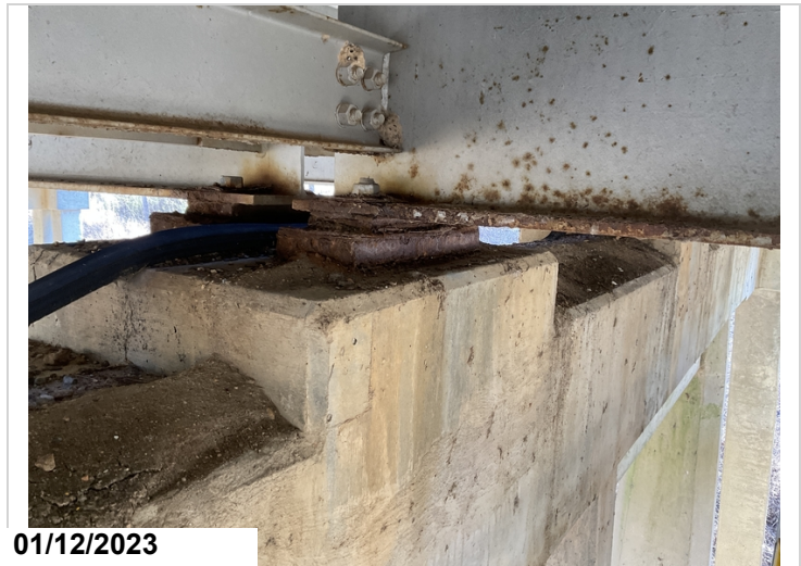
Bent #7 corrosion on girder ends and bearing.
