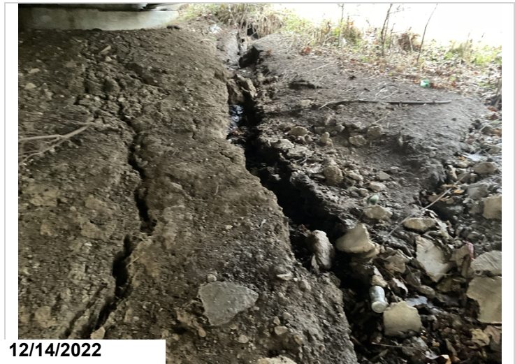
Abutment #2 slope right side has erosion vein up to 2' deep due to roadway runoff
