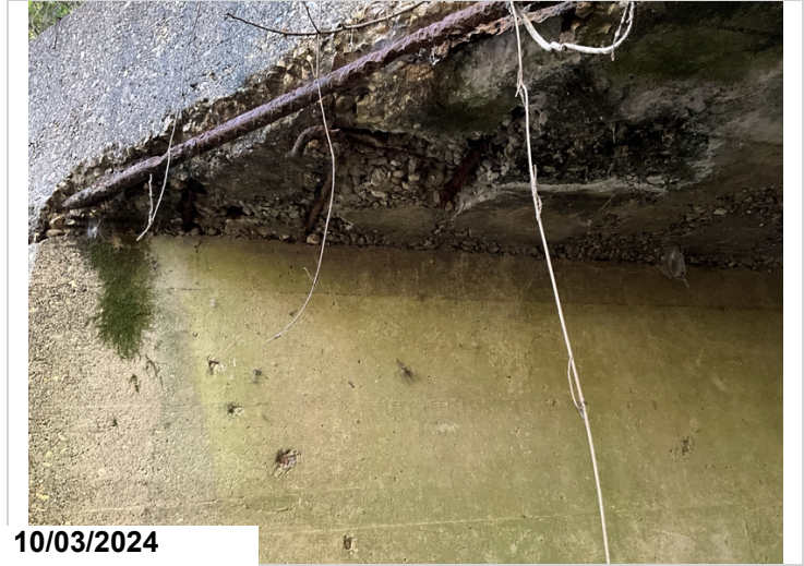
Barrels 1 & 2, Left, Undersurface: Spalling with exposed reinforcing steel. CS3.
