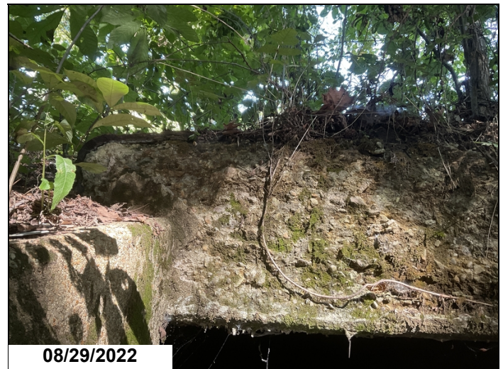
Exposed rebar right side head wall
