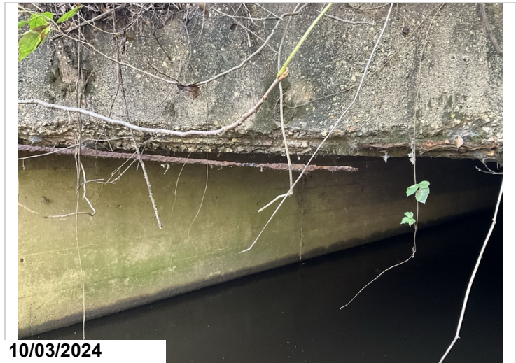
Barrel 1, Left Headwall: Spalling with exposed reinforcing steel with 100% section loss and loss of bond. CS4. 1'.
