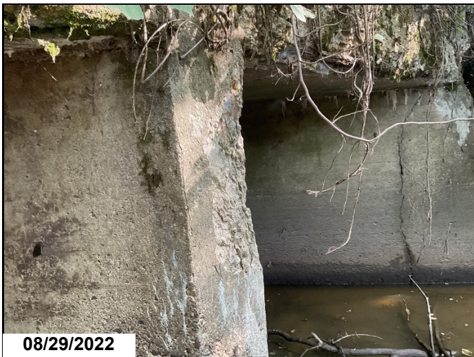
Interior wall right side spalled with no exposed rebar.
