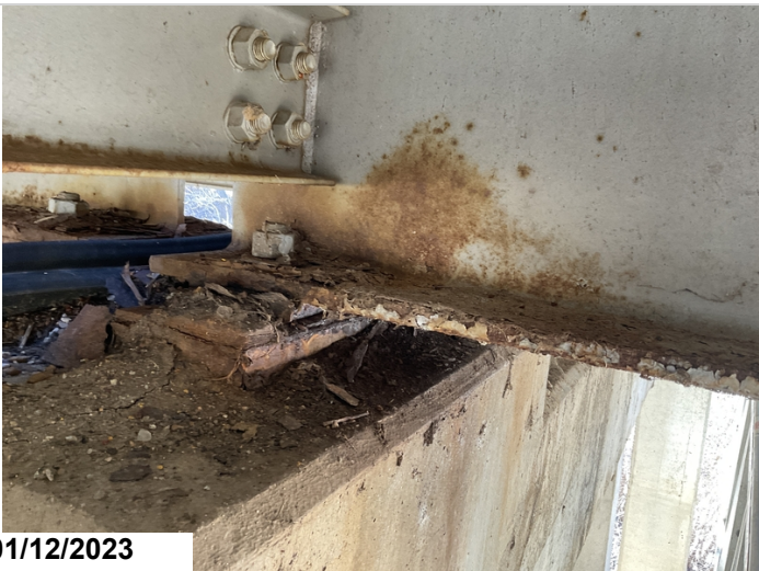
Corrosion on bearings and girder ends
