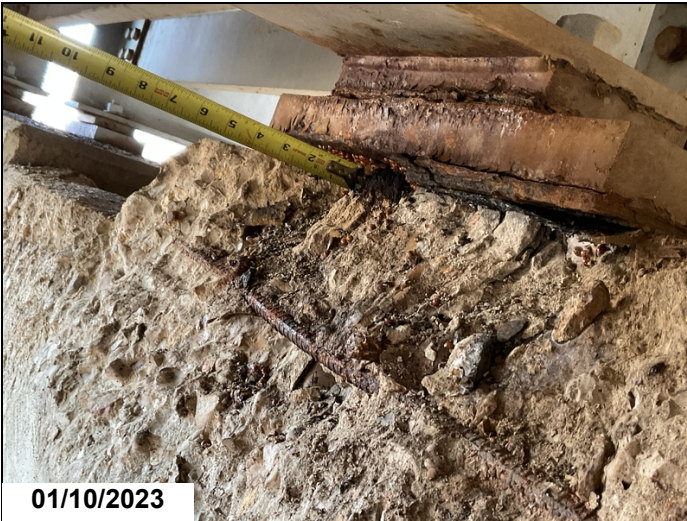
Bent #3 cap back face bearing riser spalled for approximately 3.5 feet under span #2 girder #2 extending up to three inches underneath bearing masonry plate with exposed rebar
