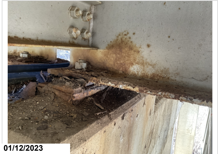
Corrosion on bearings and girder ends
