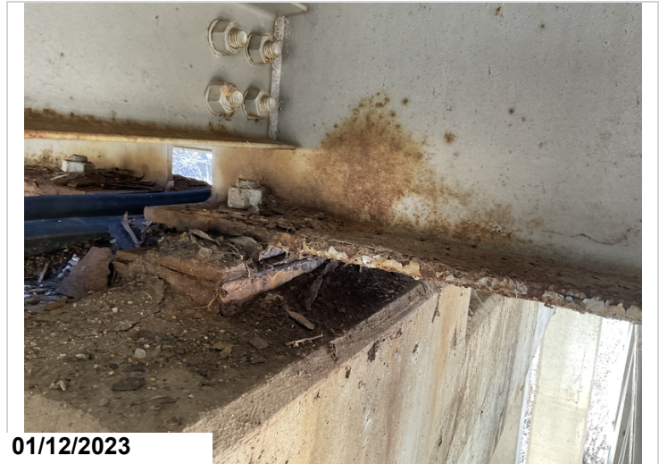
Corrosion on bearings and girder ends
