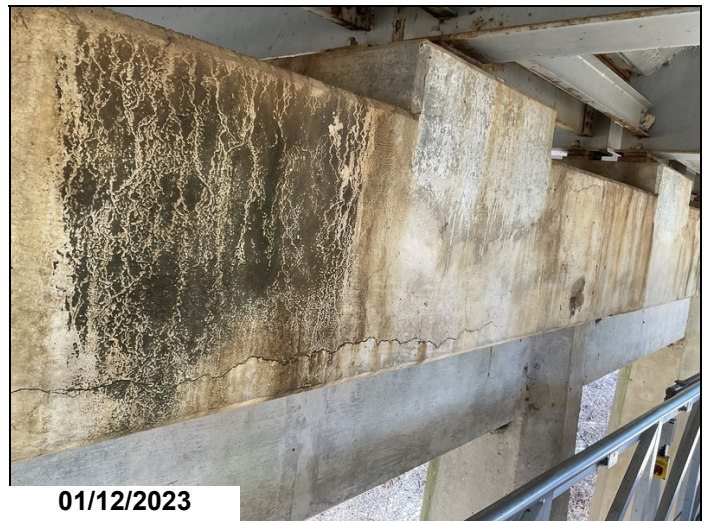
Bent #6 cap back face has ten feet of cracking between girders #2 and 5.
