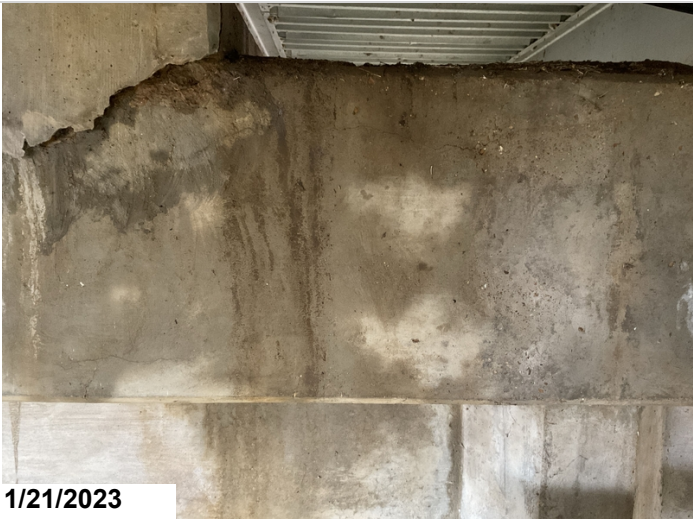
Bent #3 cap back face has cs2 cracks for 6' between girders #2, 5.
