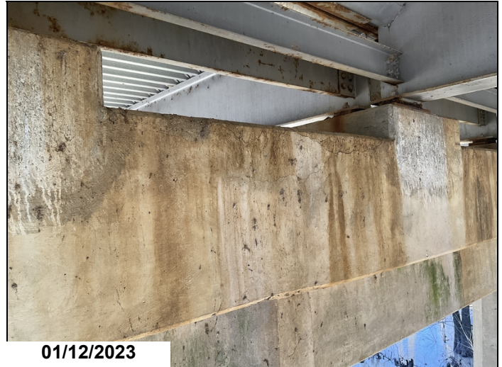
Bent #6 cap ahead face between girders #3 and 4 cracked horizontally for four feet
