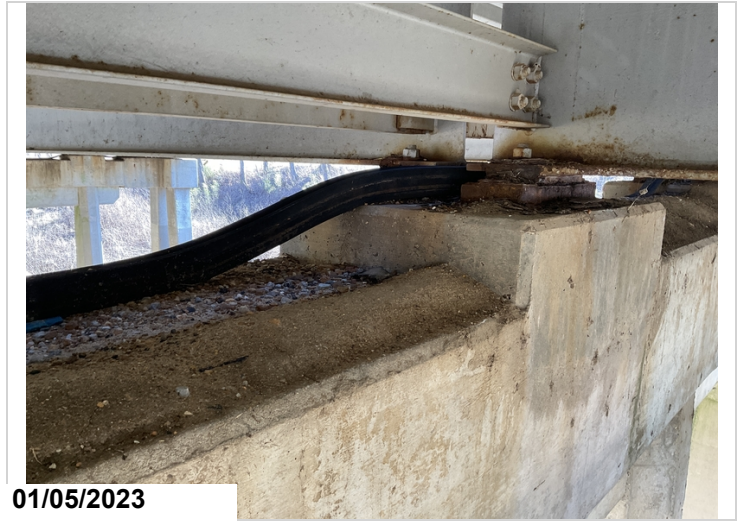
Bent #7 dirt and debris on caps
