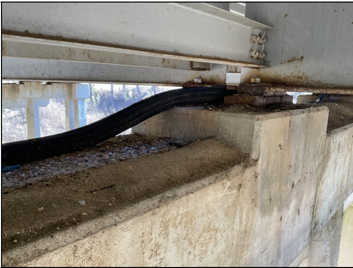
Bent #7 dirt and debris on caps
