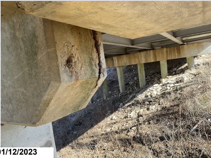
Bent #10 cap ahead face right side has a six inch delamination and a four inch spall with exposed rebar with 10% section loss.
