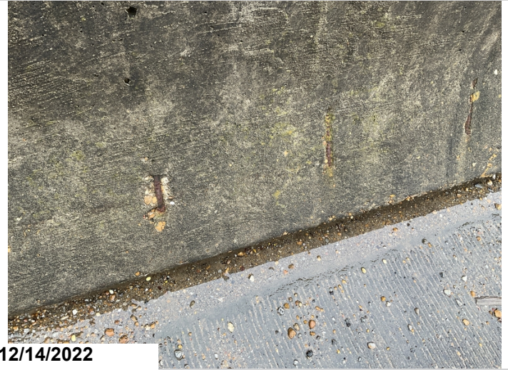
Typical exposed rebar in concrete bridge rail
