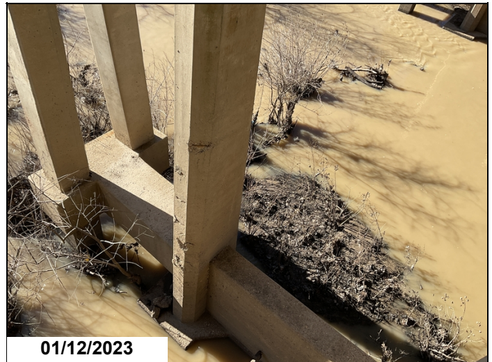
Bent #5 column #3 ahead face has several exposed rebar areas due to poor concrete coverage 5% section loss.
