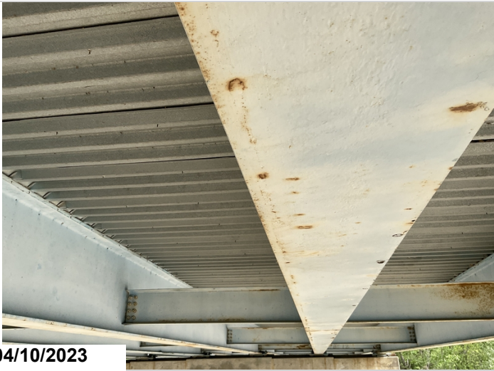
Span #11 girder #5 bottom flange has narrow ribbon of delamination full length.
