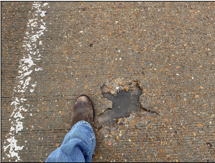
Span #5 deck left lane has one foot spall near mid span
