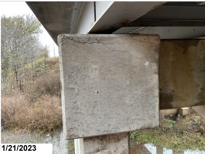
Bent #5 cap ahead face right side extension is cracked and delaminated for 2' at top.
