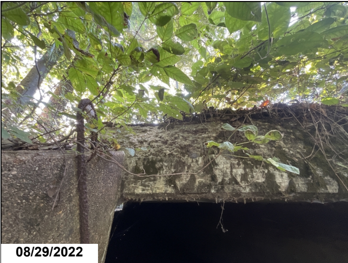
Left side head wall heavily scaled with exposed rebar with up to 100% section loss
