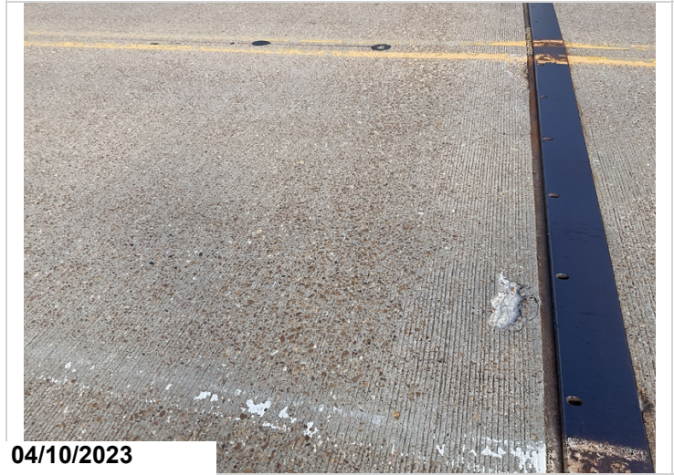
Span #8 at bent #9 center and right lane has 2 one foot shallow spalls each with no exposed rebar.
