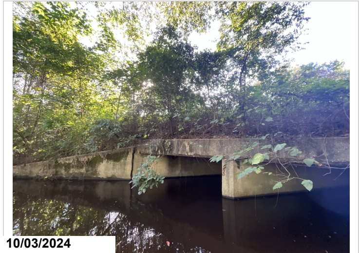
Left side of Culvert: Vegetation growth.
