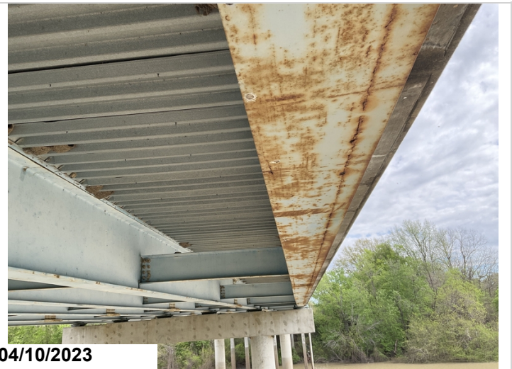
Span #10 girder #6 bottom flange has small ribbon of delamination in center section between field splices.
