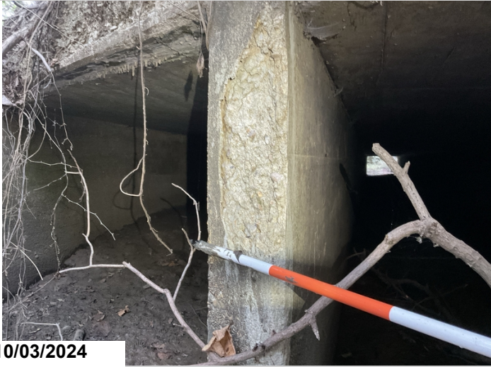
Intermediate wall, right side: spall. 1LF CS3.
