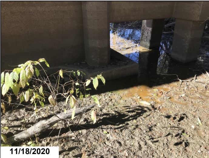
Bent #6 footing exposed full length left side and 1 1/2' to ground level on right.
