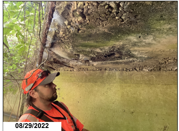
Exposed rebar in barrel #1 soffit, left side
