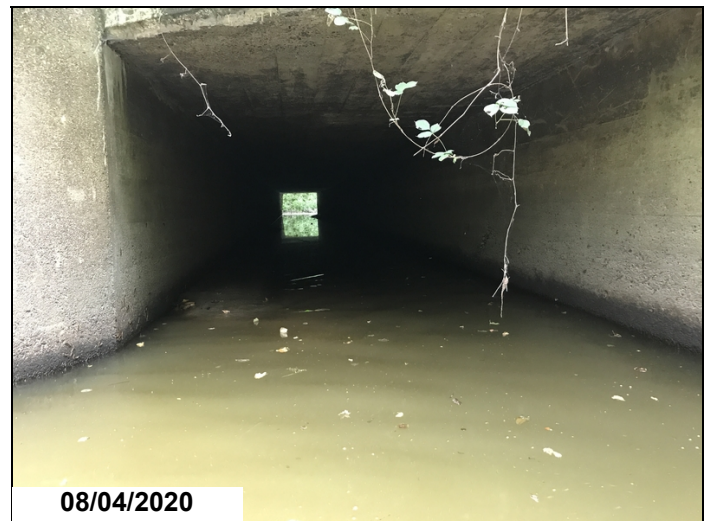
Barrel #2 has 3' of silt full length
