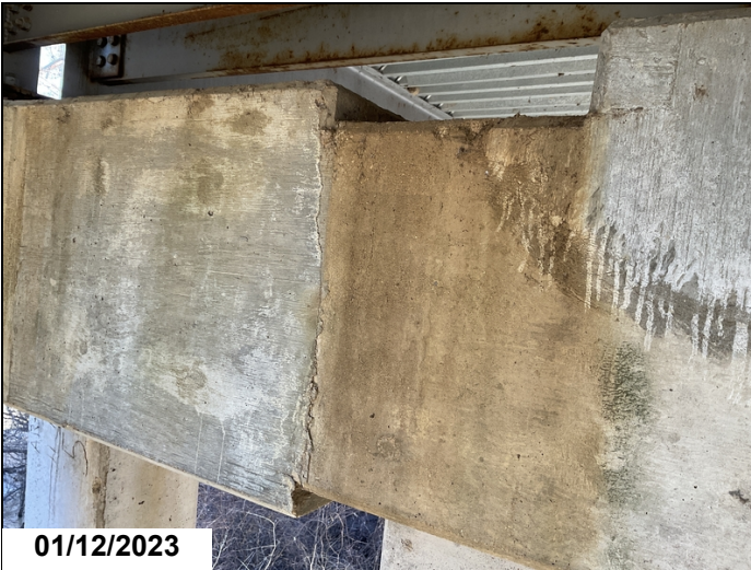
Bent #6 cap has vertical crack at cold joint between girders #1 and 2.
