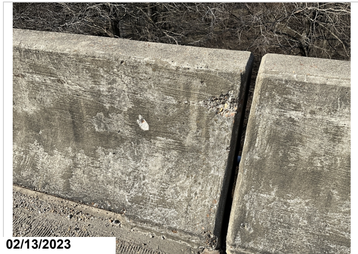
Span 5, right , spall cs 2. Typical 6, 7
