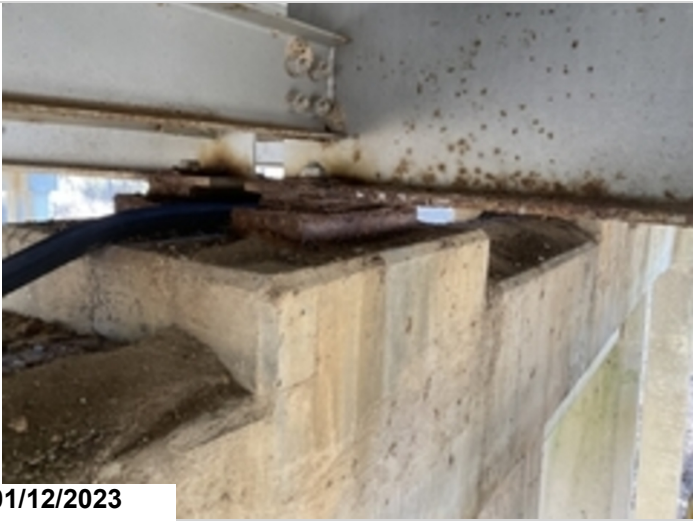
Corrosion on girder ends and bearings at bent #7
