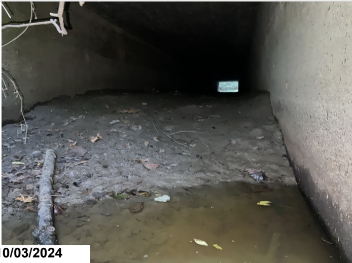
Barrel 1: sediment build up up to 4.5 feet.
