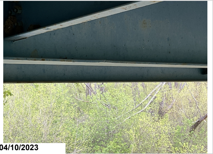
Span #2 girder #2 4' ahead of field splice has a small area bottom flange is bent upward slightly.
