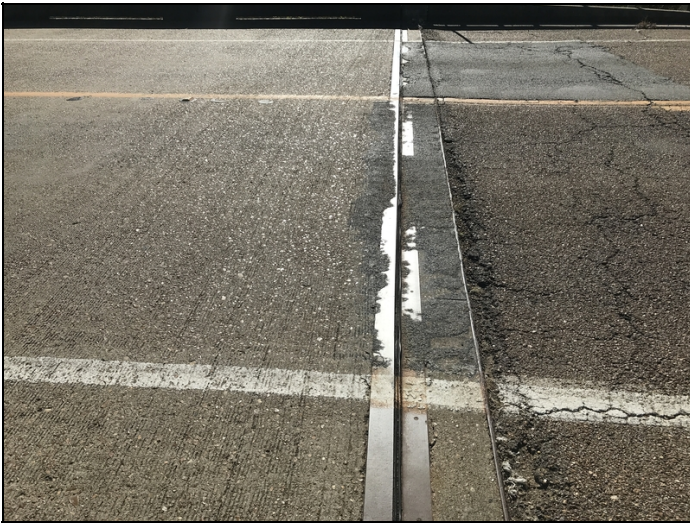
Abutment #1 joint.
