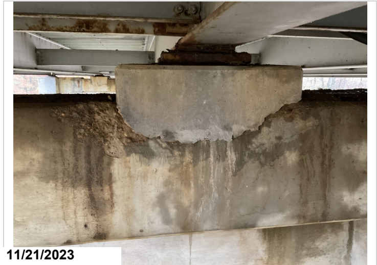
Bent #3 cap back face under girder #3 bearing riser is cracked and spalled for 3' extending under bearing masonry plate.
