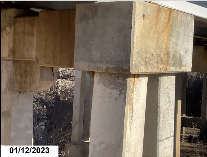
Bent #5 cap right side of original cap delaminated on end. Bent #5 cap right end has one foot of cracking and delaminated area.
