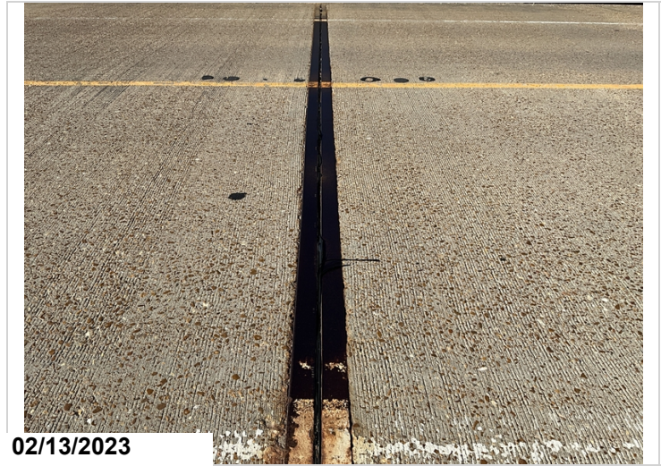
Bent 9, torn seal, cs 3.
