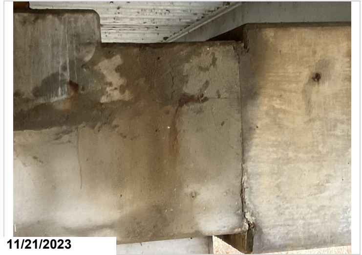
Bent #9 back face right side has a 1' crack/delaminated area with rust staining between girders #5, 6.
