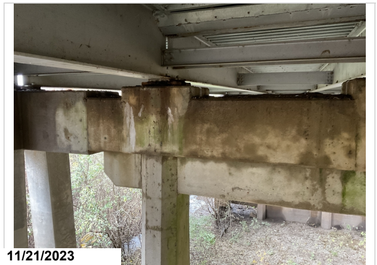
Bent #8 cap ahead face under girder #5 has several hairline cracks with light efflorescence.
