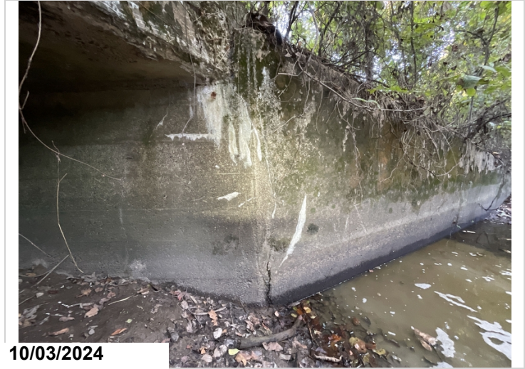
Beginning of structure, left side, wing wall: cracking and efflorescence.
