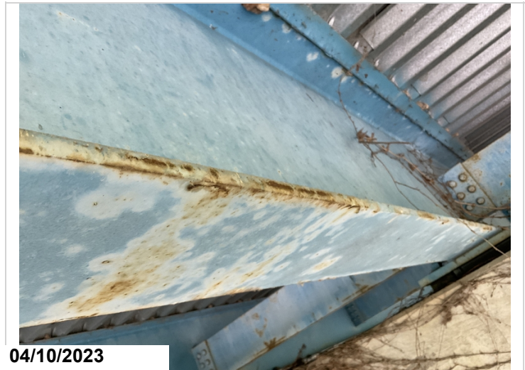
Typical area of delaminated on bottom flange of girder.
