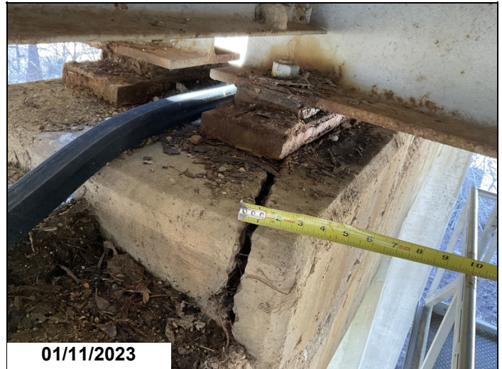
Bent #8 cap ahead face bearing riser cracked and delaminated and spalled under girder #3.
