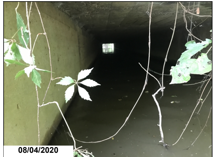
Barrel #1 two feet of silt in barrel full length.
