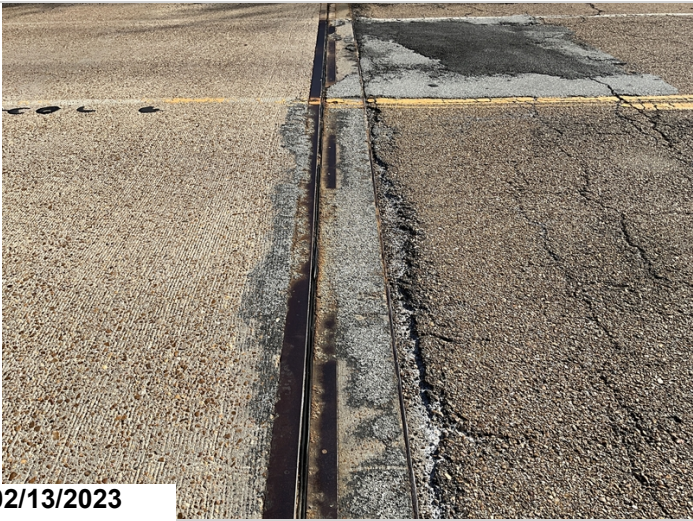
Bent 12, damage to joint seal, cs 2.
