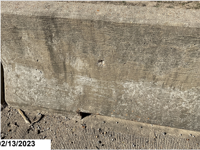
Span 11, right, spall cs 2.
