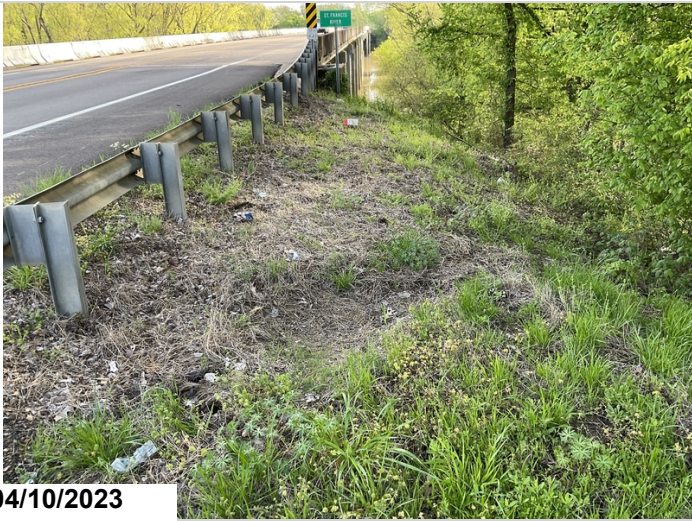
Two foot sink hole abutment #1 right side fifty feet from bridge end.
