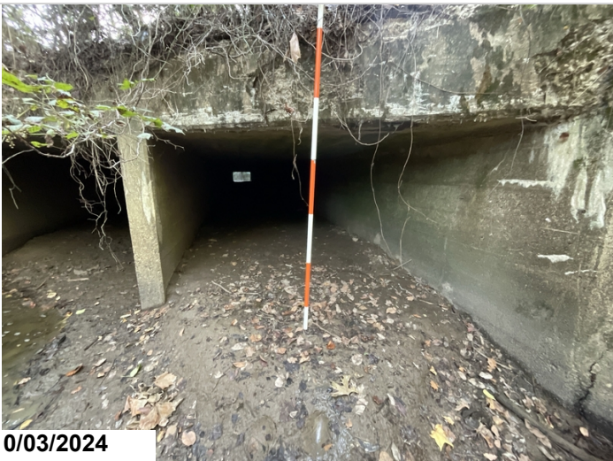
Barrel 2, left side: sediment build up.
