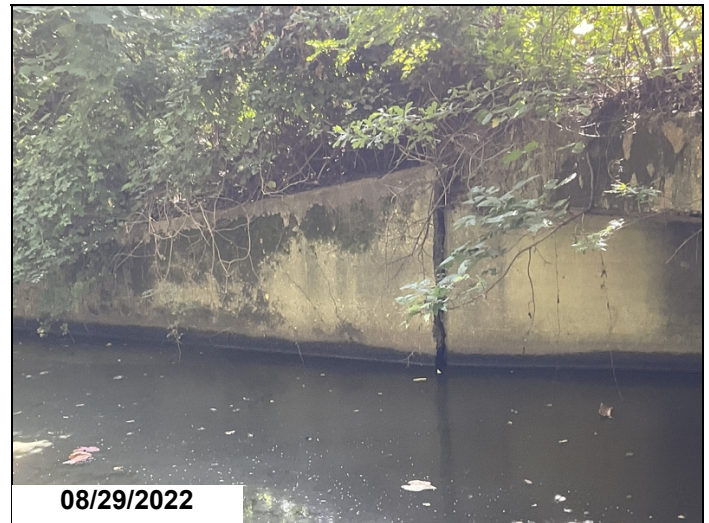
Barrel #2 left wing separated and leaning in
