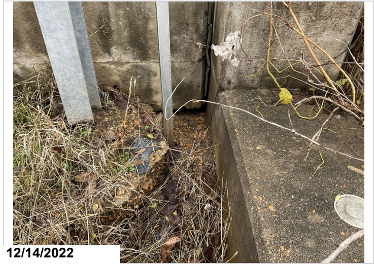
Abutment #1 right approach gutter has small void underneath at bridge end
