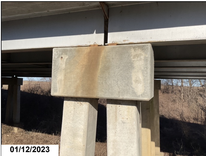
Bent #4 cap right end has vertical hairline crack
