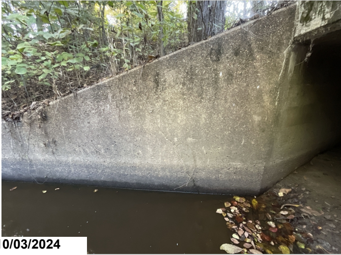
End of structure, left side, wing wall: diagonal crack.
