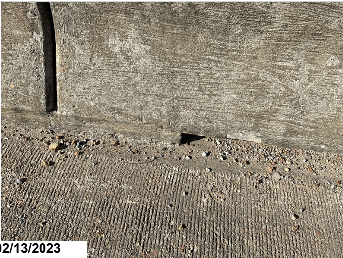
Span 8, right side, crack cs 2.
