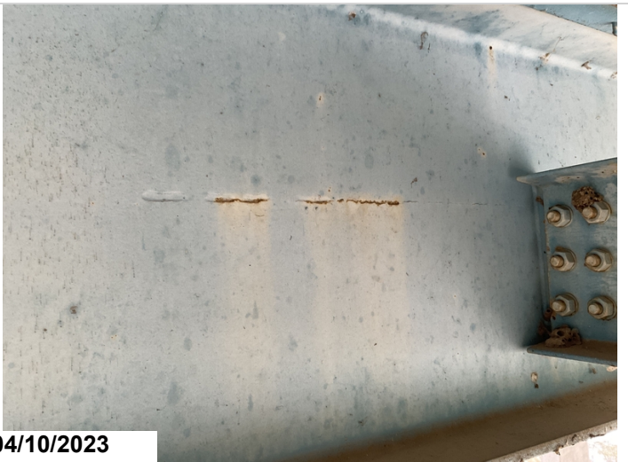
Span #7 girder #4 right side center span center of web has area of gouges where welds have been removed.
