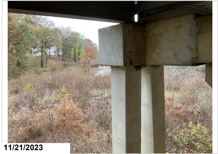
Bent #6 cap ahead face right side under girder #6 has cracks and delaminated for 1' with exposed rebar minor section loss.
