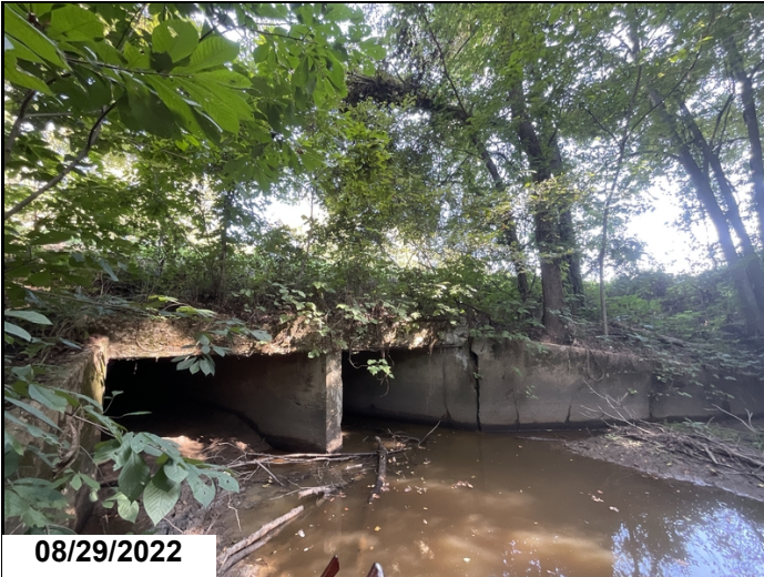
Trees and vegetation growing behind wing walls and on top of culvert ends
