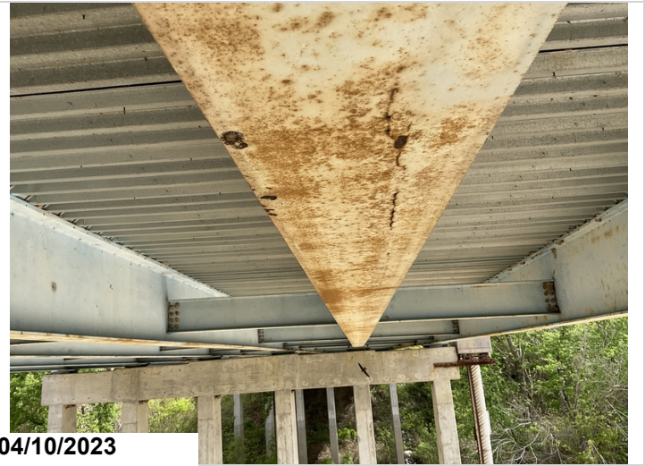
Span #12 girder #5 has an area a quarter span on bottom of bottom flange for two feet that a thin layer of metal is delaminated.
