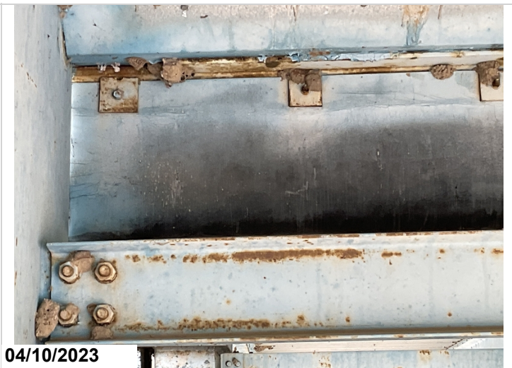
Bent #9 seal cracks and weathered
