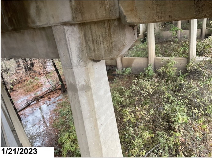
Bent #5 cap right end has 1' of cracking and delaminated area at end of old cap and new cap.
