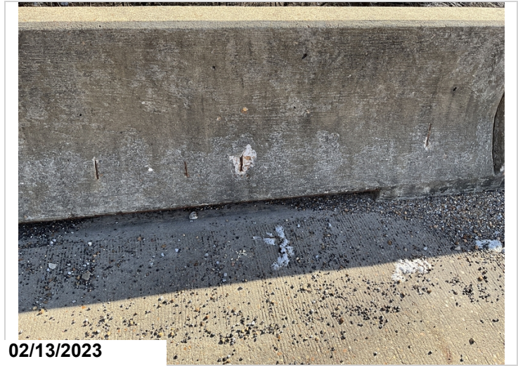
Span 11, left, exposed reinforcing steel, cs 2.
