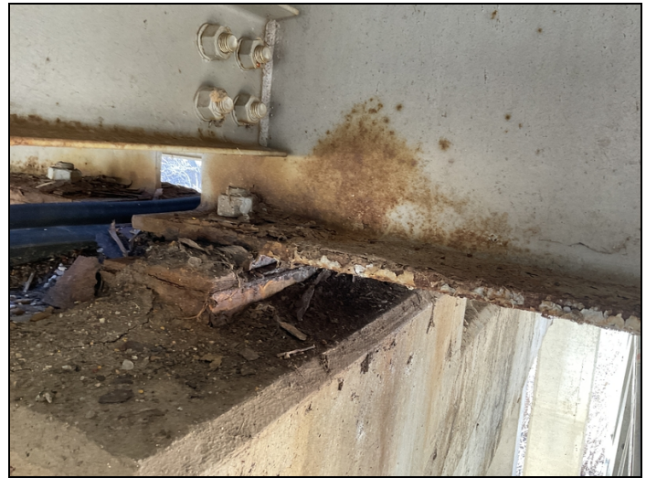
Corrosion on bearings and girder ends
