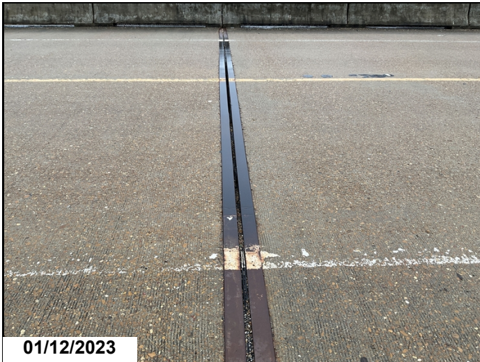
Bent #3 joint seal has 10' that has fallen out and 8' with lost adhesion and sagging
