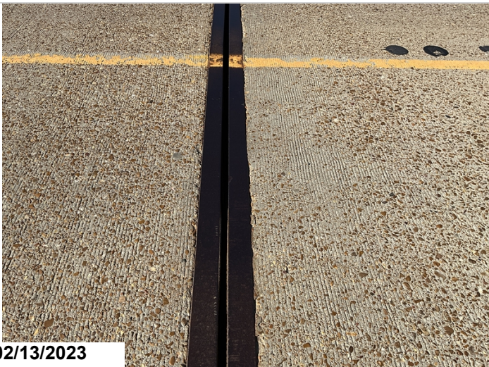
Bent 10, joint fallen out, leakage, cs 4.
