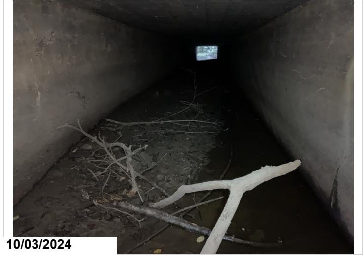
Barrel 2: sediment build up, up to 4 feet.
