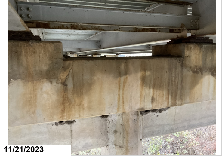
Bent #5 cap back face at top has cs3 cracks horizontally for 12' starting at girder #3.
