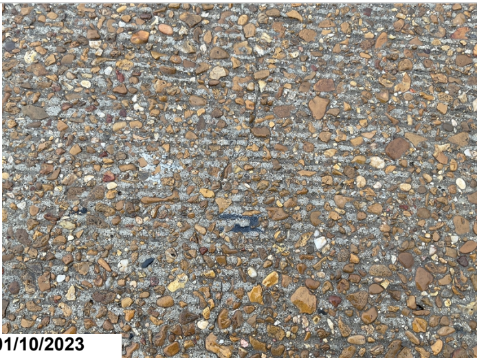
Typical longitudinal deck crack
