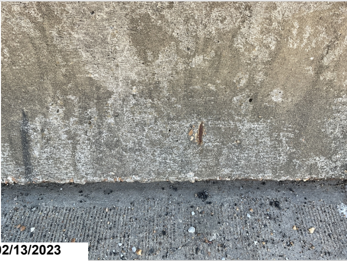
Span 9, left , exposed rebar, cs 2.
