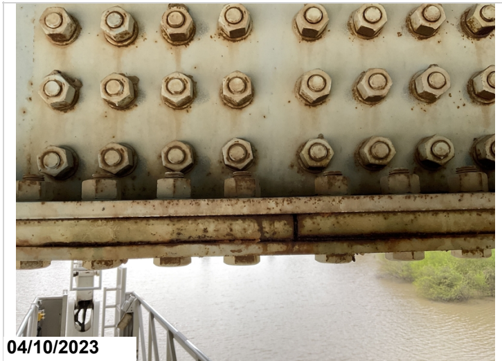
Field splices on bottom of bottom flange are beginning to form pact rust little to no section loss.
