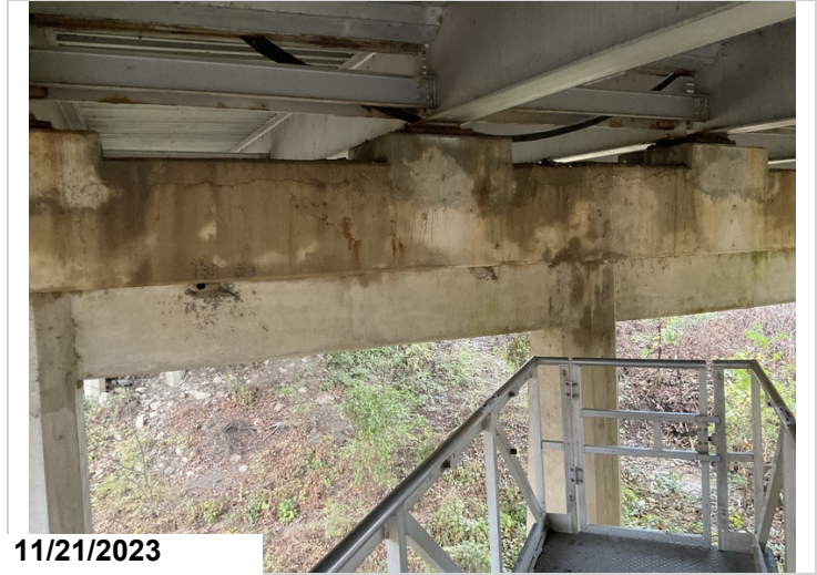
Bent #3 cap ahead face has horizontal cs3 cracks for 15' with a 2' delaminated area between girders #4, 5 between girders #3 and 5.
