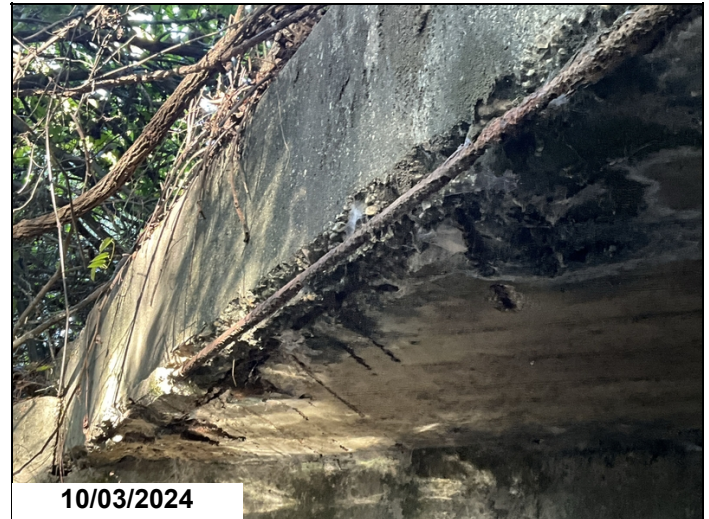
Barrel 1, Right, Undersurface: Spalling with exposed reinforcing steel. CS3.
