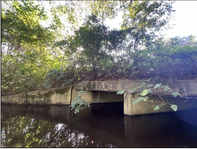
Left side of Culvert: Vegetation growth.
