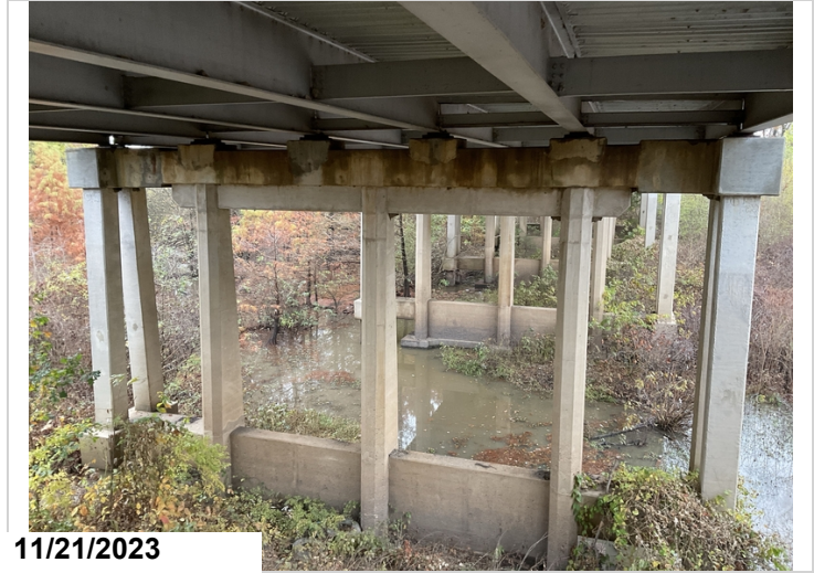
Typical interior bent
