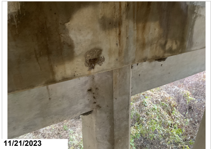
Back #6 cap back face has 6" spall with exposed rebar minor section loss above column #2.
