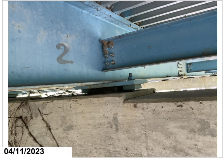
Typical interior paint condition
