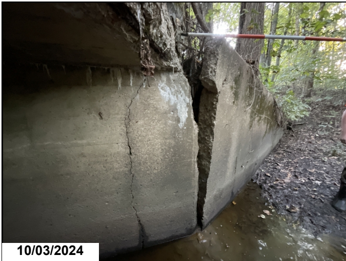
End of structure, right side wing wall: cracked and separated 1ft. at the top. due to large vegetation growing behind wing wall.
