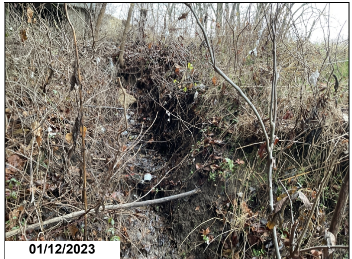
Span #10 slope right side eroded up to three feet deep under deck drains
