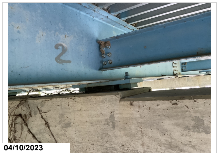
Typical interior paint condition
