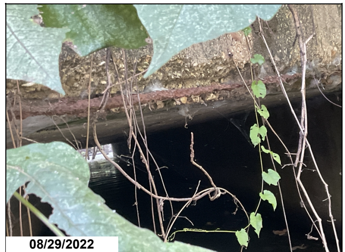
Exposed rebar left side of culvert head wall
