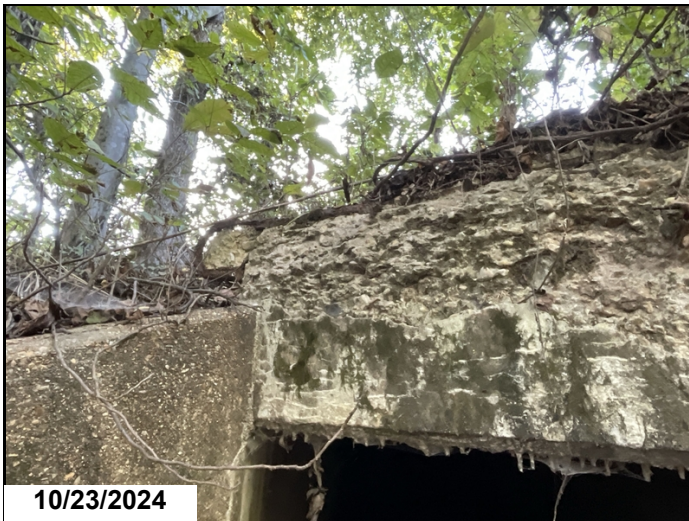
Barrel 2, end of structure, left side, head wall: spall with exposed reinforcing steel with 100% section loss. 1' CS4.
