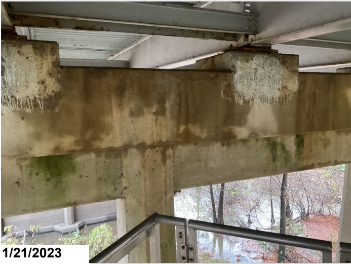
Bent #6 cap ahead face has cs3 cracks horizontally for 4' between girders #3, 4.
