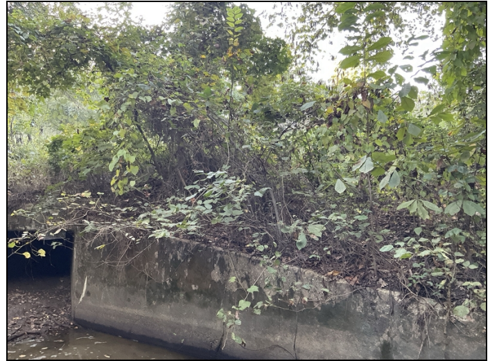
Culvert: heavy vegetation growth on both sides.
