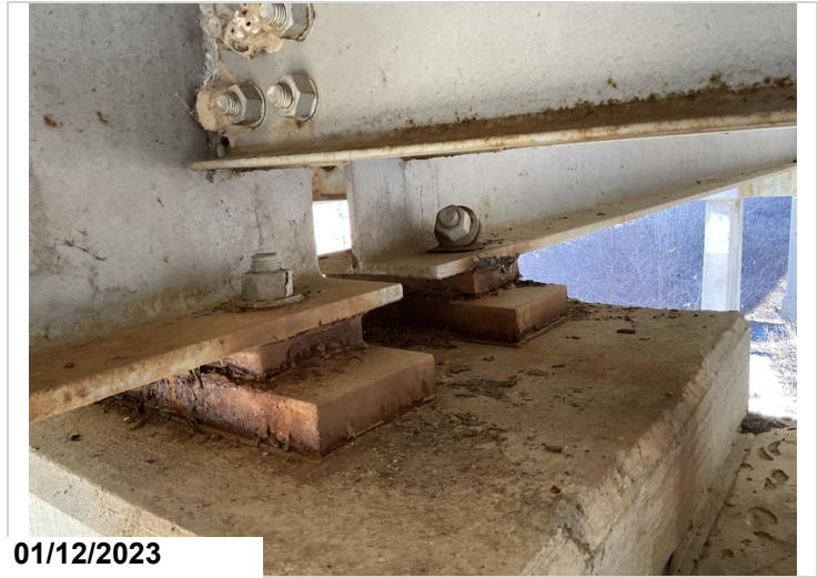
Span #6 bent #6 girder #2 right anchor bolt broken.
