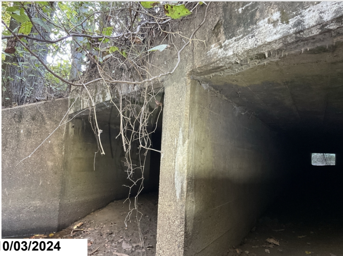
Left side: head wall is disintegrating with efflorescence and spalling. 1LF CS3. Left side, intermediate wall efflorescence with build up. 1LF CS3.
