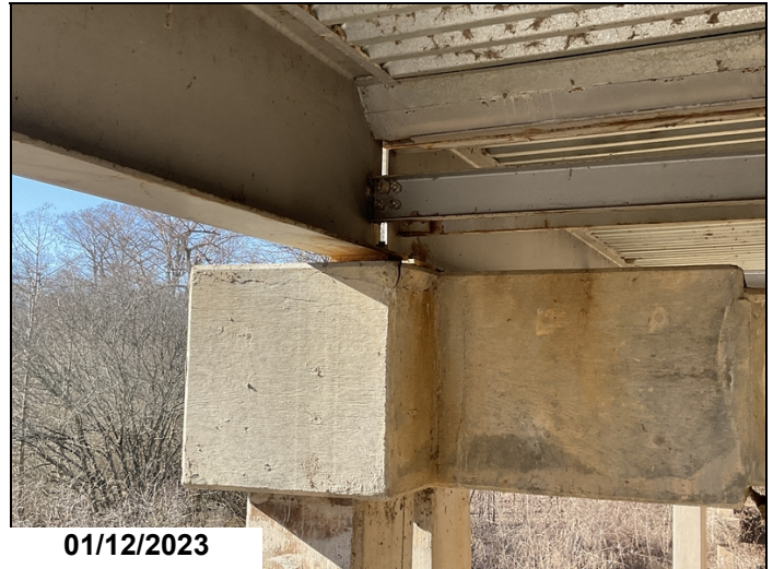
Bent #5 cap ahead face right side extension cracked and delaminated for two feet at top.
