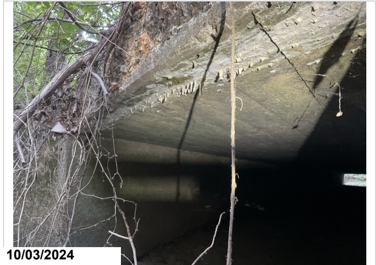
Barrel 1, right end: efflorescence with build up along top box edge. 1LF CS3.
