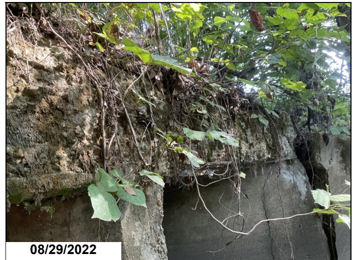
Right side head wall heavily scaled with exposed rebar with 100% section loss.
