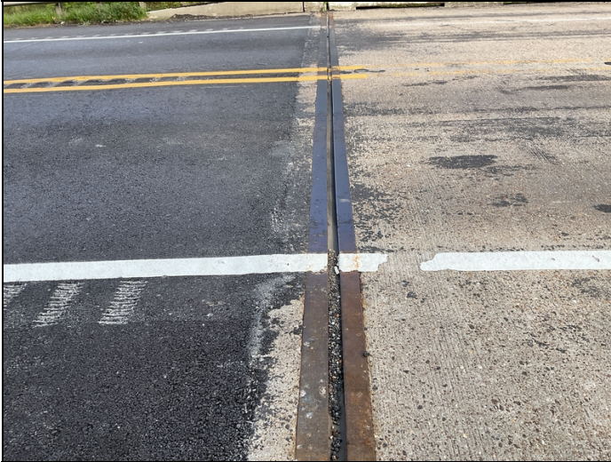
Abutment #1 joint
