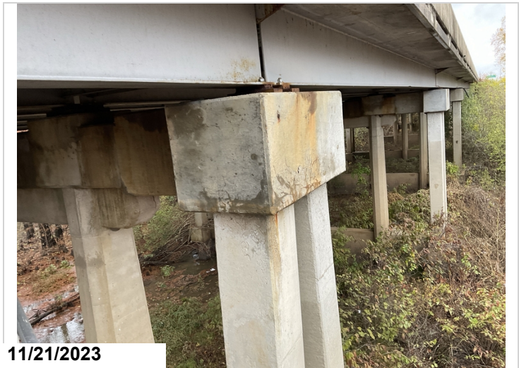
Bent #5 cap right end has 1' of cracking and delaminated area at end of old cap and new cap.
