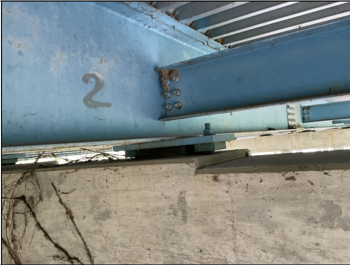
Typical interior paint condition
