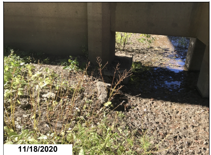
Bent #7 footing on left end is exposed 1 1/2'.
