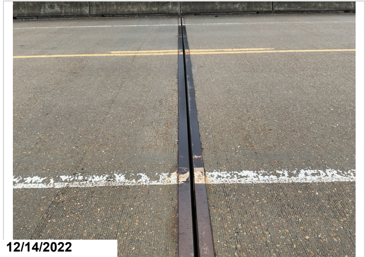
Bent #8 joint has fallen out
