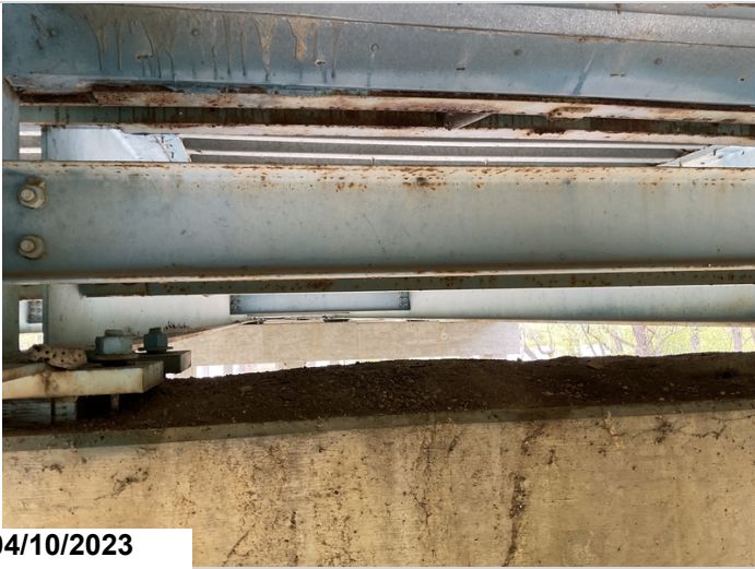
Typical debris on cap bent #5
