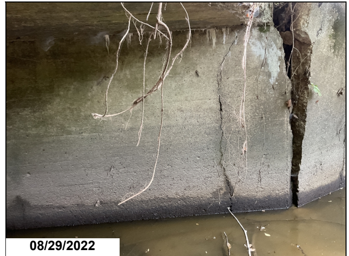
Cracking in barrel #2 outer wall right side
