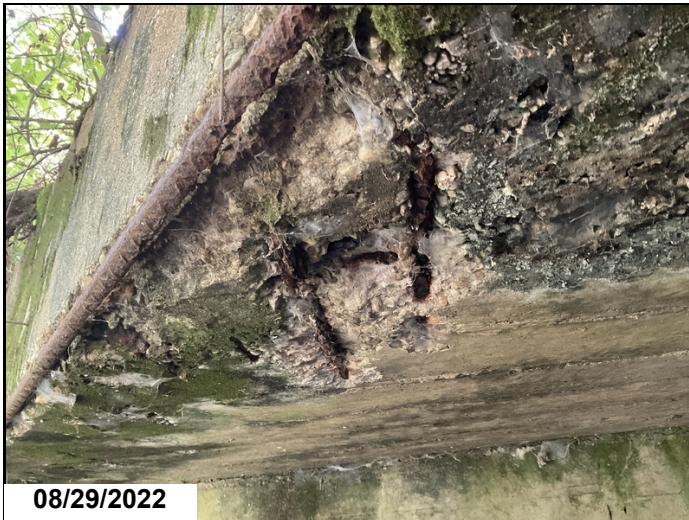
Exposed rebar in barrel #2 soffit, left side
