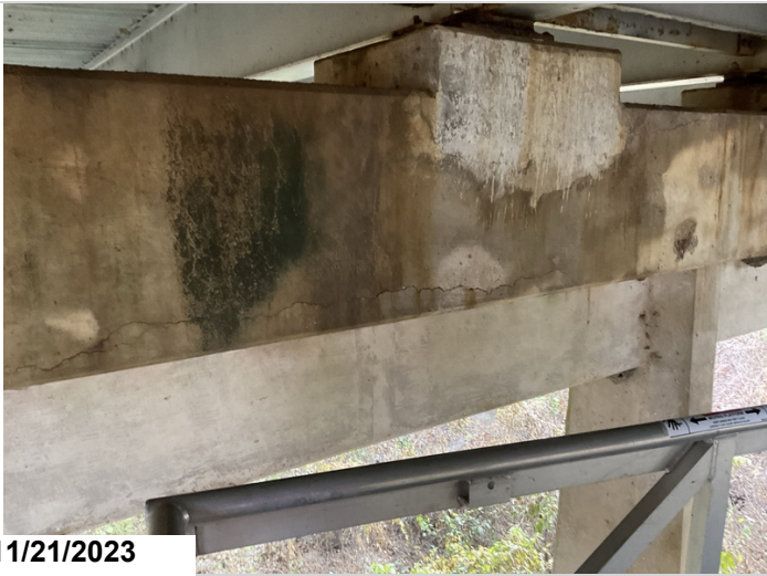
Bent #6 cap back face has cs3 cracks for 10' between girders #2, 5.
