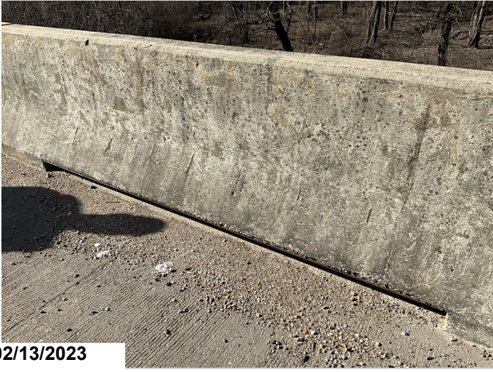
Span 1, right, exposed reinforcing steel, cs 2. Typical 2,3,4, 5, 6, 9
