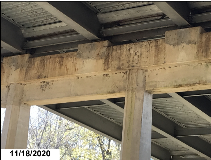
Bent #3 cap ahead face is cracked near top for twenty feet between girders #3,5.
