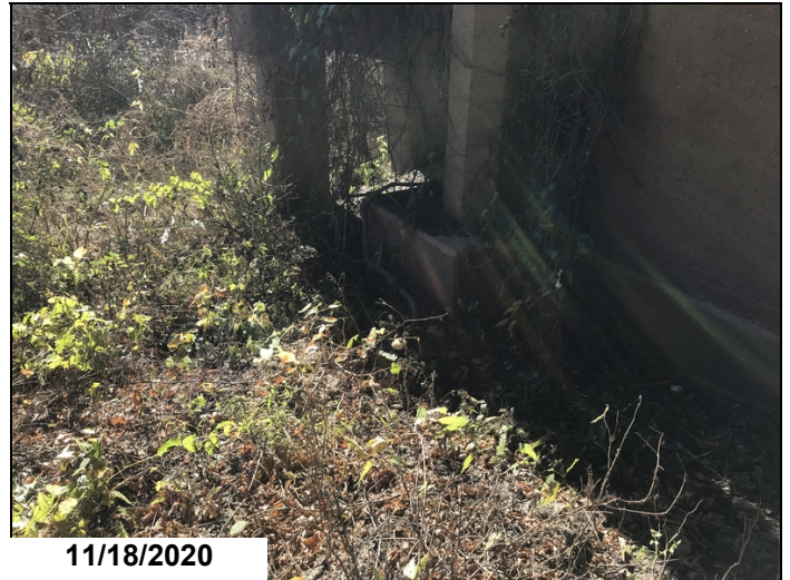
Bent #3 footing on right end exposed 1 1/2 foot.
