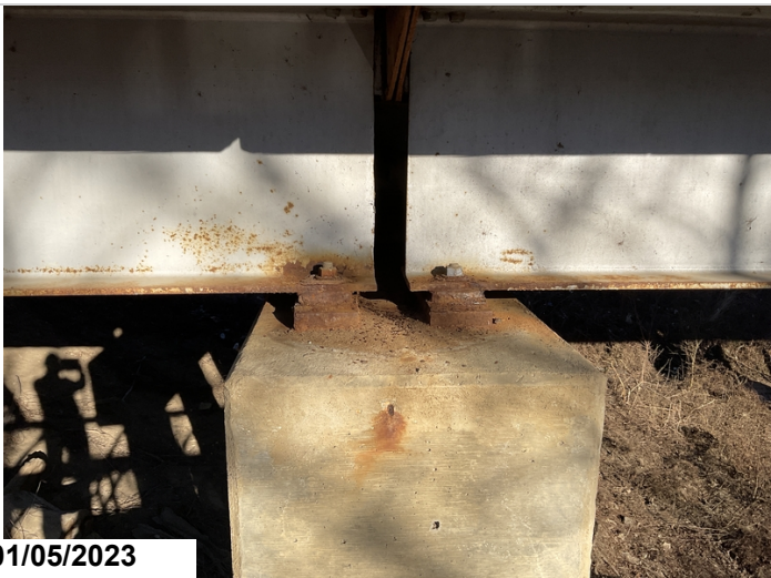
Bent #2 girder #6 bearings are corroded and span #1 and 2 girder #6 bottom flange outside has scaly rust
