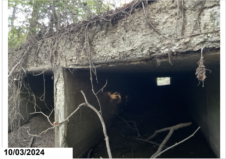
Barrel 2, right end: exposed rebar. 1LF CS3.
