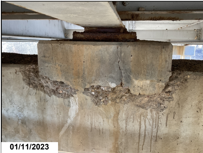
Bent #3 cap back face bearing riser under girders #4 bearing risers have three foot crack with delamination extending underneath bearing masonry plates.
