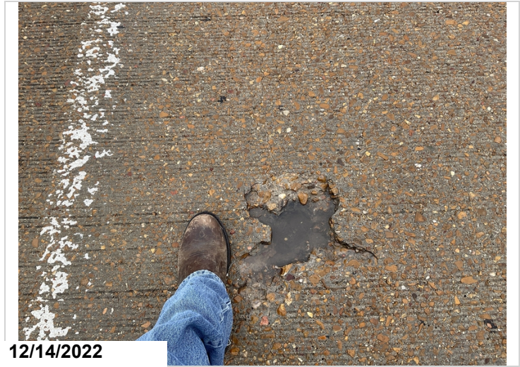
Span #5 deck left lane has one foot spall near mid span
