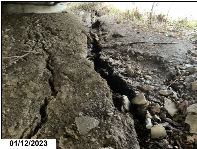
Abutment #2 slope right side has erosion vein up to 2' deep due to roadway runoff
