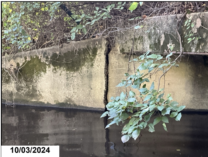
Barrel 2, Left wing wall: 6" of separation from culvert.
