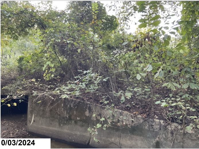
Culvert: heavy vegetation growth on both sides.
