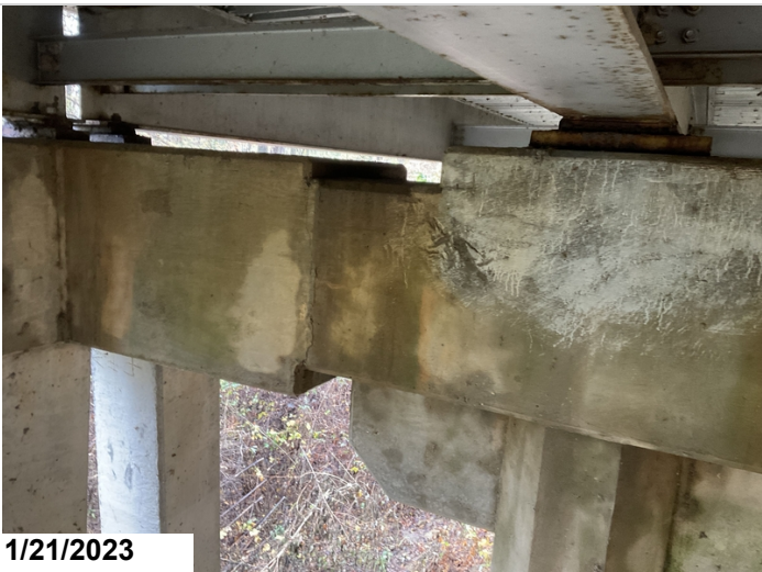
Typical vertical crack at construction joint.
