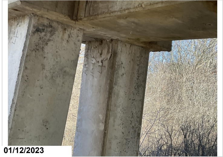
Bent #7 pile #2 has 1' shallow delaminated area at top back face.
