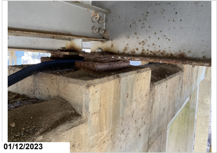
Bent #7 corrosion on girder ends and bearing.
