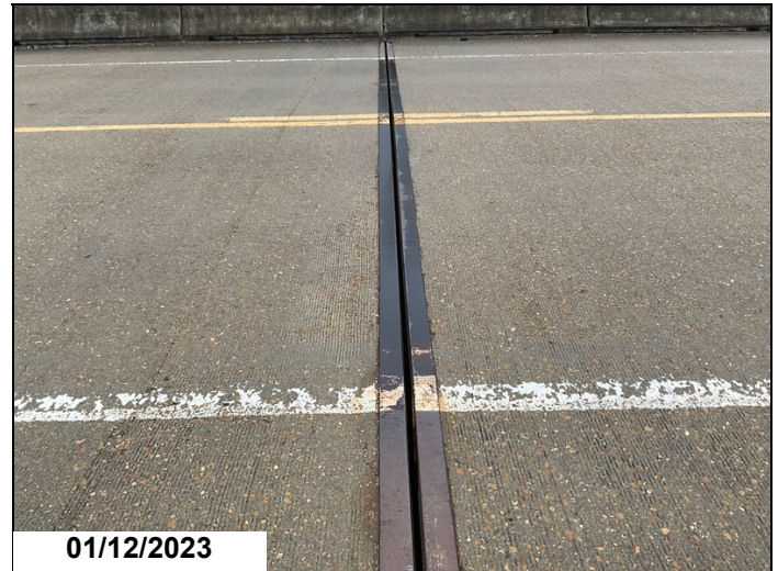
Bent #8 joint has fallen out
