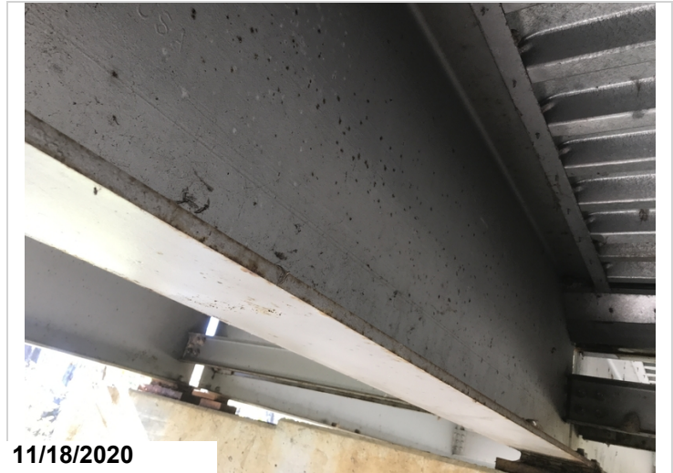
Typical girder paint condition
