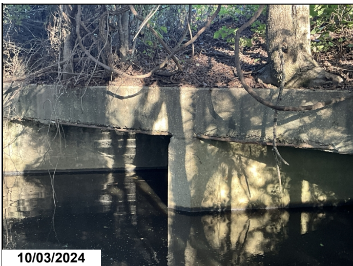
Barrels 1 & 2, Right Headwall: Spalling with exposed reinforcing steel with section loss and loss of bond from concrete. CS4. 2'.
