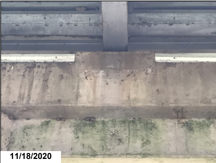
Bent #8 cap ahead face bearing riser under girder #3 is cracked longitudinally full width.
