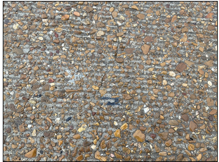
Typical longitudinal deck crack
