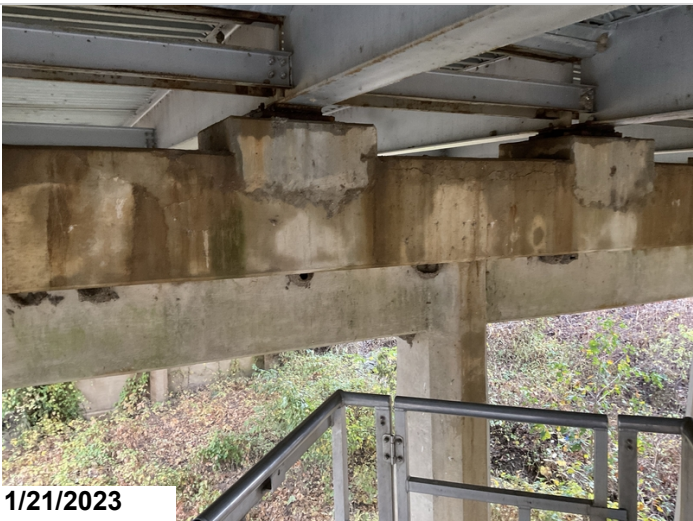
Bent #4 cap ahead face has horizontal cs3 cracks for 20' between girders #2, 5.
