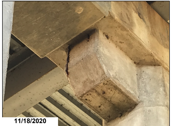
Bent #4 cap bottom left corner near column #3 has one foot spall exposed rebar with 15% section loss.
