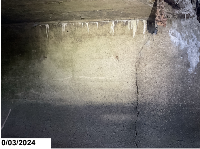
Barrel 2, right end: efflorescence along top corner. 4LF CS2. Vertical crack. 1LF CS3.
