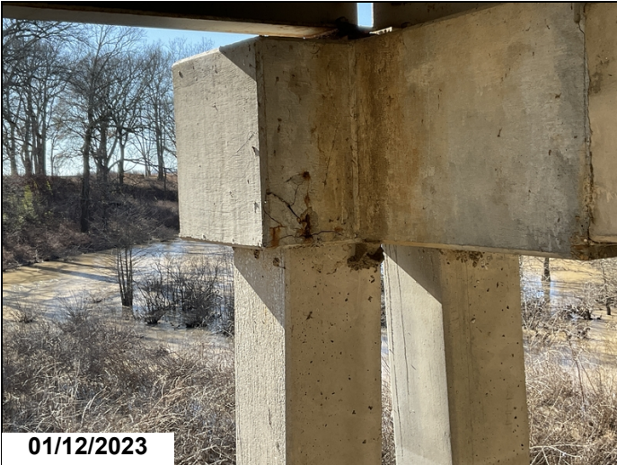
Bent #6 cap ahead face right side under girder #6 cracked and delaminated for one foot with exposed rebar
