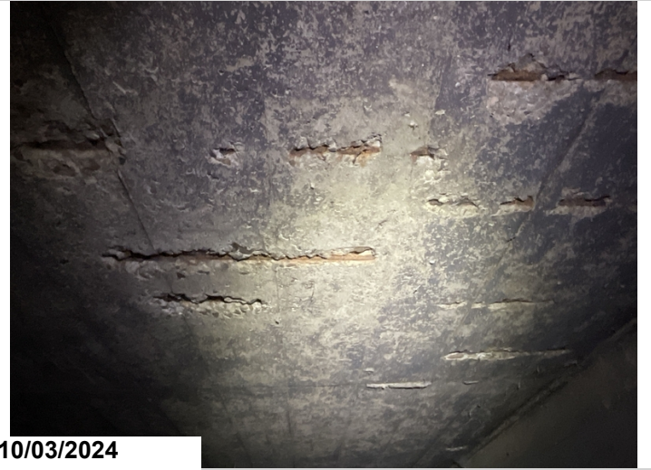
Barrel 2, 15' from left side: exposed rebar. 9 LF cs3
