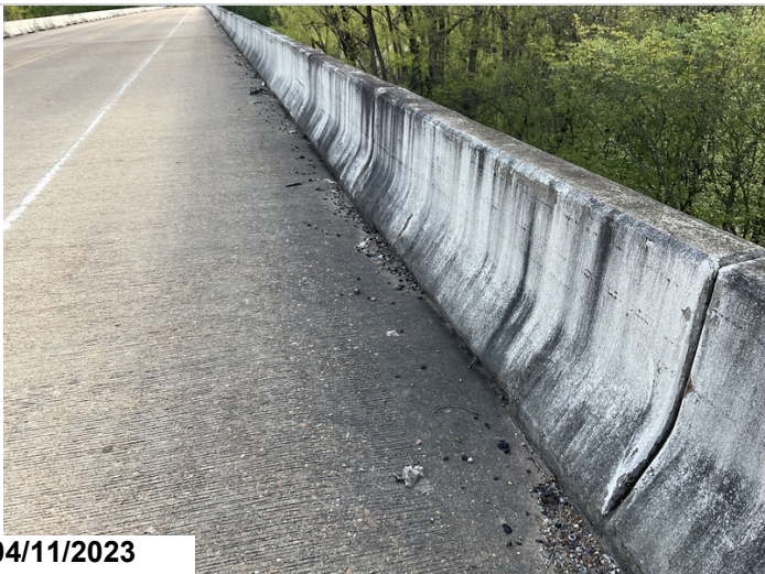
Typical debris in gutters
