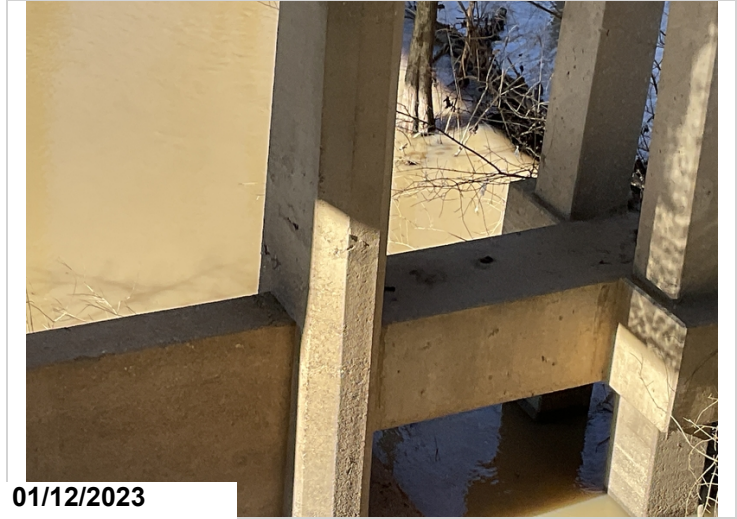
Bent #6 column #1 ahead face and right side above web wall has two spalls with exposed rebar and one delaminated area. Cs3
