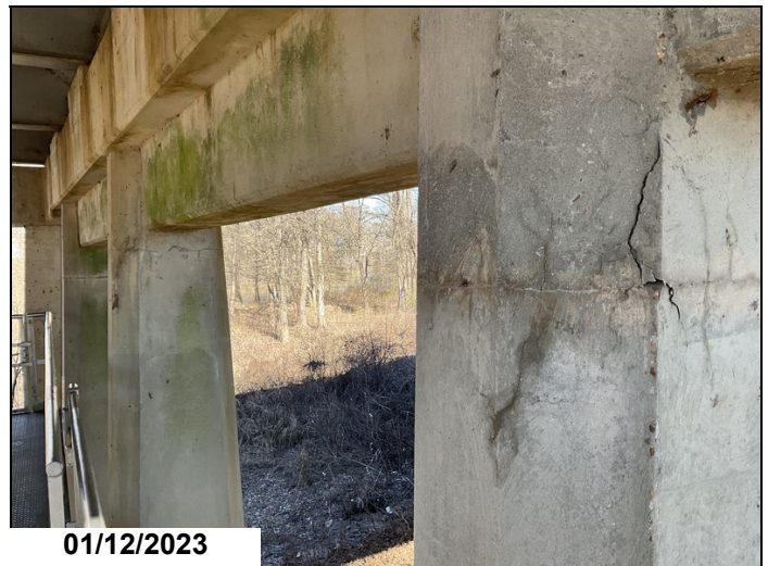
Bent #10 columns #1, 2, 3 have horizontal cracking with light efflorescence six inches to one foot below cap.
