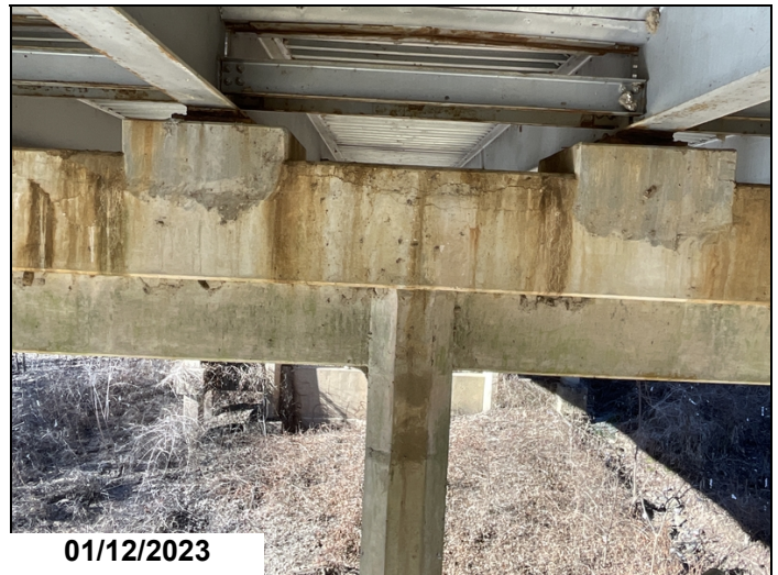
Bent #4 ahead face has horizontal cracking between girders #2 and 5 for twenty feet. Cs3
