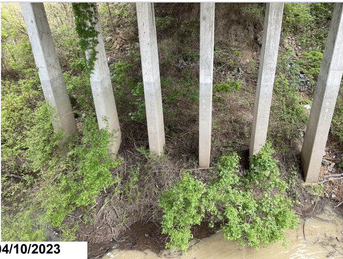
Bent #14 footing is exposed on each end for a few feet.
