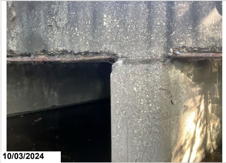
Intermediate wall, Right: Minor spall. CS2.
