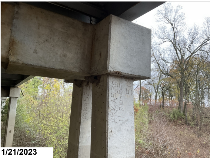
Bent #6 cap back face right side has small spall on corner with exposed rebar minor section loss.
