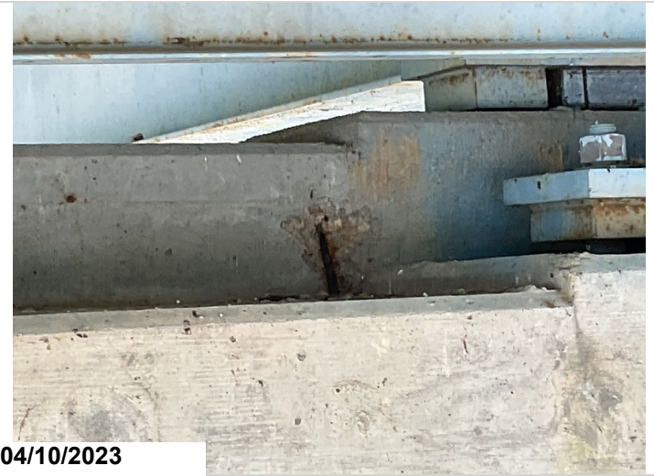
Bent #9 cap on step up between girders #5,6 has a 6" spall with exposed rebar.
