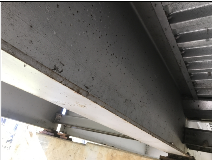
Typical girder paint condition
