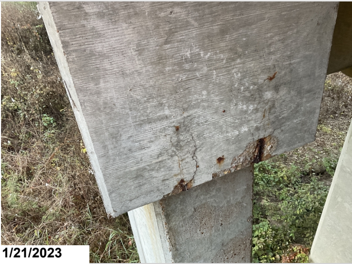
Bent #10 cap ahead face right side has a 6" delaminated area, and a 4" spall with exposed rebar with moderate section loss.
