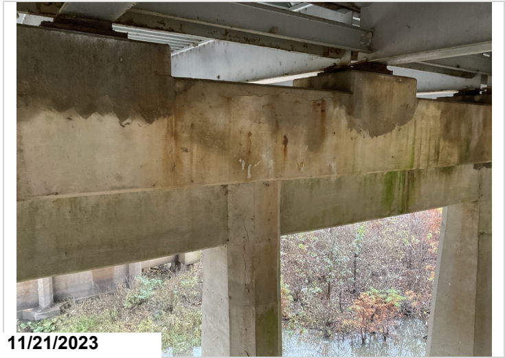
Bent #5 ahead face has cs3 cracks horizontally for 20' between girders #3, 5.
