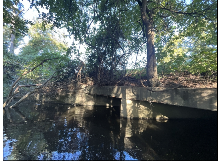
Right side of Culvert: Vegetation growth.
