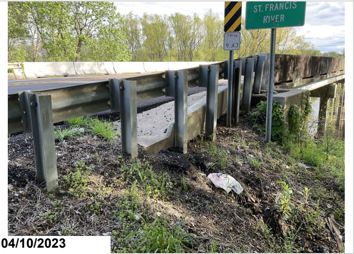
Approach gutter abutment #1 right side has large void under it and has settled.
