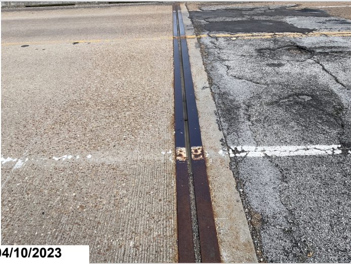
Abutment #2 joint
