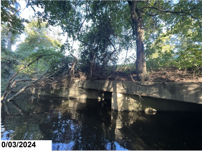
Right side of Culvert: Vegetation growth.
