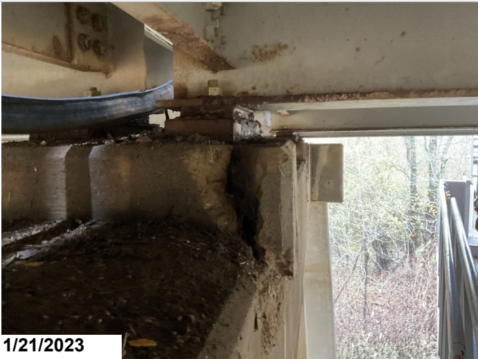
Bent #3 cap back face under girder #4 bearing riser has 3' crack with delamination extending underneath bearing masonry plates.
