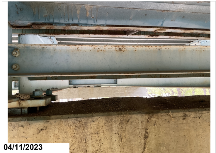
Typical debris on cap bent #5
