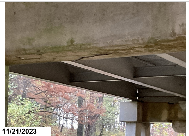
Bent #9 cap bottom has cracks and delaminated area for 2' between columns #4 and #5.
