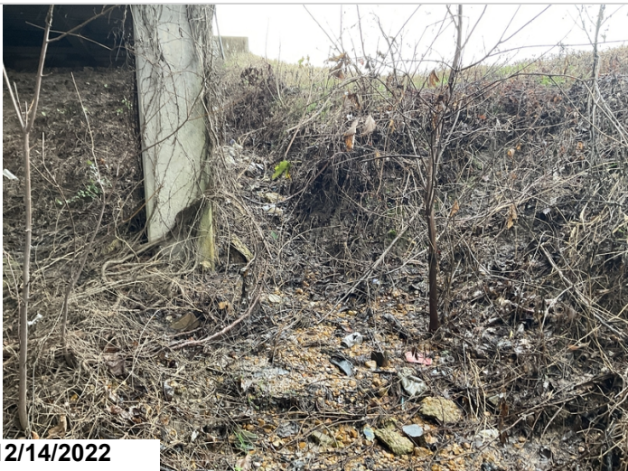
Spans #1 and 2 left slope eroded up to three feet beside bridge
