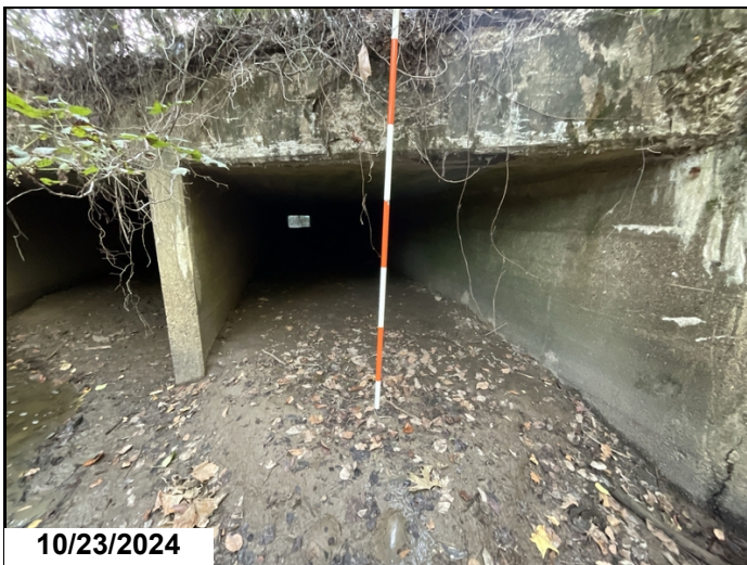
Barrel 2, left side: sediment build up.
