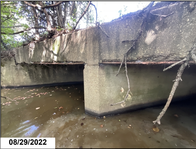
Exposed rebar in right side head wall
