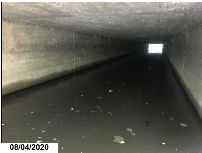
Barrel #2 two feet of silt in barrel full length.
