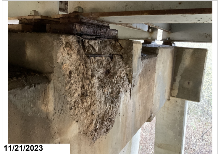
Bent #3 cap back face bearing riser spalled under girder #5 for 3' extending underneath bearing masonry plate up to 1" with exposed rebar moderate section loss.
