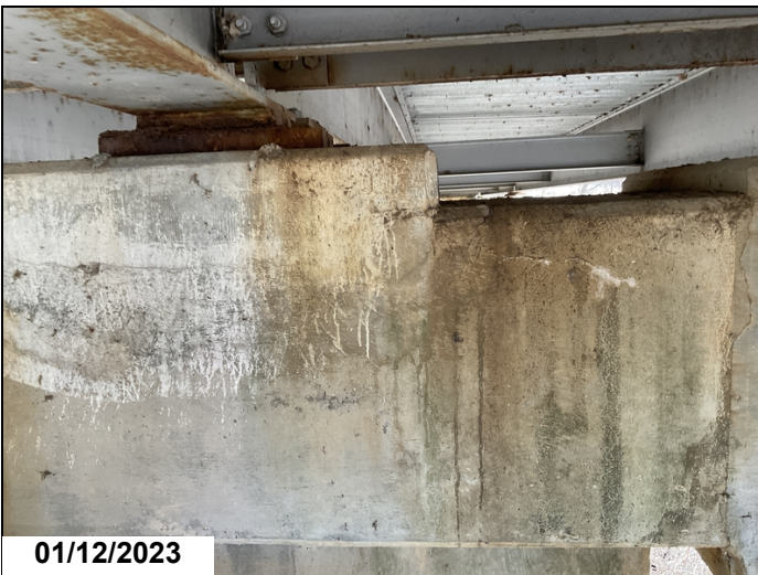
Bent #10 cap back face under girder #5 has two feet of horizontal cracking with light efflorescence
