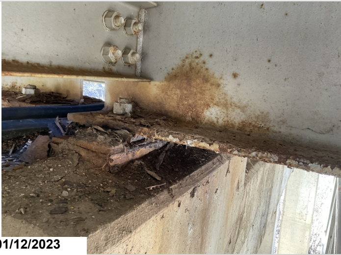
Corrosion on bearings and girder ends
