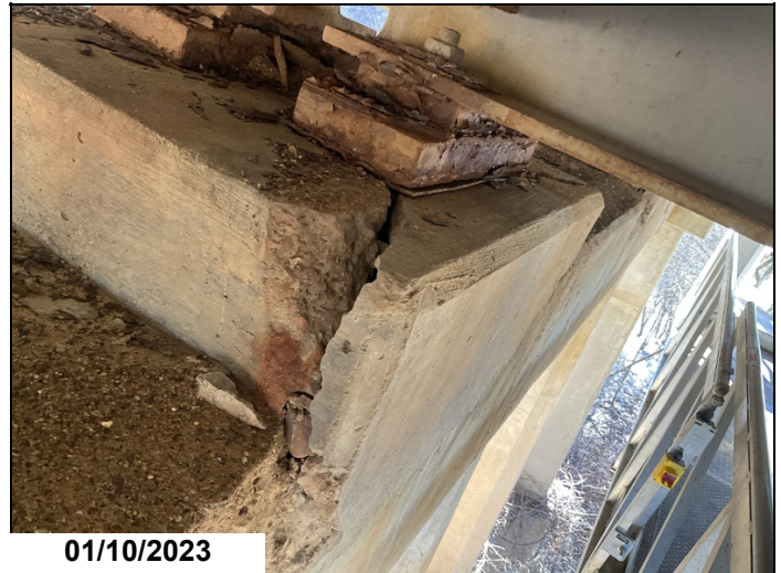
Bent #3 cap back face bearing riser under girder #3 bearing risers have three foot crack with delamination extending underneath bearing masonry plates.
