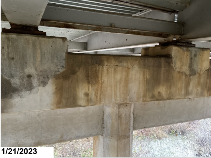
Bent #4 cap back face has horizontal cs3 cracks for 4' between girders #3 and 4.
