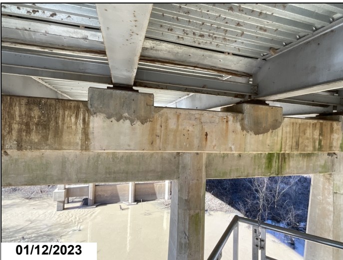
Bent #5 cap ahead face cracked horizontally between girders #3 and 5 twenty feet near top. Cs3
