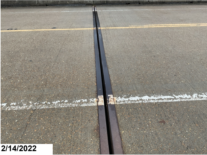
Bent #7 joint has fallen out
