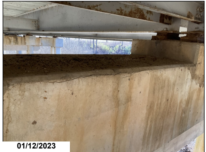
Bent #5 cap back face at top cracked horizontally for twelve feet. Cs3
