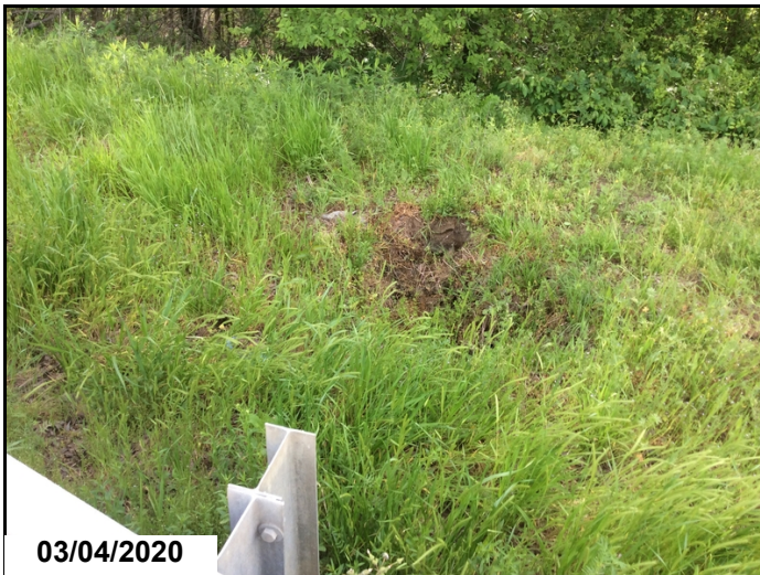
2' sink hole abutment #1 right side 50' from bridge end.
