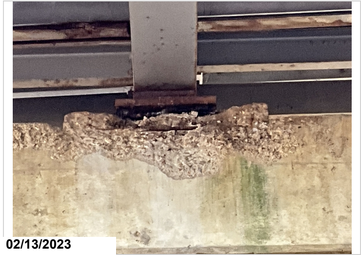
Bent 10 ahead bearing 5, loss of bearing area cs 3. 30%.
