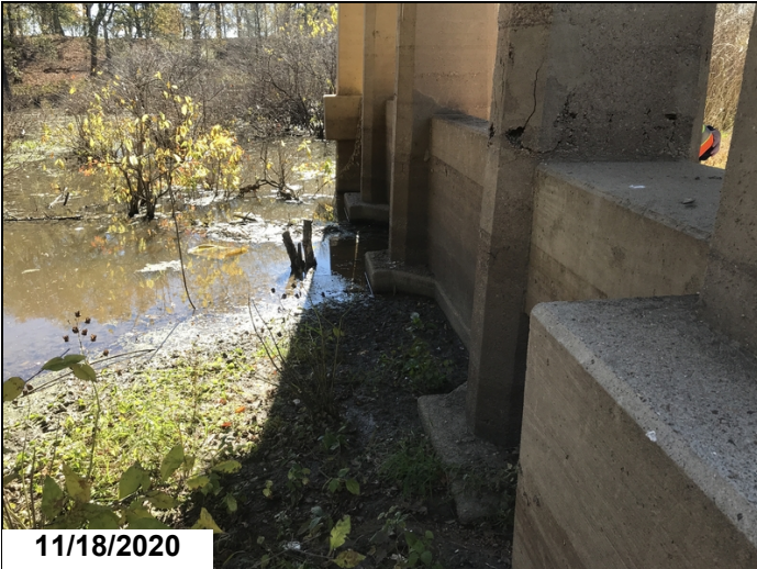
Bent #4 footing exposed right end 2' and 3' on the left end.
