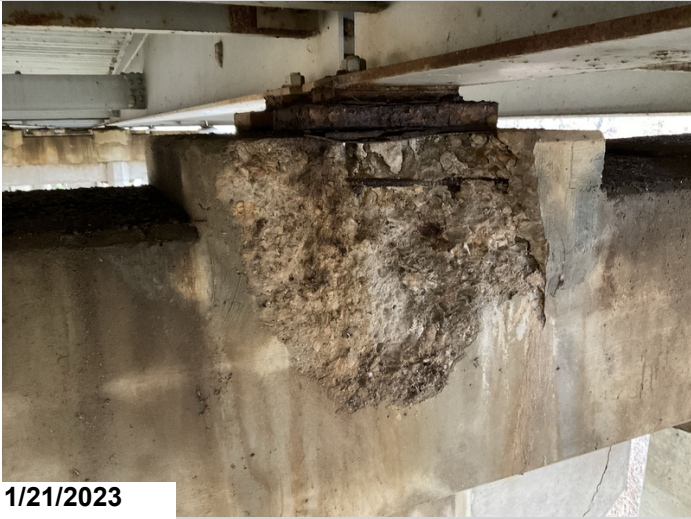
Bent #3 cap back face bearing riser spalled under girder #5 for 3' extending underneath bearing masonry plate up to 1" with exposed rebar moderate section loss.
