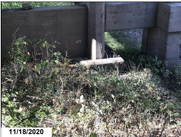
Bent #10 footing on left end is exposed 2'.
