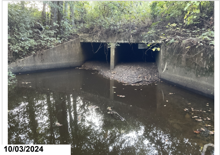
Left end of structure. Sediment accumulation in both boxes.
