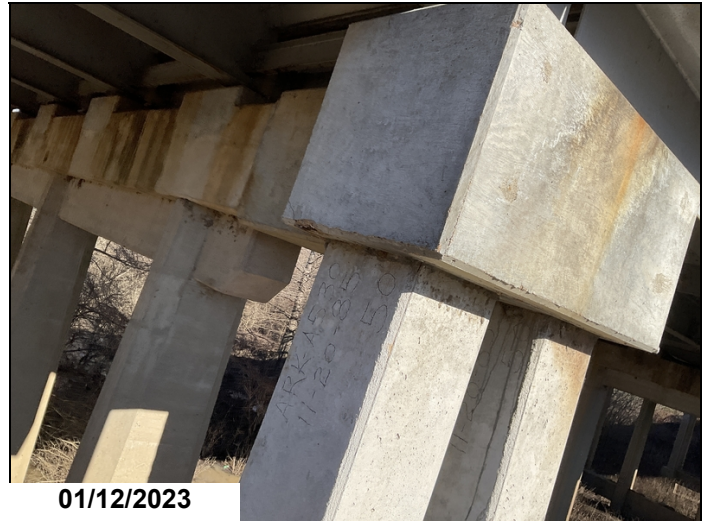
Bent #6 cap back face right side has small spall on corner with exposed rebar.
