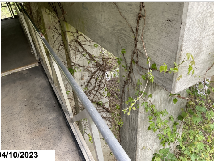
Typical vines growing on bent
