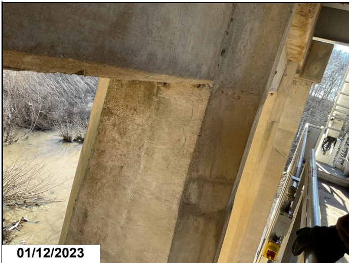
Bent #4 column #2 has one foot of vertical cracking near top. Cs2
