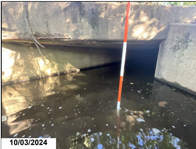
Barrels 1 & 2: 2' of silt build up.
