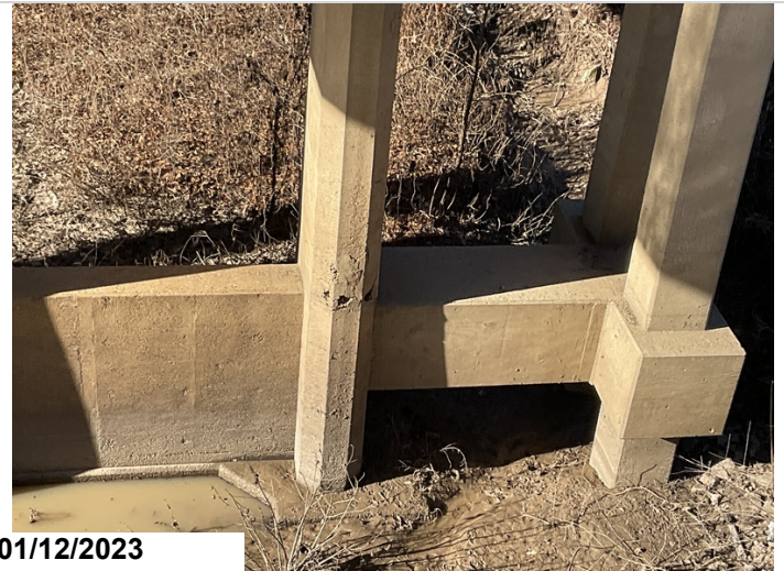
Bent #4 column #1 ahead face has one foot delaminated area with spalling at footing.
