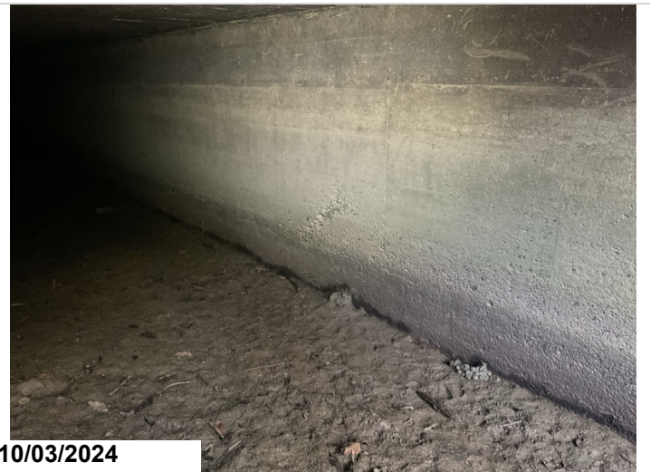
Barrel 2, intermediate wall, 20' from left end: abrasion with aggregate loss. 2LF CS3.
