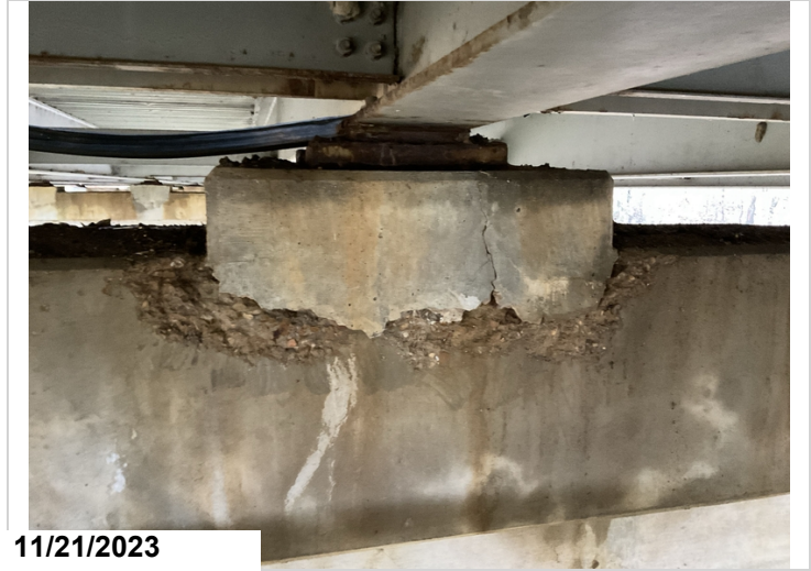
Bent #3 cap back face under girder #4 bearing riser has 3' crack with delamination extending underneath bearing masonry plates.
