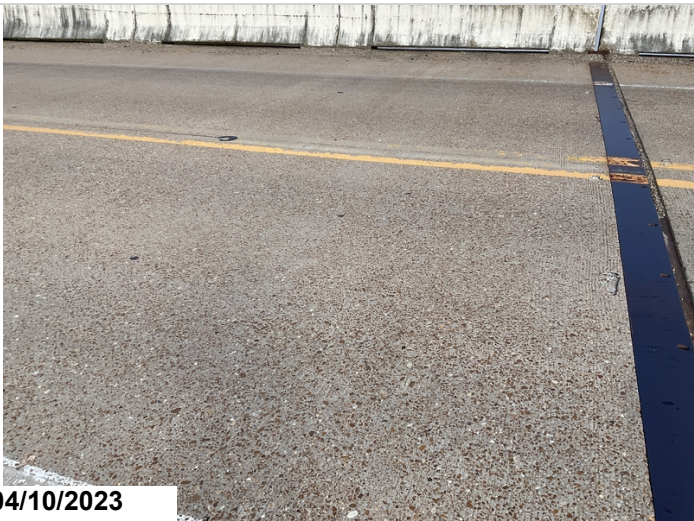
Span #11 at bent #12 joint has two six inch shallow spall in each lane with no exposed rebar.
