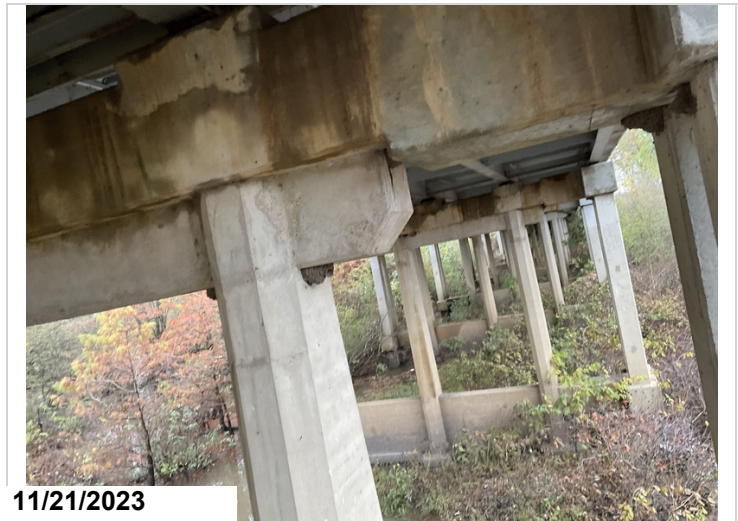
Bent #4 cap right end of old cap section at bent # 3&5 has small spalls with exposed rebar minor section loss.
