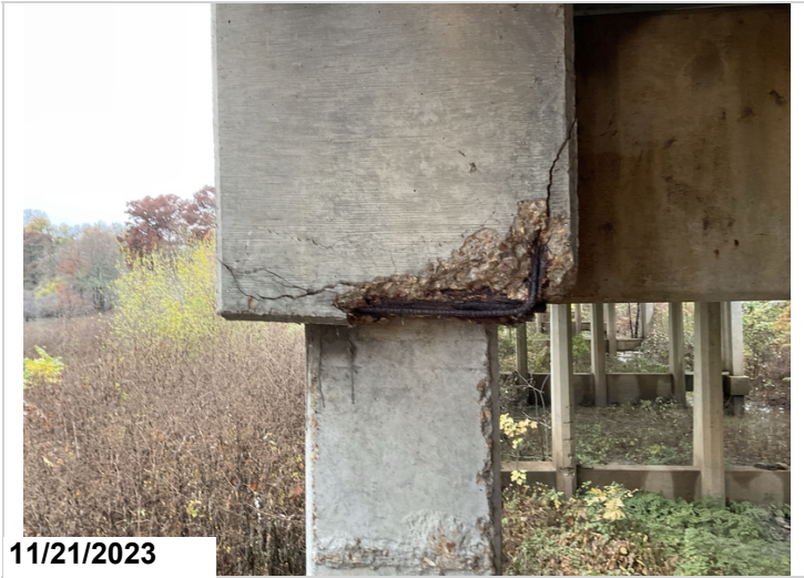
Bent #9 cap ahead face right side has cracks and spalled with exposed rebar minor section loss for 2'.
