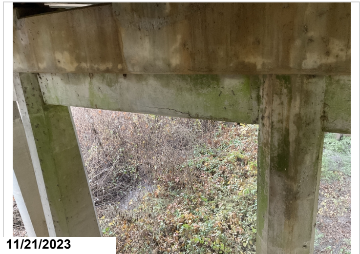
Bent #9 cap ahead face has cs3 cracks and delaminated area for 2' between columns #2, 3.
