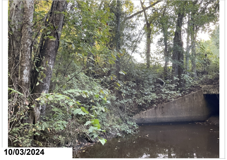
Culvert: heavy vegetation growth on both sides.
