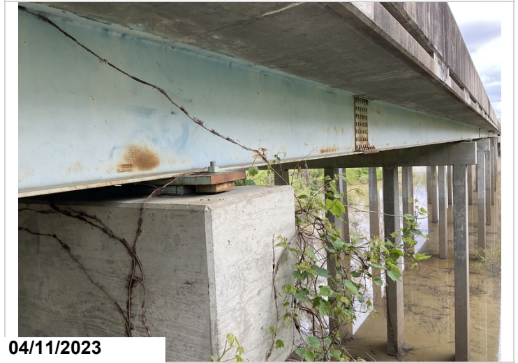
Typical outside girder condition
