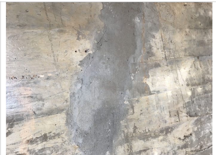
Abutment 1 outside of girder 4, diagonal crack.
