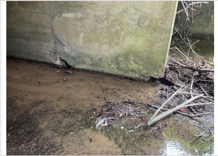
Barrel # 2 Lt interior wall concrete deterioration with full depth voids.
