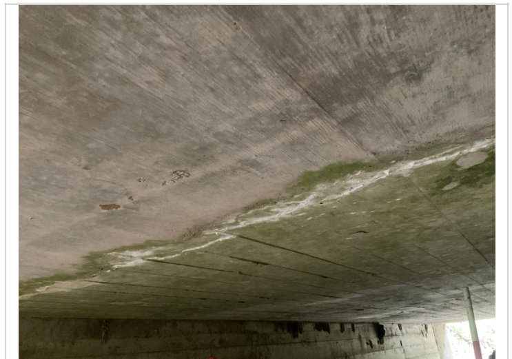
Barrel # 2 Lt top slab transverse cracking with light efflorescence buildup
