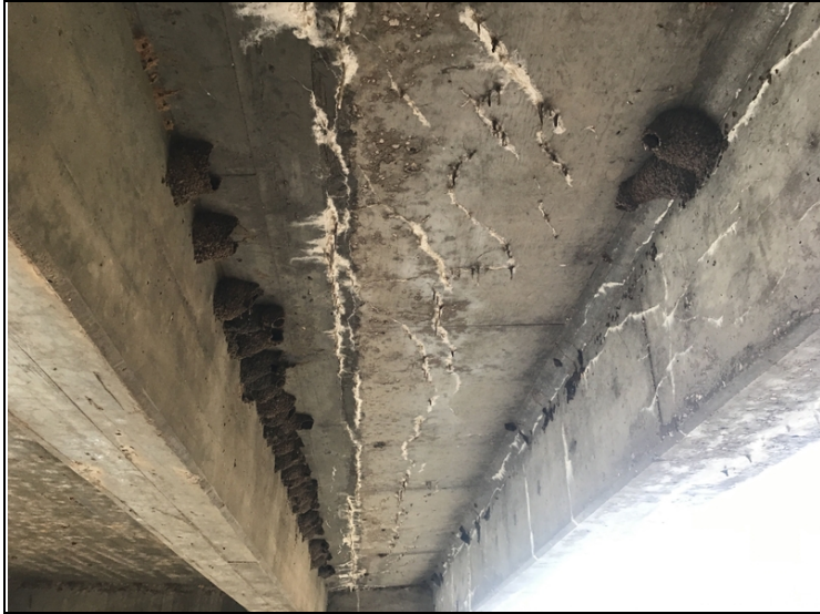
Span 1 bay 3, cracks with efflorescence buildup in the soffit.
