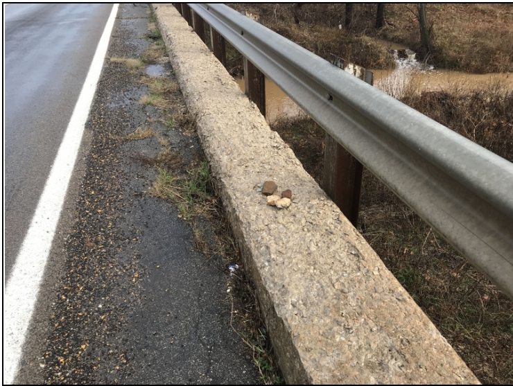
Left curb, concrete deterioration.
