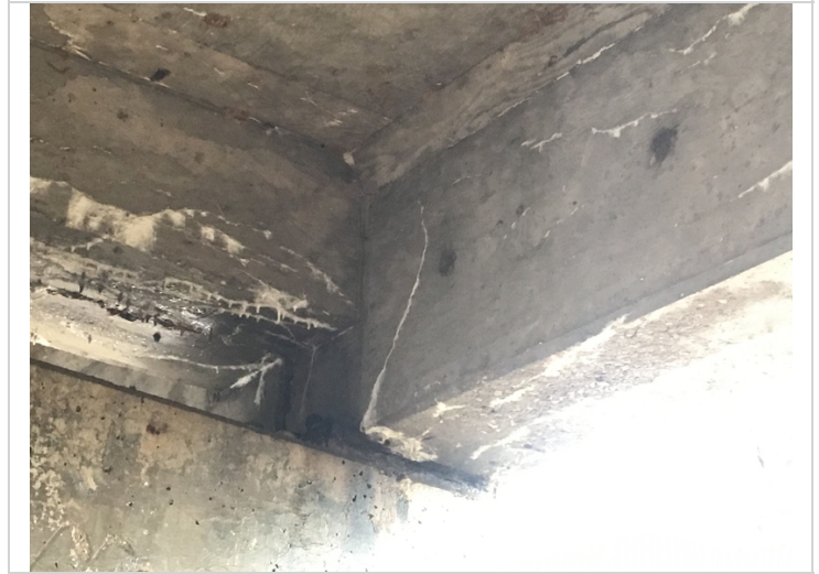
Span 2 girder 1 at bent 2, diagonal crack with efflorescence.
