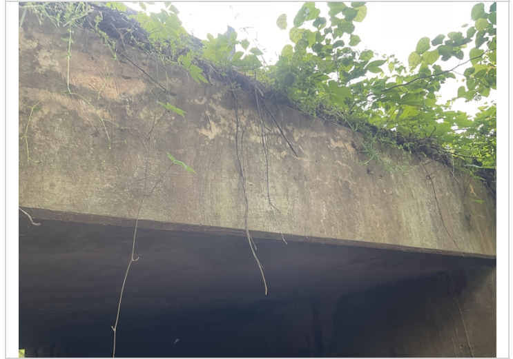
Barrel # 2 Lt headwall map cracking with efflorescence buildup.
