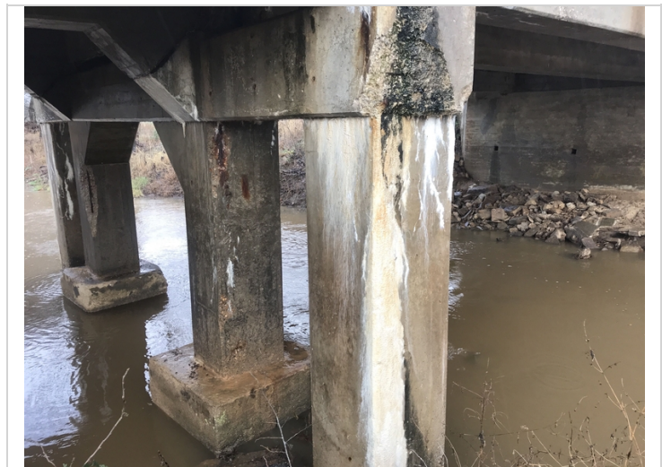
Bent 2 c1 efflorescence with build up C2 exposed rebar with section loss
