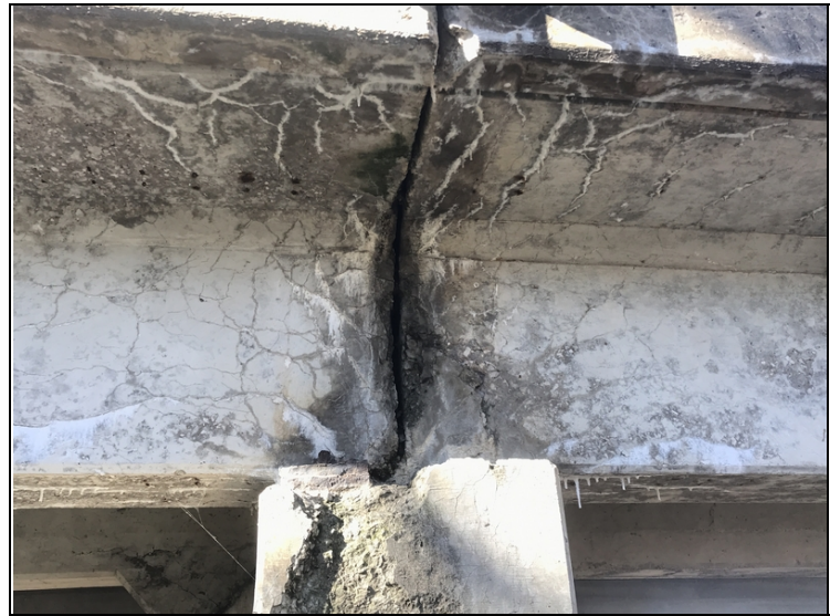
Girder # 1 over bent # 2-Heavy map cracking.
