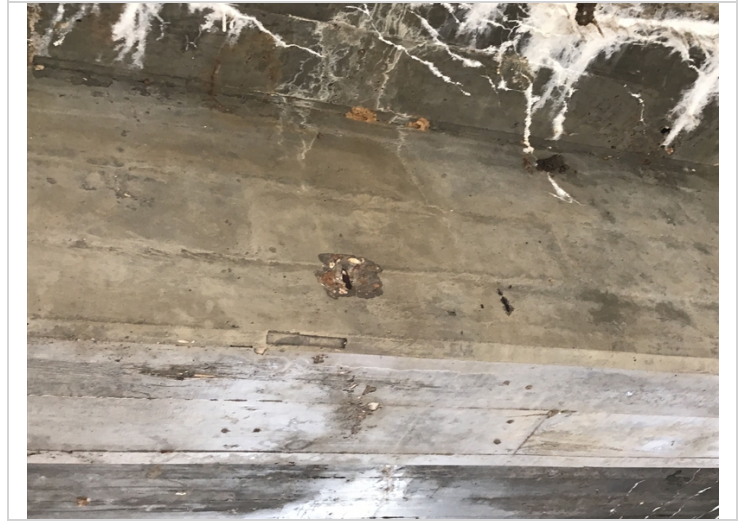
Span 2 girder 2, exposed rebar.
