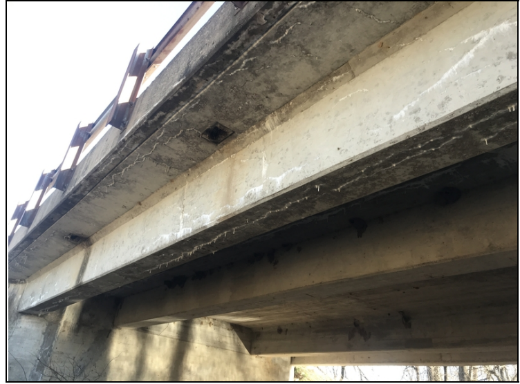
Span # 1, girder # 4-Cracking with efflorescence.
