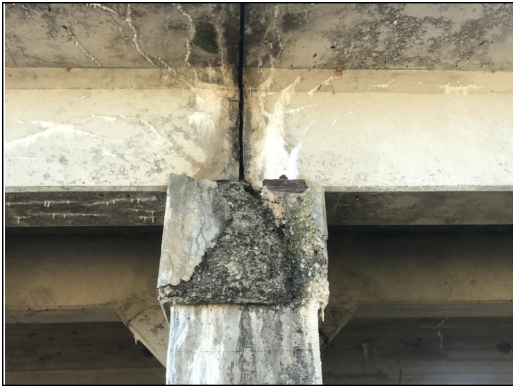
Bent # 2 cap, right side-Concrete deterioration / spalling.
