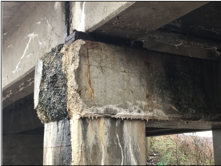
Bent 2 right side, large spall and map cracking with efflorescence.
