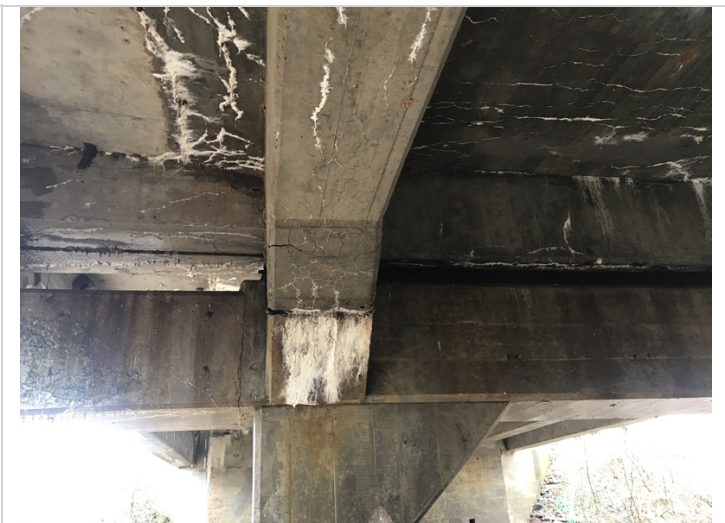
Span 2 girder 3 at bent 2, large cracks in the haunch.
