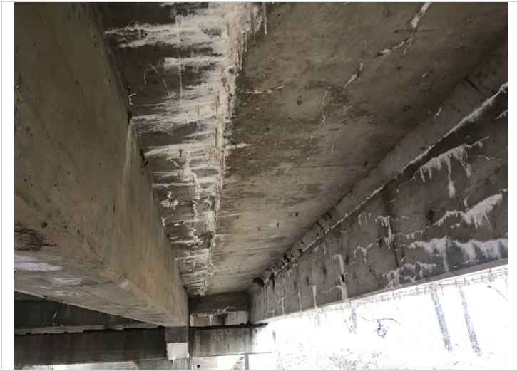
Span 2 bay 1, cracks with efflorescence in the soffit.
