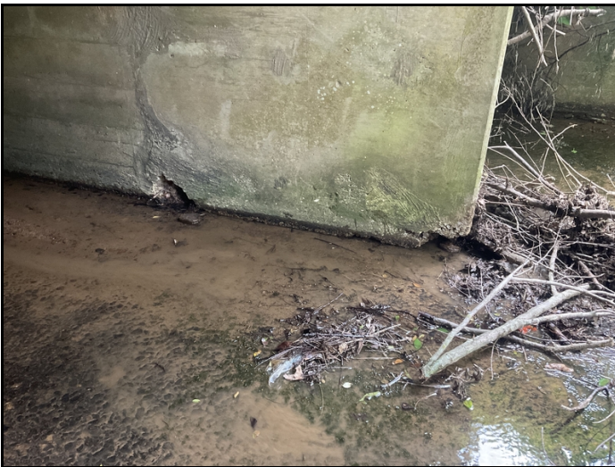
Barrel # 2 Lt interior wall concrete deterioration with full depth voids.
