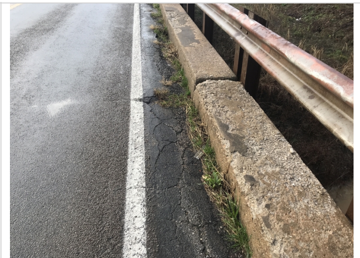
Right side , wearing surface cracked and delaminated.
