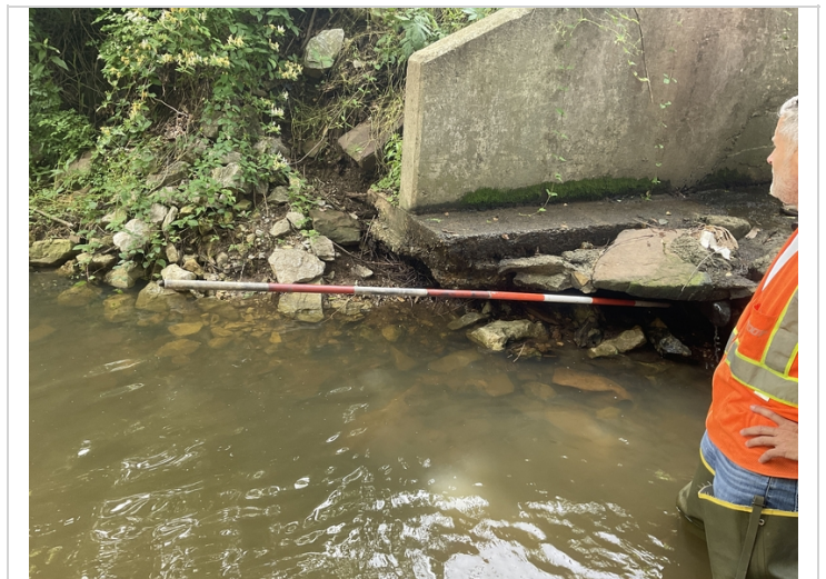
Barrel # 1 Rt wing wall undermining.
