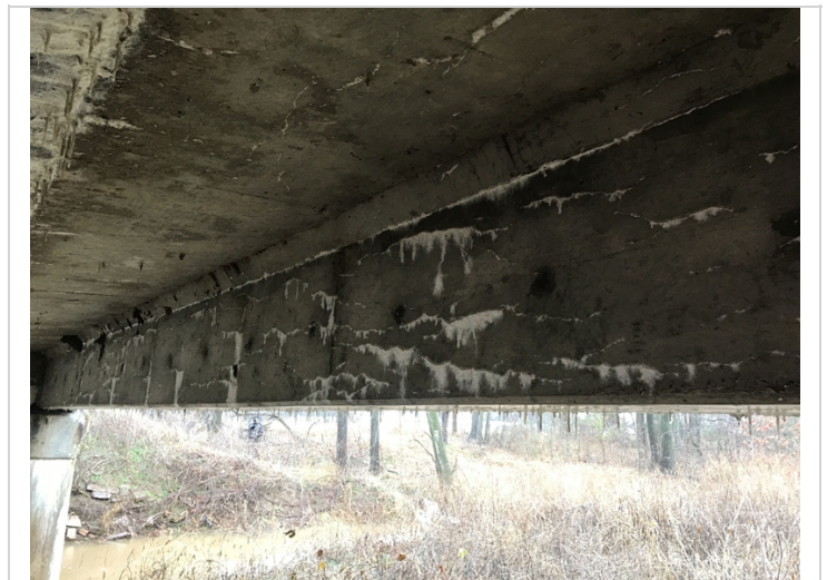
Span 2 girder 1, cracks with efflorescence.
