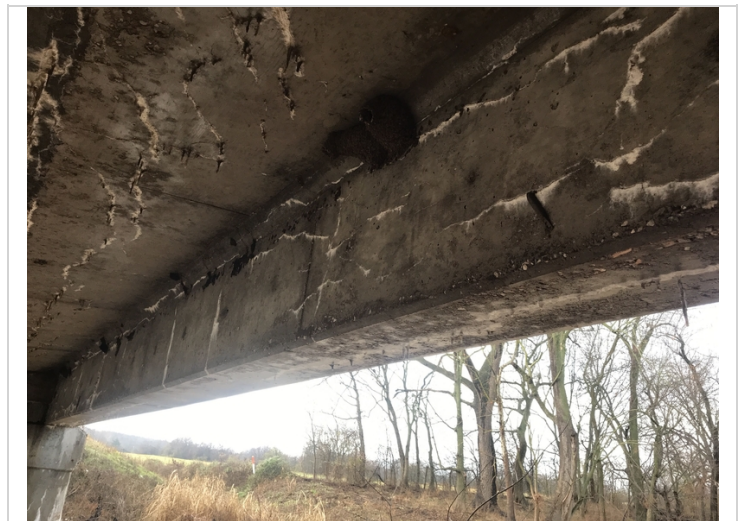
Span 1 girder 4, cracks with efflorescence.
