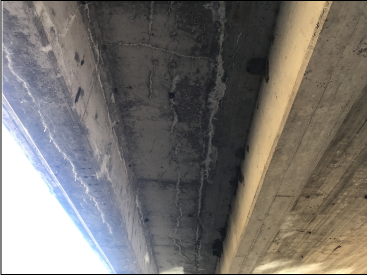
Span # 1, bay # 3-Cracking with efflorescence.
