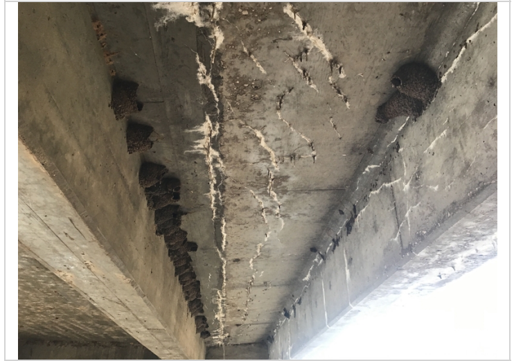
Span 1 bay 3, cracks with efflorescence buildup in the soffit.
