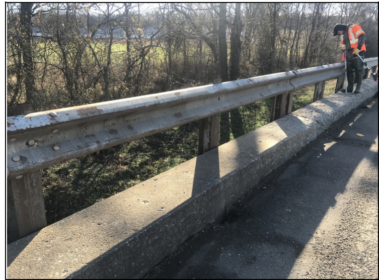
Rust forming on bridge railing.
