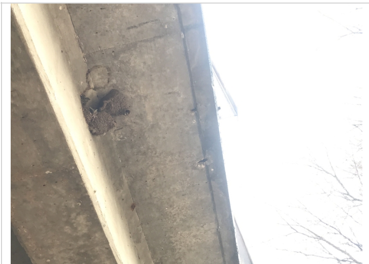
Span 1 left edge, exposed rebar.
