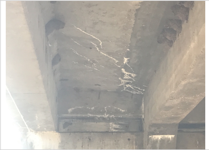
Span 1 bay 1 at bent 2, cracks with efflorescence in the soffit.
