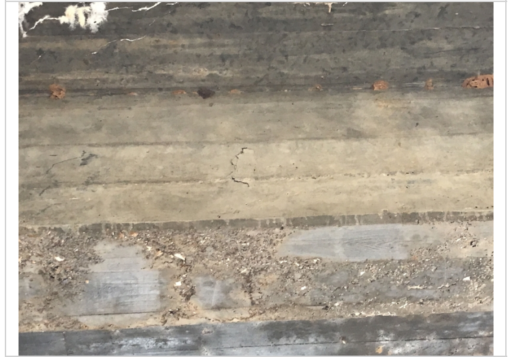
Span 1 girder 2 near bent 2, delaminated area.
