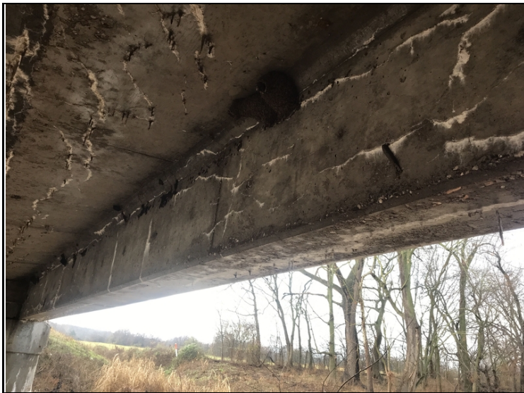
Span 1 girder 4, cracks with efflorescence.
