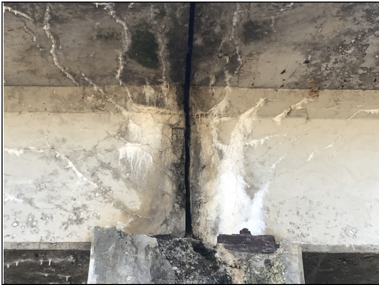
Girder # 4 over bent # 2-Cracking with efflorescence.
