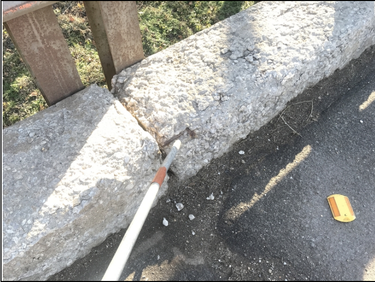
Span # 2, left curb at bent # 2-Concrete spalling with exposed reinforcing steel.
