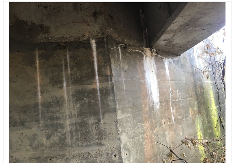
Abutment 2 at girder 4, efflorescence with buildup.
