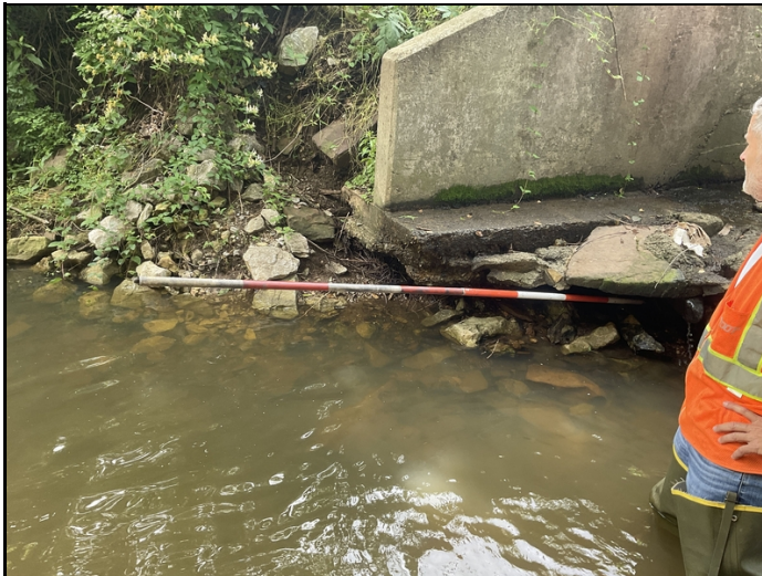
Barrel # 1 Rt wing wall undermining.
