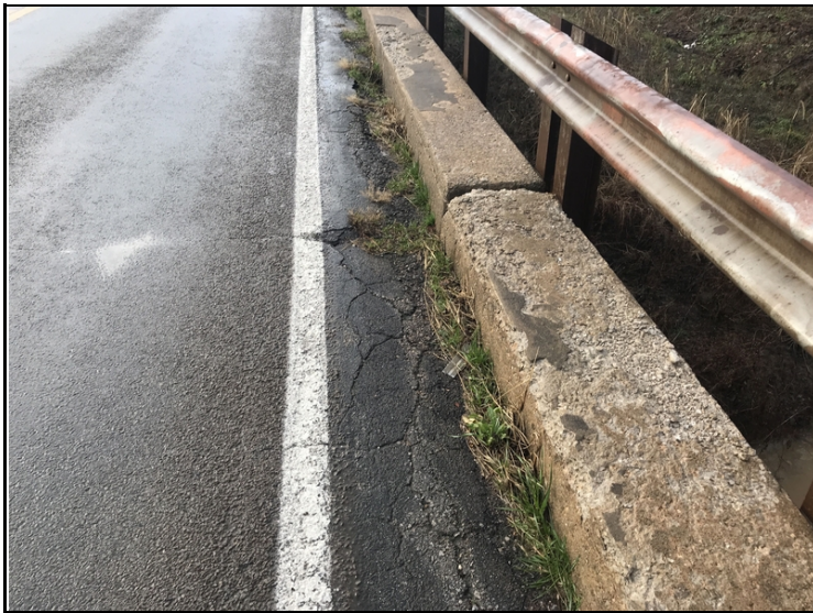
Right side , wearing surface cracked and delaminated.
