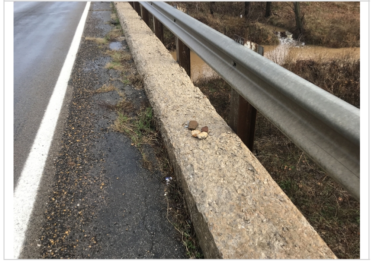
Left curb, concrete deterioration.
