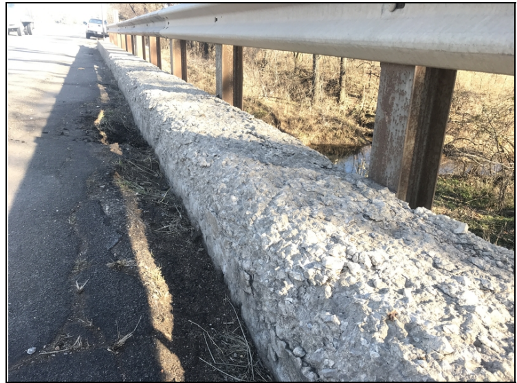
Span 2, left curb-Concrete deterioration / spalling.
