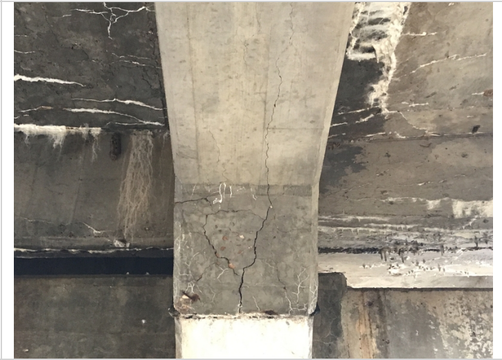
Span 2 girder 2 at bent 2, large crack in the girder.
