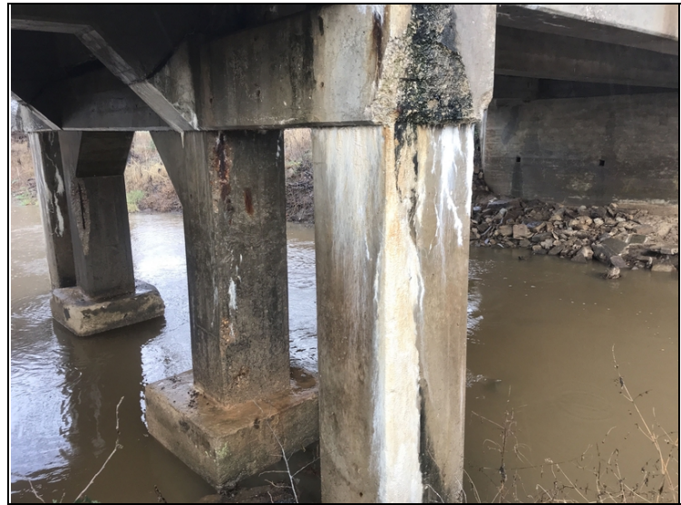
Bent 2 c1 efflorescence with build up C2 exposed rebar with section loss
