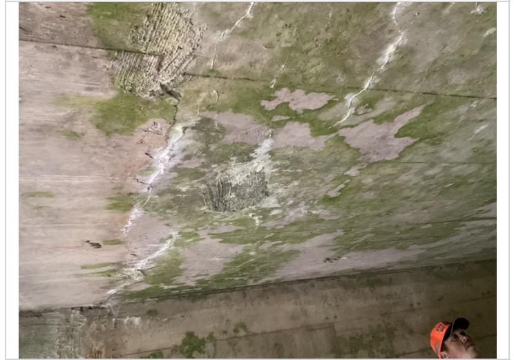
Barrel # 2 Lt top slab cracking with efflorescence buildup.
