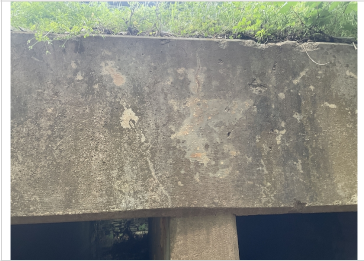
Rt headwall diagonal shear type crack and partial height vertical crack over the interior wall.
