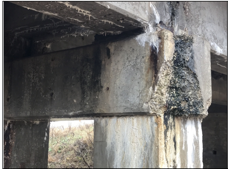
Bent 2 left side, large spall and map cracking.
