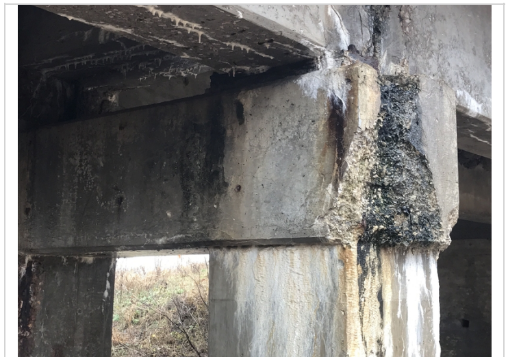
Bent 2 left side, large spall and map cracking.
