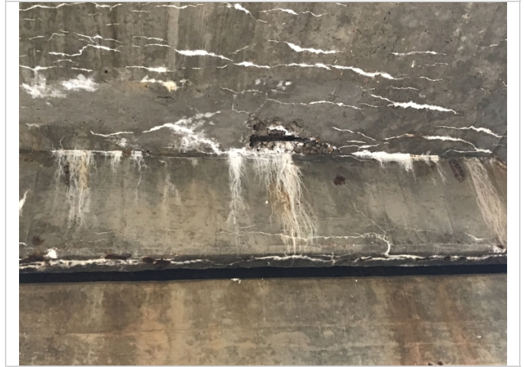
Span 2 bay 2, exposed rebar in soffit near bent 2.
