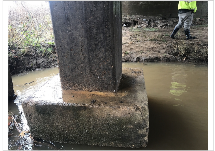
Bent 2 column 2, cracks in the column and collar.
