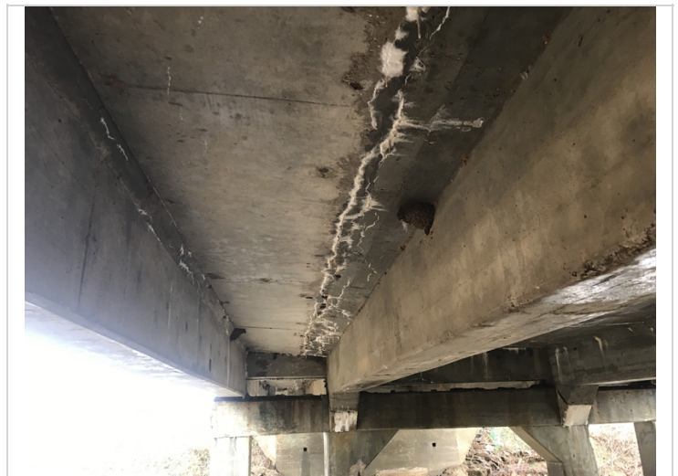
Span 2 bay 3, cracks with efflorescence in the soffit.
