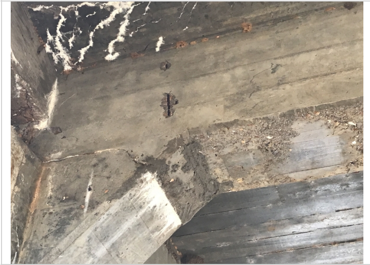
Span 1 girder 2 near bent 2, exposed rebar.
