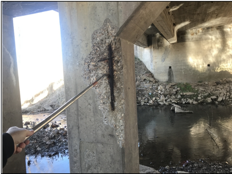
Bent # 2, column # 3-Spalling with exposed reinforcing steel.
