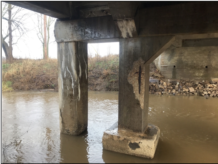
Bent 2 C3 exposed rebar with section Loss C4 efflorescence with heavy build up
