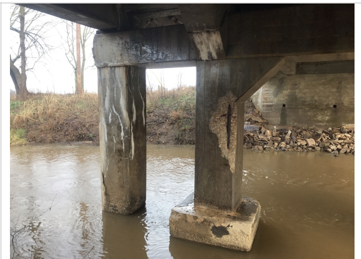
Bent 2 C3 exposed rebar with section Loss C4 efflorescence with heavy build up
