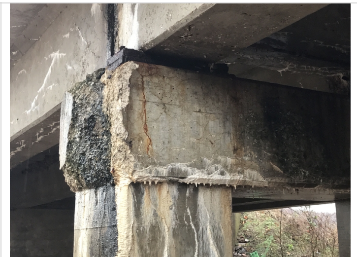
Bent 2 right side, large spall and map cracking with efflorescence.
