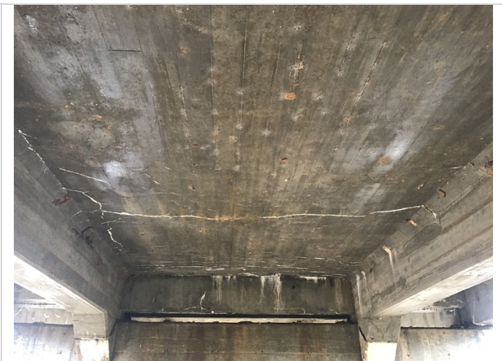
Span 2 bay 2, cracks with efflorescence in the soffit.
