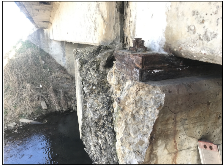
Bent # 2 cap, right end-Concrete deterioration / spalling.
