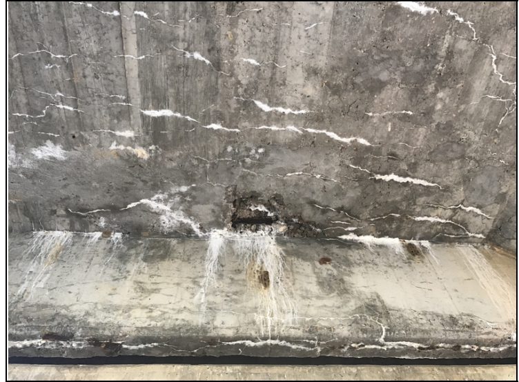
Span # 2, bay # 2 at bent # 2-Spalling with exposed reinforcing steel.
