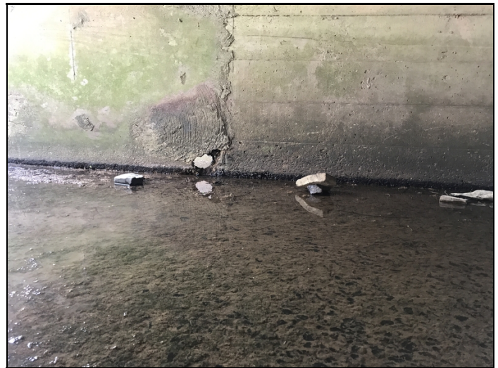
Hole through center wall. Inlet end of structure.
