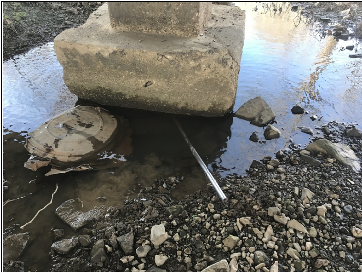
Bent 2, Column # 3-Undermining that reaches face of column.
