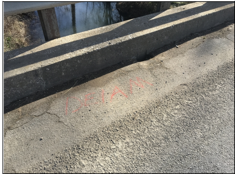
Asphalt in shoulders appears to be delaminated when sounded.
