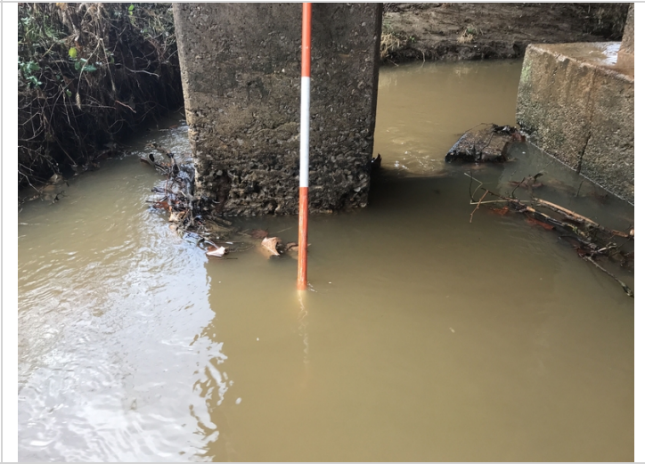
Bent 2 column 1, severe abrasion and exposed rebar.
