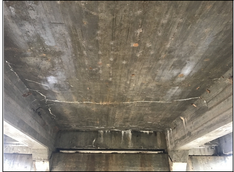
Span 2 bay 2, cracks with efflorescence in the soffit.
