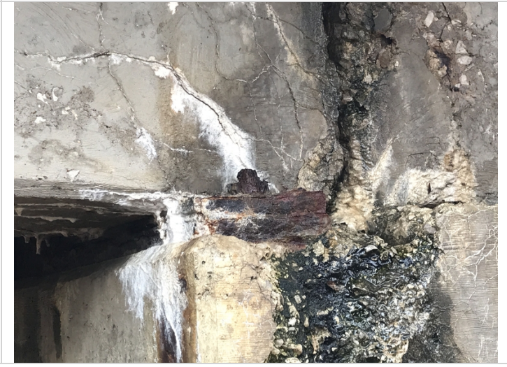
Girder 1 bent 2 ahead side, flaking rust.
