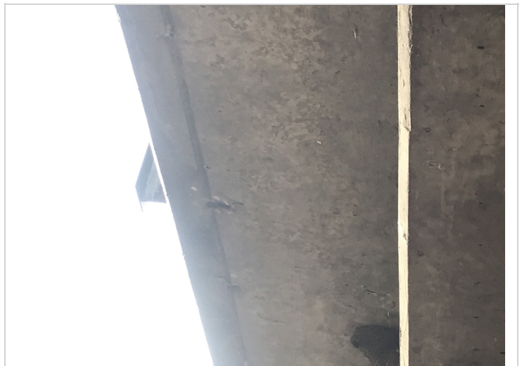
Span 1 left side, exposed rebar in the overhang soffit
