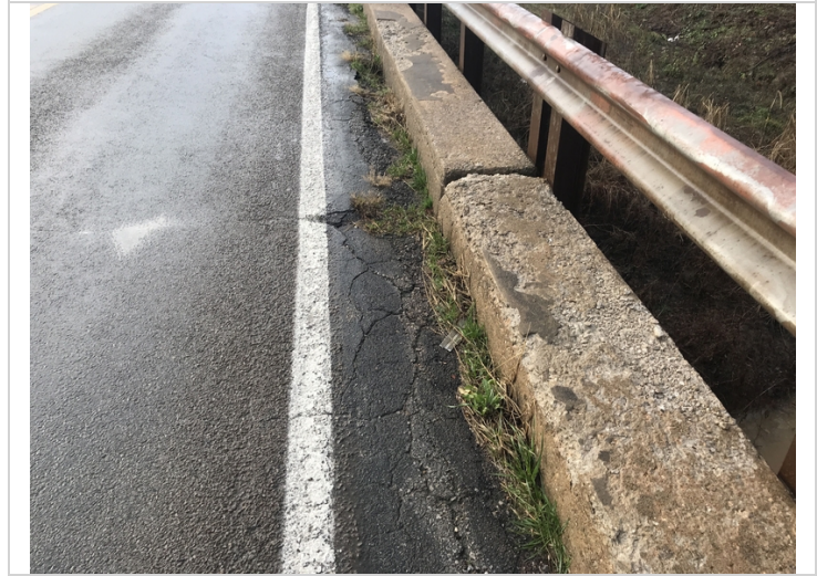
Right side , wearing surface cracked and delaminated.
