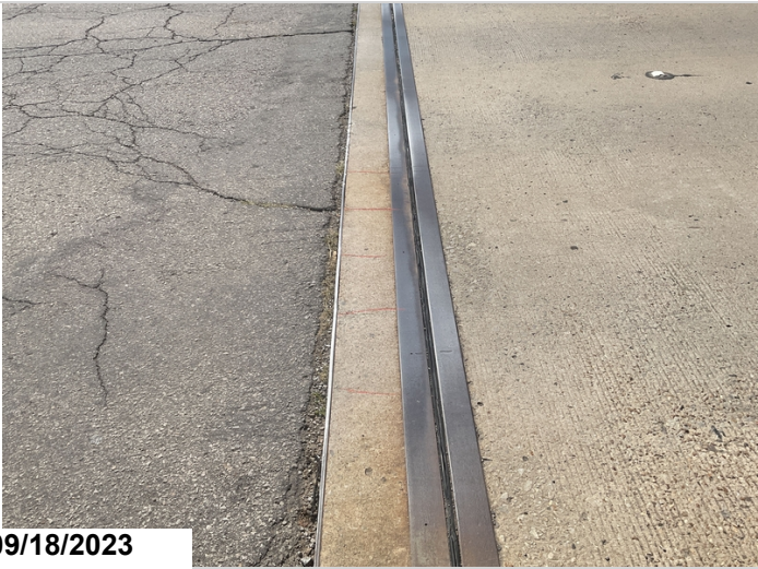
Abutment 2-Transverse cracks in top of backwall
