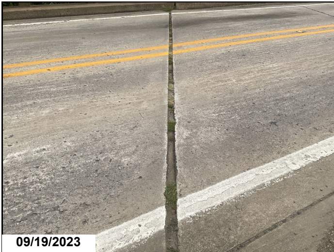
09/19/2023 Abutment # 2 expansion joint-Debris impaction.
