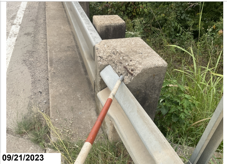
Abutment 2, left end post-Collision damage
