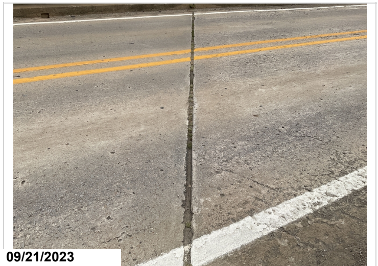
09/19/2023 - RSM & SPC: Slab expansion joint sealant is deteriorated/ missing with incompressible material in the joints.
