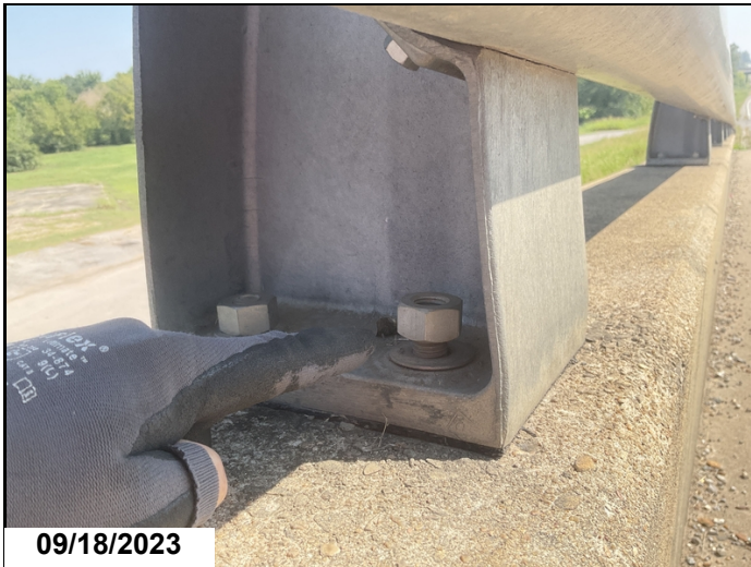
Loose anchor bolt nuts that attach metal railing posts to concrete railing.
