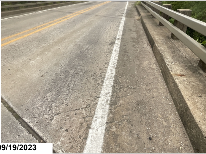
Span 4, right lane-Scaling
