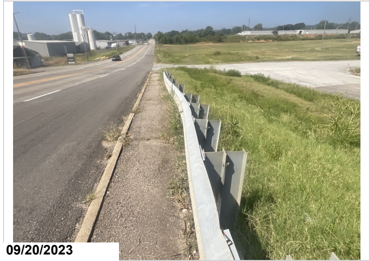
Abutment 1 left approach railing-Collision damage
