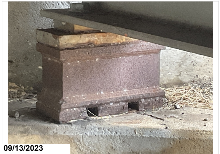
Abutment # 2 bearing # 7 corrosion.
