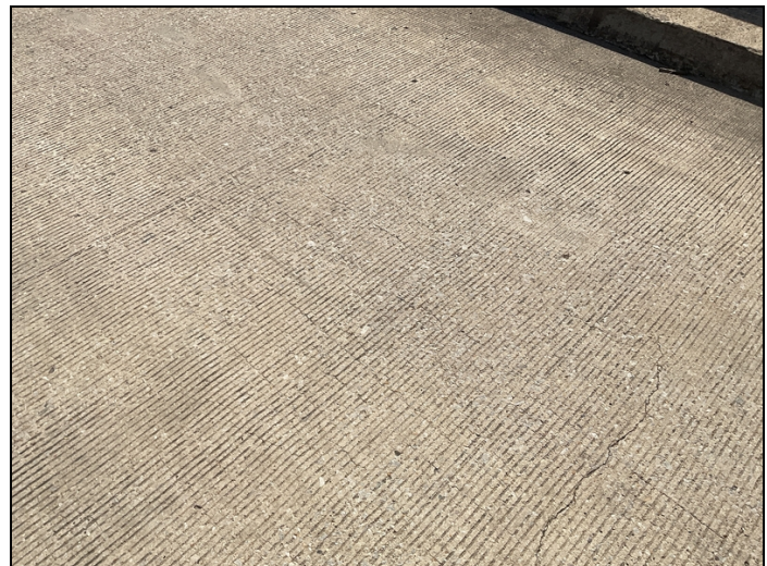
Span 5, right outside lane-Mapcracking in wheel path
