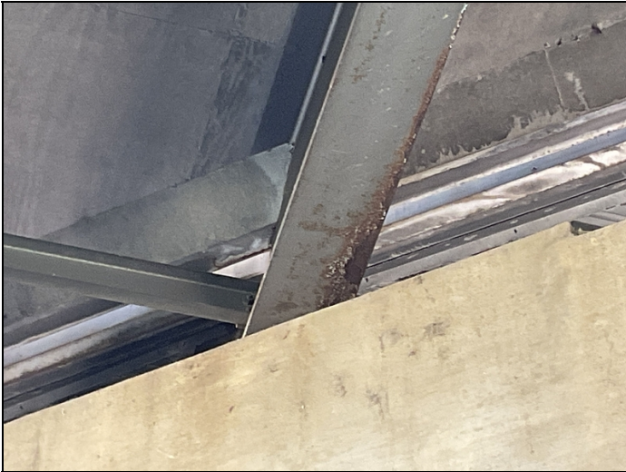
Bent # 4 beam # 4 corrosion
