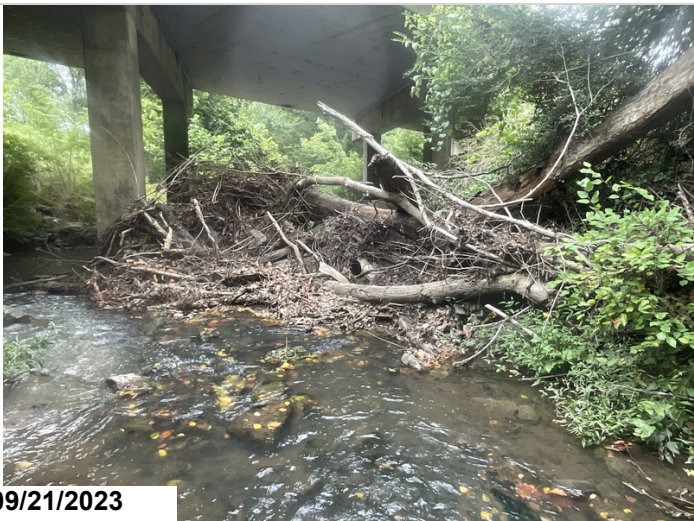
Heavy drift accumulation at bent 2
