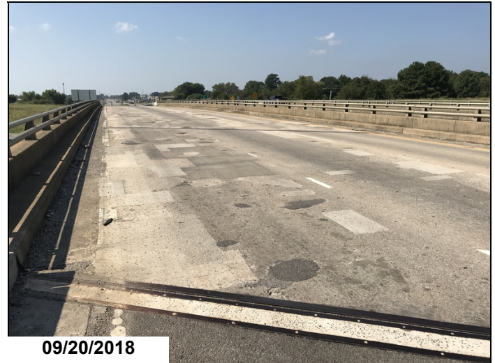
Large areas of scale, concrete deterioration, delaminated concrete, and spalls with exposed reinforcing steel on the driving surface of the deck and in isolated areas of the undersurface. Numerous previous repairs are deteriorating and delaminated.
