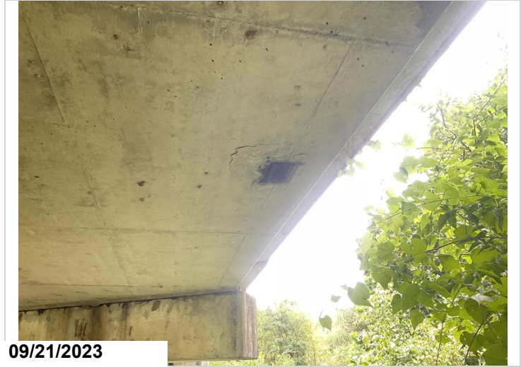
Span 2 undersurface on right side-Delaminated area adjacent to deck drain
