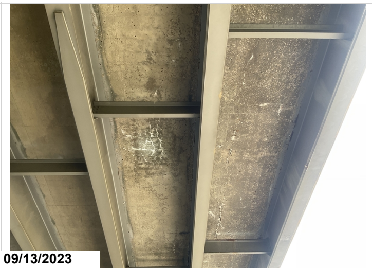
Span # 4 deck undersurface in bay # 5 has an area approximately 30" x 24" of mapcracking with efflorescence, discoloration with leaching. The affected area is over the Northbound inside lane yellow line.
