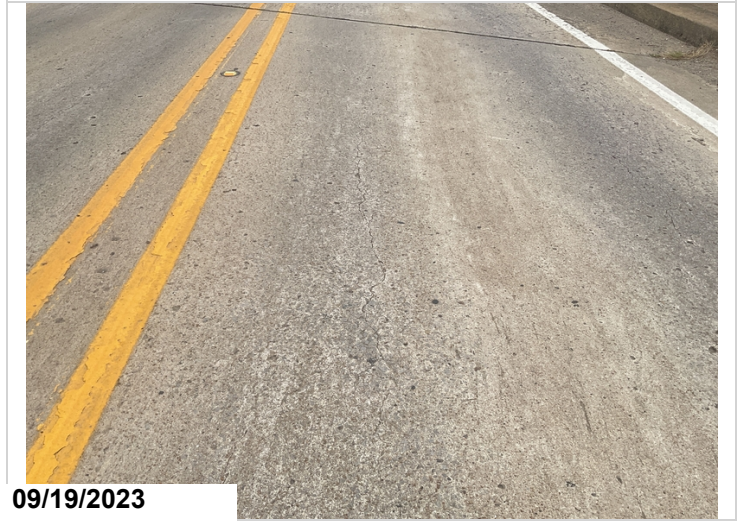
Span # 3 driving surface of right lane has diagonal cracks adjacent to bent # 3 and a longitudinal crack near the centerline.
