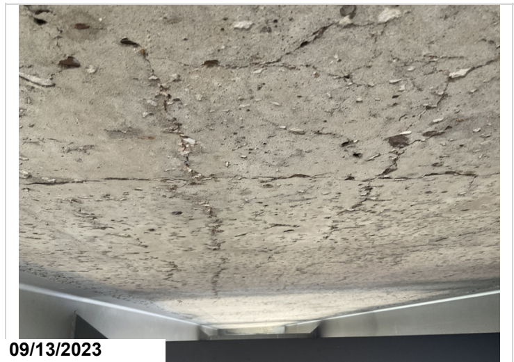
Span # 5 deck undersurface-Scaling and cracking
