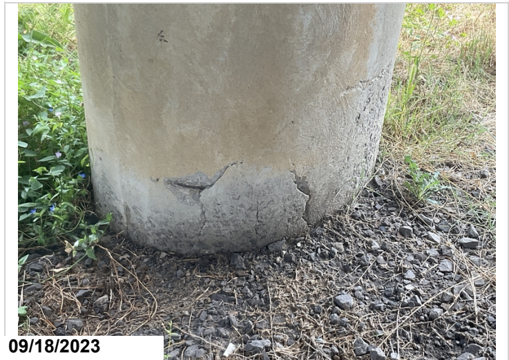
Bent # 3 Column # 3 has a 14" delaminated area / spall with exposed reinforcing steel at the base.
