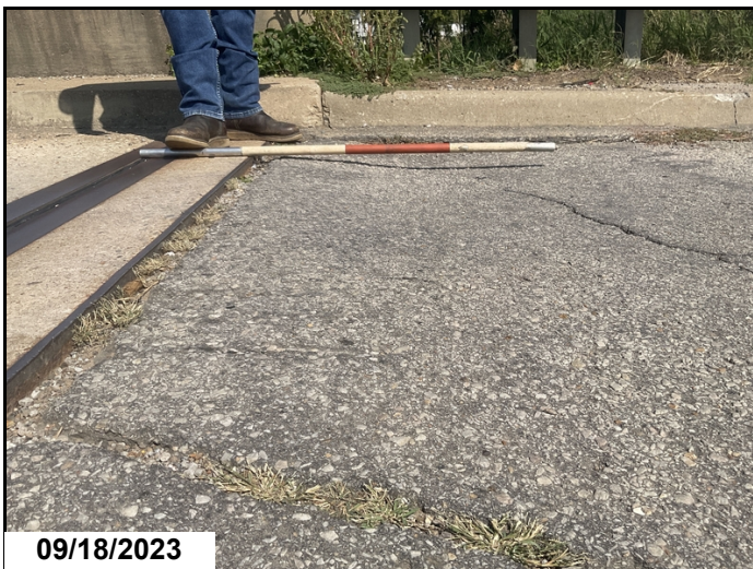
East approach Roadway-Settlement at bridge end.
