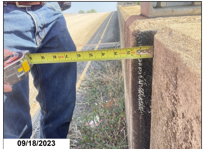
Abutment # 1 right retaining wall -Leaning away from roadway.
