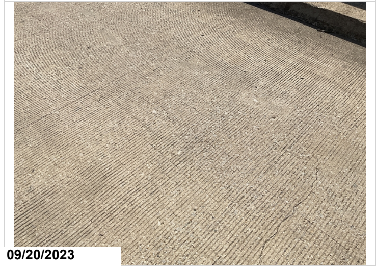
Span 5, right outside lane-Mapcracking in wheel path
