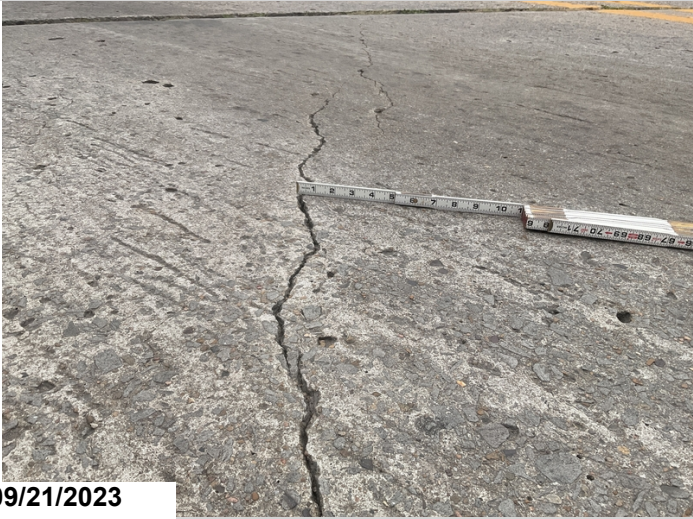
Span # 5, left lane at abutment # 2 has wide diagonal cracking.
