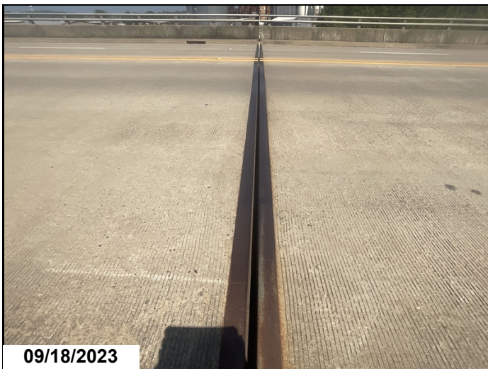
Bent # 6 expansion joint seal has fallen out of the assembly.
