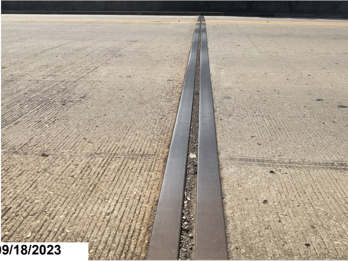
Dirt and debris in expansion joint
