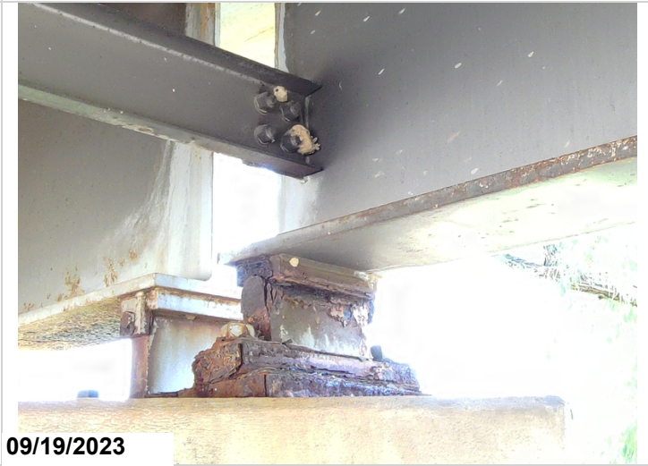
Drone Photo-Heavy corrosion
