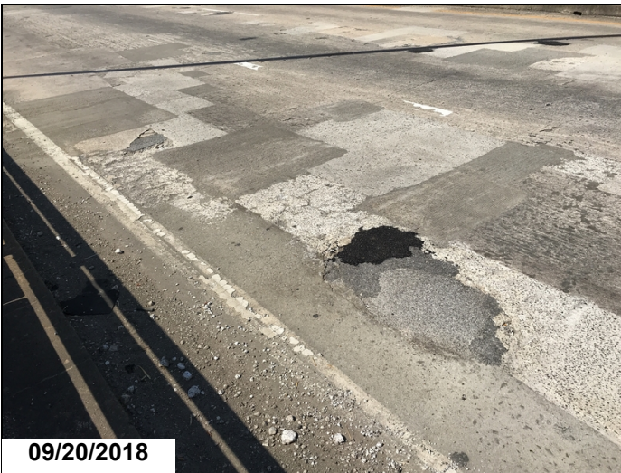
Deterioration of the older repairs.
