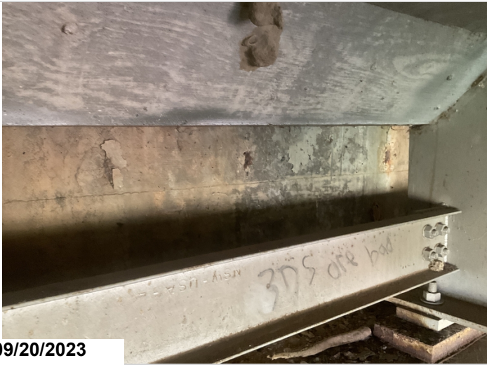
Abutment # 2, East abutment, has several delaminated areas and baseball sized spalls with exposed reinforcing steel.
