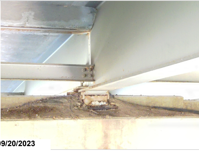
Drone Photo-Heavy dirt and debris accumulation on bent cap
