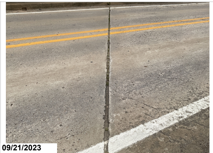
Bent 4 expansion joint
