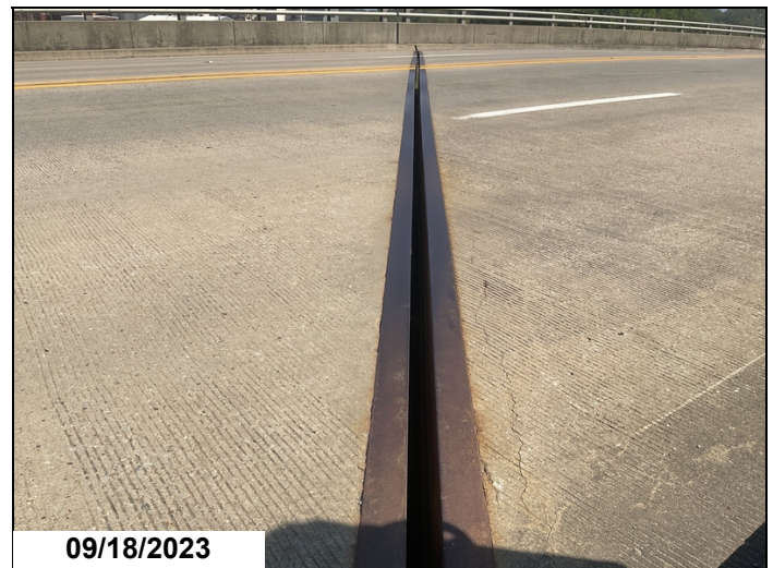
Bent # 4 expansion joint seal has fallen out of the assembly.
