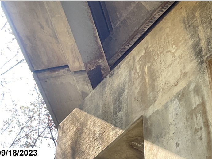
Bent # 5 beam # 7 corrosion
