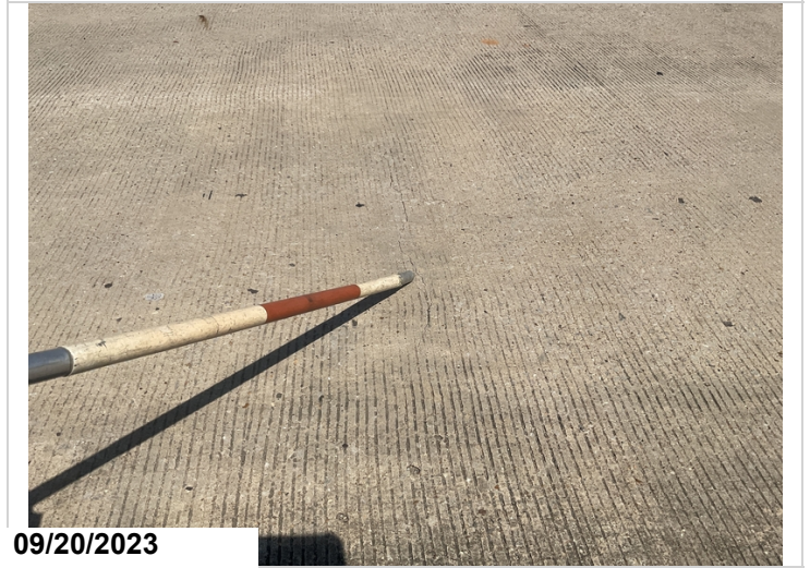
Transverse deck cracking
