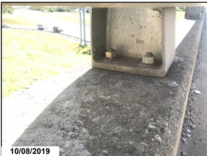
Numerous loose anchor bolt nuts.
