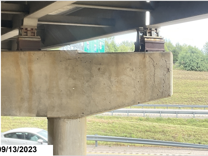
Bent # 2, Right side of cap has horizontal cracks and areas of map cracking, delaminated areas, and spalls with exposed reinforcing steel.
