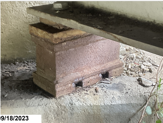
Abutment # 1 bearing # 1 corrosion
