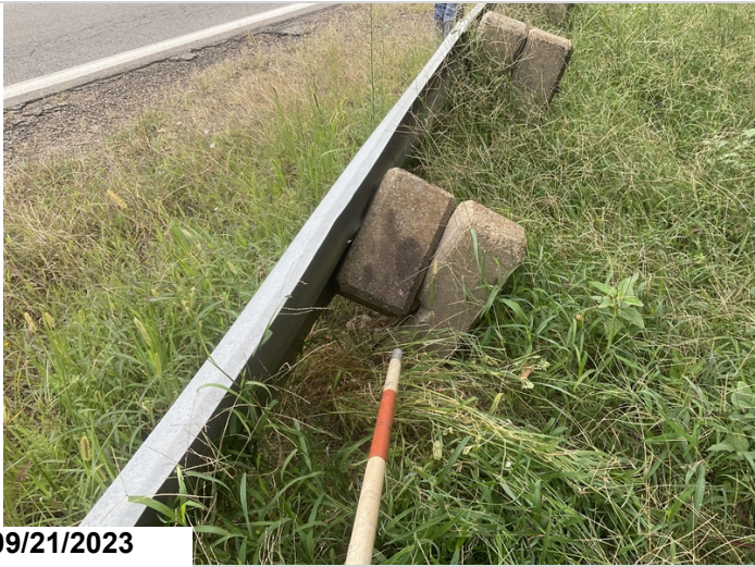
Abutment 1 right approach railing-Collision damage
