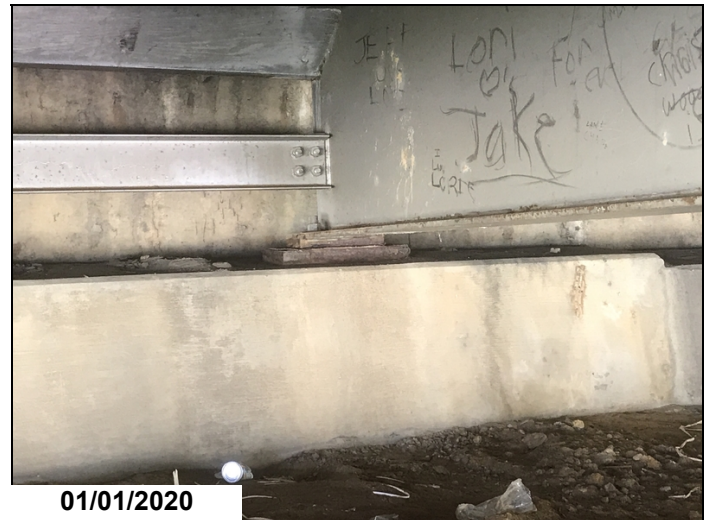
Bent # 9 bearings with active corrosion and layers of flaking rust on the bearings.
