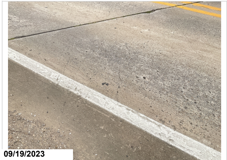
Span 3, right lane-diagonal cracks adjacent to bent 3
