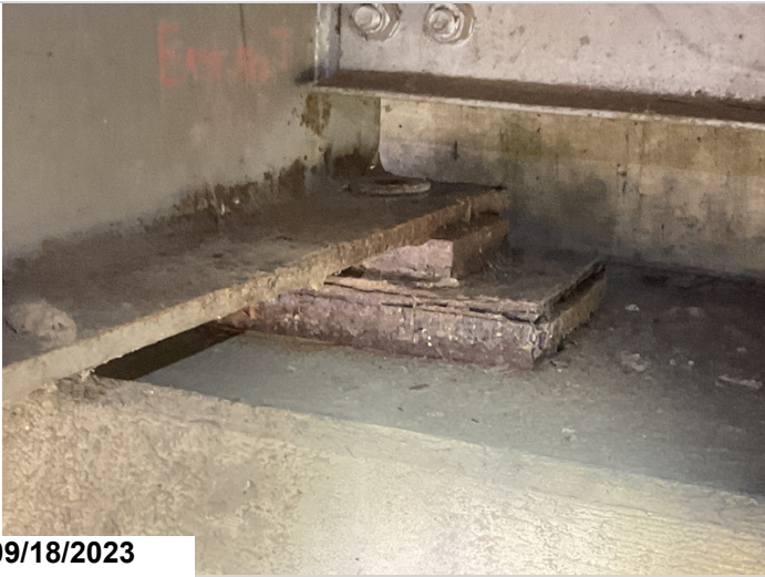
Abutment # 2, Beam # 5, has 1 fractured anchor bolt.
