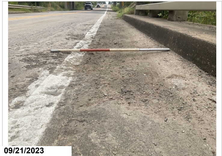
Span # 5, right shoulder has heavy scaling up to approximately 2" deep
