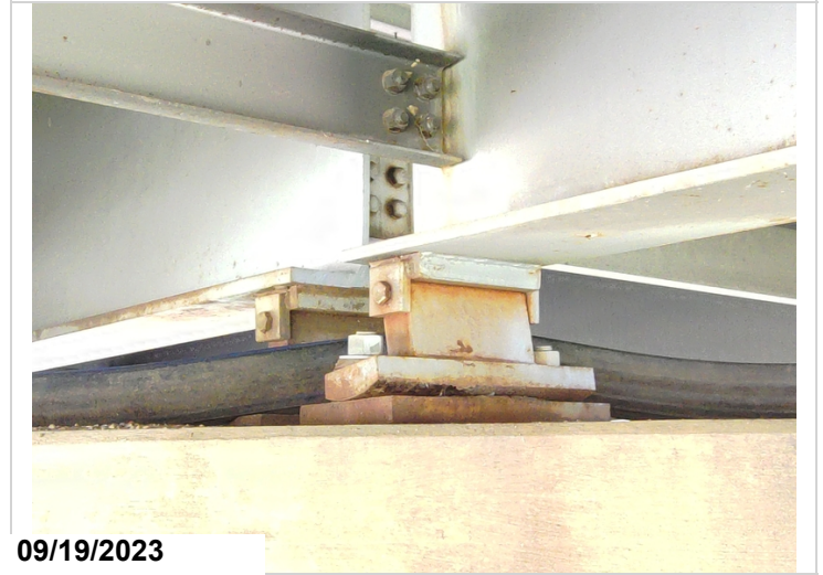
Drone Photo-General view of moveable bearing
