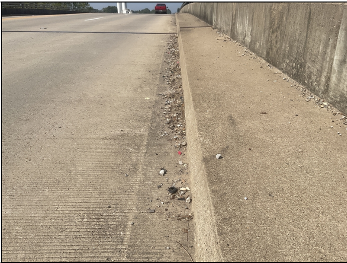
09/18/2023 - RSM & SPC: The gutters have dirt and debris accumulation.
