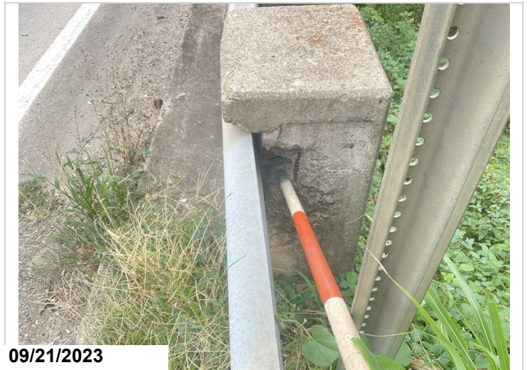
Abutment 1 right end post-Collision damage
