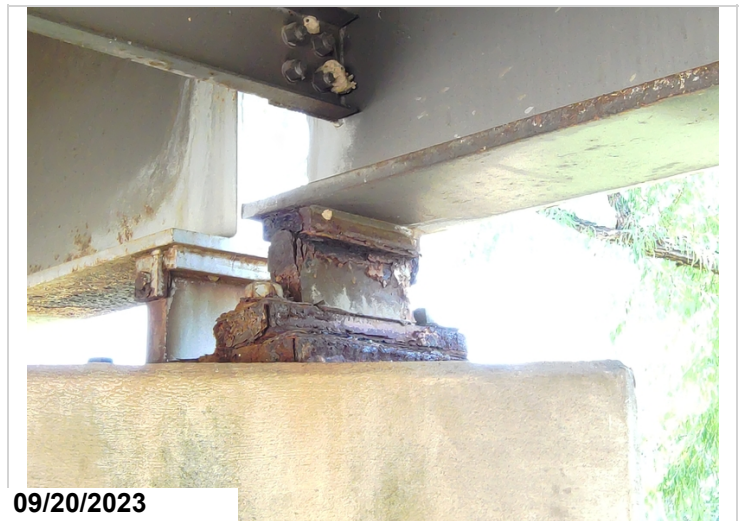
Drone Photo-Heavy corrosion
