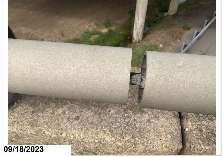
Span 4 left railing-Telescoping connector displaced
