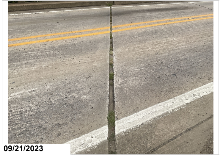
Abutment 2 expansion joint-Debris impaction
