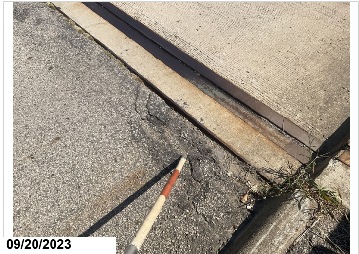
West approach roadway-Settlement with pothole forming in right outside lane
