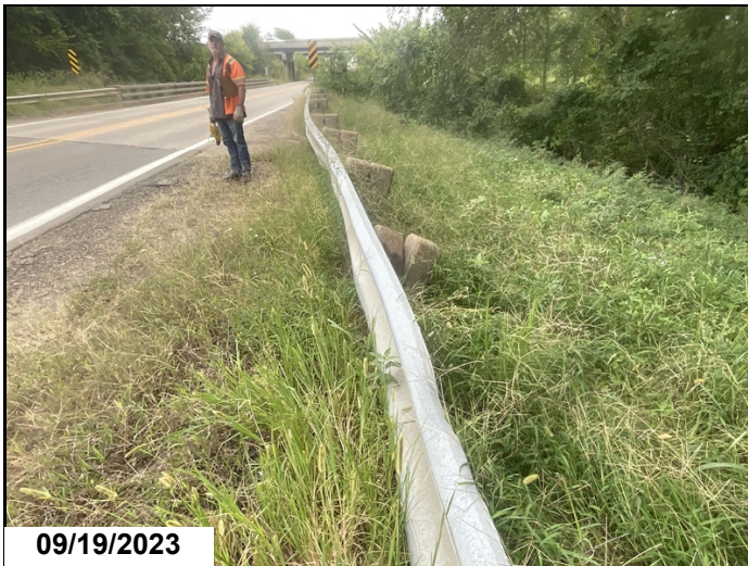
Abutment # 1 right approach railing-Collision damage.
