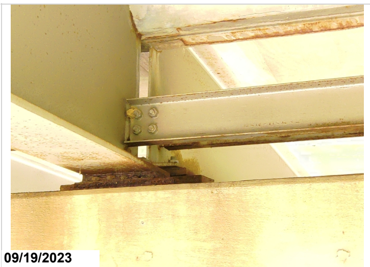
Drone Photo-Corrosion to bearing
