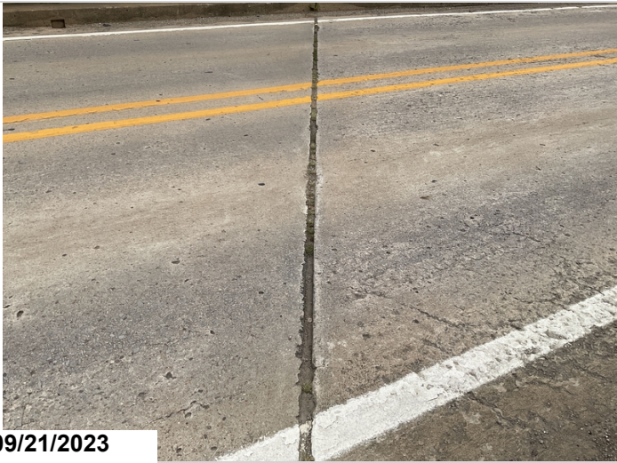
Bent 4 expansion joint
