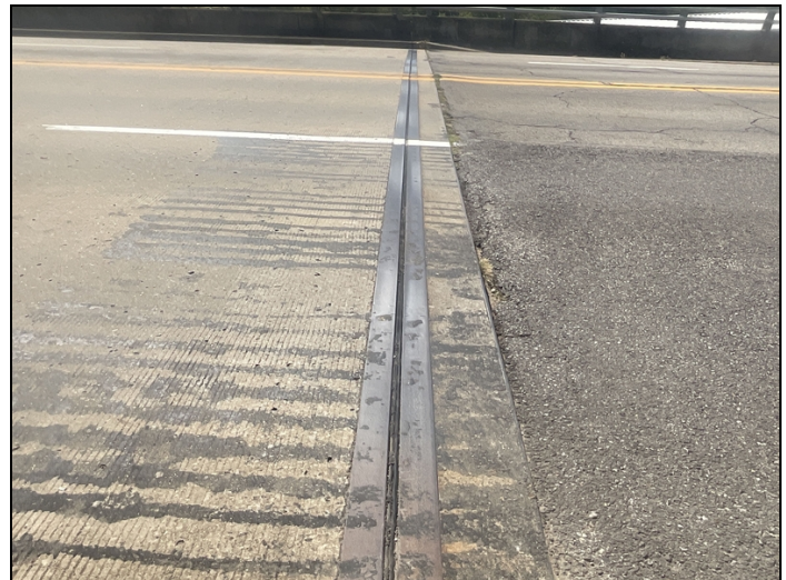
Abutment # 1 expansion joint seal deteriorated.
