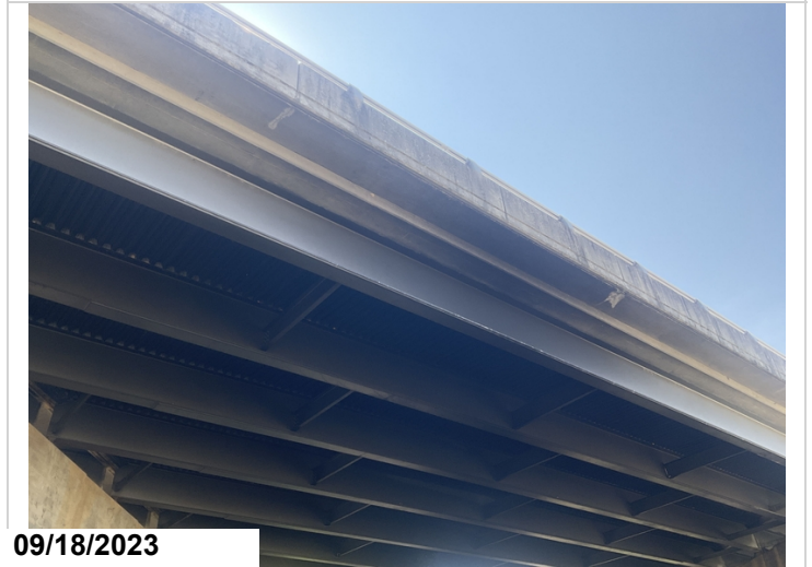
Span # 4 left overhang efflorescence
