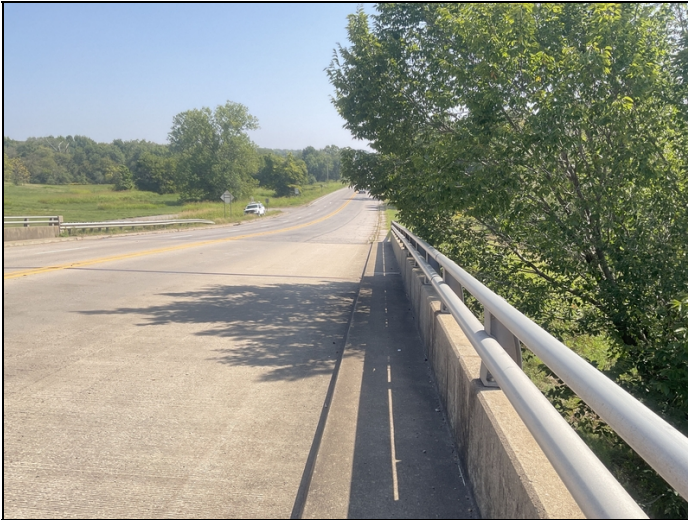
Vegetation is growing over right bridge railing and into driving lane at East bridge end.
