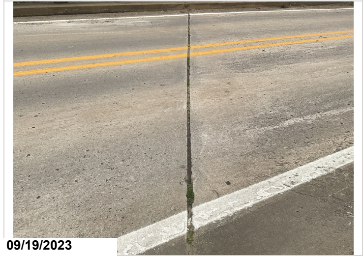
Bent 2 expansion joint-Debris impaction
