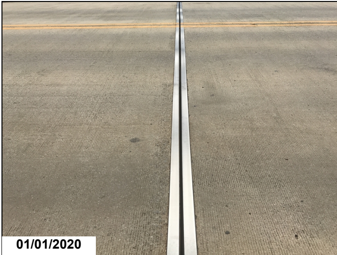
Bent # 6-Joint seal has fallen out of the assembly.
