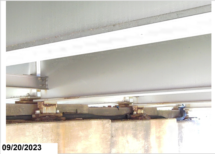
Drone Photo-Corrosion to bearings
