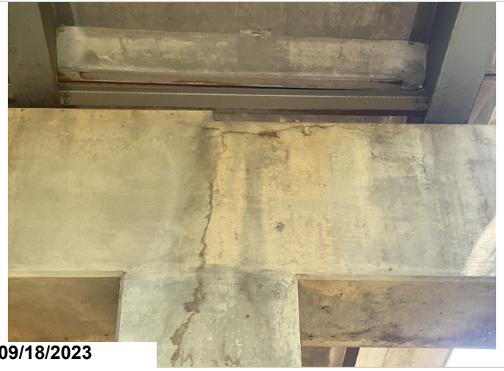
Bent # 8 has a 3' horizontal crack at the top of the cap between beams # 6 & 7.
