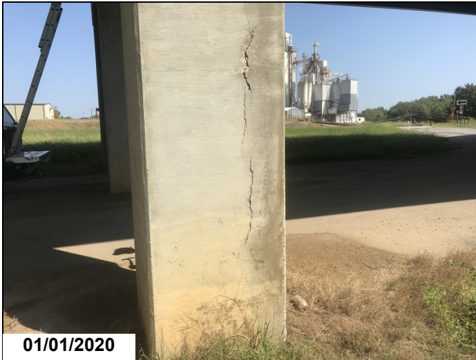
Bent # 3, column # 3-Delaminated area.
