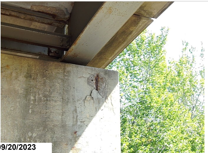
Drone Photo-Spall in bent cap with exposed reinforcing steel.
