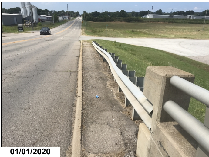
Abutment # 1 left approach railing-Collision damage.
