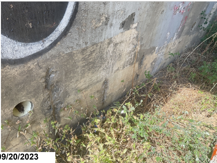
Abutment # 1 stem with 3 spalls that expose reinforcing steel in the base of the bent under bay # 6.
