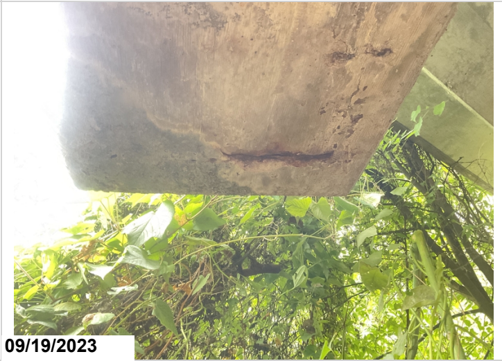
Bent 2 cap undersurface on right side-Spall with exposed reinforcing steel
