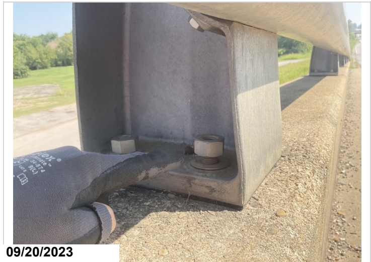
Loose anchor bolt nuts that attach metal railing posts to concrete railing
