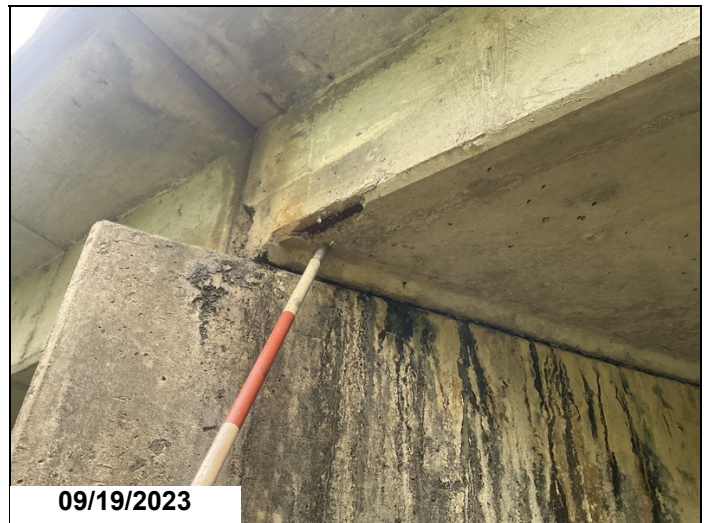
Span # 1 left exterior side adjacent to bent # 2 has an 8" spall with exposed reinforcing steel in bottom edge.
