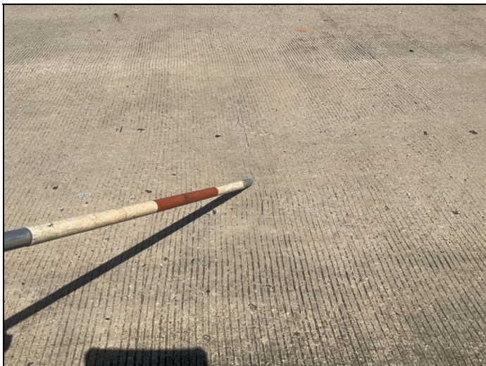
Transverse deck cracking
