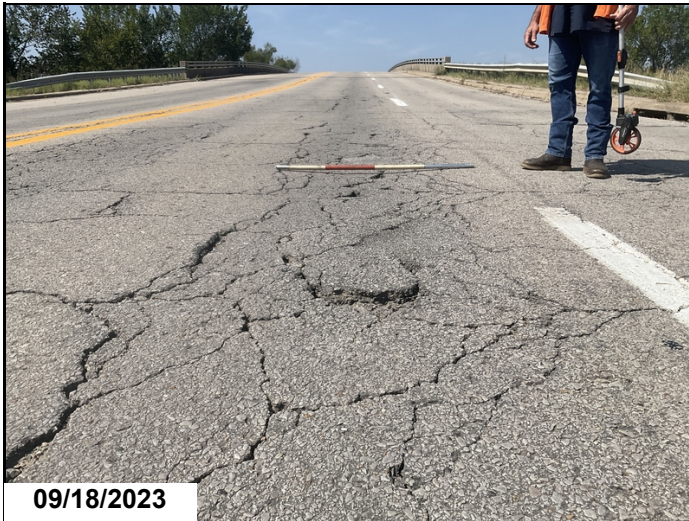
East approach roadway has rutting in the Eastbound lanes with potholes forming.
