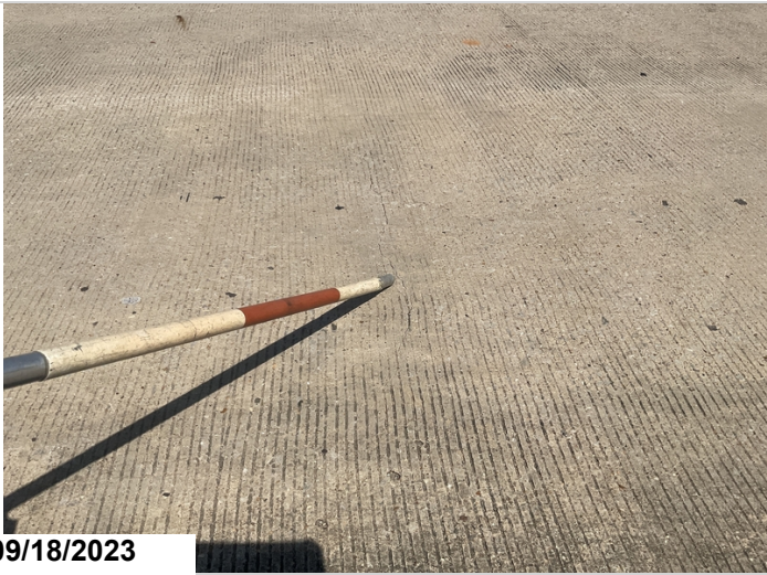
Transverse deck cracking
