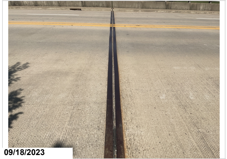
Bent 7 expansion joint
