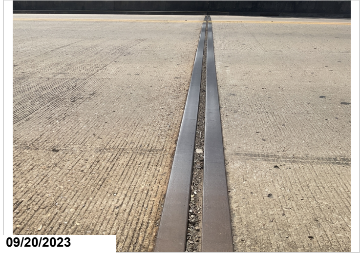
Dirt and debris in expansion joint
