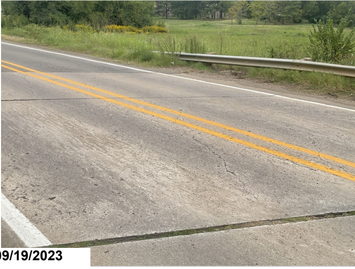
Abutment 1 approach slab-Wide longitudinal cracking
