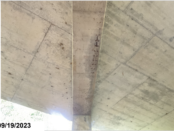
Bent 4 cap undersurface-Spalling/ delaminated areas with exposed reinforcing steel
