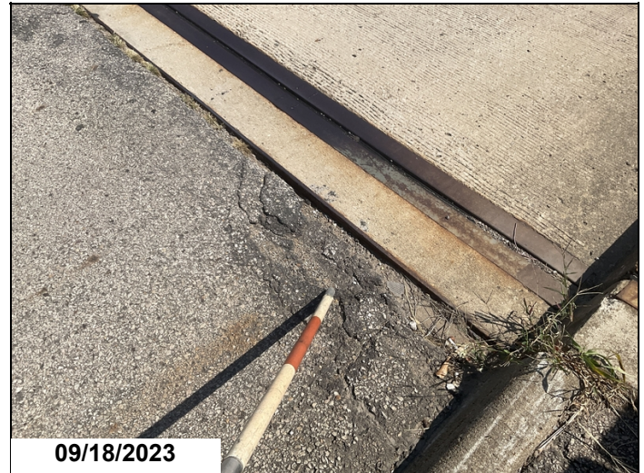
West approach roadway-Settlement with pothole forming in right outside lane.
