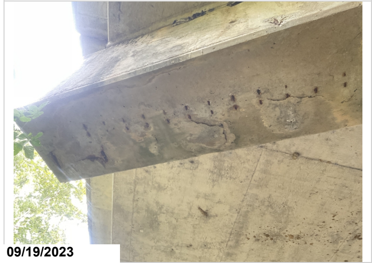
Bent # 3 cap left undersurface-Shallow spalls with exposed reinforcing steel
