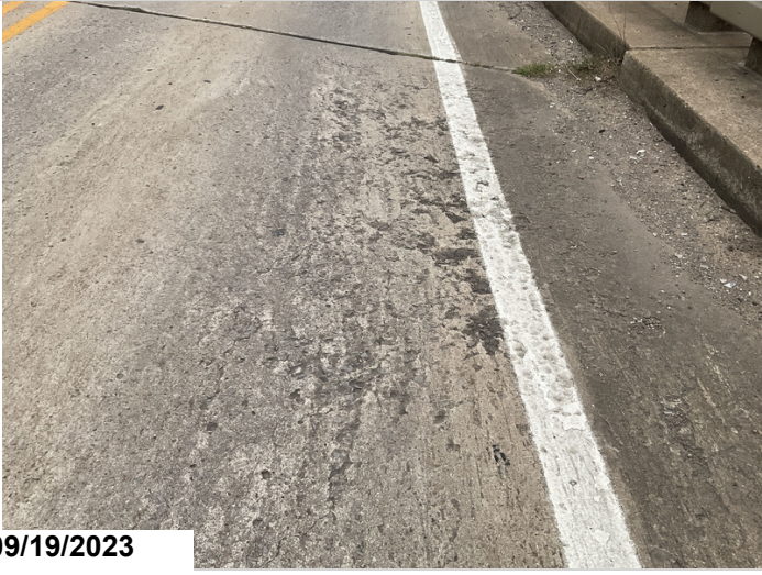
Span 2, right lane-Medium scaling
