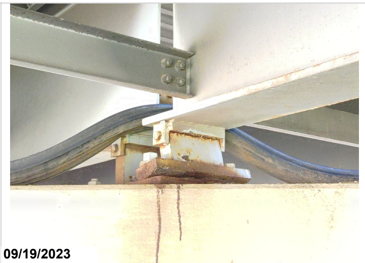
Drone Photo-Corrosion with pack rust between bearing plates.
