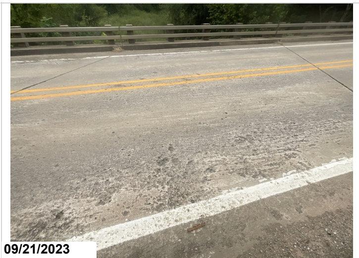
Span 4 driving surface-Scaling
