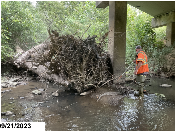
Channel has heavy drift accumulation/ large trees at bent # 2.
