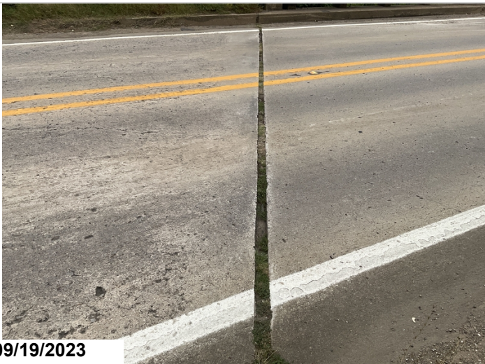
Abutment 1 expansion joint-Debris impaction
