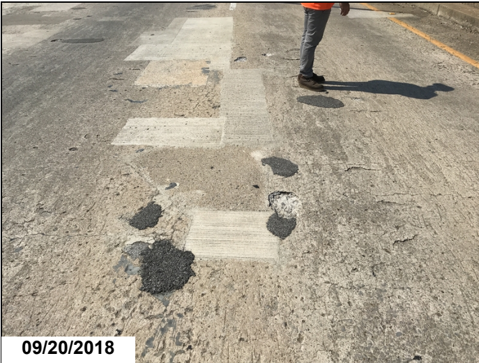
Span # 3 potholes forming on the deck.
