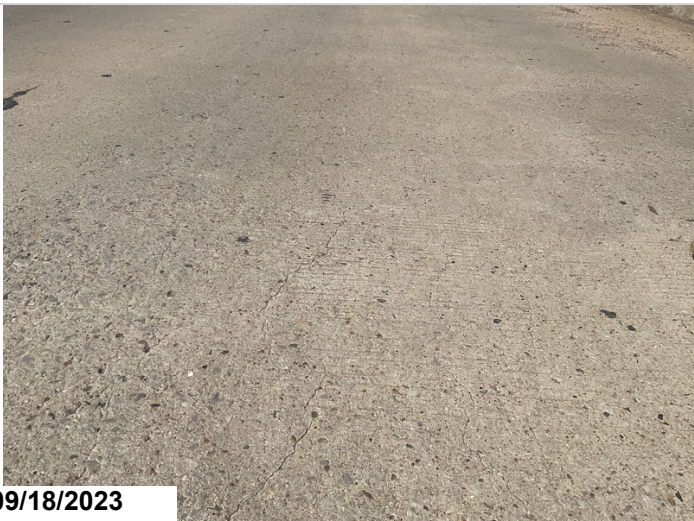
Cracking in wheel path
