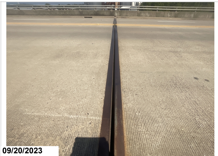
Bent 6 expansion joint seal fallen out of the assembly
