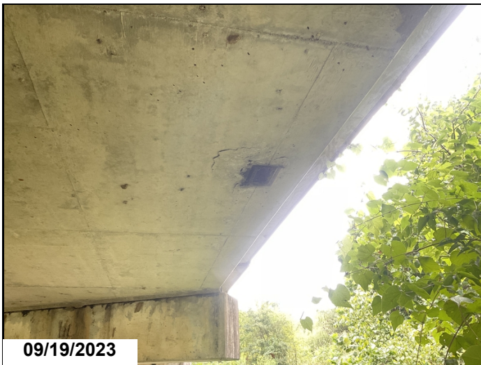
Span # 2 undersurface on right side-Delaminated area adjacent to deck drain.
