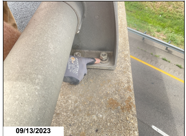
Loose nut on anchor bolt nut that connects railing to concrete bridge railing.
