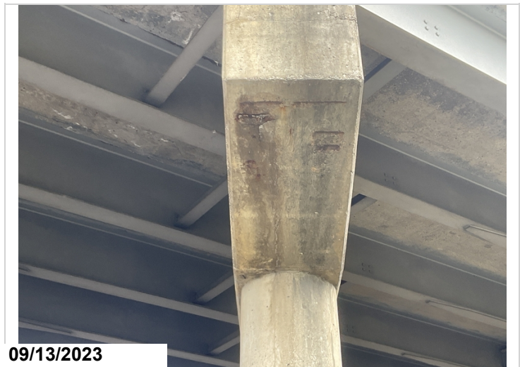
Bent # 5 Right side of cap has a 2' area with concrete spalls with exposed reinforcing steel visible from the undersurface of the cap.
