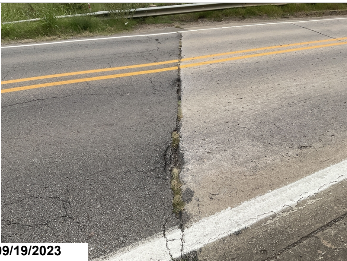
West approach roadway-Potholes forming at bridge end
