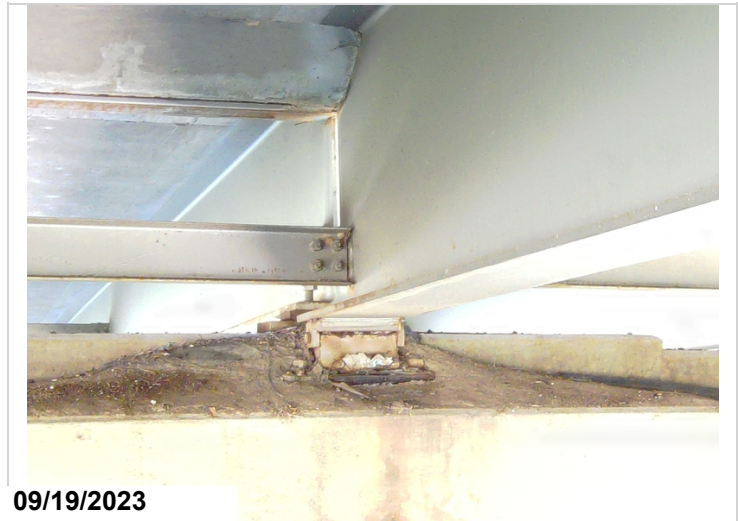
Drone Photo-Heavy dirt and debris accumulation on bent cap
