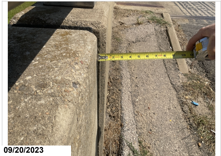
Abutment # 1 left retaining wall-Leaning away from roadway.
