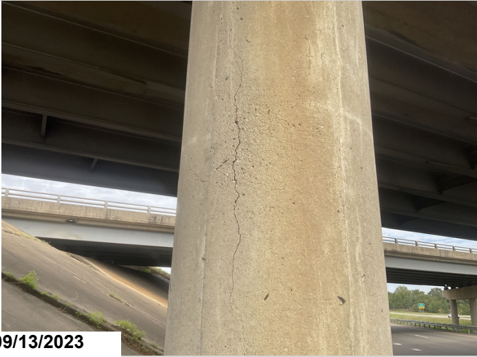
Bent # 2, column # 3 has a CS3 vertical crack 8' from ground level.
