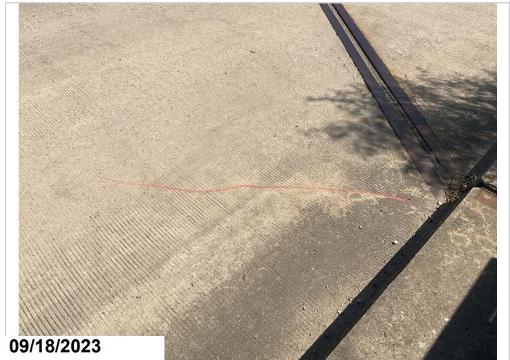
Span 4 has a longitudinal crack (Perpendicular to expansion joints) in right outside lane at bent 5
