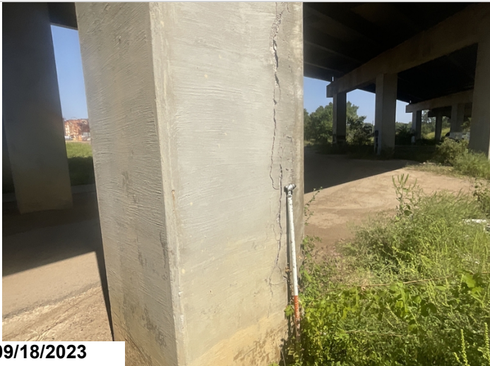
Bent # 3, column # 3 has an 8' high vertical delamination in the base.
