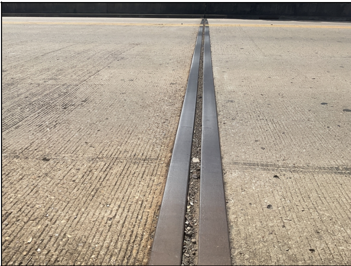
Dirt and debris in expansion joint
