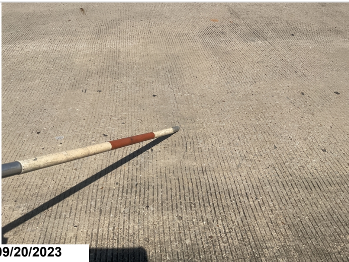
Transverse deck cracking
