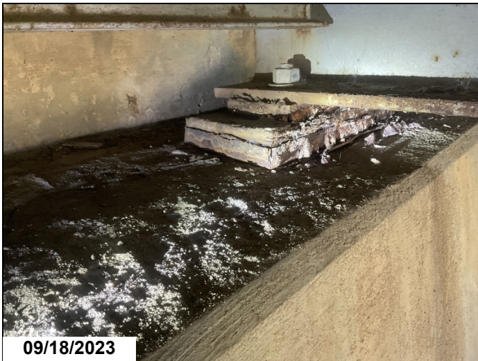
Abutment # 2 bearing # 3-Corrosion.
