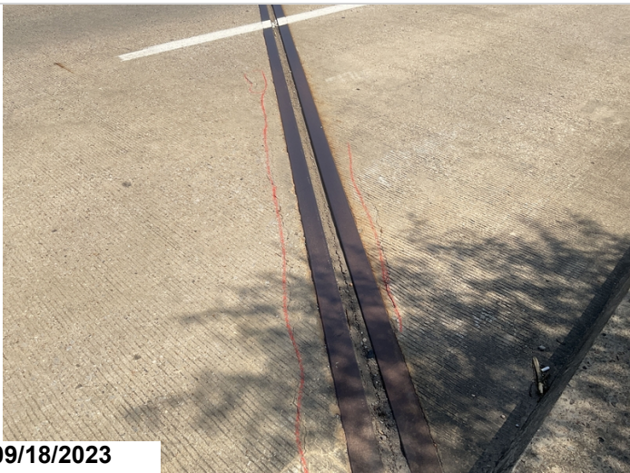
Span 4 right outside lane at bent 5-Transverse cracking with delaminated area adjacent to expansion joint assembly
