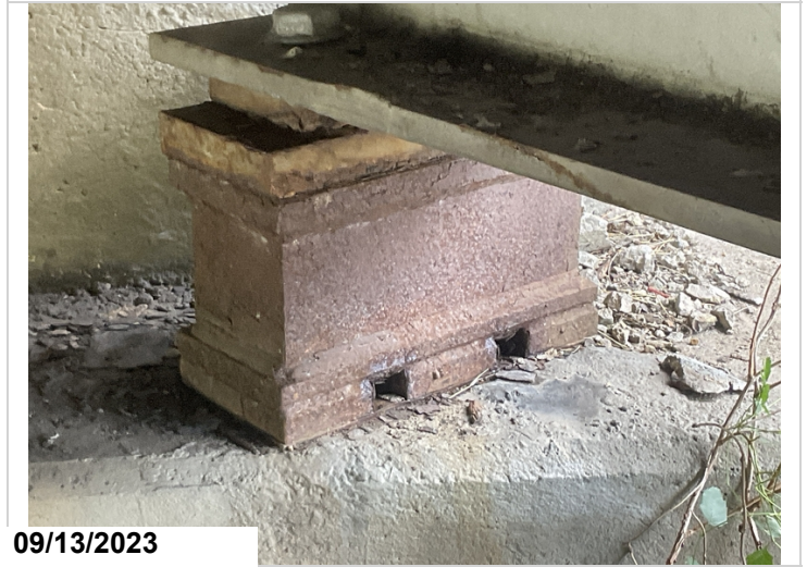
Abutment # 1 bearing # 1 corrosion
