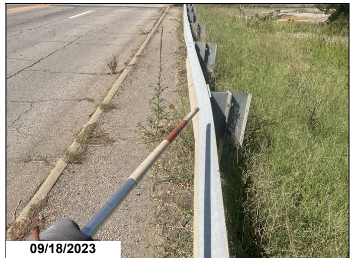
Abutment # 2 left approach railing-Collision damage.
