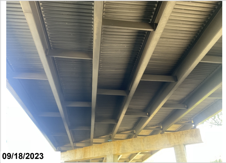
Span # 4 beams have staining from train exhaust.
