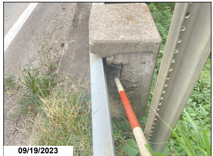
Abutment # 1 right end post-Collision damage.
