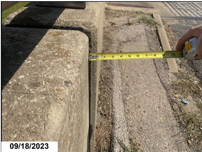
Abutment # 1 left retaining wall-Leaning away from roadway.
