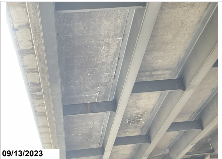
Span # 4 bay # 5-Area of cracking and leaching of efflorescence to the deck undersurface.
