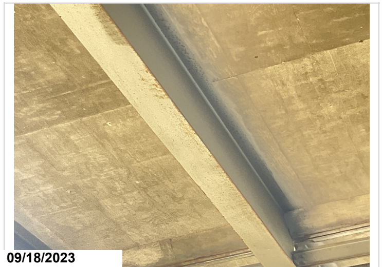
Typical beam corrosion
