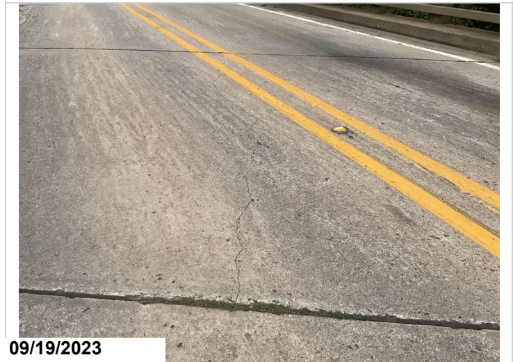
Abutment 2 approach slab-Longitudinal cracking.
