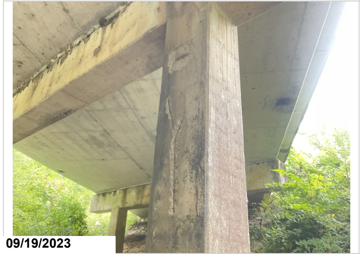
Bent # 4, column # 2-Spalling with exposed reinforcing steel
