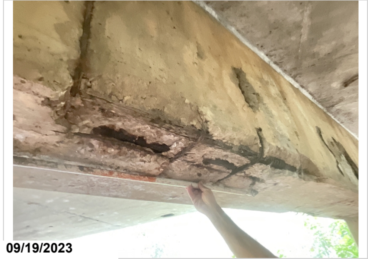
Bent # 5 cap aheadface has numerous The spalls with exposed reinforcing steel and delaminated areas. The cap undersurface near centerline has a spalled area approximately 4' long x 12" wide that exposes several stirrups and two of the primary reinforcing bars. Exposed primary bars have heavy corrosion with thick flaking rust and an estimated 1/8" section loss.
