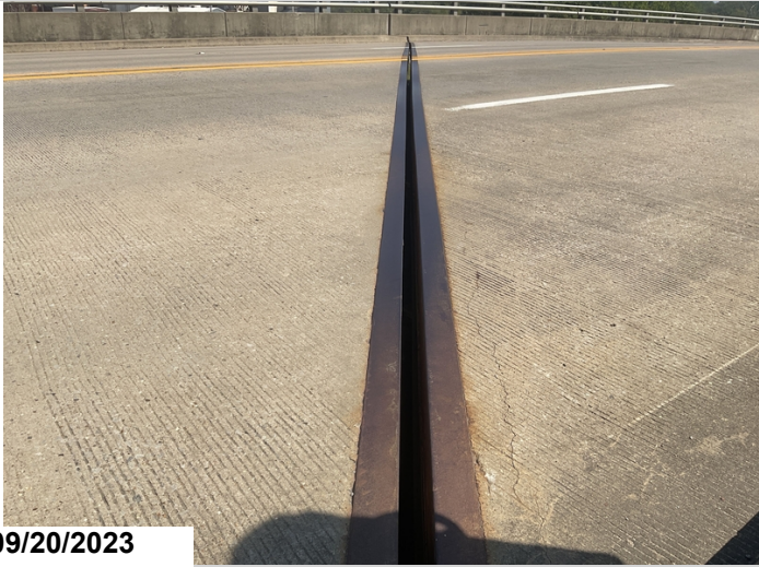
Bent 4 expansion joint seal fallen out of position
