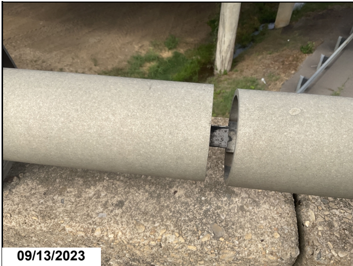
Span # 4 left railing-Telescoping connector vibrated out of position.
