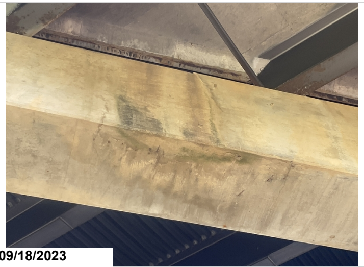
Bent # 5 cap cracking
