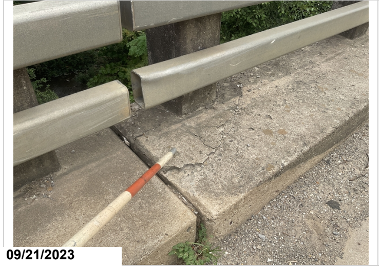
Span 4, post 1-Collision damage
