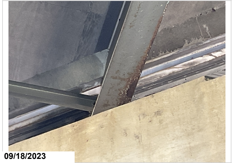
Bent # 4 beam # 4 corrosion
