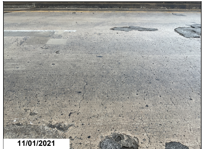
Sealable deck cracking.
