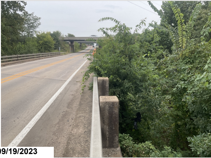
Vegetation growing over right bridge railing.
