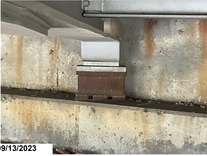
Abutment # 2 typical bearing
