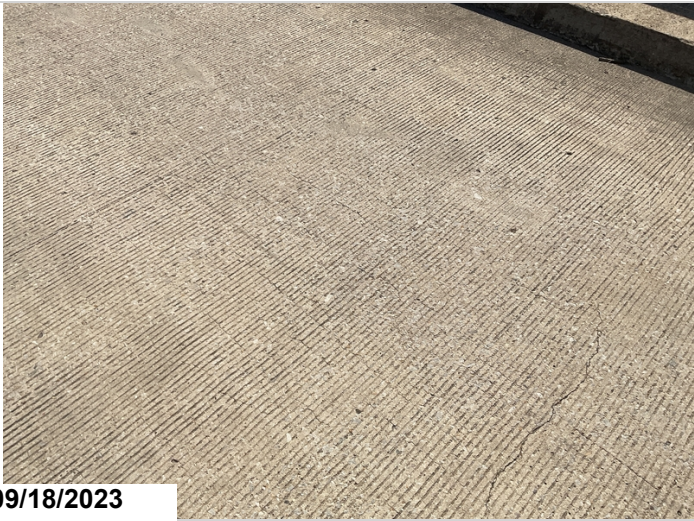
Span 5, right outside lane-Mapcracking in wheel path
