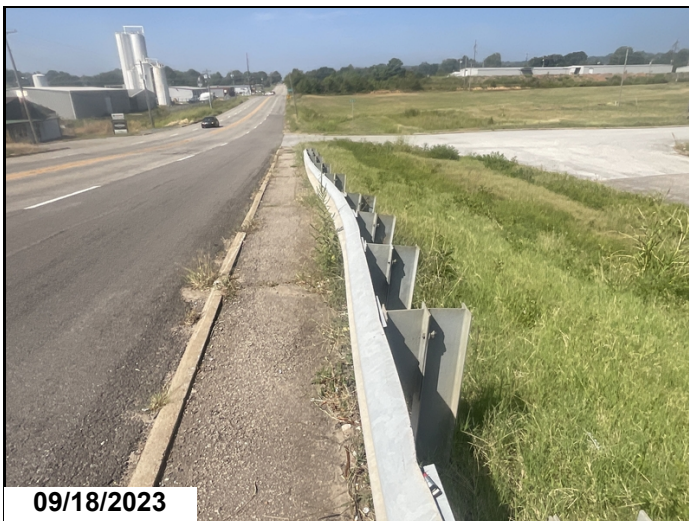
Abutment # 1 left approach railing-Collision damage.
