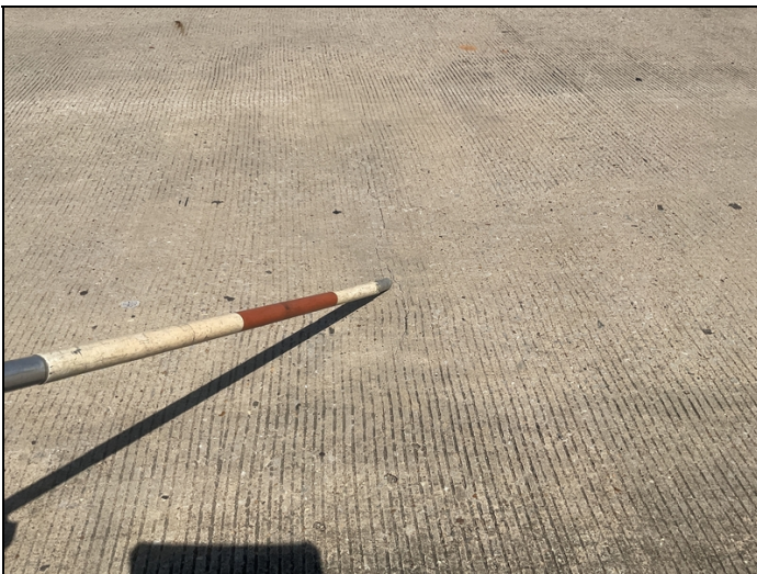
Transverse deck cracking
