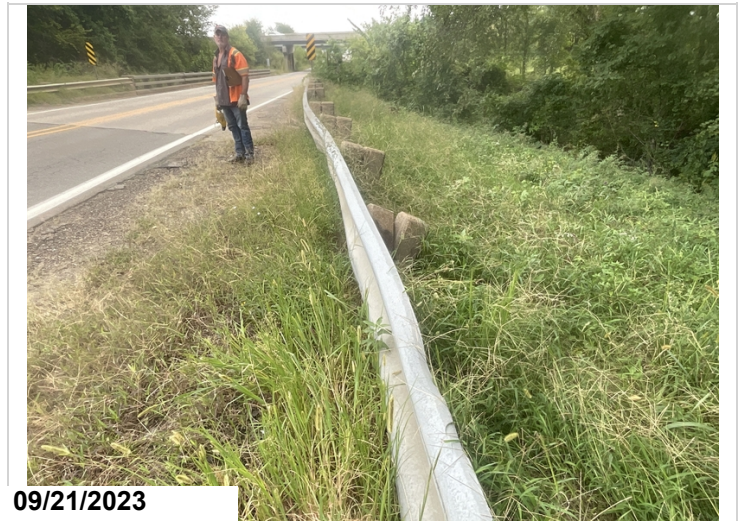
Abutment 1 right approach railing-Collision damage
