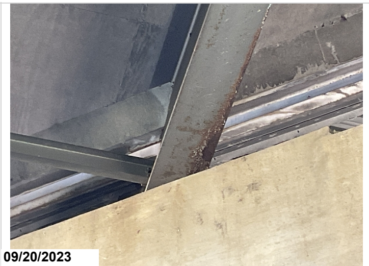
Bent # 4 beam # 4 corrosion
