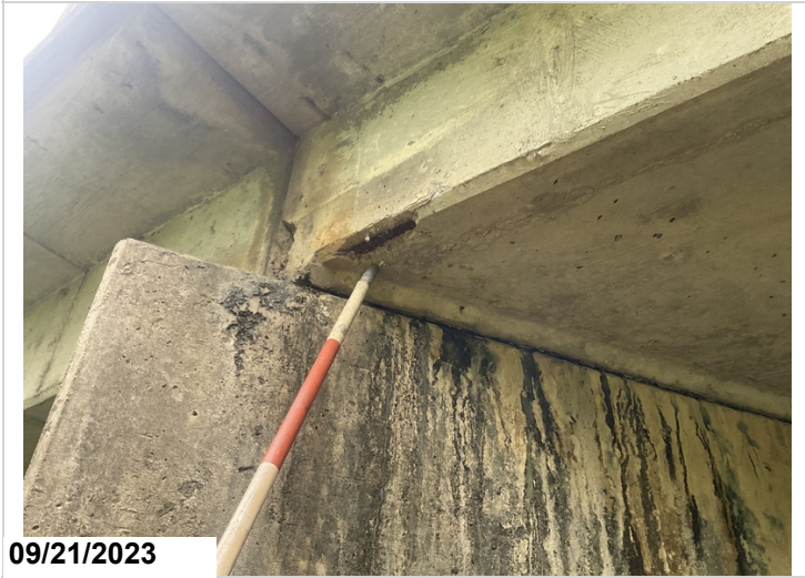
Span # 1 left exterior side adjacent to bent # 2 has an 8" spall with exposed reinforcing steel in bottom edge.
