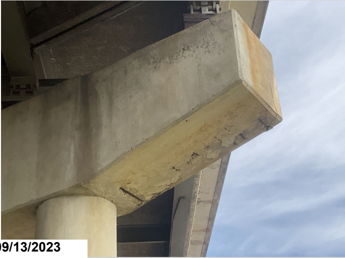
Bent # 4 Right side of cap has a 6' section of spalls with exposed reinforcing steel.
