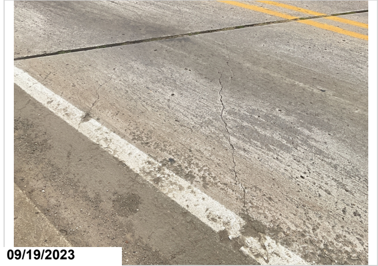
Span # 5, left lane at abutment # 2 has wide diagonal cracking.
