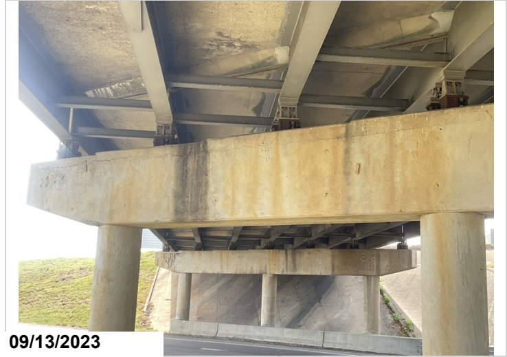
Bent # 3 cap has a horizontal crack that is located approximately 8" below the top of cap for approximately 1/2 the width of the cap.
