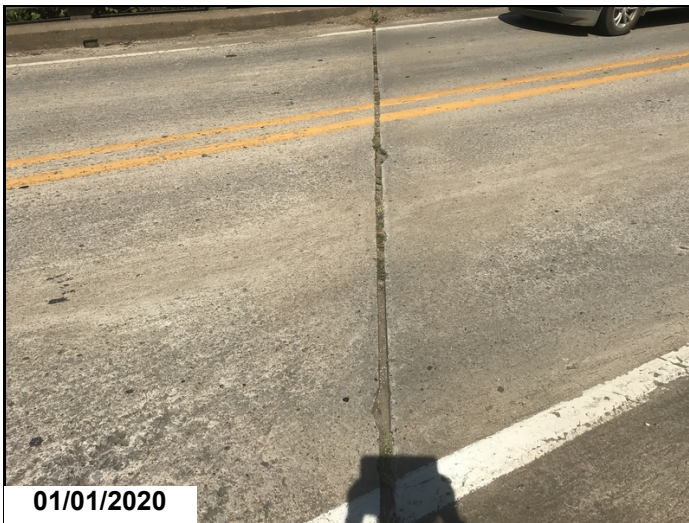
01/01/2020 Deck joint sealant is deteriorated with the joints compacted with incompressible materials.
