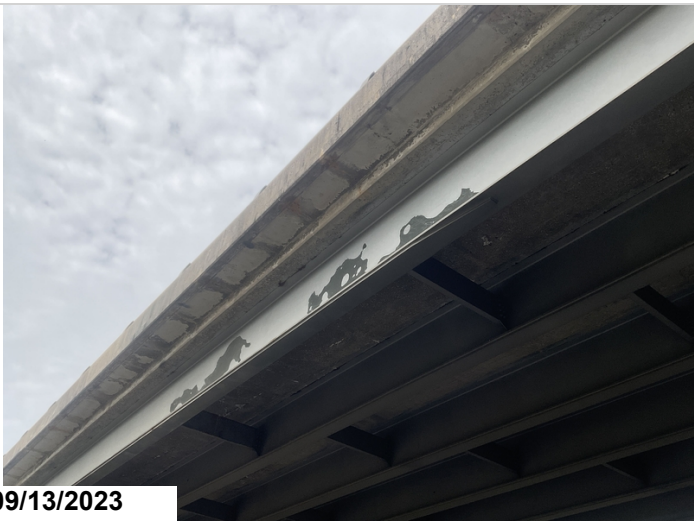
Span # 4 beam # 7 failed paint
