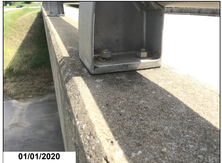
Numerous loose anchor bolt nuts on the bridge rail.
