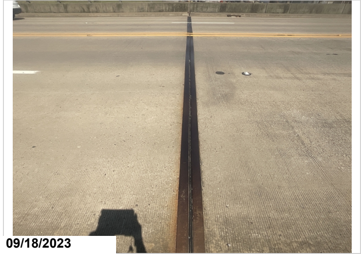
Bent 3 expansion joint
