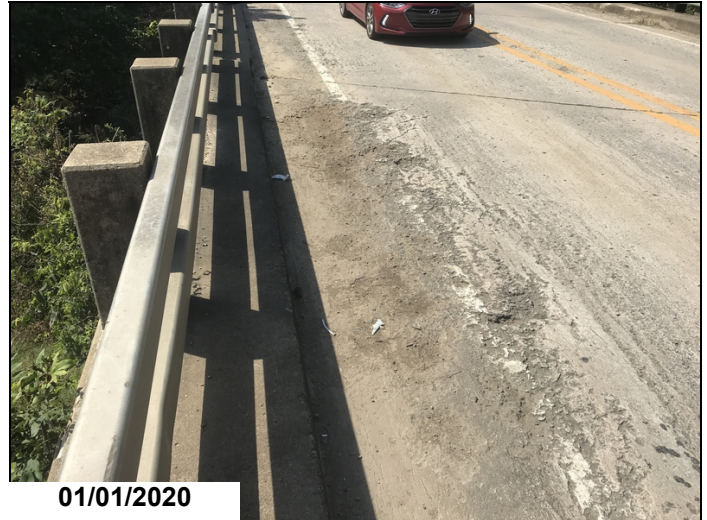
Span # 4 & 5 left concrete deterioration with section loss.
