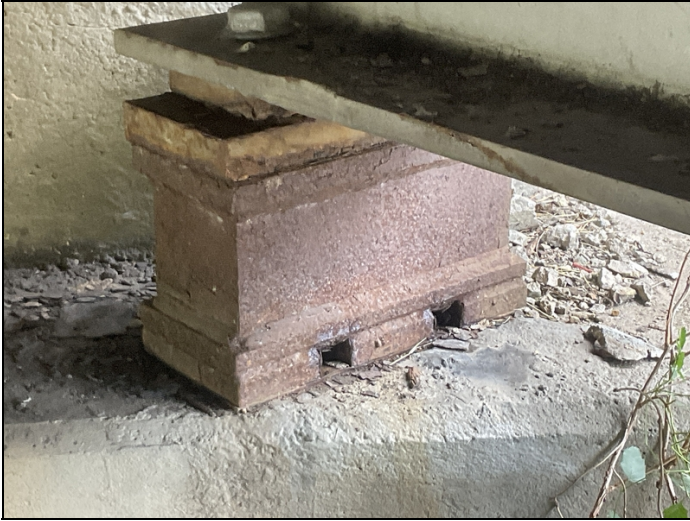
Abutment # 1 bearing # 1 corrosion
