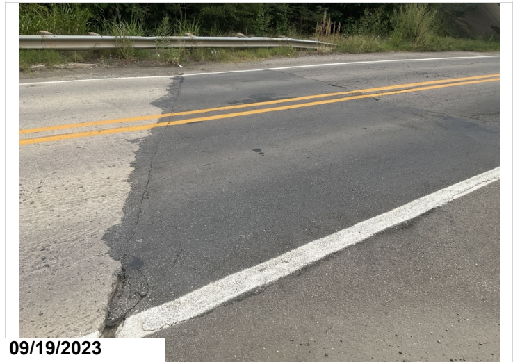
Repairs to East approach roadway
