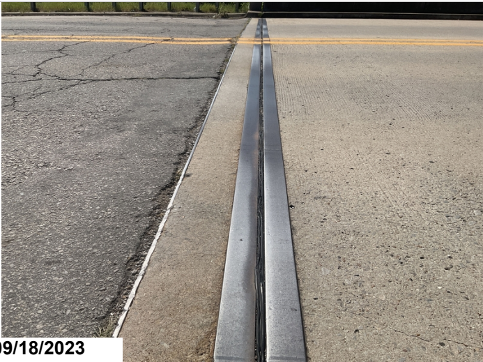
Abutment 2 expansion joint seal
