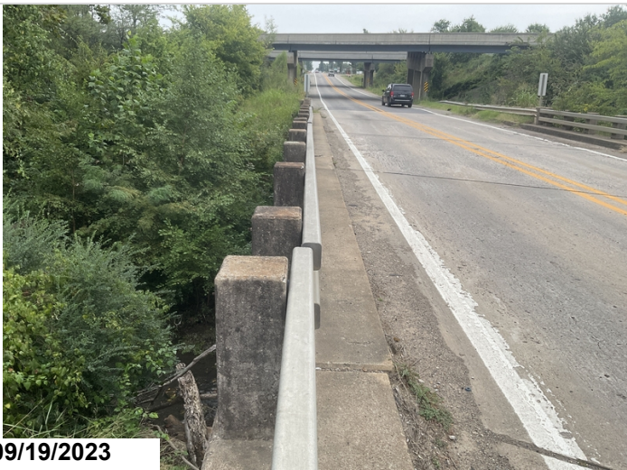
Misalignment of spans
