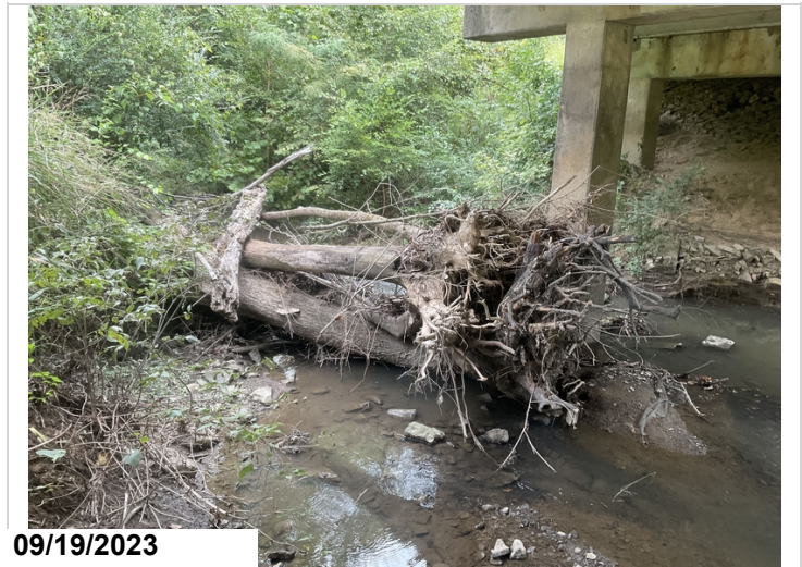
Channel has heavy drift accumulation/ large trees at bent # 2.
