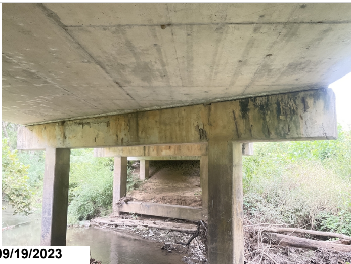
Bent # 4 cap aheadface has numerous spalls with exposed reinforcing steel and delaminated areas.
