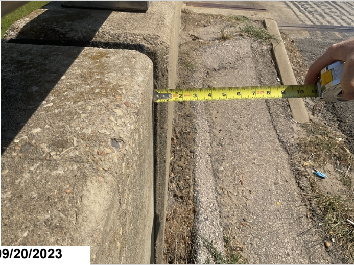
Abutment # 1 left retaining wall-Leaning away from roadway.
