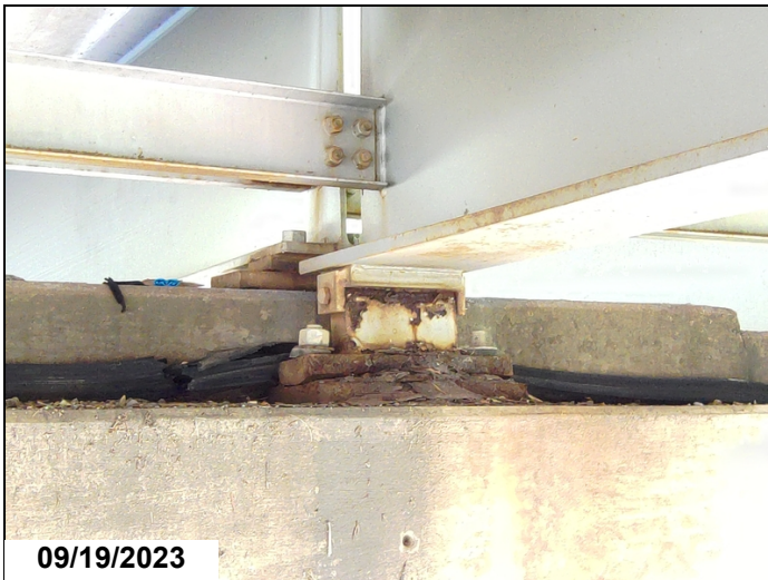
Drone Photo-Heavy corrosion to bearings.
