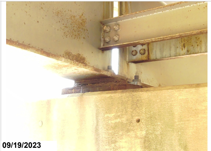
Drone Photo-Bearing corrosion with pack rust between bearing plates.
