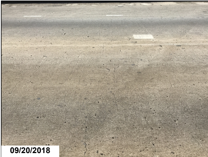
Sealable deck cracking.
