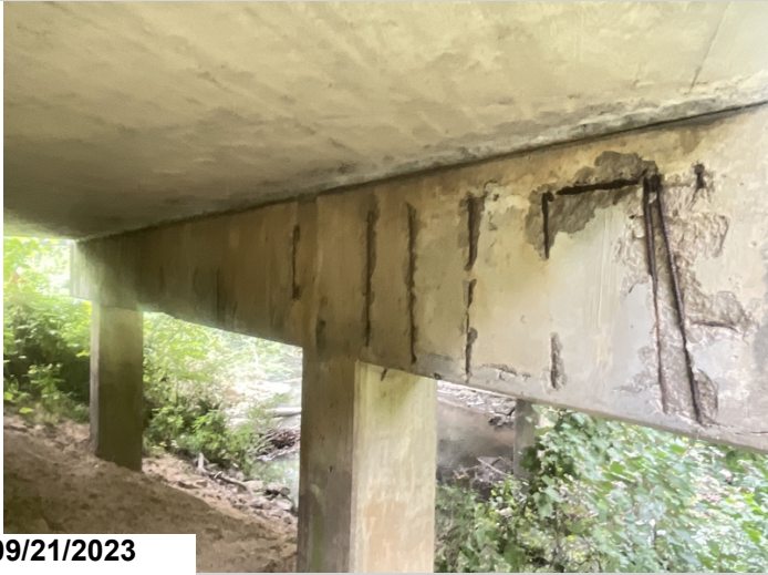
Bent 5 cap aheadface-Numerous spalls with exposed reinforcing steel
