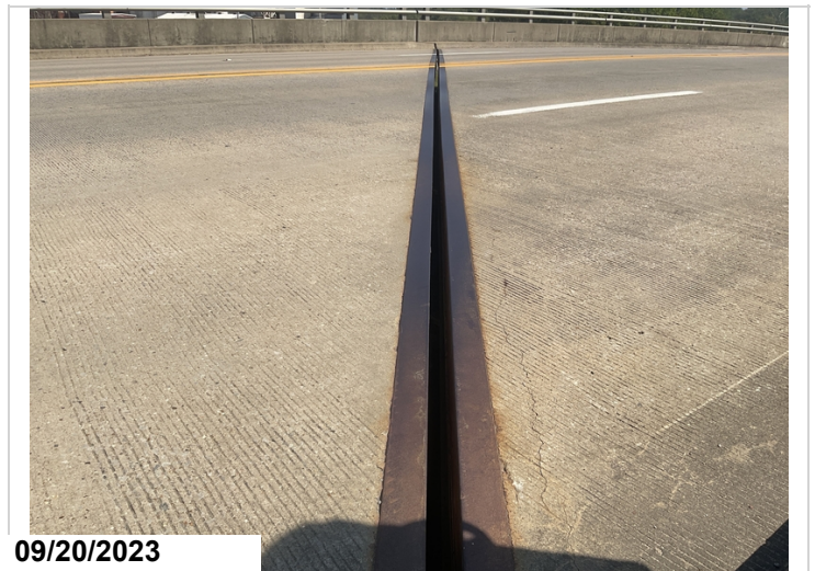
Bent # 4 expansion joint seal has fallen out of the assembly.
