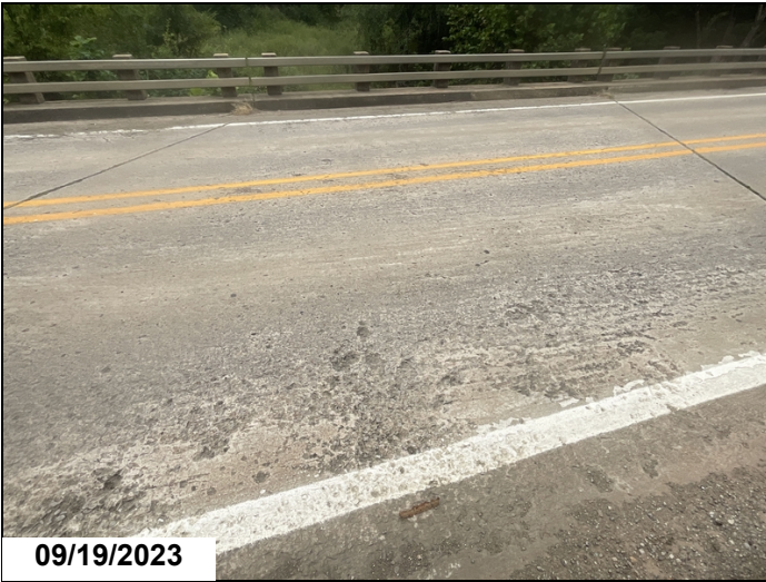
Span #4 driving surface-Scaling.
