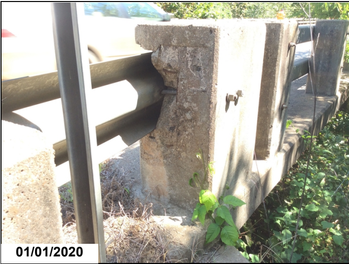
Abutment # 1 right end post-Collision damage.
