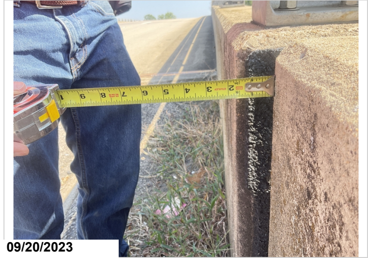
Abutment # 1 right retaining wall -Leaning away from roadway.
