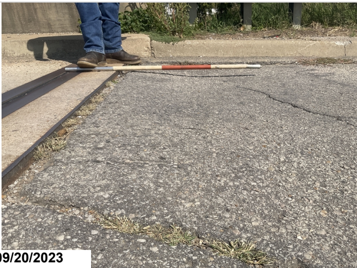
East approach Roadway-Settlement in left lane
