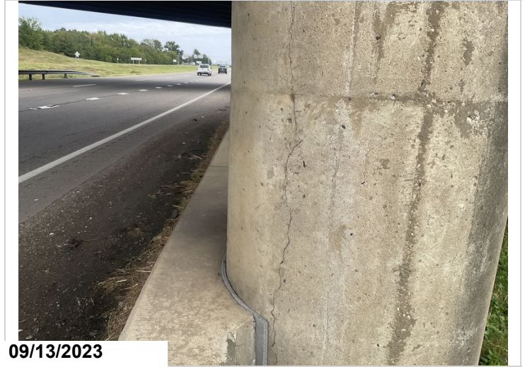
Vertical hairline crack in column at Bent # 5 Column # 3 this inspection.
