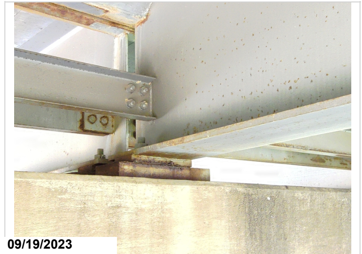
Drone Photo-Bent # 2, corrosion to bearing
