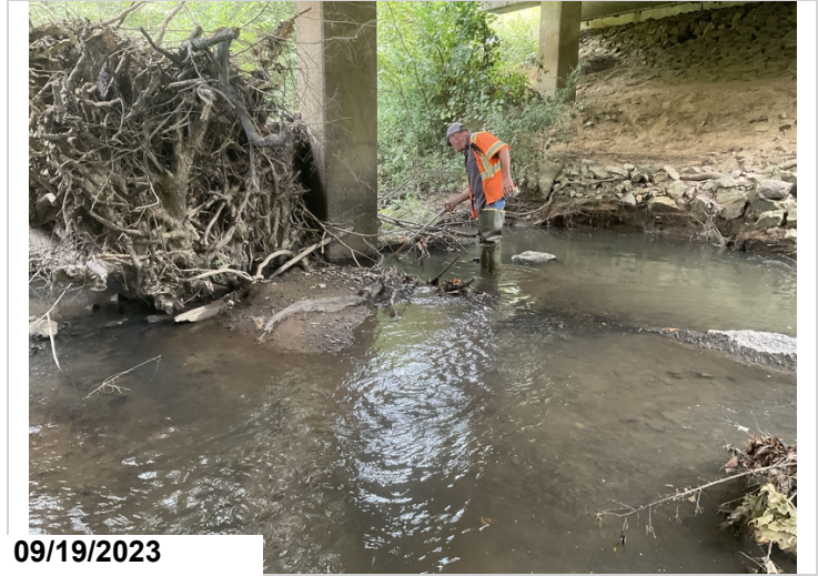
Probing substructure
