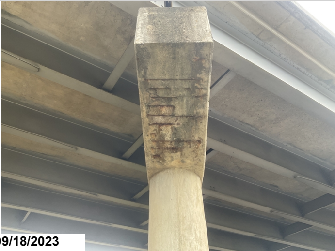
Bent # 5 Left side of cap has a 5' area with concrete spalls with exposed reinforcing steel visible from the undersurface of the cap.
