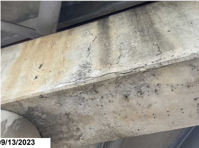
Bent # 2 aheadface has horizontal cracks and areas of map cracking, delaminated areas, and spalling.
