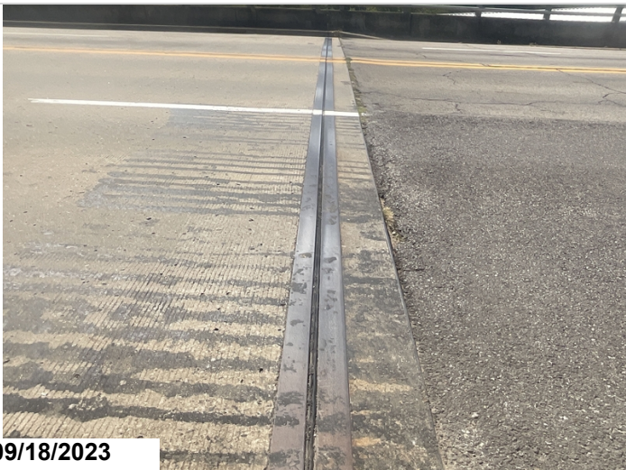
Abutment # 1 expansion joint seal deteriorated.
