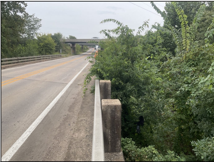
Vegetation growing over right bridge railing.
