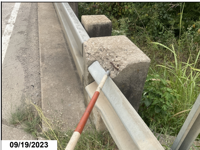
Abutment # 2, left end post-Collision damage.
