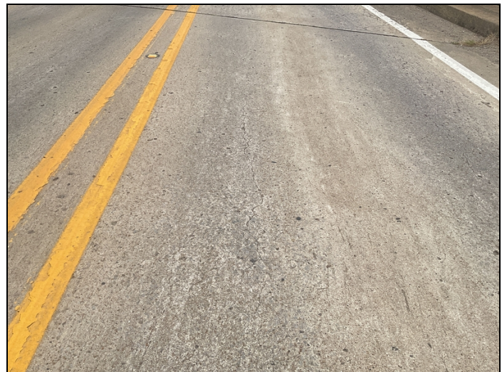
Span # 3 driving surface of right lane has diagonal cracks adjacent to bent # 3 and a longitudinal crack near the centerline.
