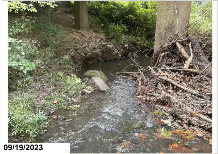
Heavy drift accumulation causing embankment erosion to East embankment.
