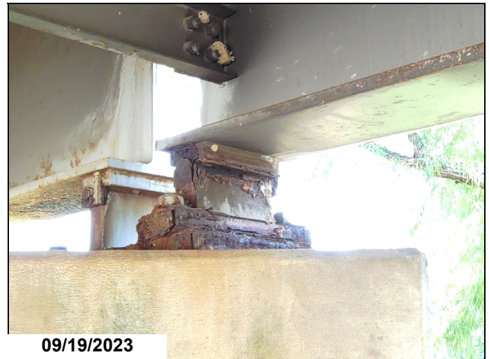
Drone Photo-Heavy corrosion to bearings.
