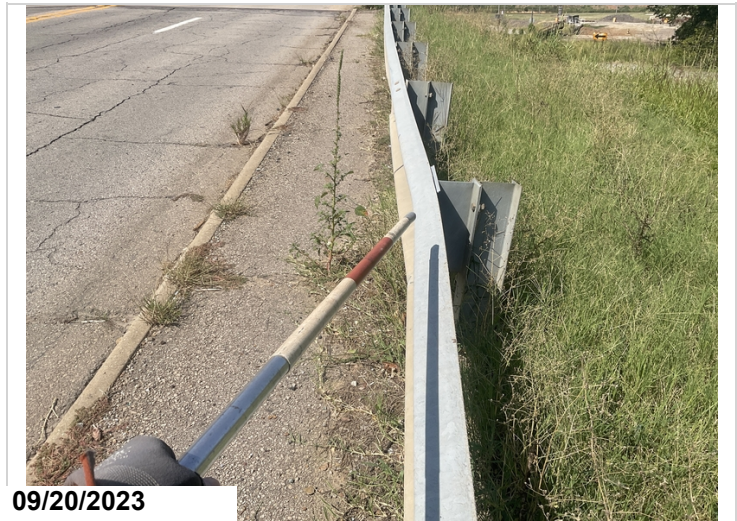
Abutment 2 left approach railing-Collision damage
