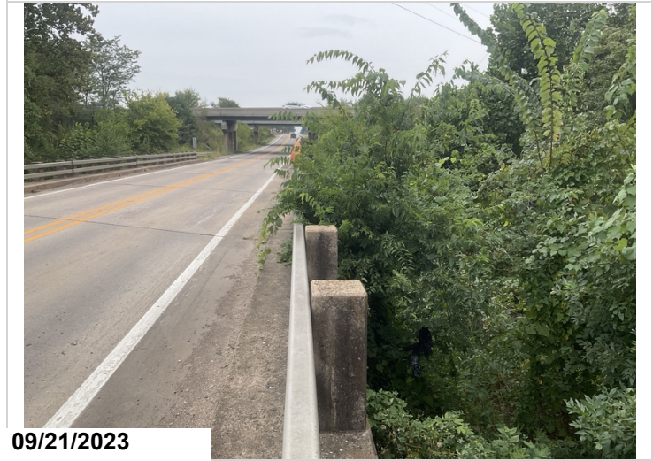
Vegetation growing over right bridge railing
