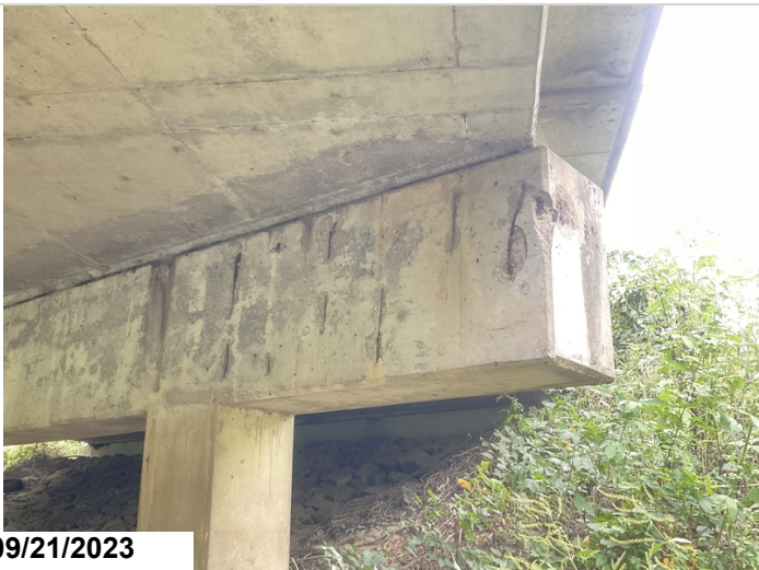
Bent # 2 cap aheadface on left side has numerous shallow spalls with exposed reinforcing steel.
