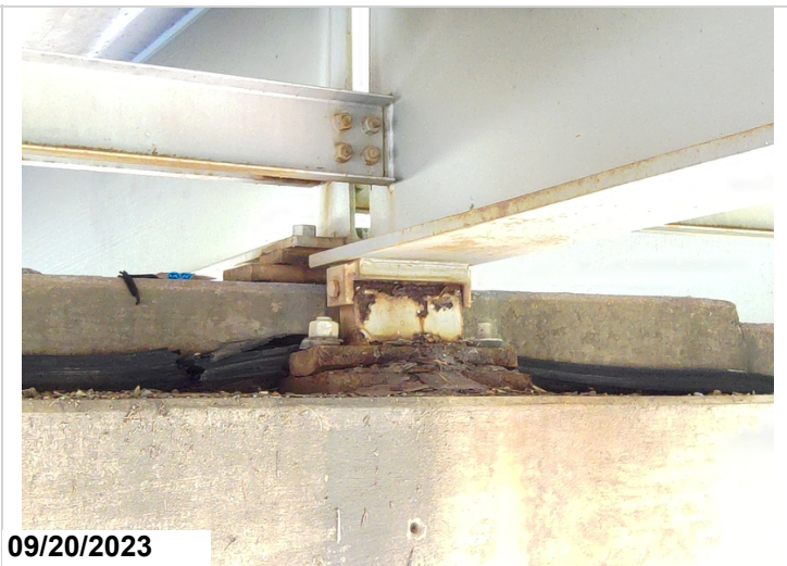
Drone Photo-Heavy corrosion
