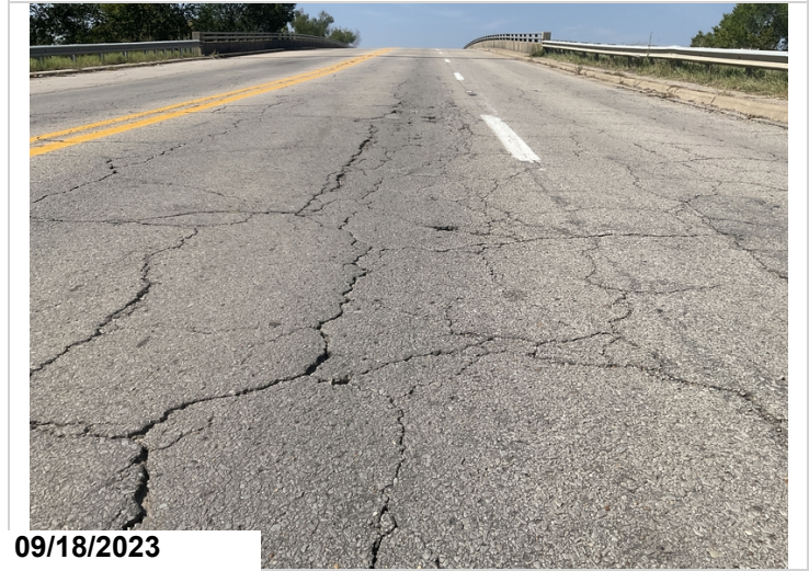
East approach roadway has rutting in the Eastbound lanes with potholes forming.
