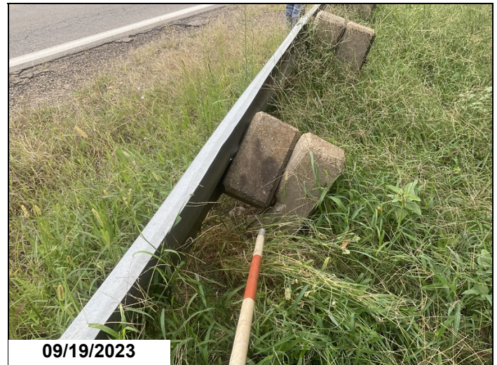
Abutment # 1 right approach railing-Collision damage.
