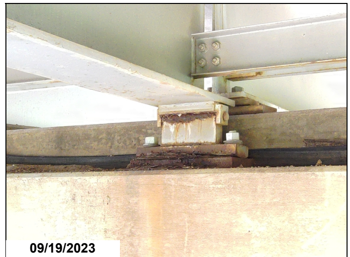
Drone Photo-Corrosion with pack rust between bearing plates.
