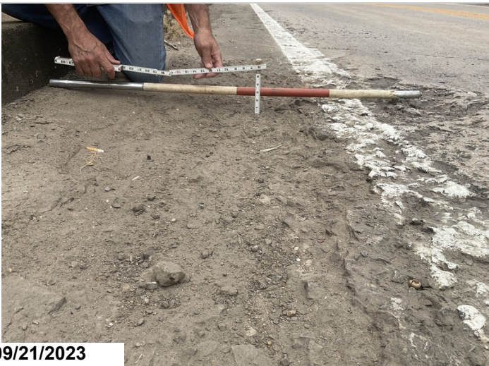
Span # 5, right shoulder has heavy scaling up to approximately 2" deep
