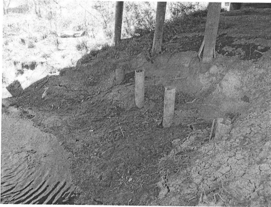
Figure 1. Up-station stream bank under the bridge
