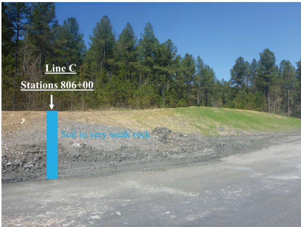
Figure 5.15- Field observation for rock cut for Line C at Station 806+00.
