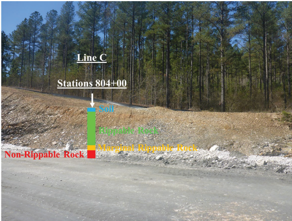
Figure 5.14- Field observation for rock cut for Line C at Station 804+00.
